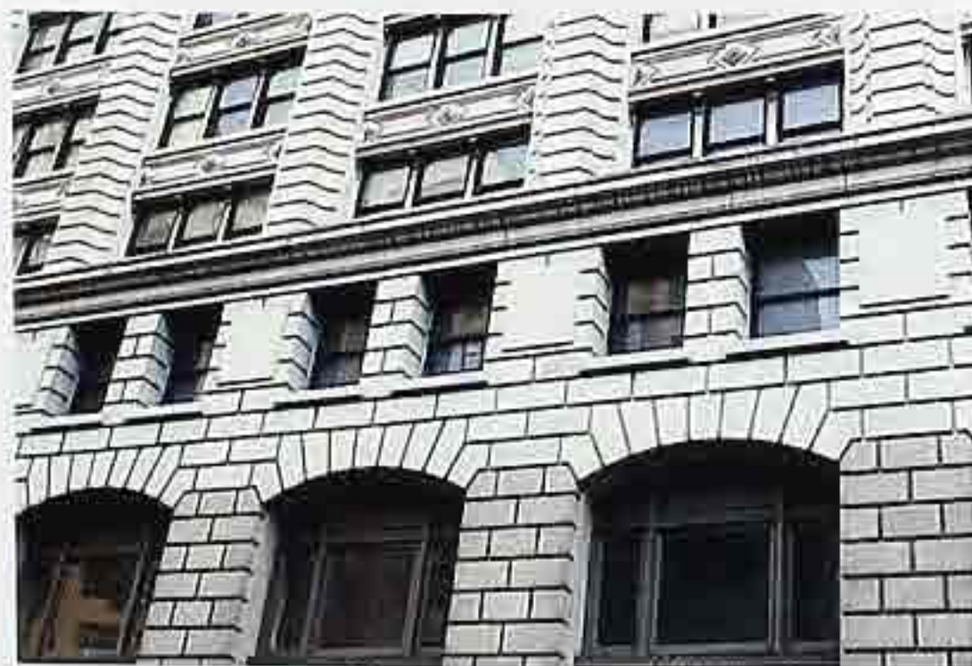
WA-118 Limestone in running bond with cornice; upper story with carved spandrels; varied window openings
