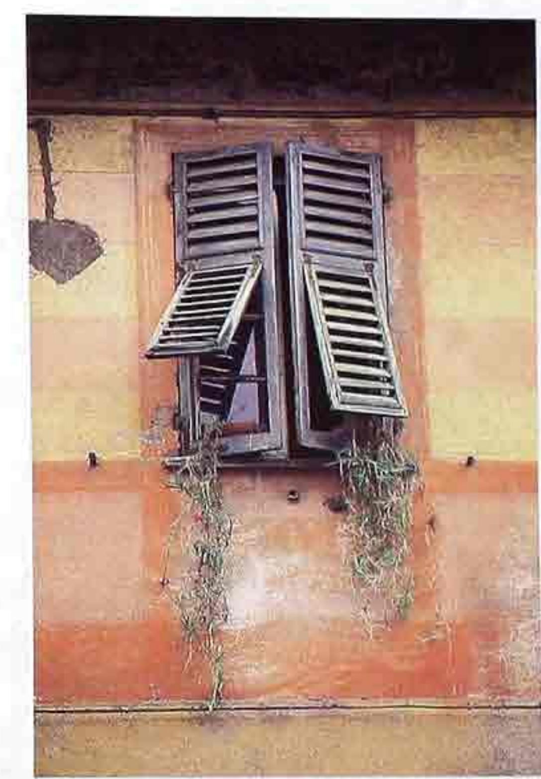
WI-180 Weathered double-hinged louvered shutters
