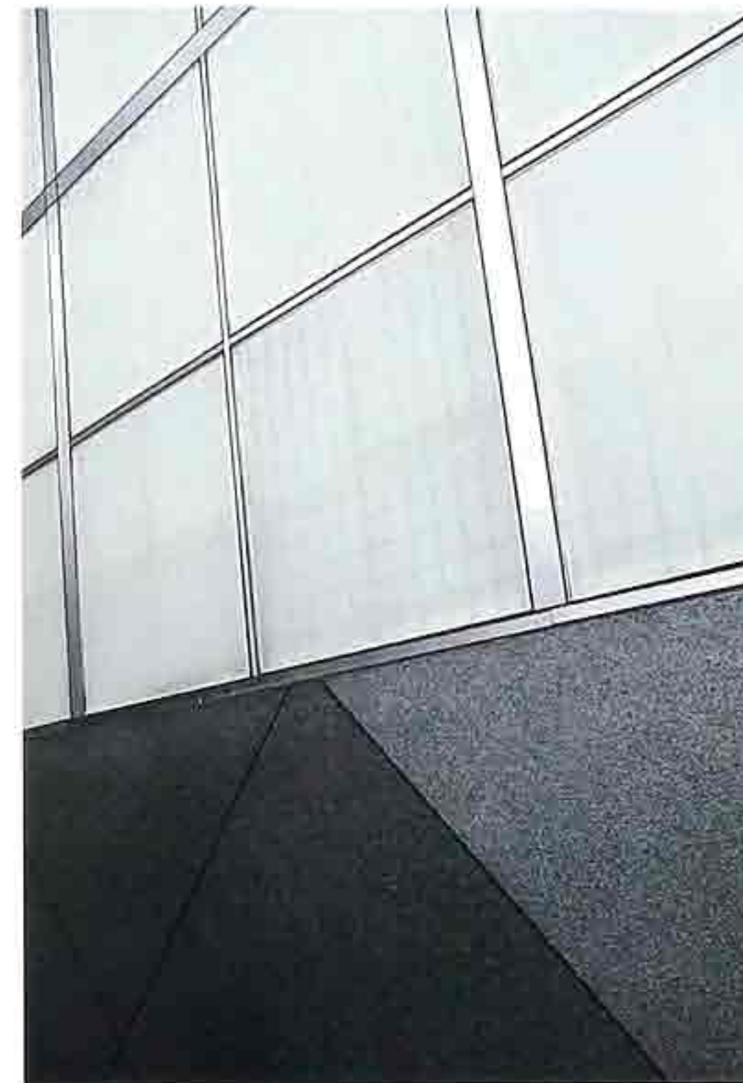
WA-293 Black granite base with metal-and-glass curtain wall, modern commercial building
