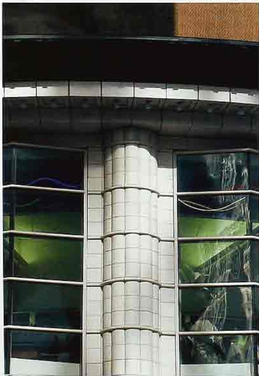
CP-98 Bundled pier on modern commercial building
