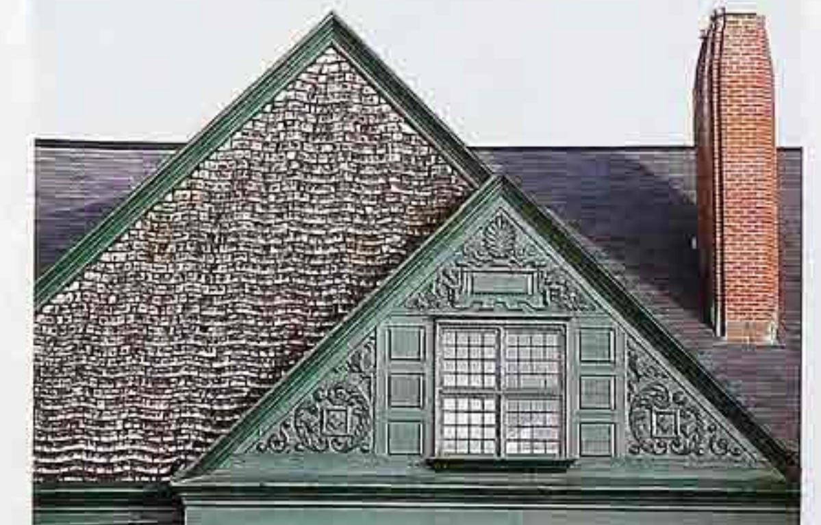
CR-83 Wall dormers. Left: shingle-clad; right: wood with carved ornament, American house
