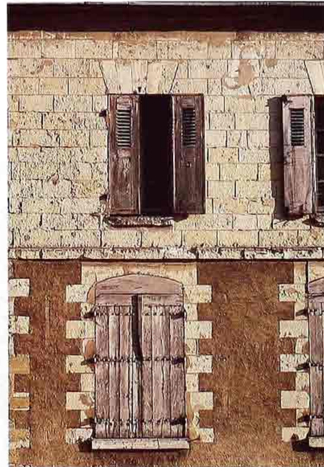
WI-197 Weathered painted wood paneled shutters
