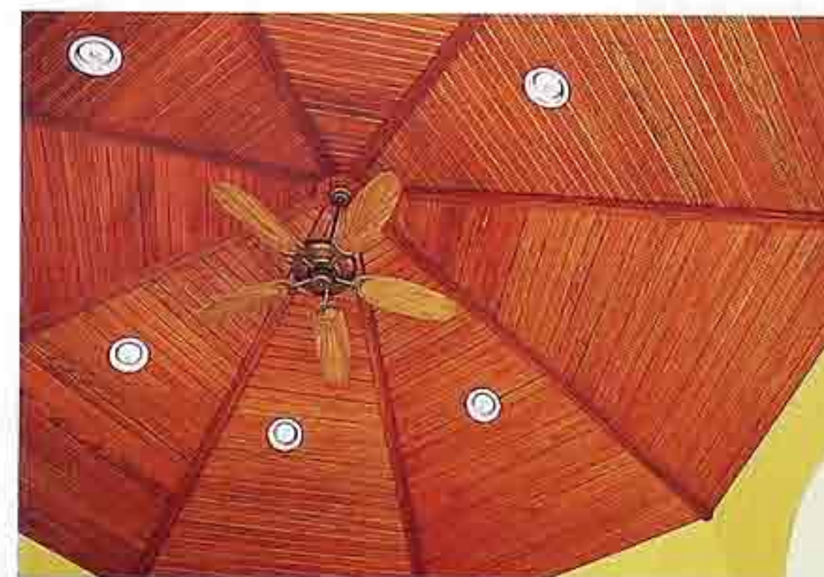
CR-7 Octagonal tongue-and-groove pool-house ceiling, modern house
