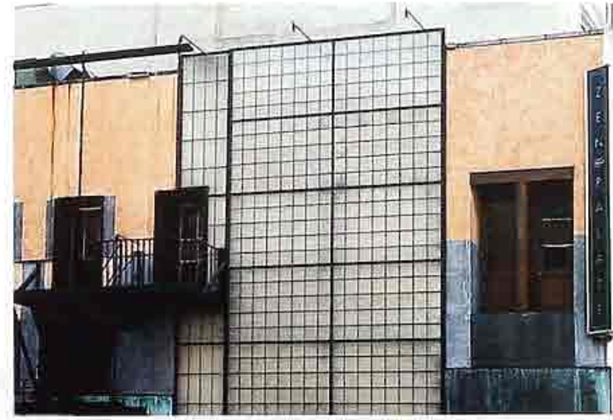
WA-298 Metal-framed glass panels with colored and patinated metal, modern commercial building
