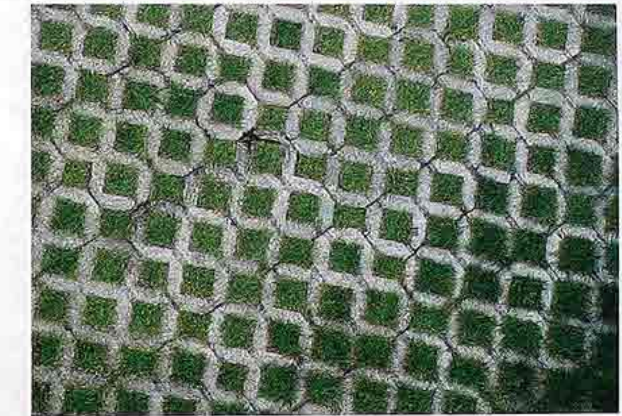
FP-88 Concrete screen-wall blocks set into the ground and planted with grass in patio
