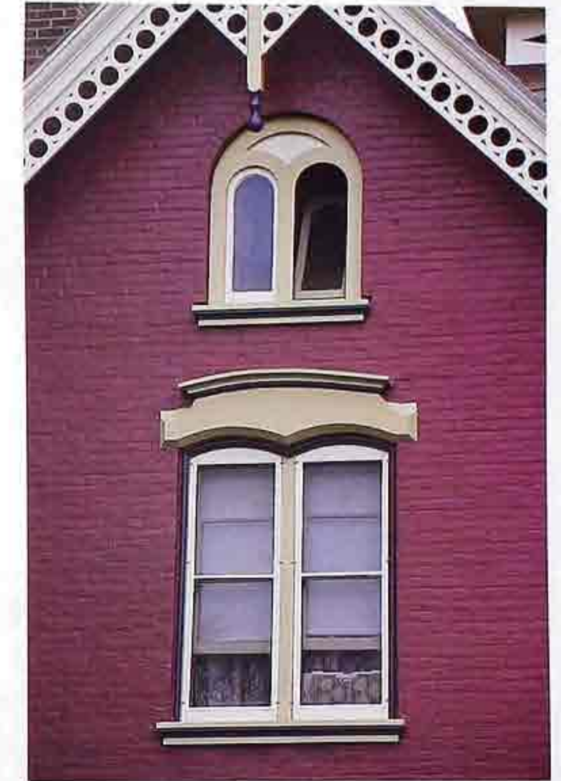
WI-108 Flat trim echoing arch profiles of window openings, American brick house
