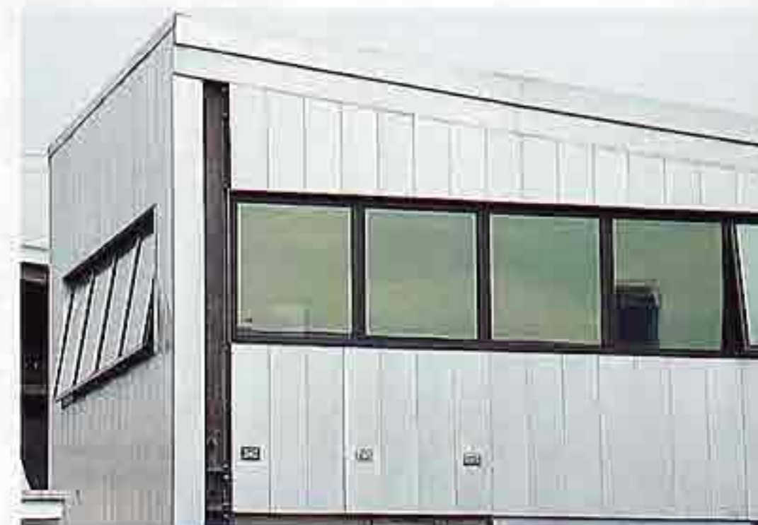
WI-43 Awning windows, modern metal-clad house
