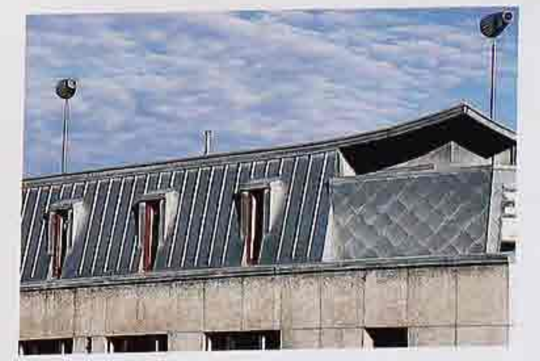
CR-104 Shed-roof dormers on gambrel roof
