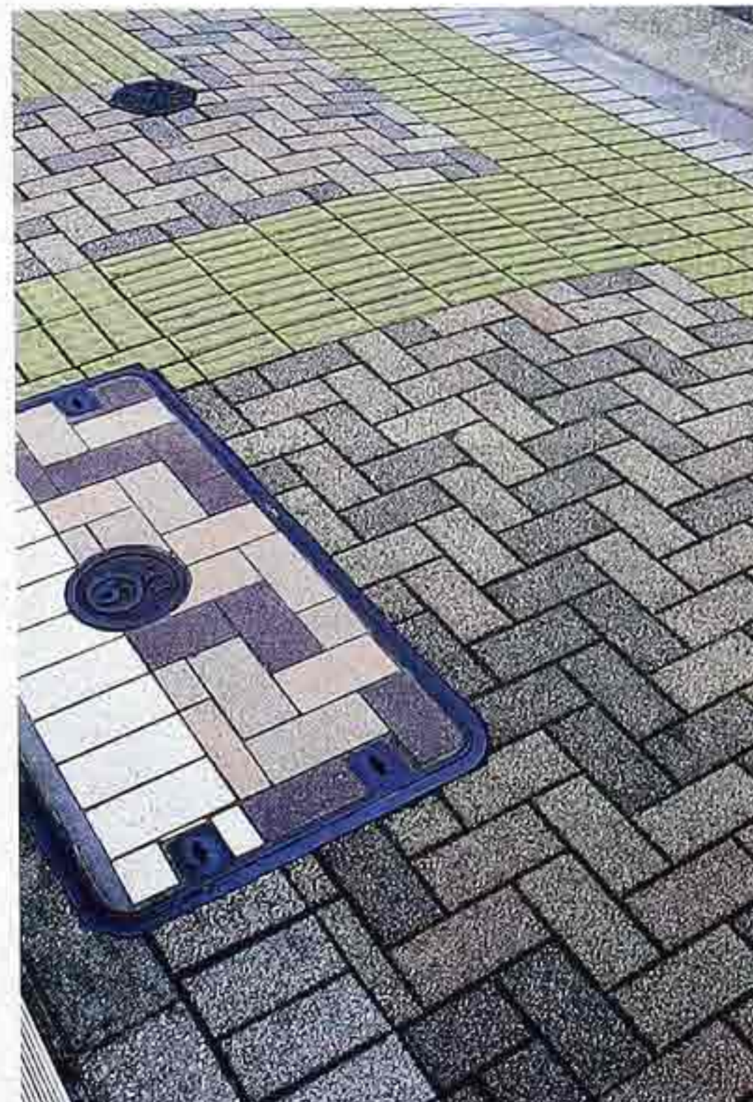
FP-84 Polychrome pre-cast concrete pavers in herringbone and banded patterns, urban street
