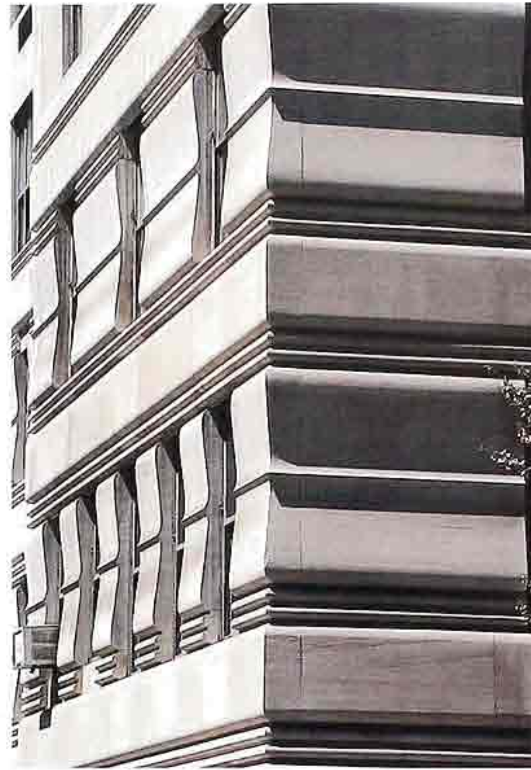
WA-98 Outside corner probably of Amherst gray limestone, sand-finished in shaped panels
