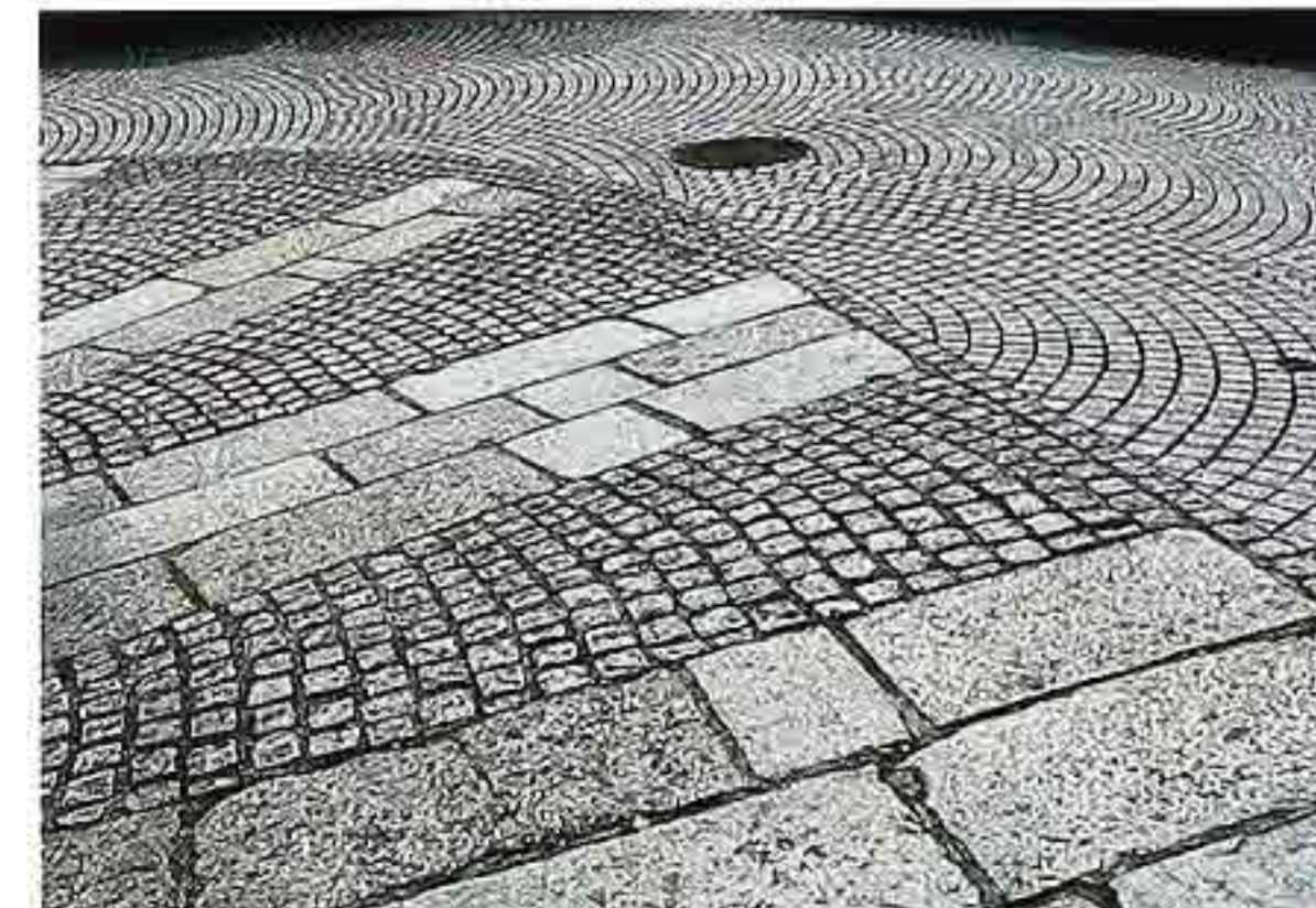
FP-25 Squared and roughly squared textured paving stones on curved walkway, urban public space
