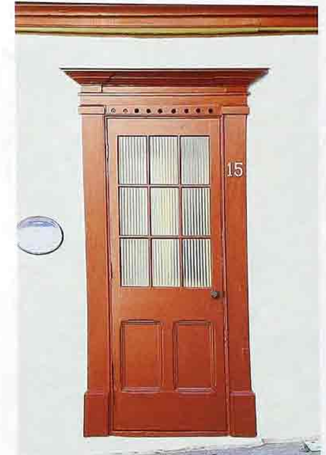
DW-20 Painted wood door; ribbed-glass panel with nine lights; wood panels flush-molded; pilaster frame
