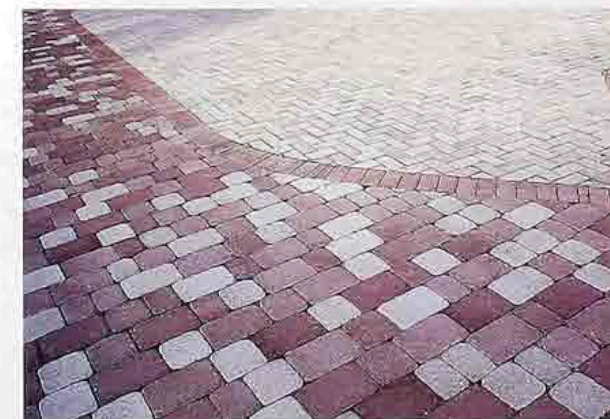
FP-89 Flexible paving: concrete pavers in herringbone pattern (top), with border course; tumbled random-size concrete pavers in running bond (bottom), urban public space
