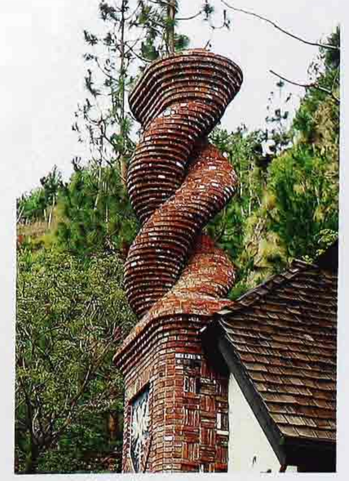
CR-154 Spiral brick chimney pot
