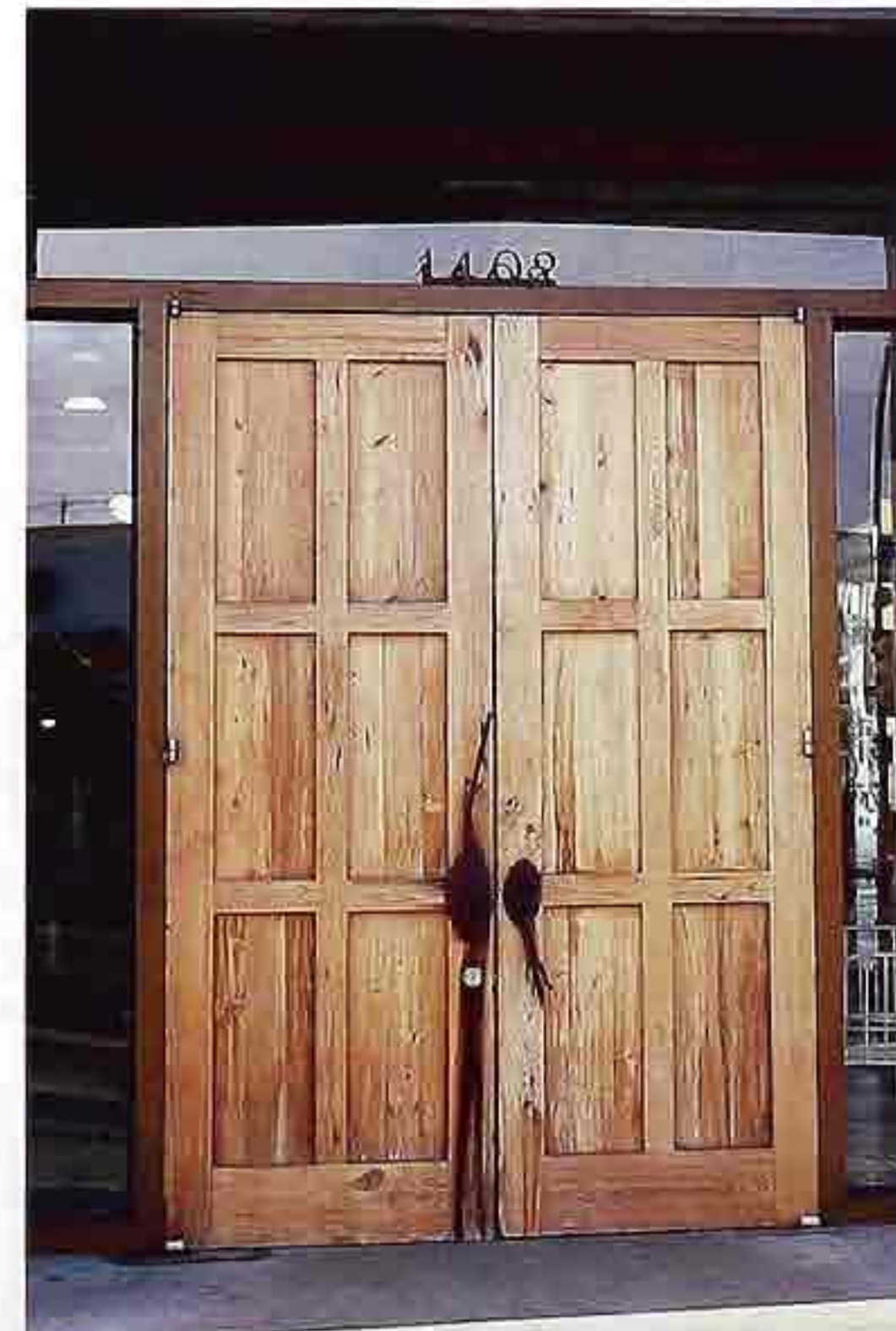
DW-7 Six panels, unfinished wood double doors with planked panels and wrought-iron handles; metal door-frame with transom light and side lights
