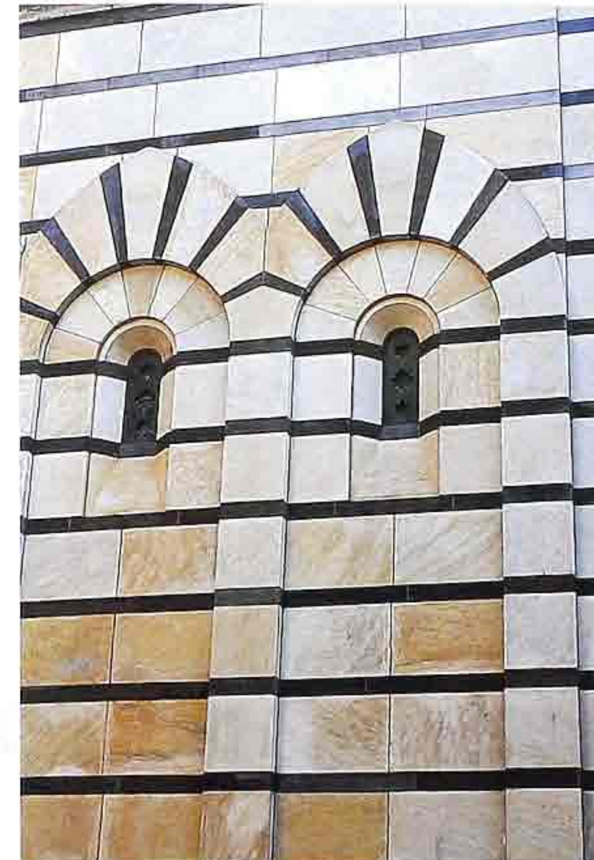
WA-120 Alternating polychrome bands of marble veneer in stack and running bonds with Moorish blind arches with recessed windows
