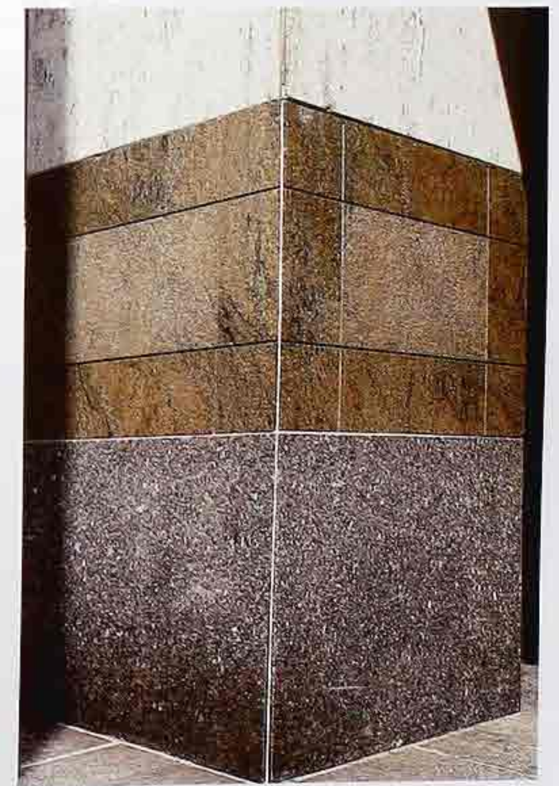
CP-48 Banded stone-veneer pier on base, grouted corner and joints, modern commercial building
