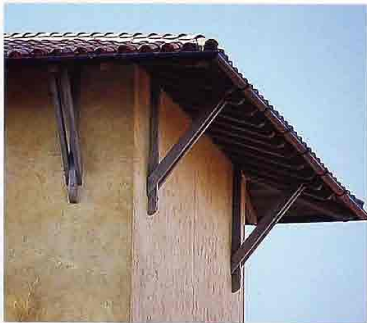
CR-107 Wood eave brackets supporting mission-tile hipped roof, American Southwestern mission-style house
