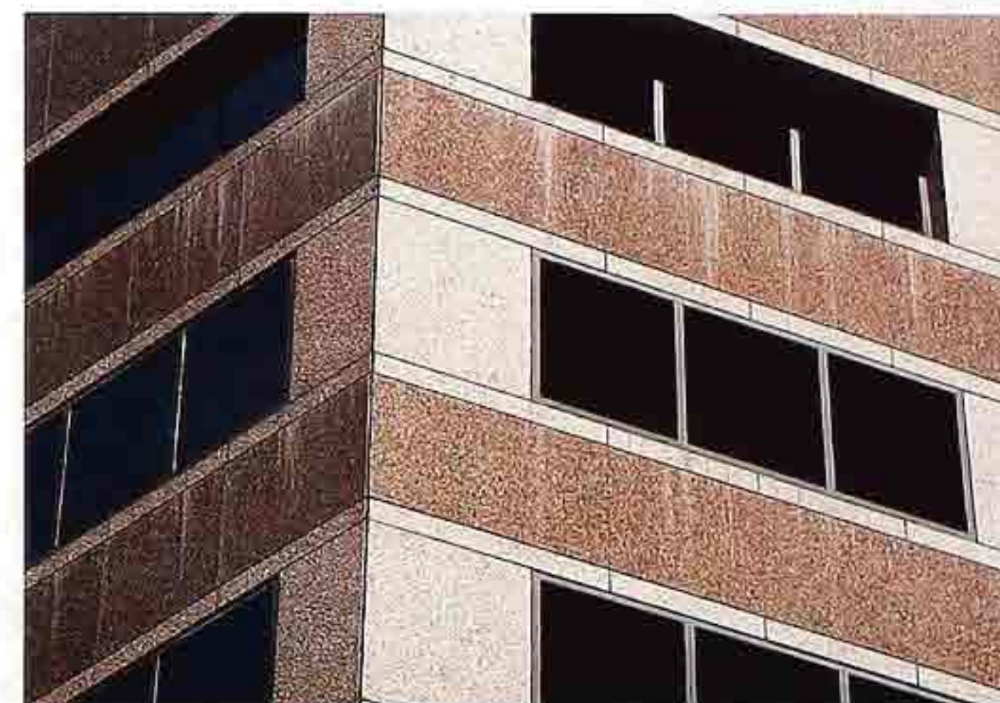
WA-136 Banded polished-granite-veneer spandrels alternating with honed granite and ribbon windows, modern commercial building
