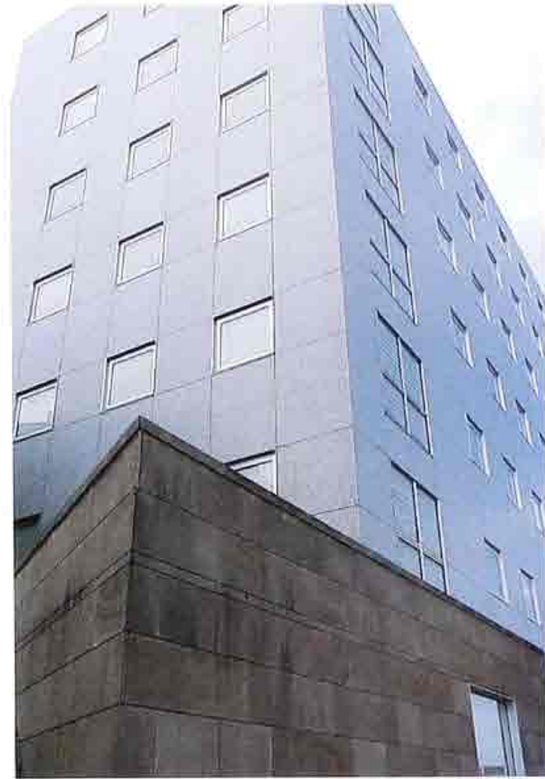
WA-307 Stone-veneered lower story and tile-clad upper stories, modern commercial building
