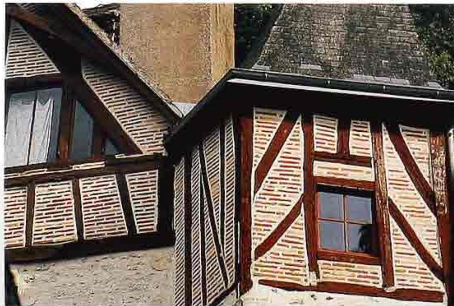
WA-277 Half-timbering with brick infill (top) and stucco (bottom), 17th-c. French house
