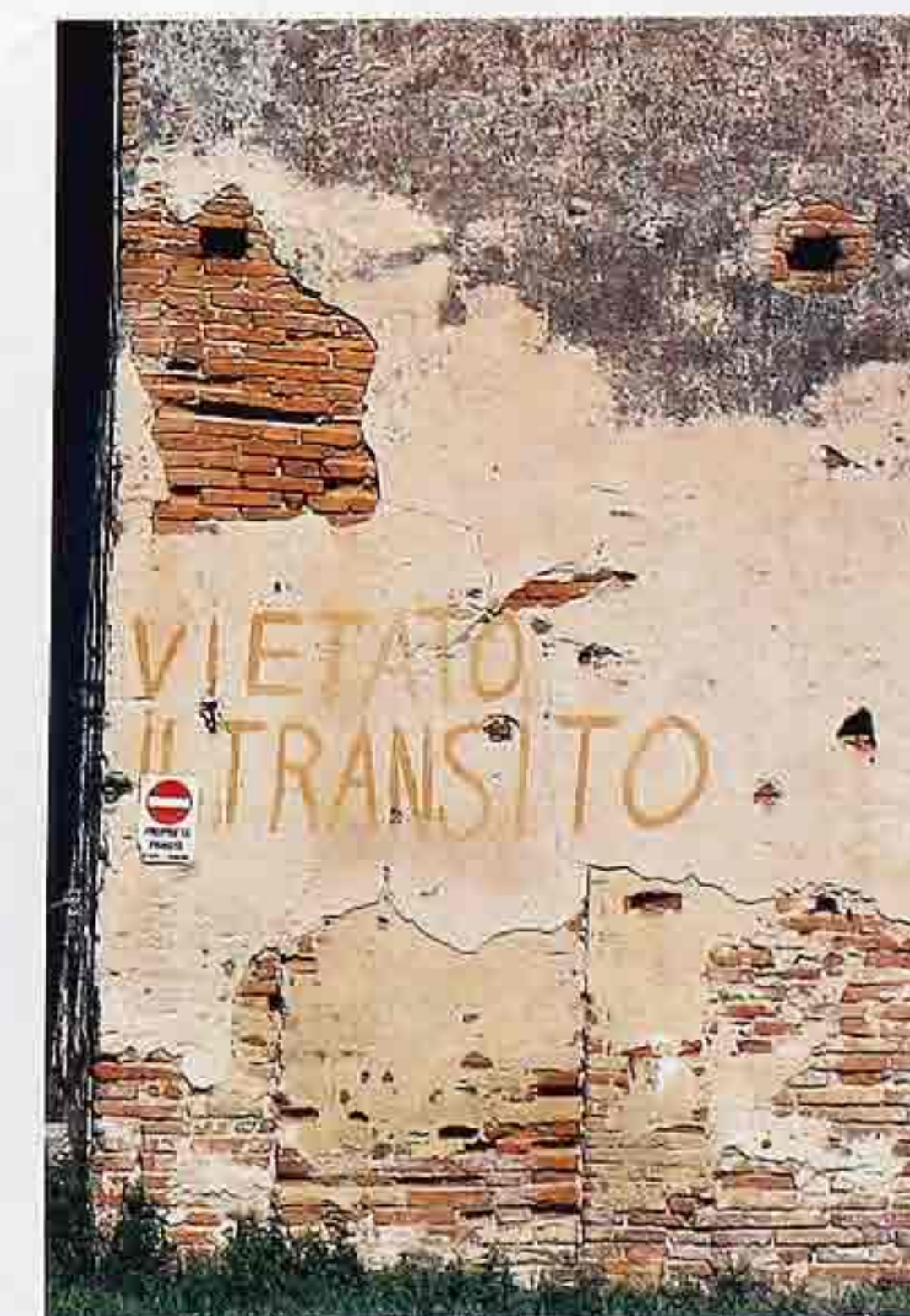
WA-263 Weathered stucco with concrete patches, graffiti, and exposed structural brick and stone
