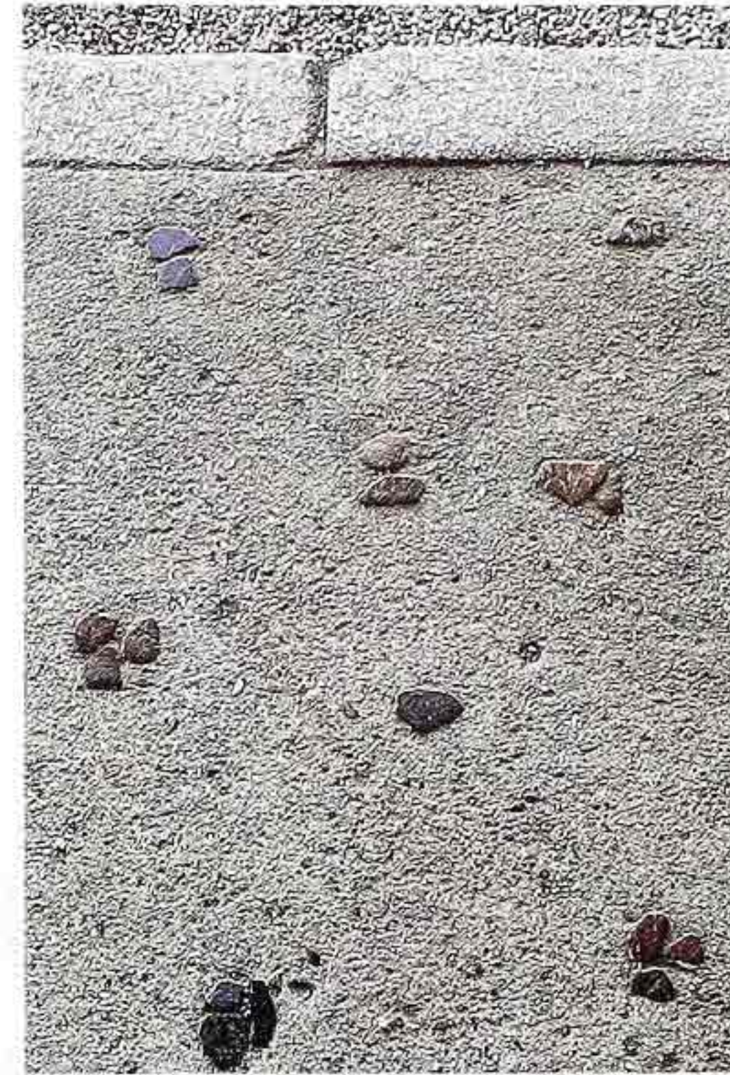
FP-68 Pebbles set in concrete in diaper pattern with stone border
