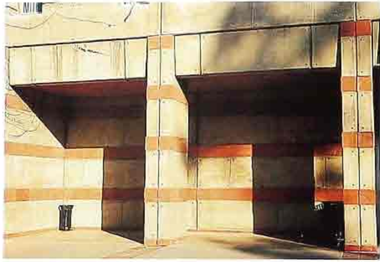
WA-212 Polychrome banded cast concrete, modern commercial building
