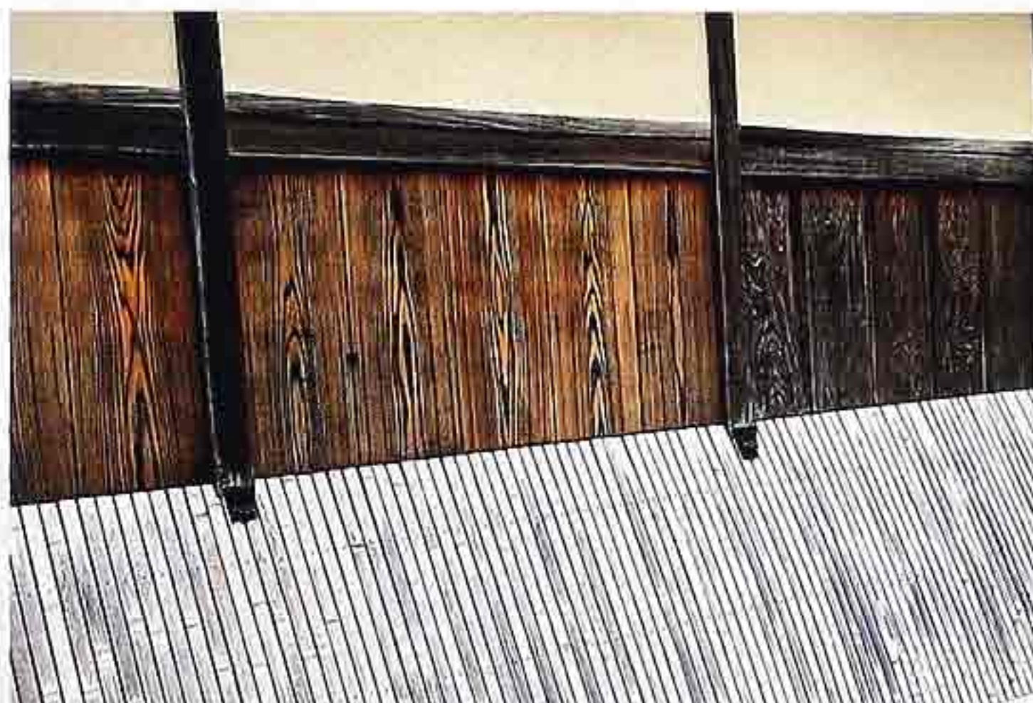
WA-45 Timber-frame with plain-sawn planks and split-bamboo removable fence
