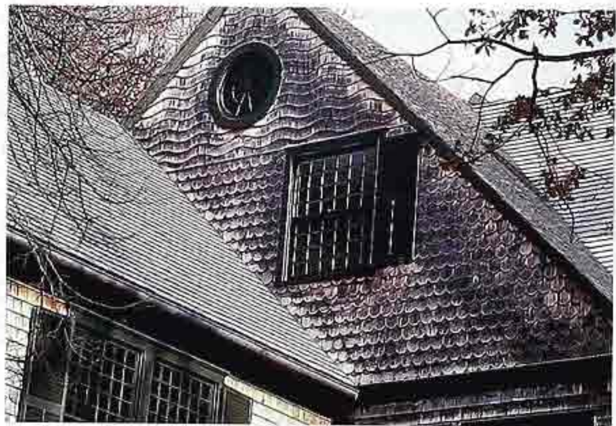
FA-50 Cut shingles on gable. Top: wave pattern around bull's-eye window; bottom: fish-scale pattern
