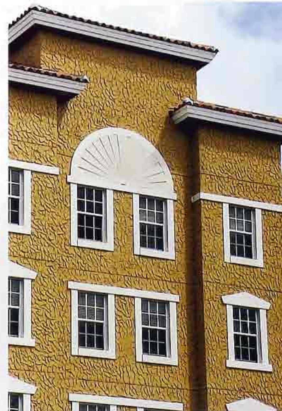
WA-246 Colored stucco with knocked-down skip-trowel finish on wall; double hung windows, Italian-villa-style modern apartment house
