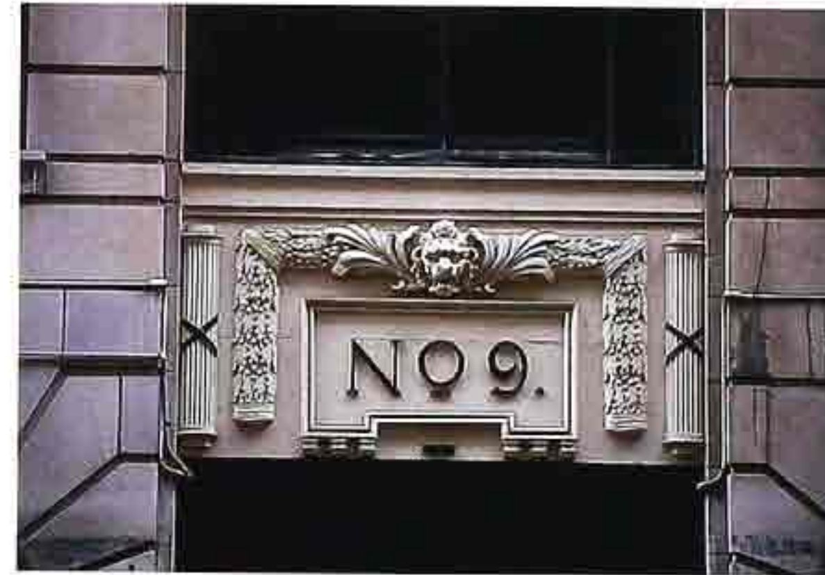
OM-24 Cartouche with building number above guttae, with festoon and center antic
