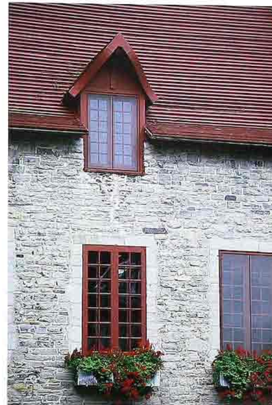
CR-89 Wall dormer on painted wood roof
