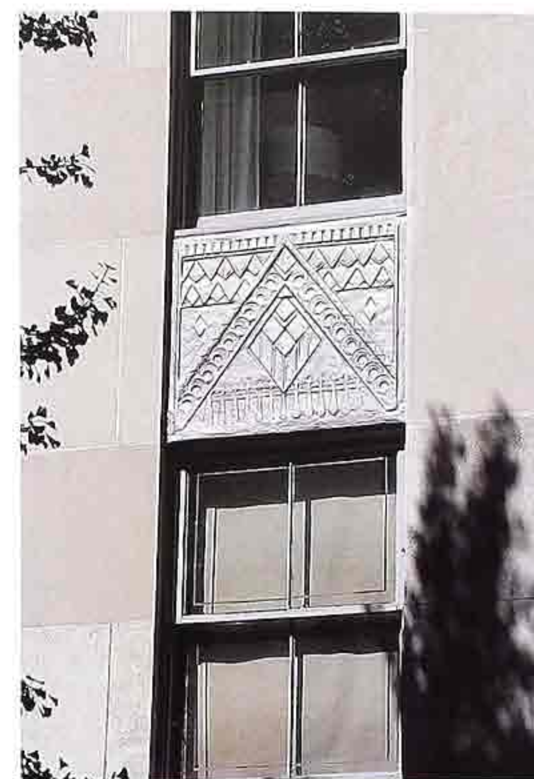
WI-146 Metal spandrel with relief design and metal casings
