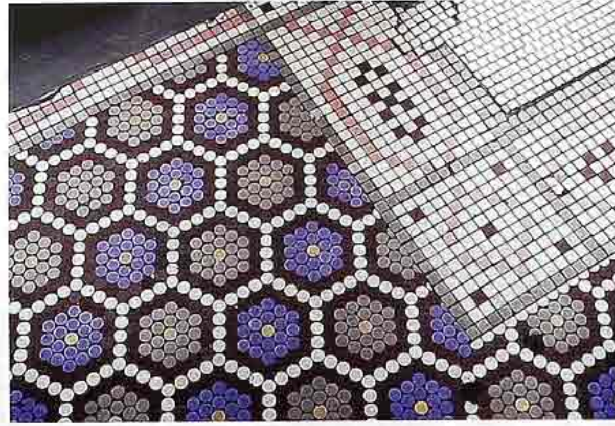
FP-92 Round porcelain tile mosaic in hexagon pattern with square border tiles, commercial entry
