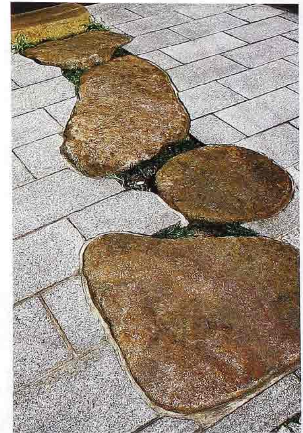
FP-41 Split, polished boulders between squared and textured paving stones in running bond, urban public space
