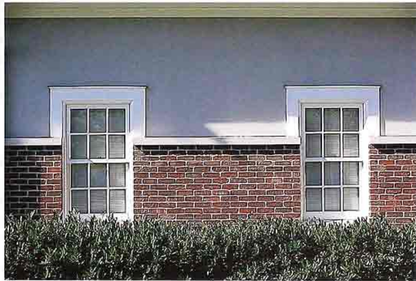
WI-105 Flat wood casing around double-hung windows in stucco and brick wall, traditional house
