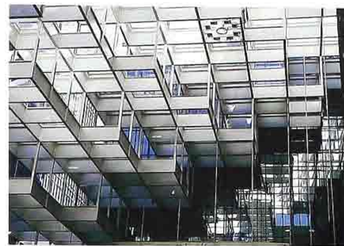
CR-16 Suspended atrium ceiling with interlocking "egg-crate" units, modern commercial building
