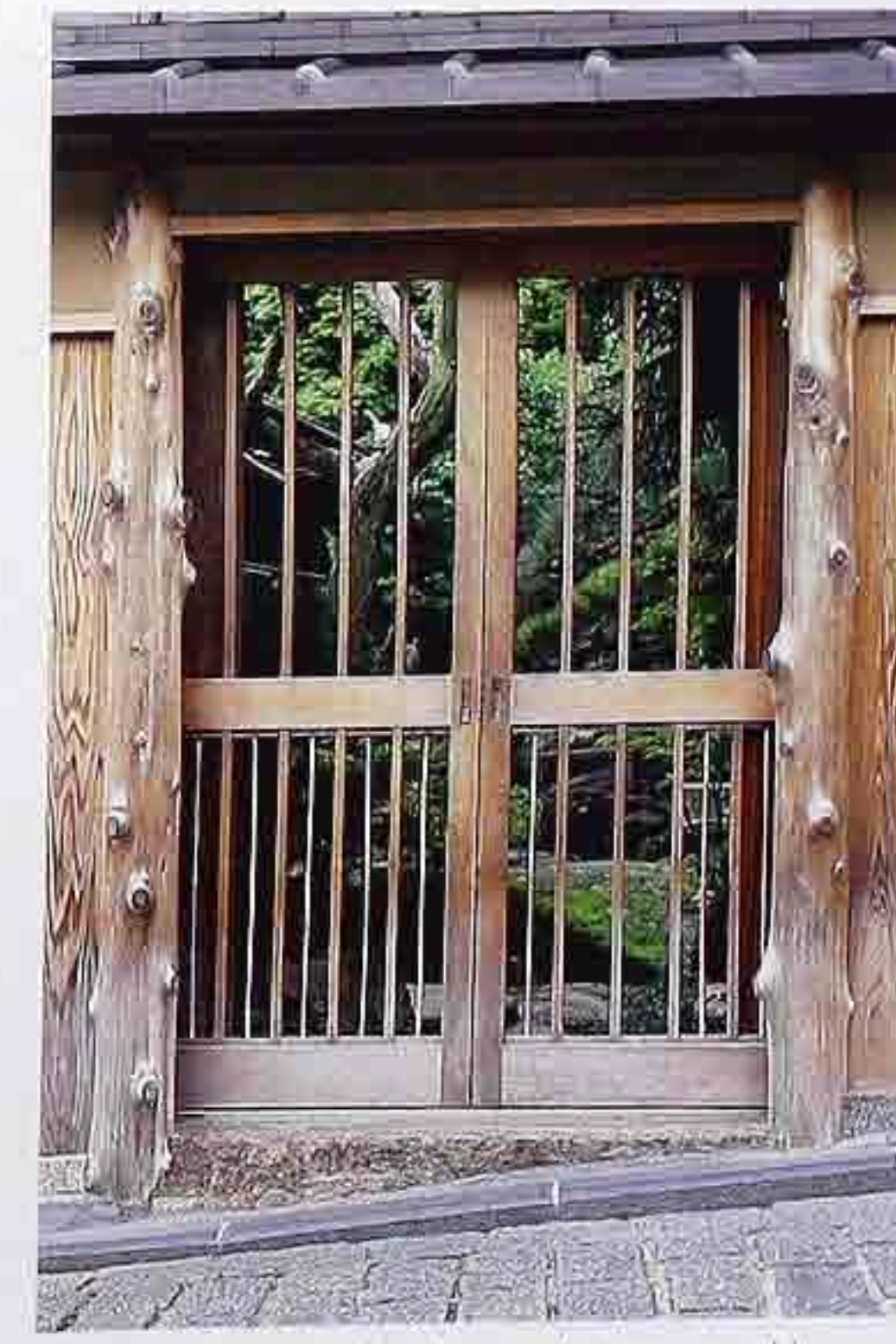
DW-113 Sliding wood-lattice gate between roughly dressed timber posts, entrance to Japanese garden
