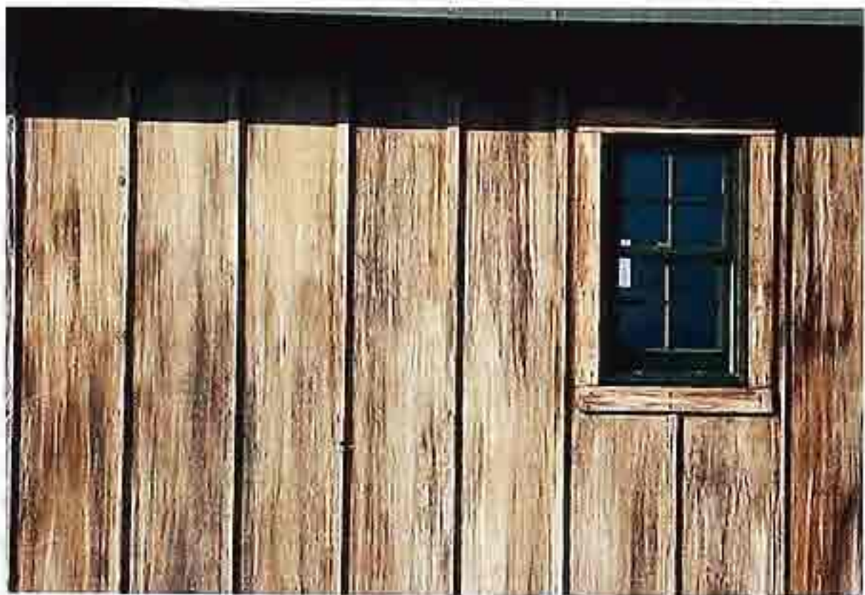
WA-214 Concrete board siding cast with a wood board-and-batten pattern
