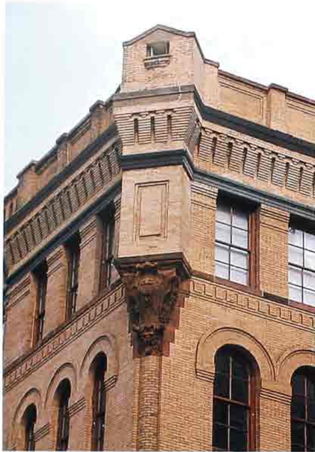
WA-189 Romanesque-style decorative brickwork with ornate corbel on corner below parapet roof
