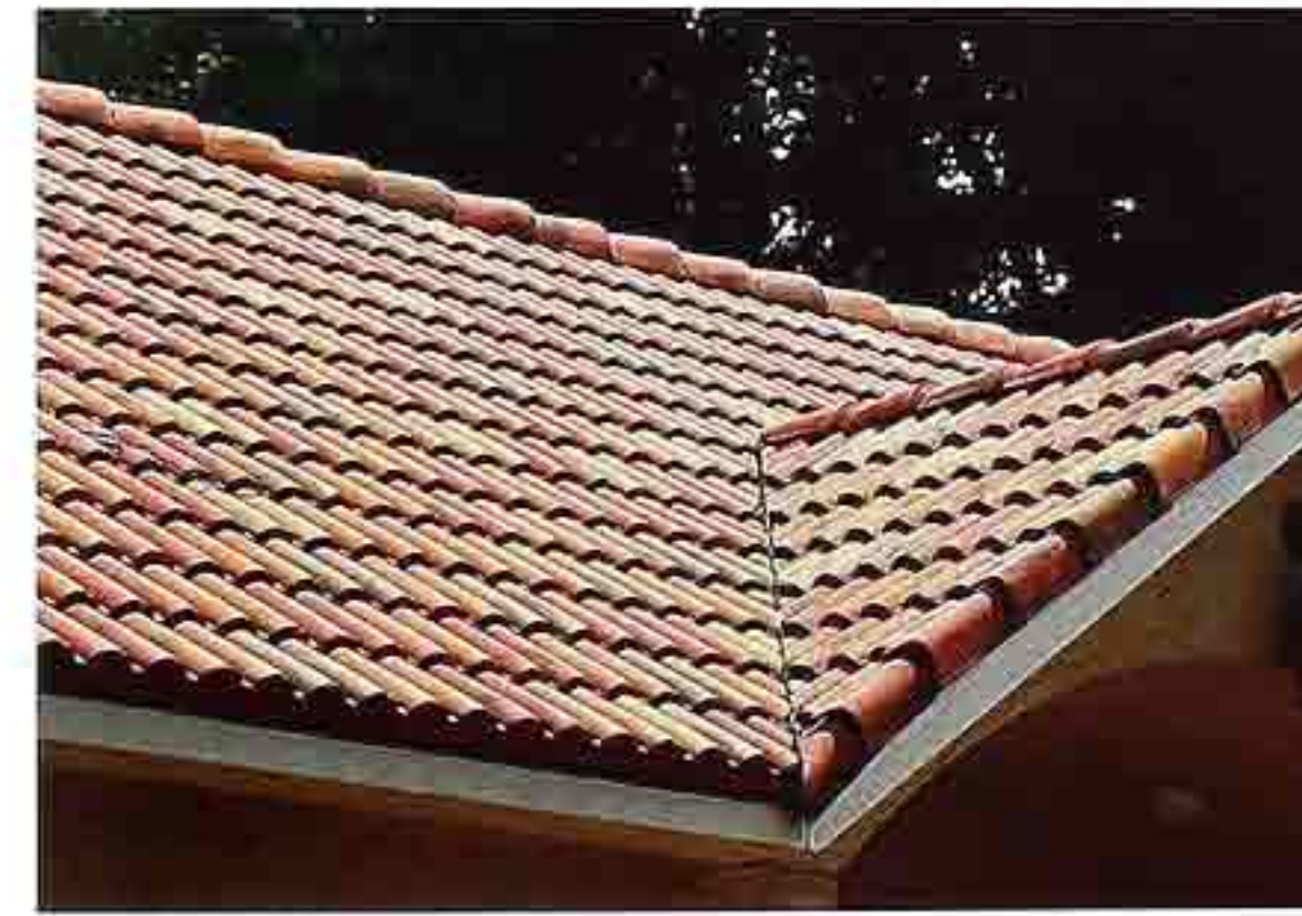
CR-51 Detail of mission tiles at junction of gable and main roof.
