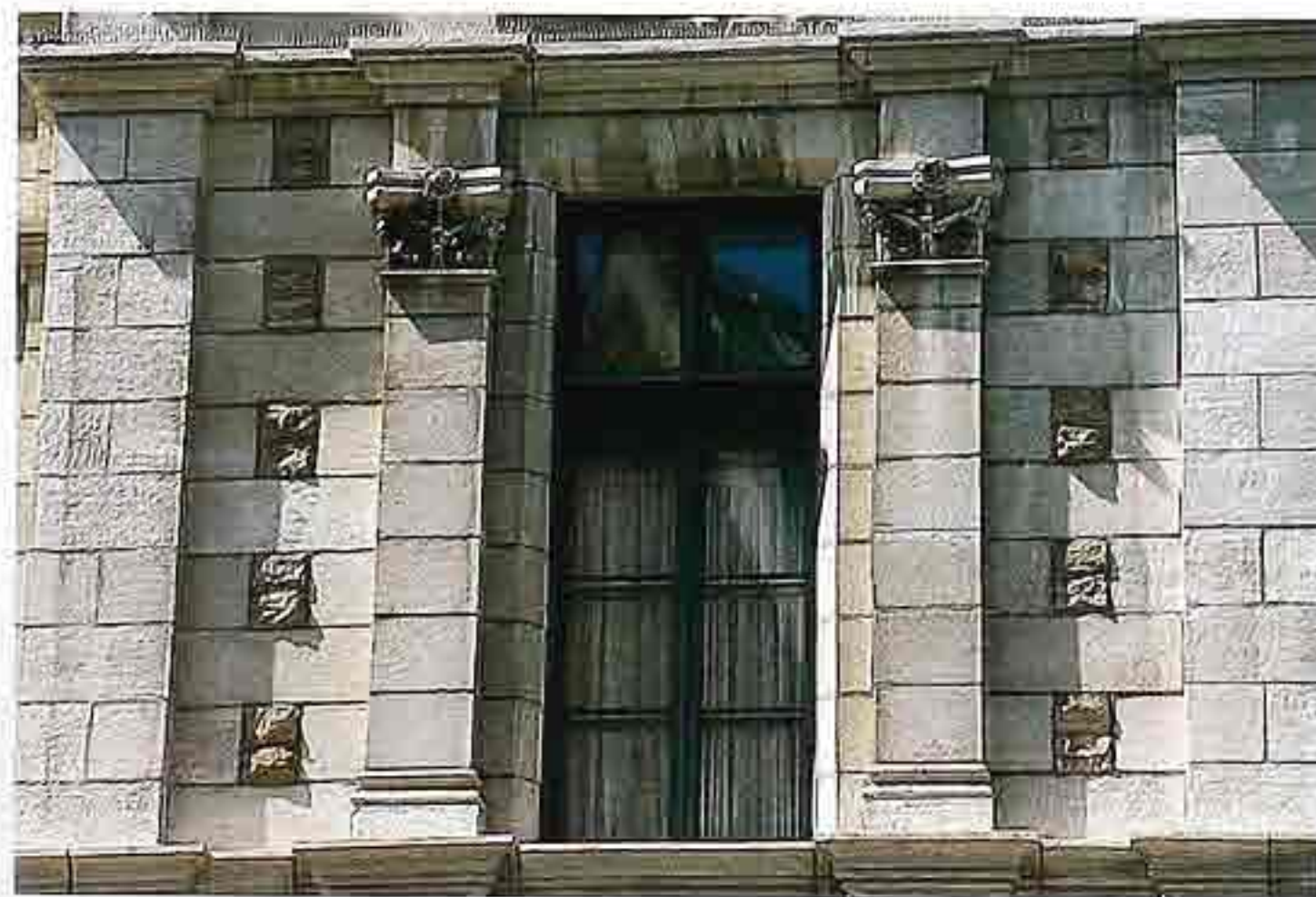
WA-125 Granite in running bond with rustic accents; neo-Corinthian pilasters in stack bond flanking entry
