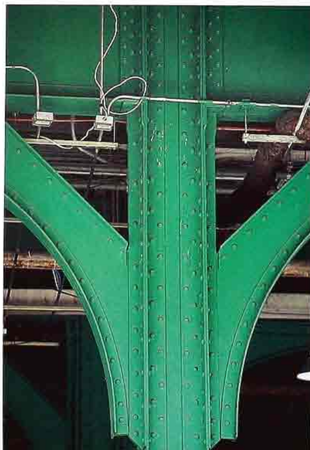
CP-125 Painted steel truss of riveted plates, industrial building
