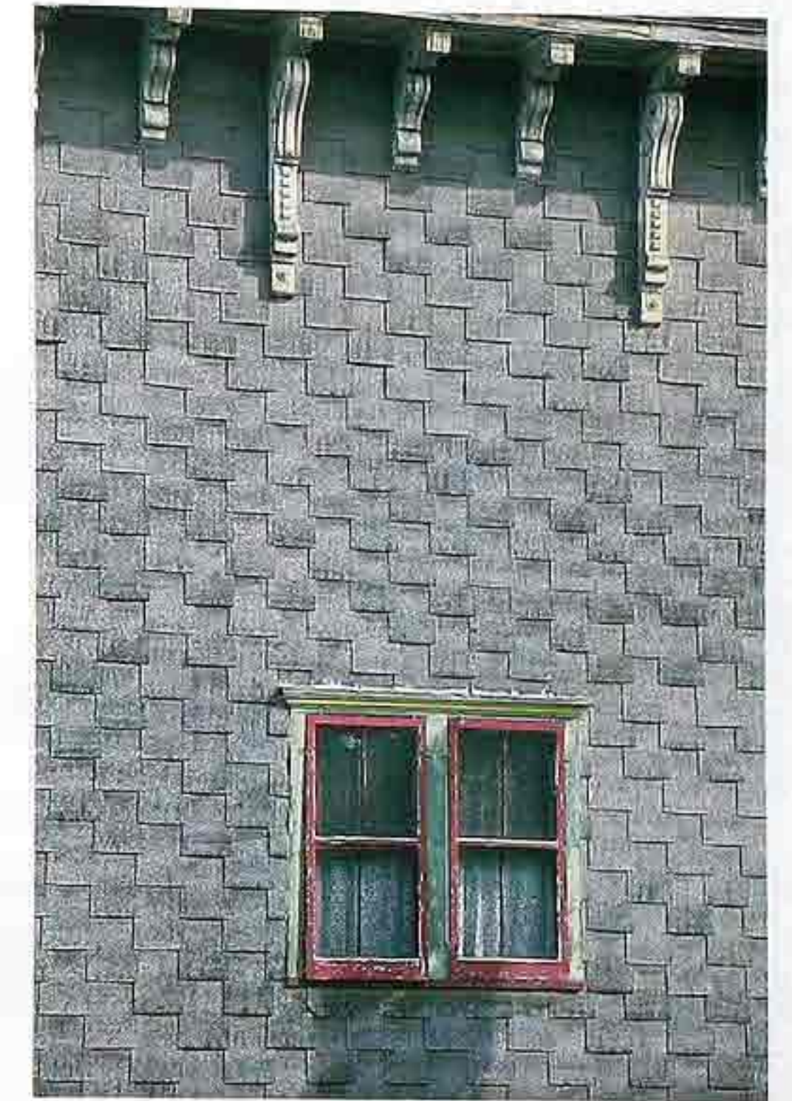
FA-54 Bituminous shingles in staggered course below bracketed cornice
