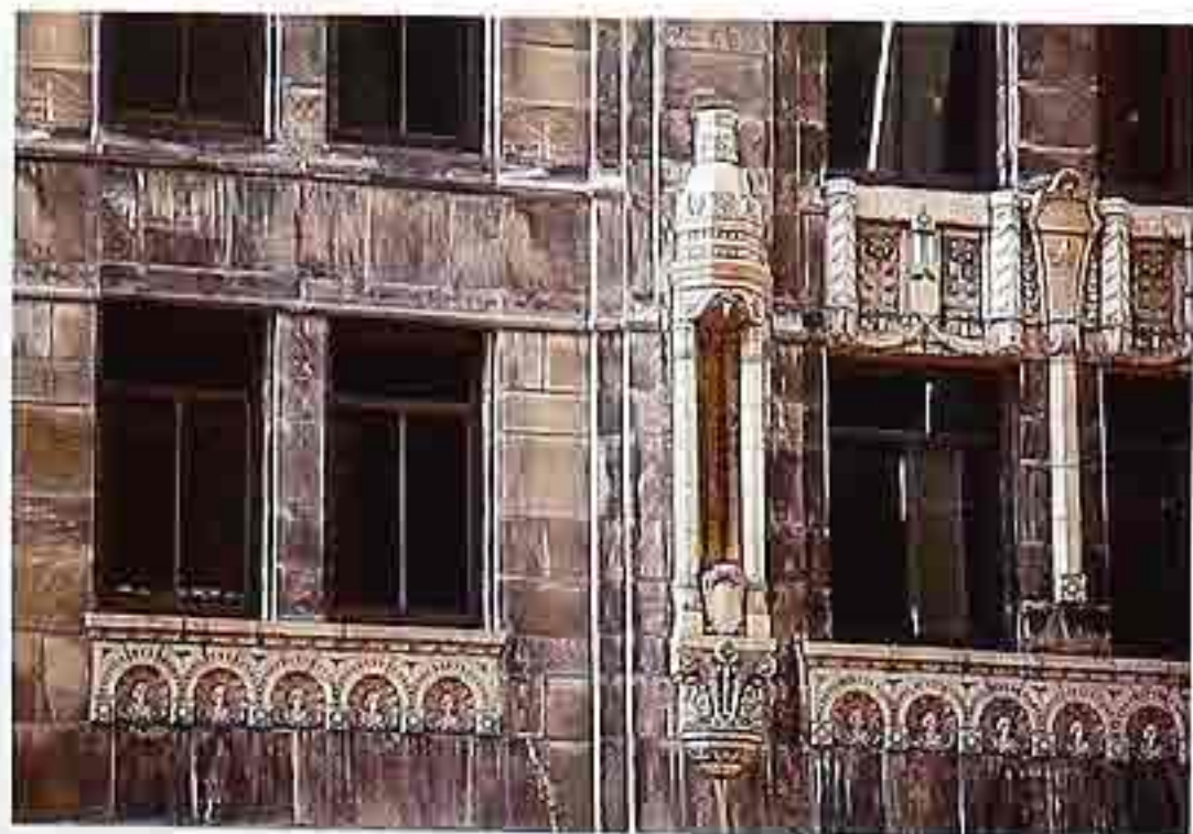
FA-63 Plain masonry facade with architectural terracotta ornament
