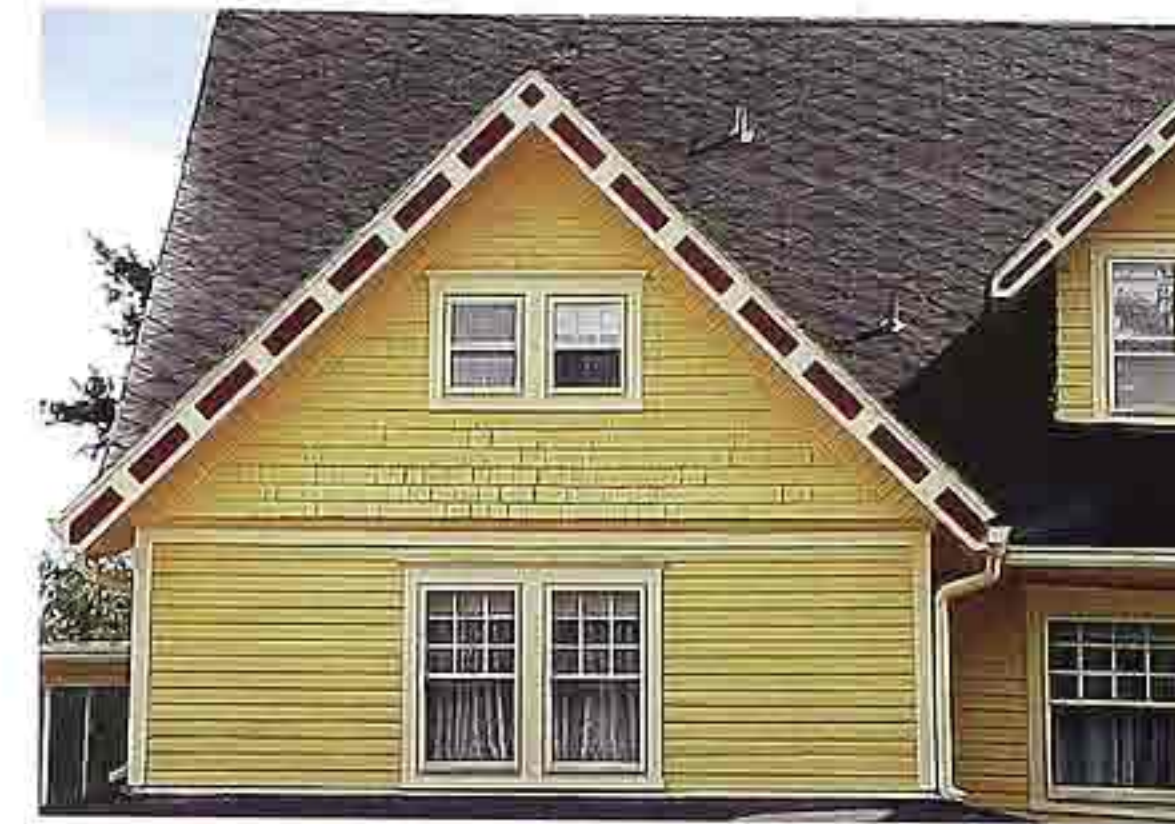
CR-80 Wall dormer with decorated bargeboard, American clapboard and shingle house
