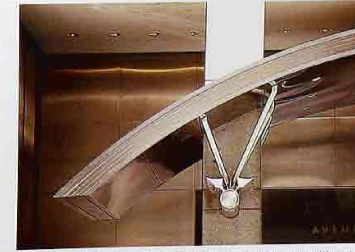
CP-121 Semicircular metal canopy supported by a metal bracket set into a masonry column, modern commercial building
