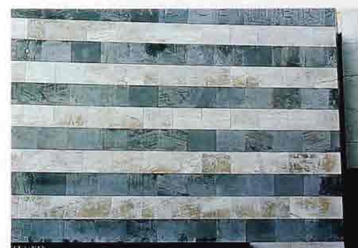
WA-70 Banded white and green marble in running bond, modern commercial building
