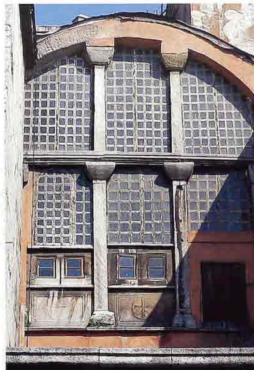
CP-89 Stone pilasters with Byzantine or Romanesque capitals against windowed wall
