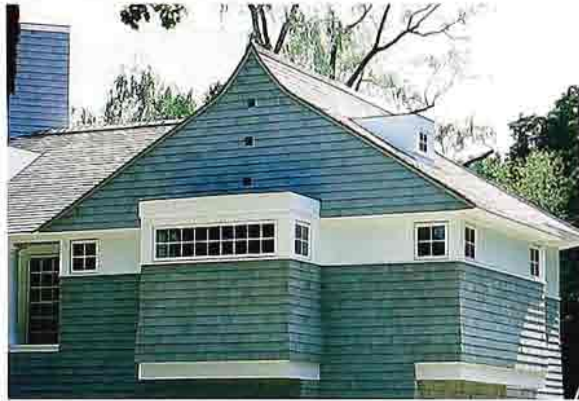
CR-117 Flared-gable shingle roof with shed dormer and shed bay window
