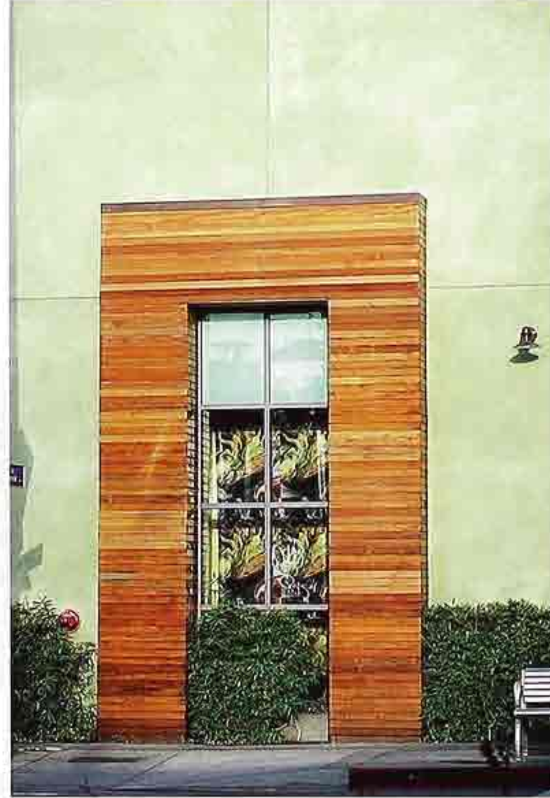
WI-151 Horizontal stacked wood board surround around fixed-light window, modern commercial building
