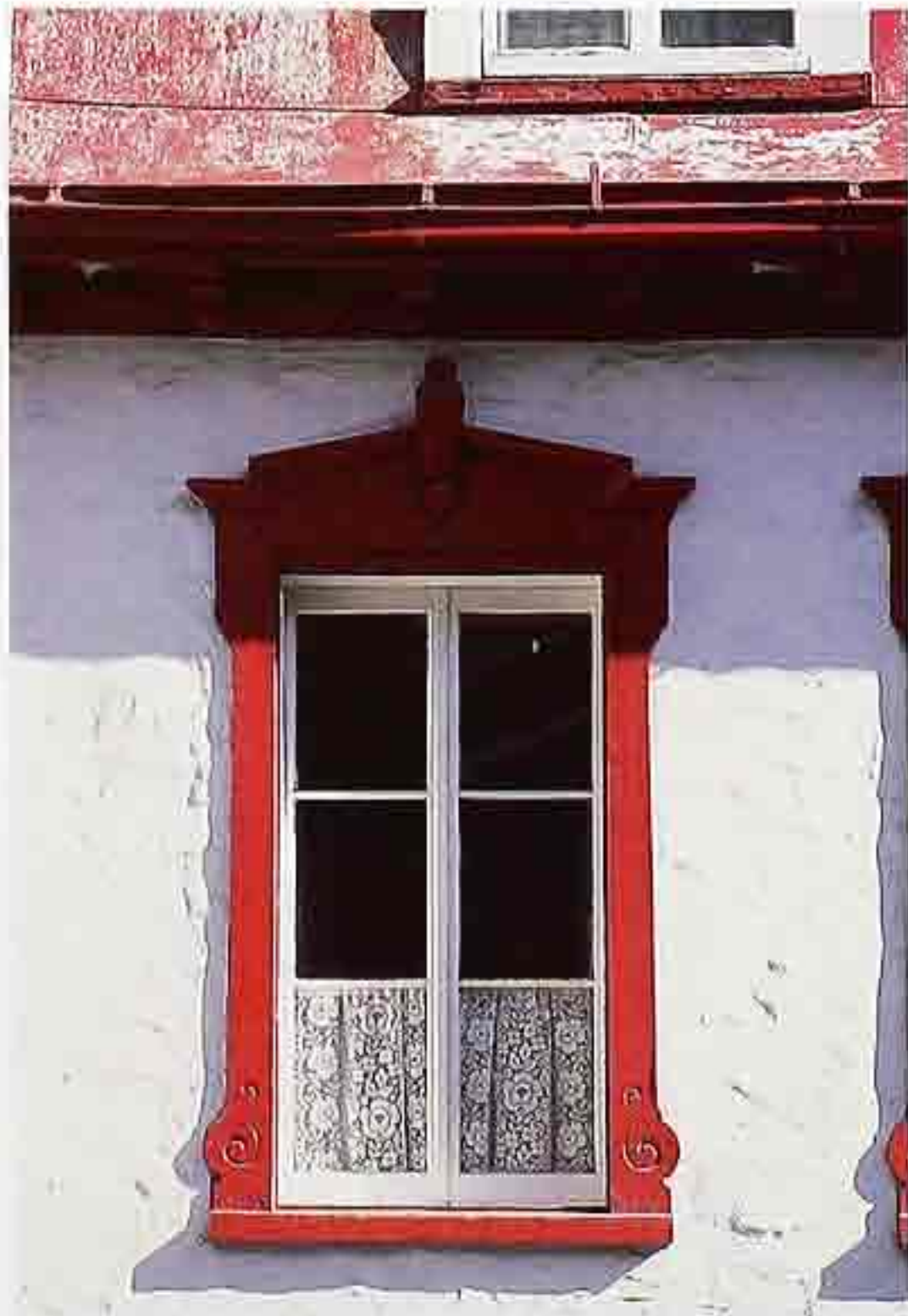
WI-113 Profiled flat casing around double-casement window
