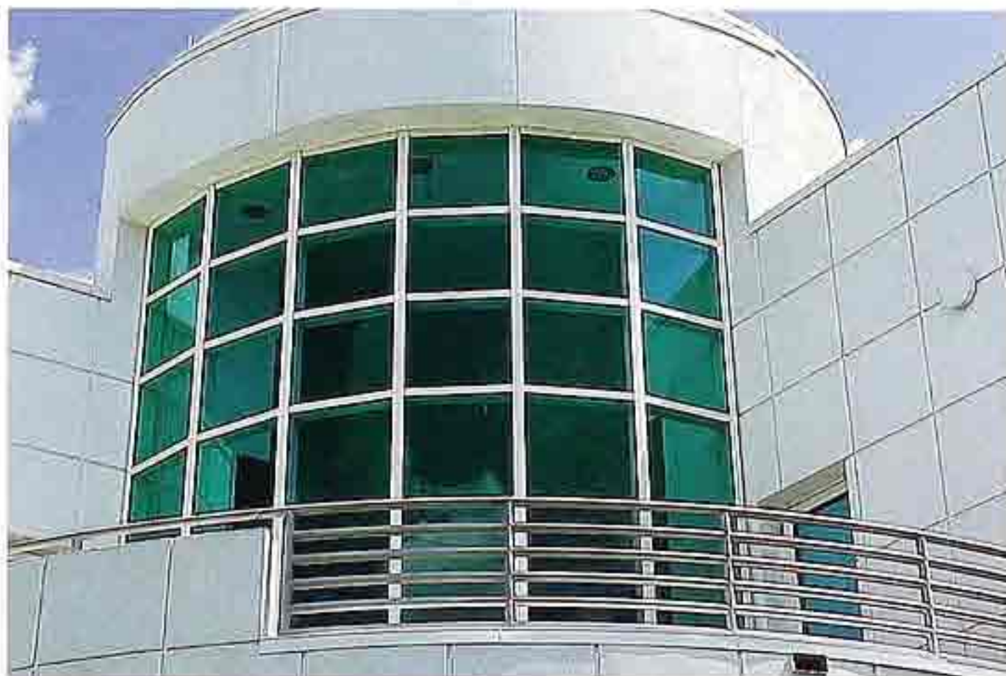
WI-74 Fixed tinted windows in stainless steel frames on curved wall, modern commercial building
