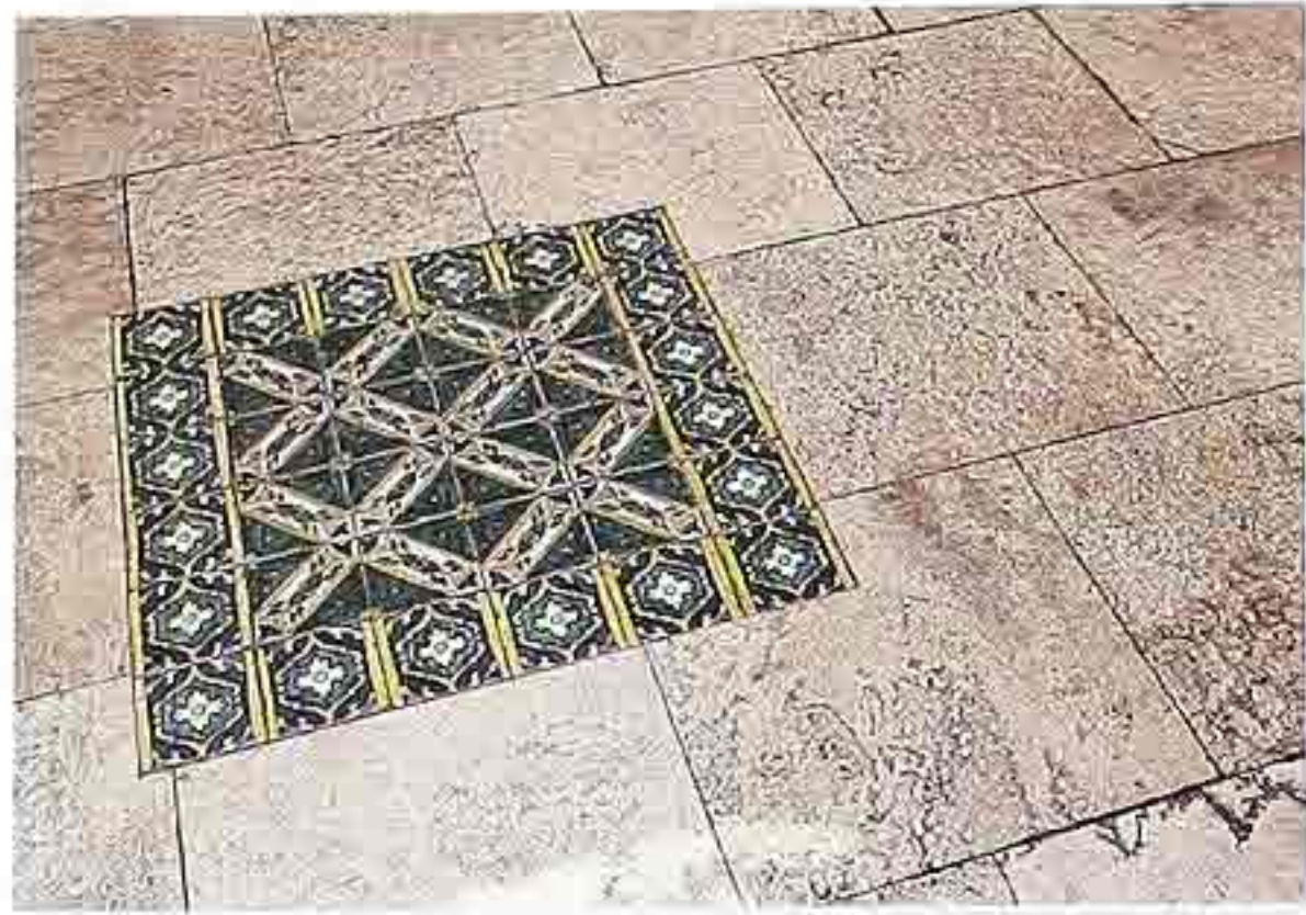
FP-91 Decorated glazed ceramic tiles surrounded by stone in running bond, commercial entry
