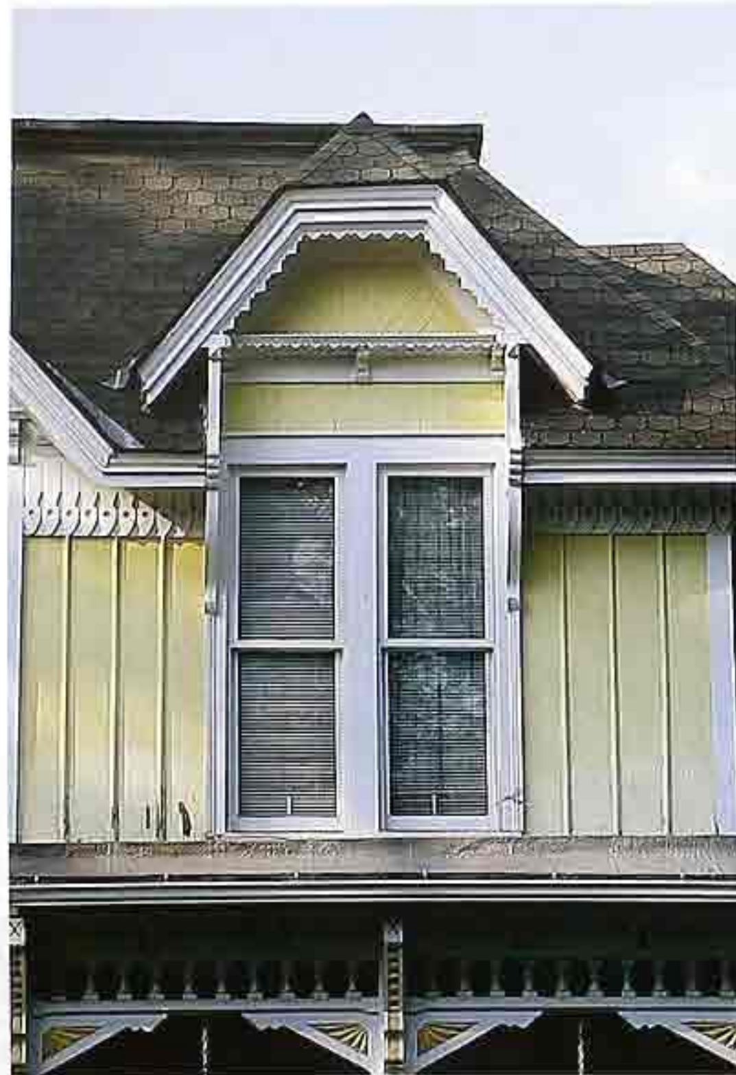
CR-76 Wall dormer with jerkinhead roof
