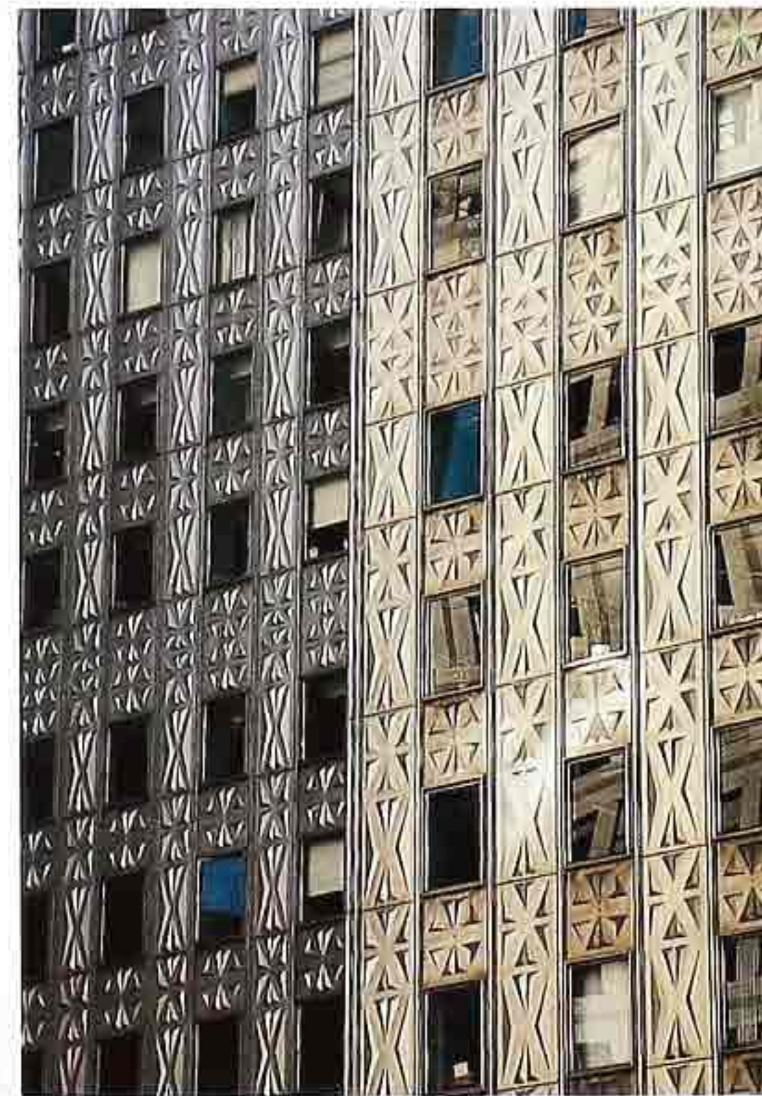
FA-14 Curtain wall; spandrel panels with dimensional geometric pattern, modern commercial building
