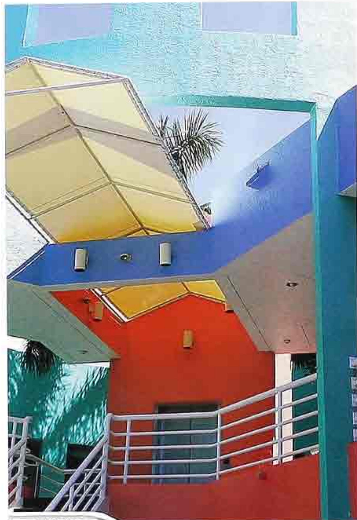
CR-141 Cantilevered fabric awning springing from freestanding stucco wall and ceiling, outdoor public space
