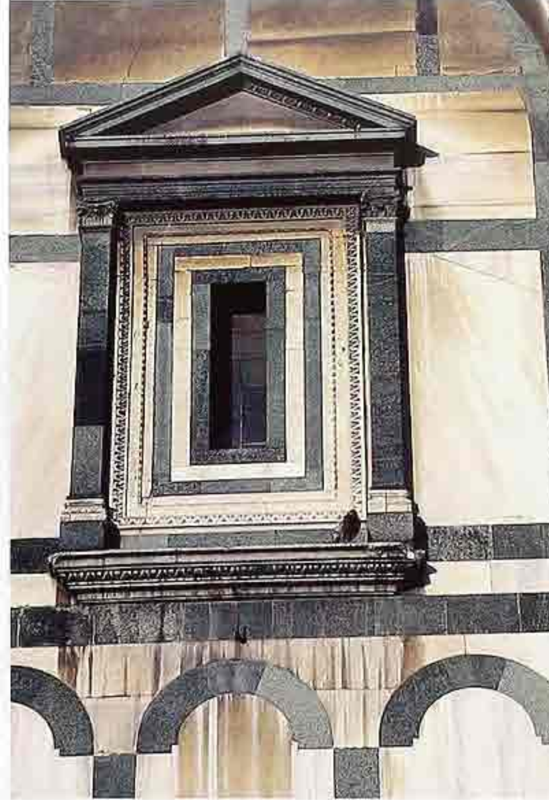
WI-133 Marble pediment and pilasters framing carved marble casing with polychrome marble bands, 12th-c. Italian church
