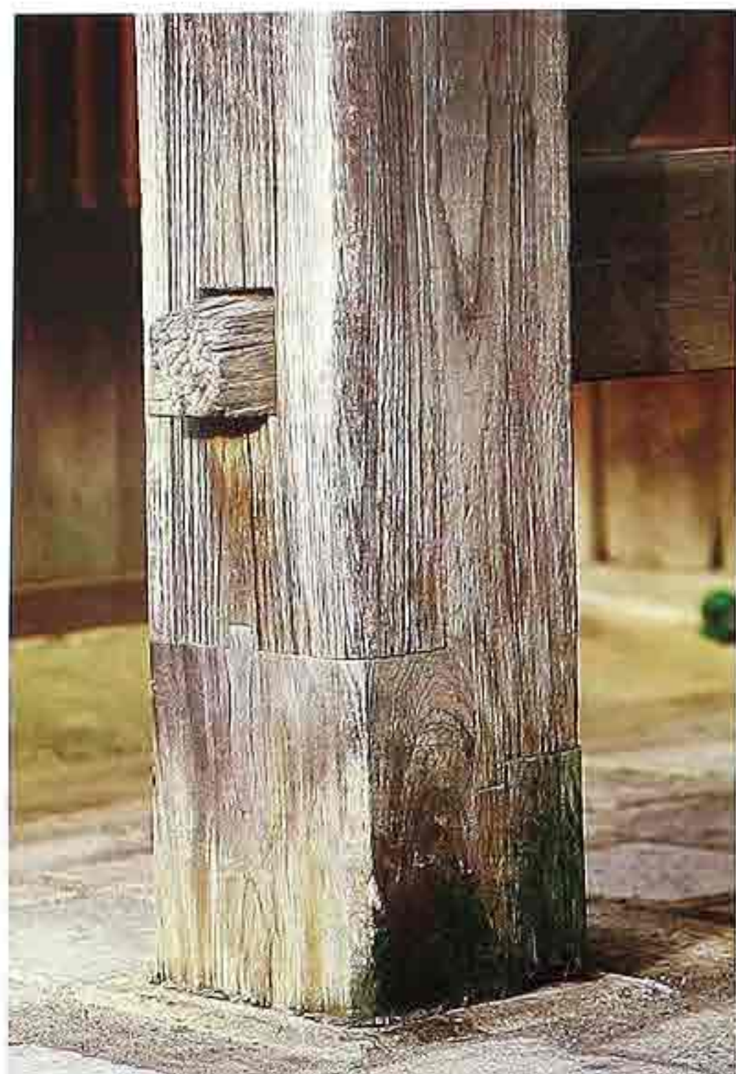
CP-105 Timber post with mortise-and-through-tenon joint.
