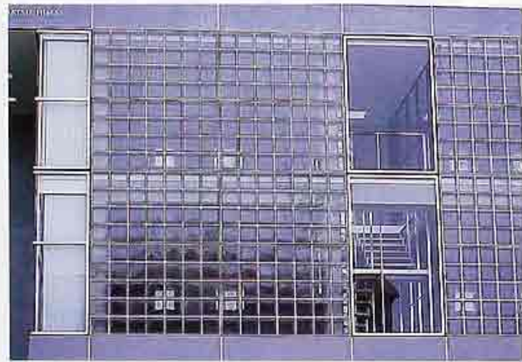
WI-21 Glass-block panels spanning two stories and flanked by fixed windows, modern commercial building
