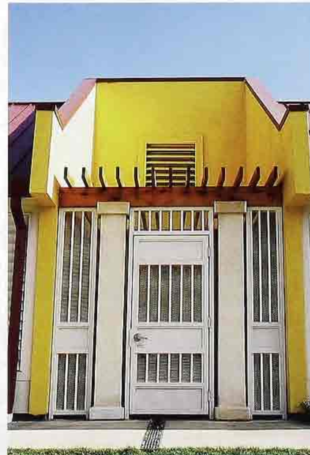
DW-99 Grille-covered door and side lights with pilasters, modern commercial building
