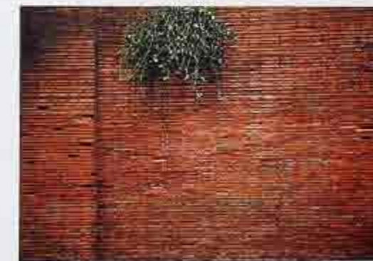
WA-162 Roman brick with pilaster, ancient wall
