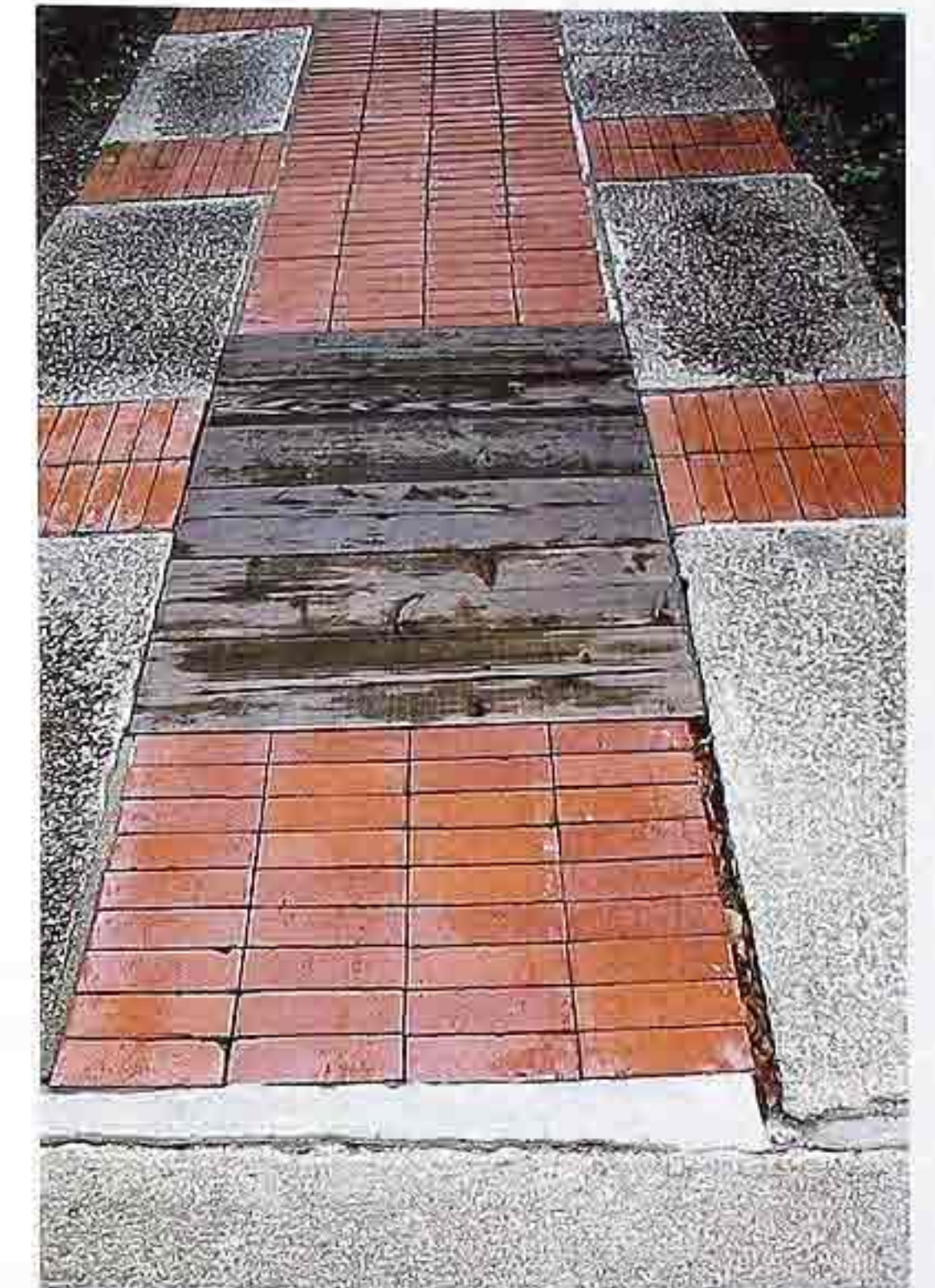
FP-62 Brick pavers in stack bond alternating with wood planks and large-aggregate concrete, urban public space
