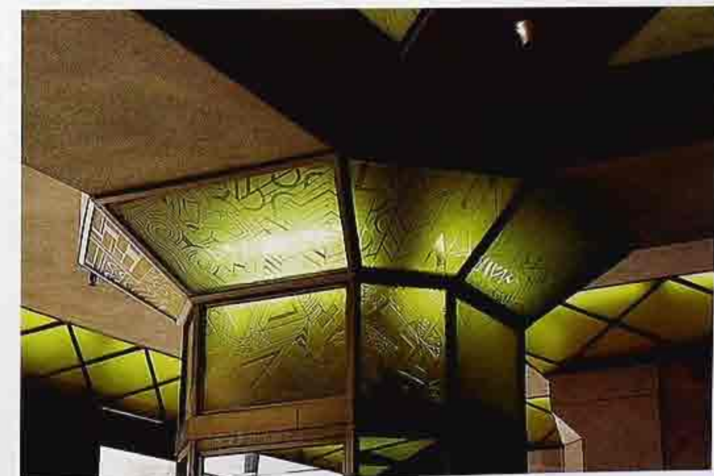
CP-30 Art Deco-style capital in glass and metal with non-regular octagonal profile, lit from inside
