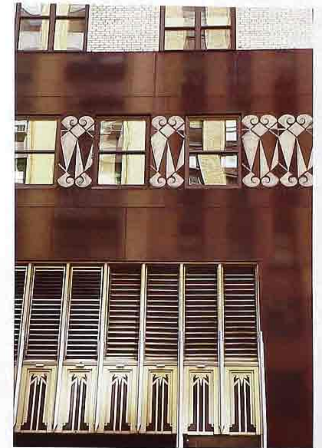
FA-116 Art Deco facade, highly polished stone cladding with geometric ornament below white glazed brick
