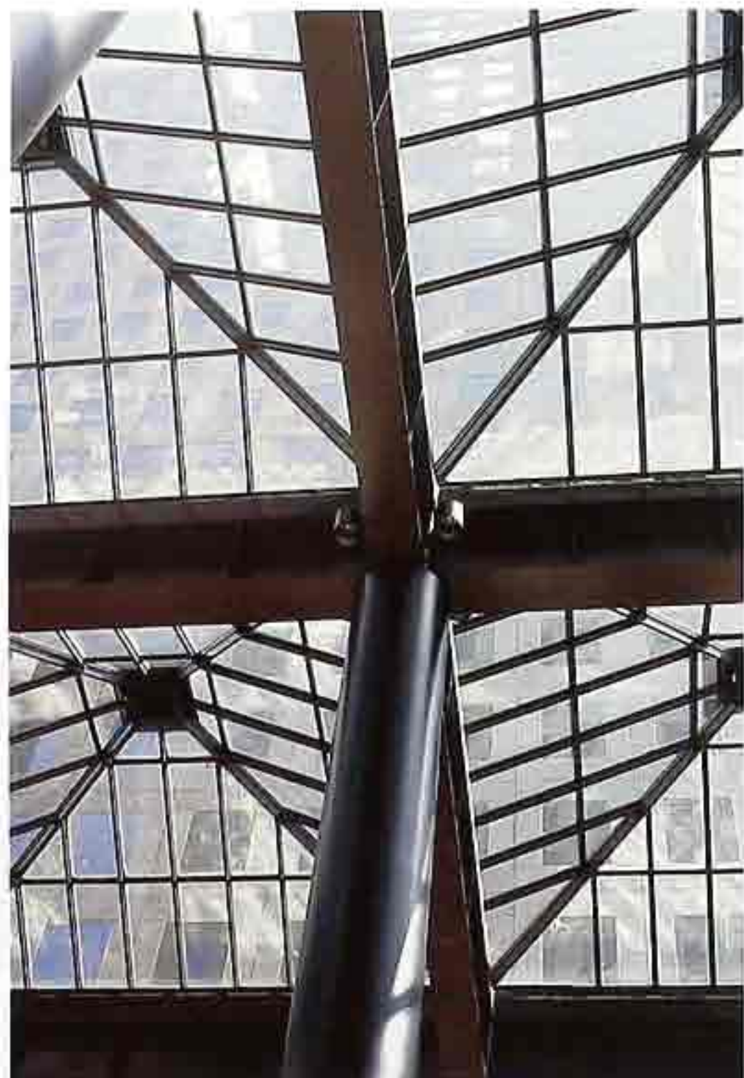
CP-112 Steel frame and tubular column; wide-flange beams supporting framed glass ceiling of modern commercial building
