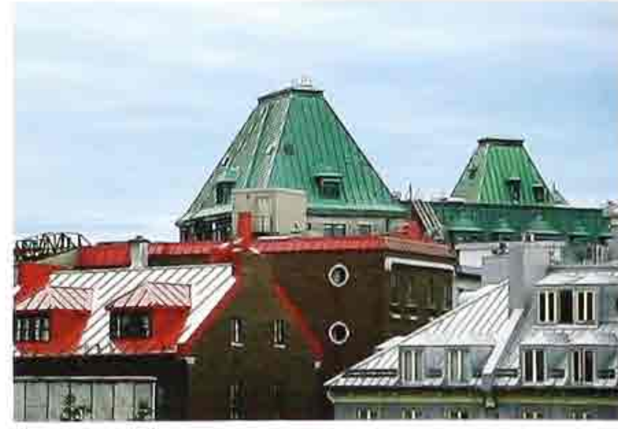
CR-116 Parapeted gable with hipped-roof dormers (left), hipped roof with hip dormers (right), and flared mansard with hip dormers (top), all sheet metal
