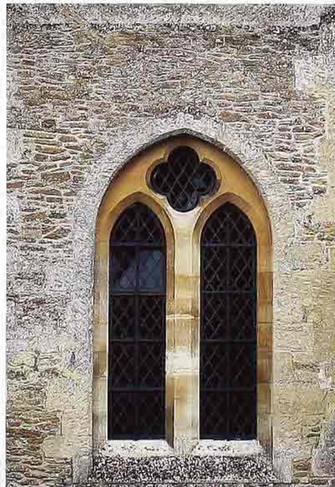
WI-135 Stone pointed segmental arch framing pair of leaded lancet windows with stone casings and leaded quatrefoil, 15th-c. English abbey
