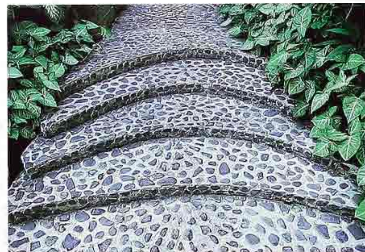
FP-75 Curved steps faced with large exposed aggregate. Aggregate applied, not revealed by washing
