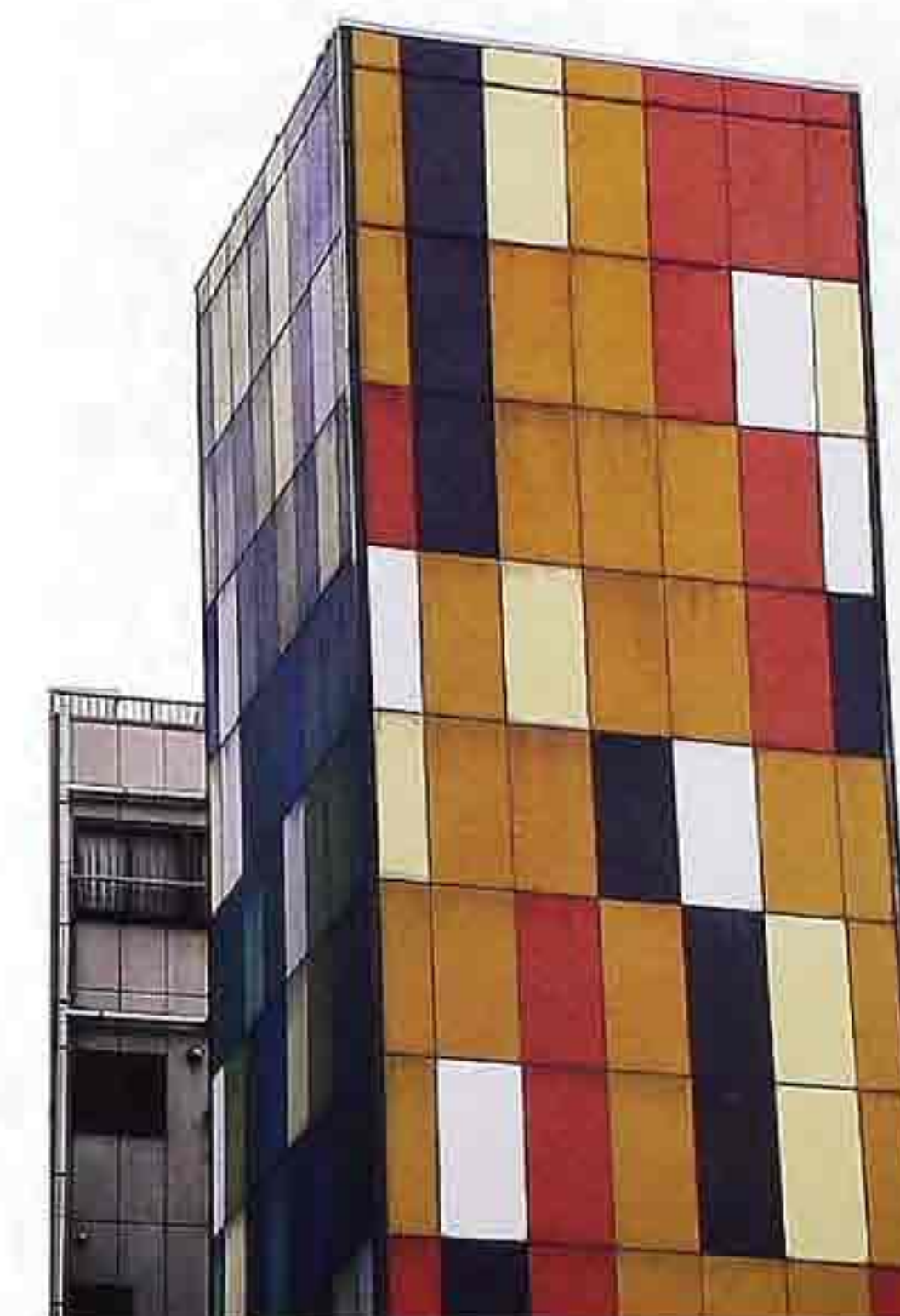
FA-89 Multicolored painted plywood cladding on building under renovation
