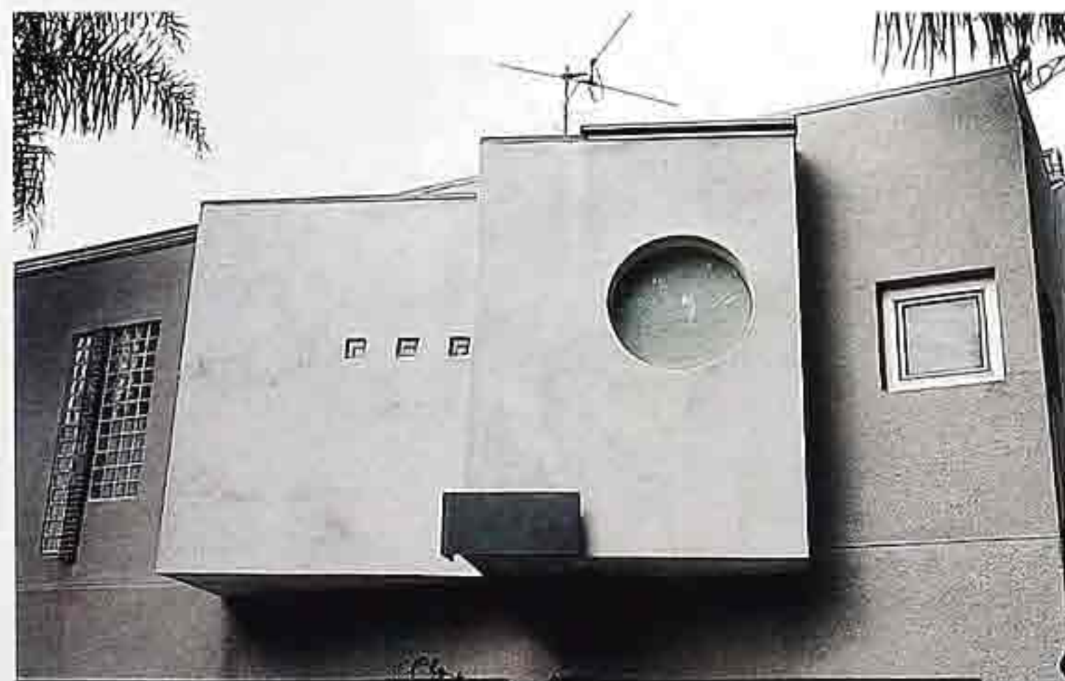
WA-216 Concrete projecting window, modern house
