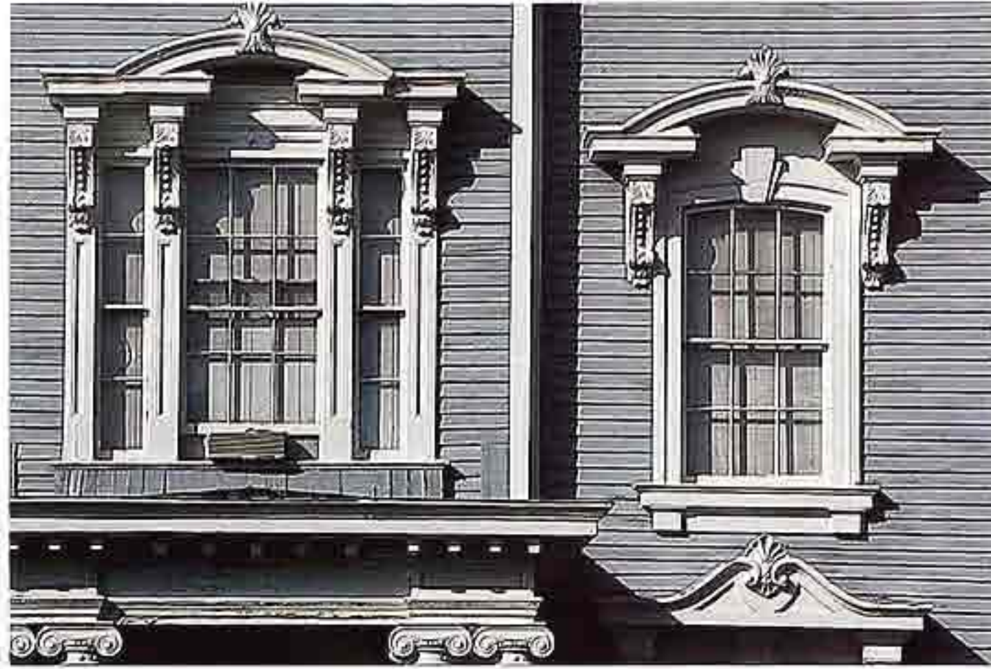
WI-104 Segmental pediment-capped window molding with consoles flanking double-hung windows, 19th-c. American house
