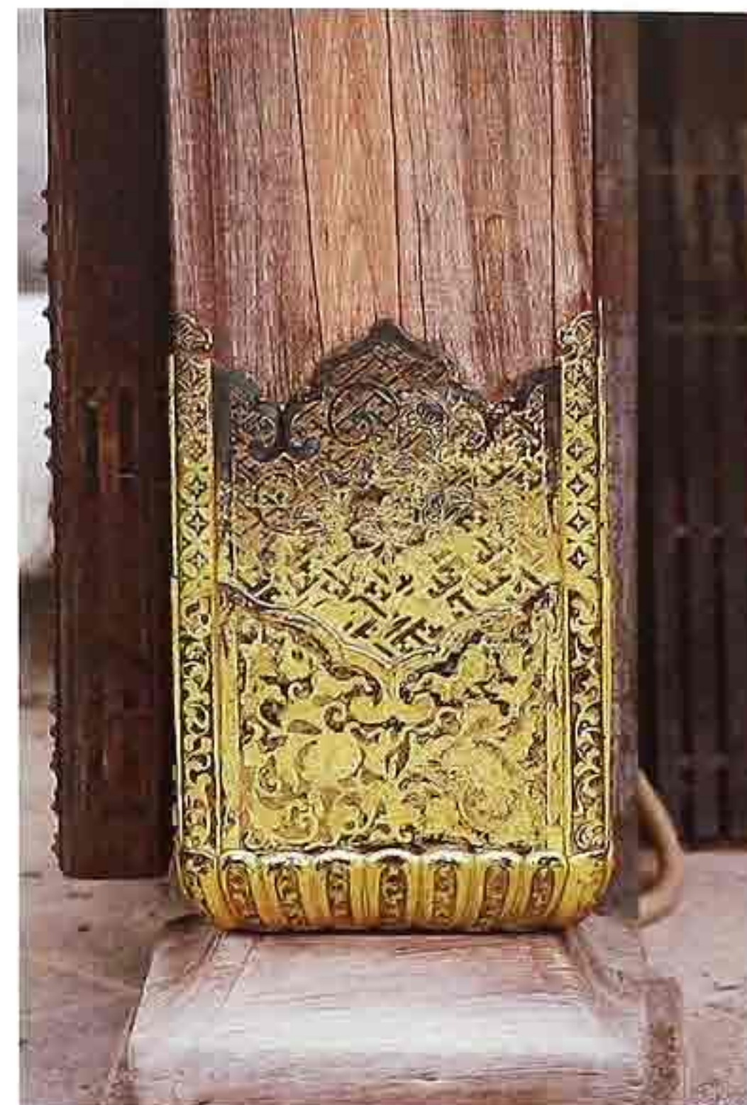
CP-54 Gilded relief ornamental metal sheath covering the base of a timber post
