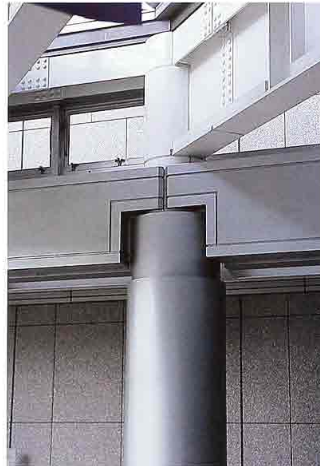
CP-123 Detail of steel frame with metal-clad column and beam beneath exposed riveted plate girders, modern commercial building
