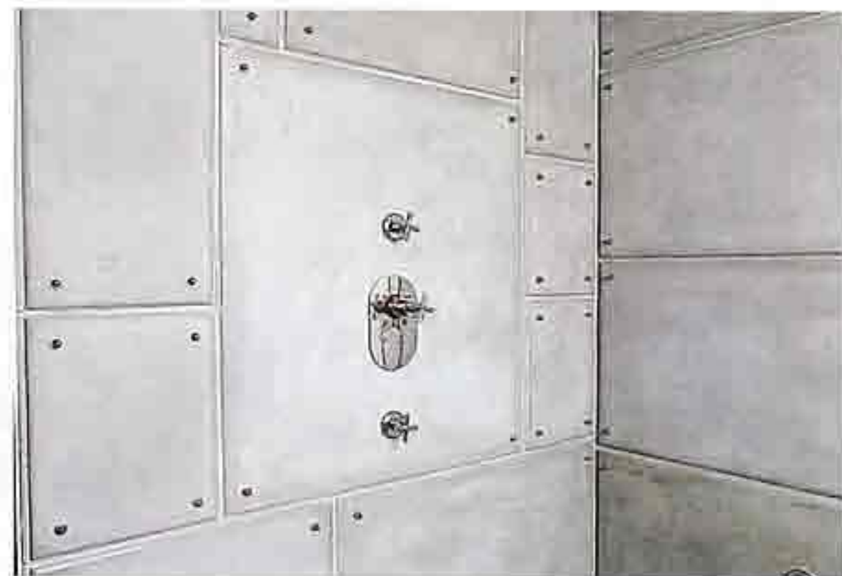
WA-215 Cast concrete, shower room
