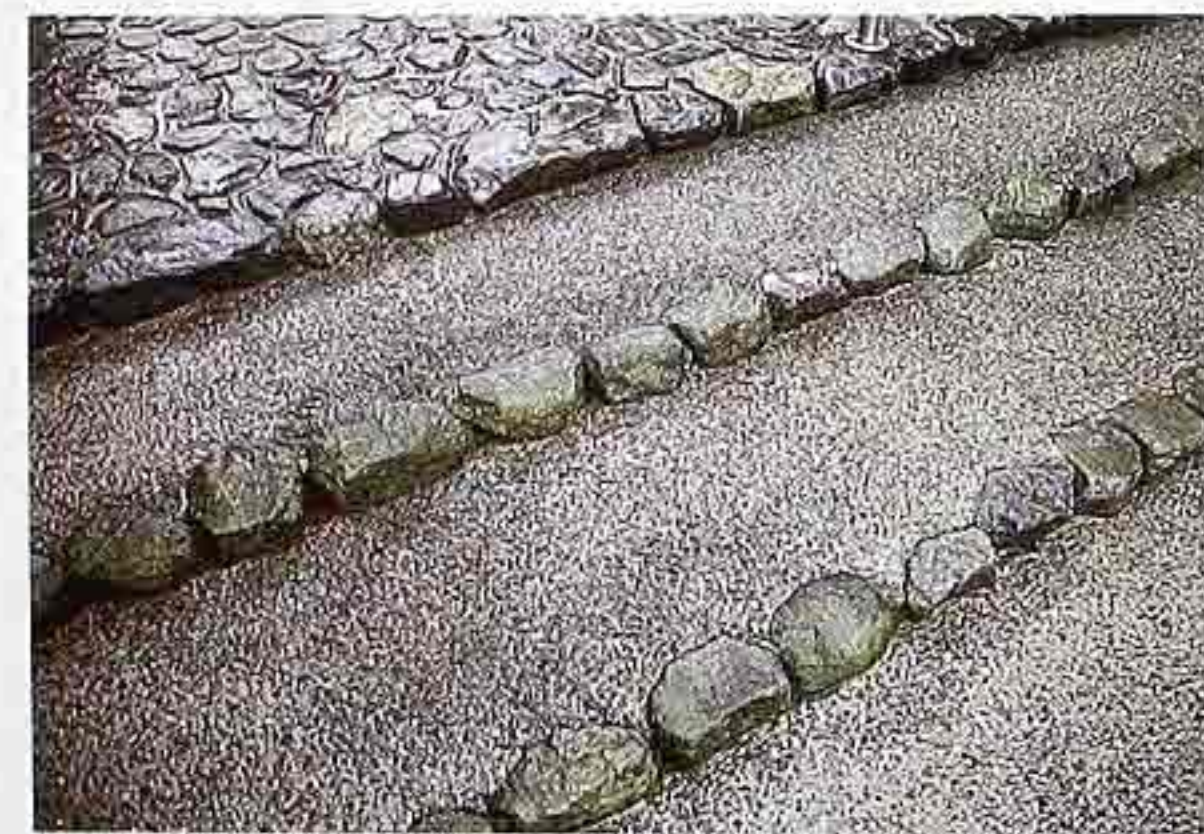
FP-76 Pea-sized gravel aggregate inset with rows of rocks and bordered by small split, polished fieldstone set in concrete
