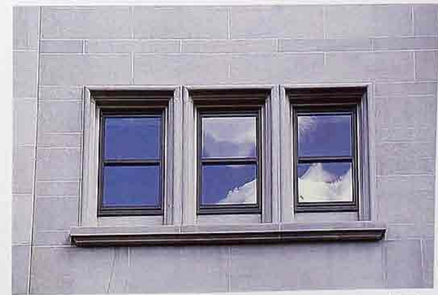
WI-131 Set of three recessed windows with stone molded casings and single molded sill, early 20th-c. commercial building
