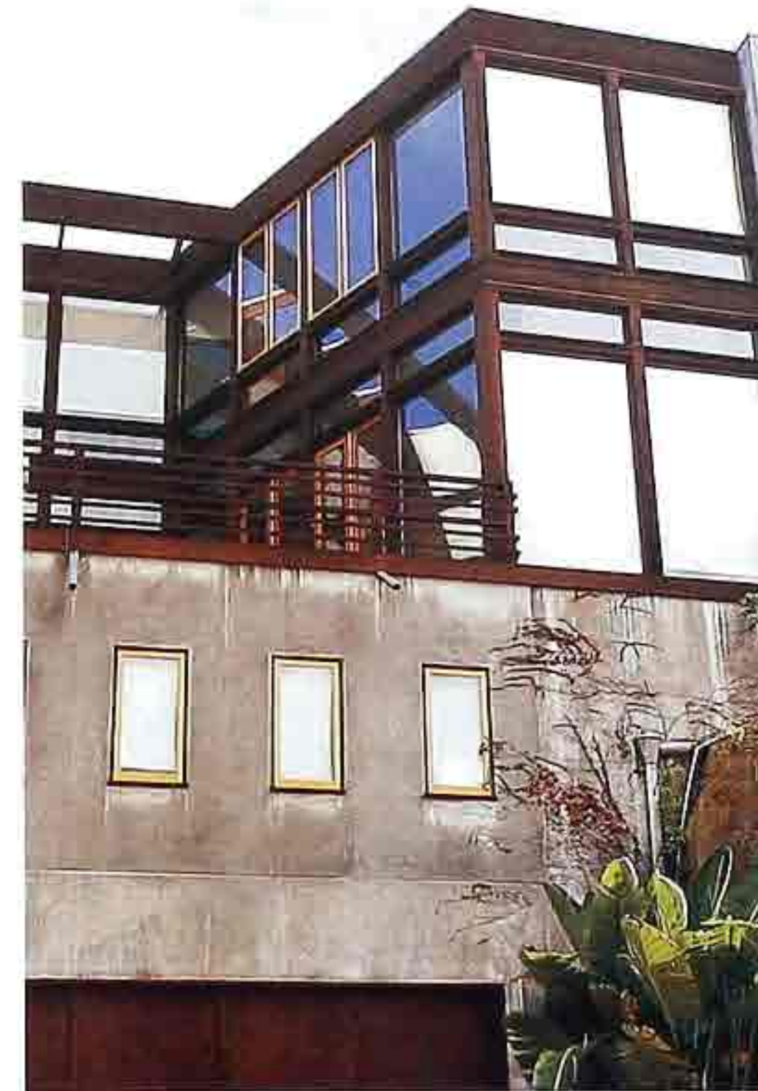
WA-208 Weathered cast-in-place concrete with smooth finish; metal and glass upper story, modern house
