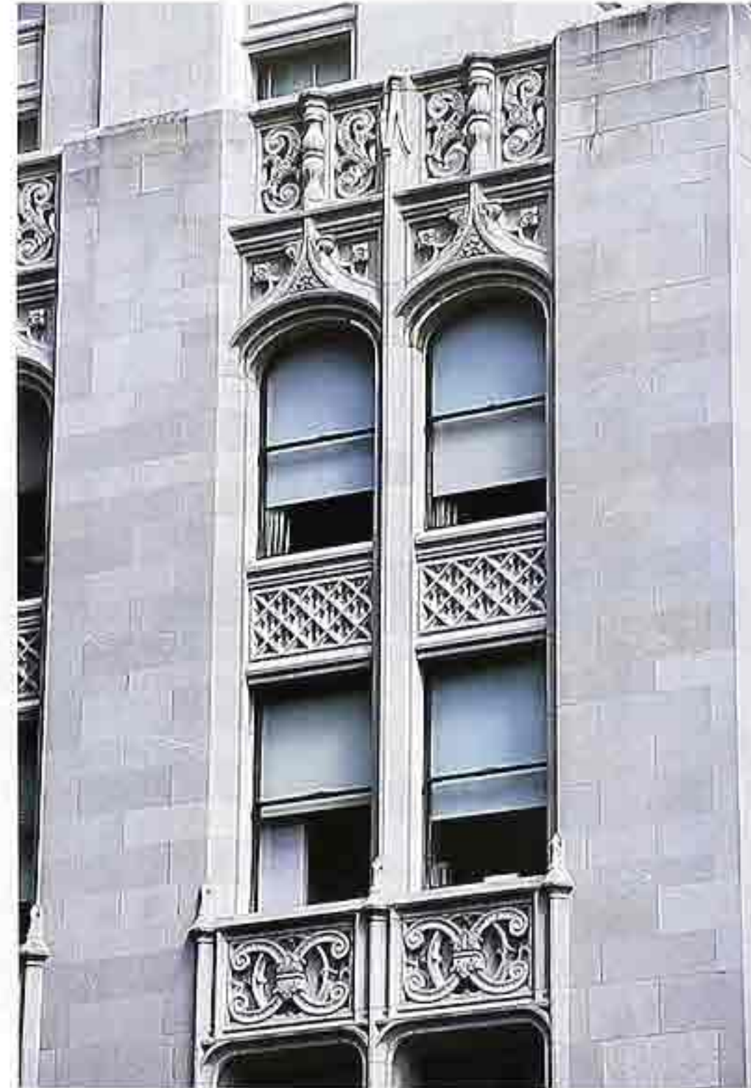
WI-141 Neo-Gothic ornament in spandrels and capping window panels, early 20th-c. commercial building
