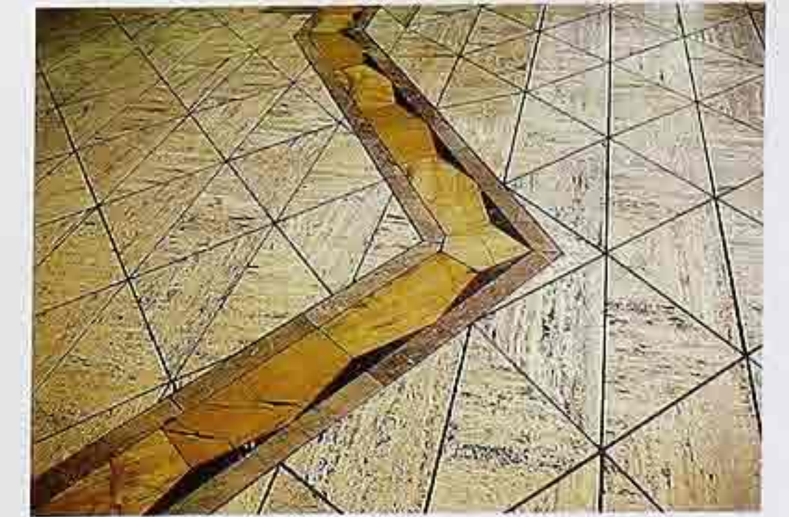
FP-18 Travertine and marble parquet in geometric pattern with marble polychrome band in foyer
