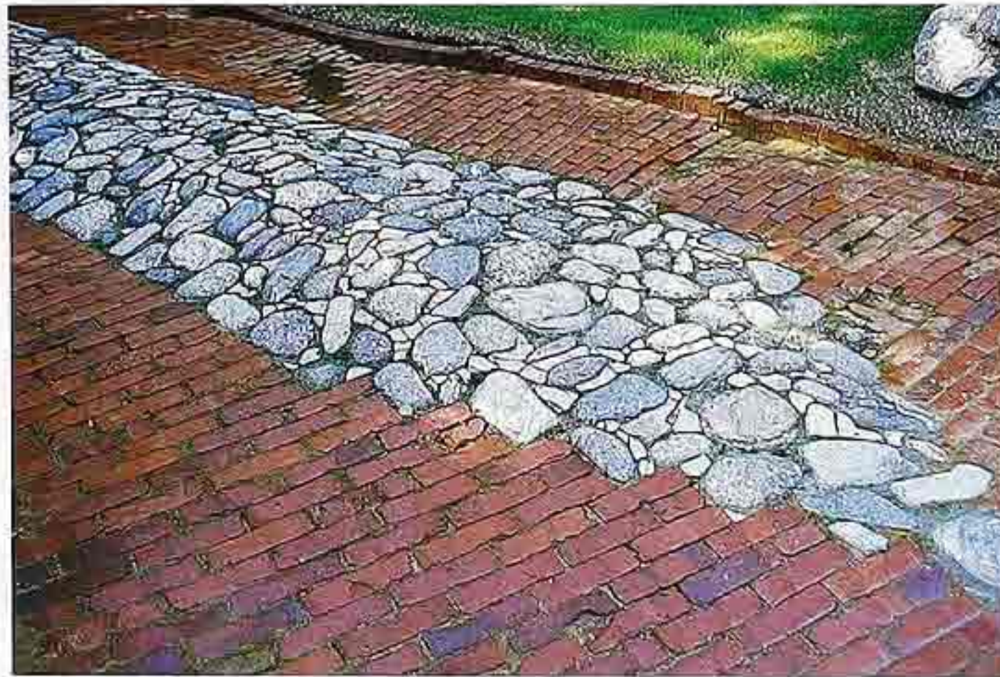
FP-38 Uncoursed fieldstone used as divider in running-bond brick driveway, Arts and Crafts residence
