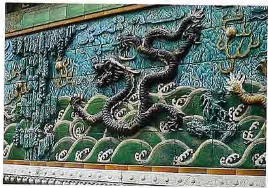
FA-62 Glazed polychrome relief tiles with dragon design on exterior wall
