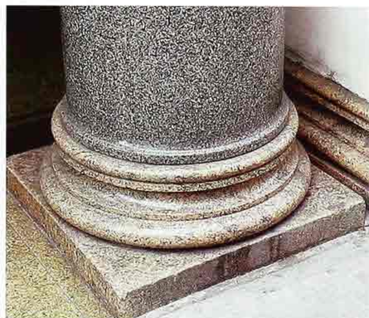
CP-34 Attic base on a thin plinth. Top to bottom: torus; fillet; scotia; fillet; torus
