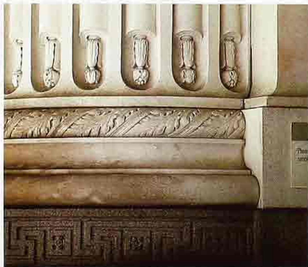
CP-33 Marble Attic base with foliated ornament on upper torus on plinth in contrasting stone with Greek-key molding; ornamented fluting
