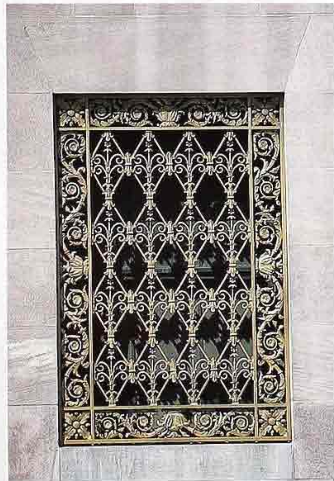
WI-169 Brass window grille with arabesque design around pierced diaper-work
