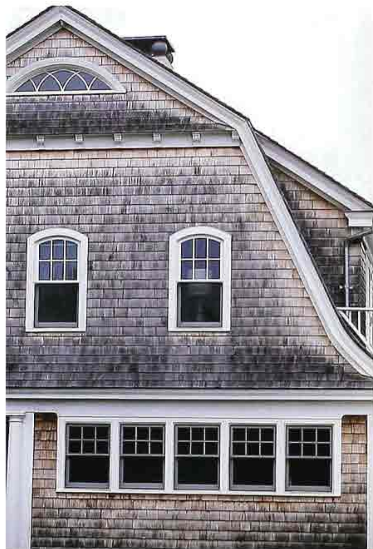
WI-49 Top to bottom: arched gable window; arched six-over-one double-hung windows; six-over-one double-hung windows, traditional shingle house
