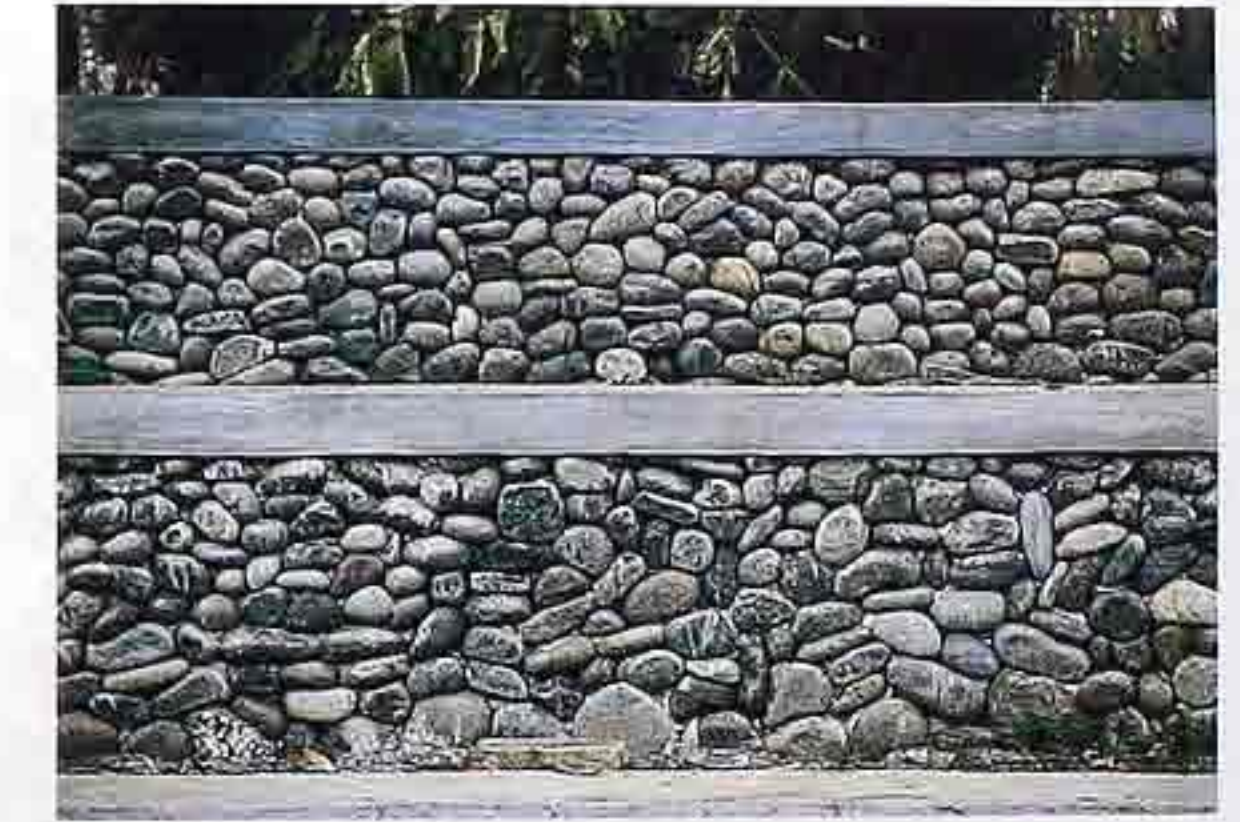
WA-79 Rubble walls of cobbles with wide squared stone step capping lower wall and coping on upper wall
