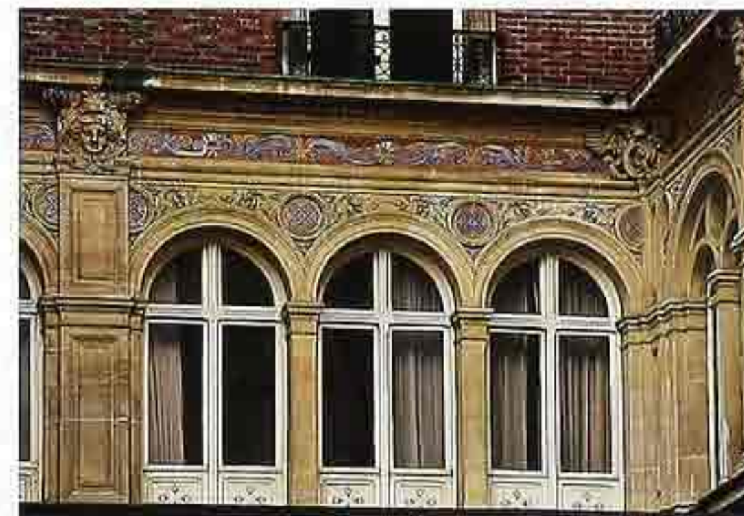
WI-143 Series of arches, pilasters, and polychrome terracotta or stone spandrels framing windows in stone casing, 19th-c. French mixed-use building
