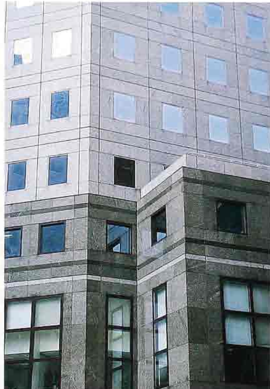
WA-141 Polished granite veneer with flush-mounted fixed windows in polychrome curtain wall, modern commercial building
