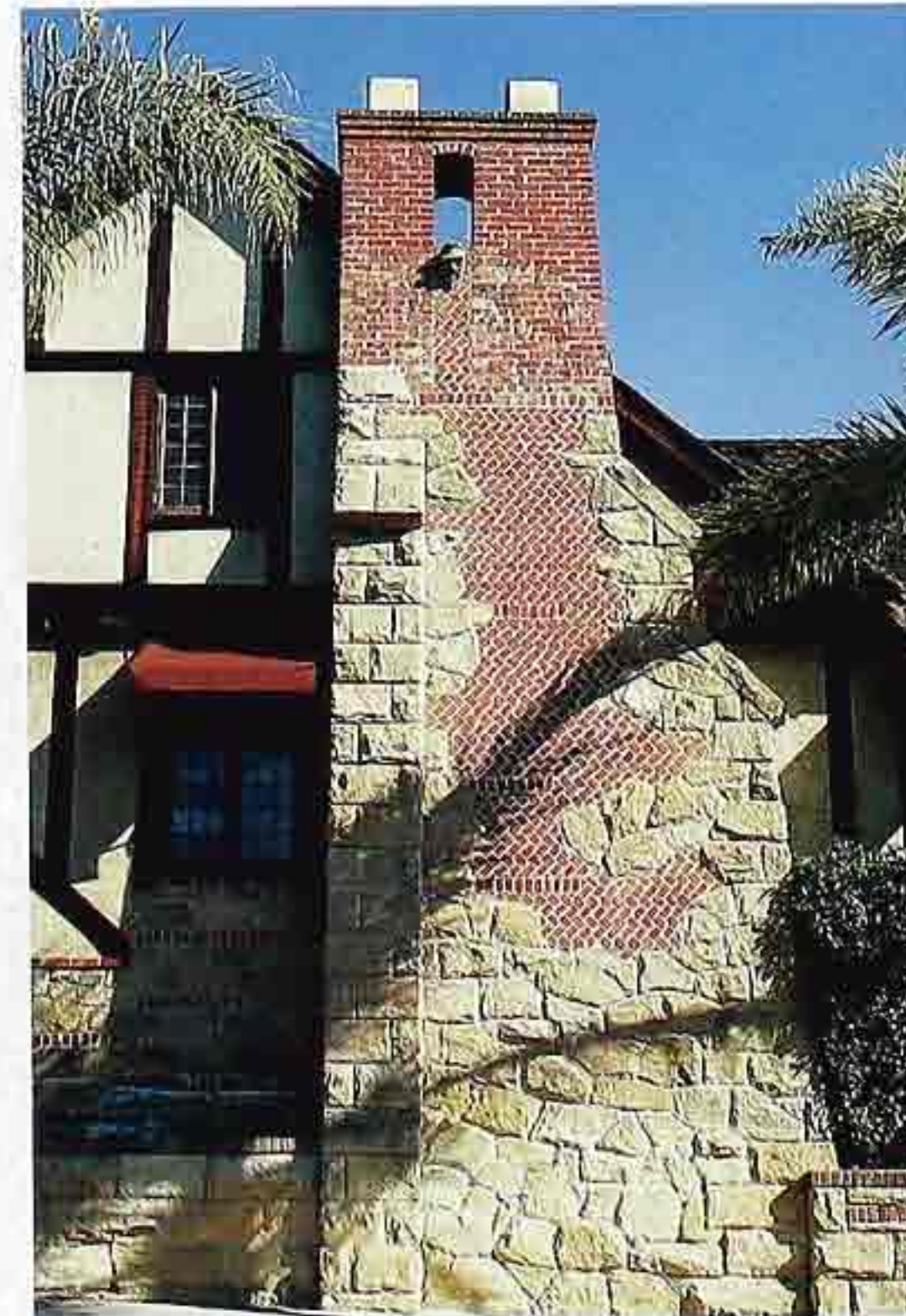
CR-150 Chimney: coursed-ashlar buttress and random ashlar stonework, herringbone brick
