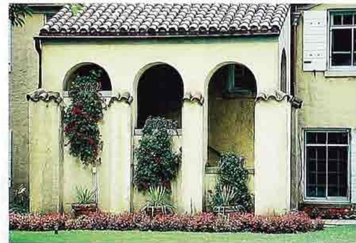
CP-165 Semicircular arcade, stucco over brick; tile roof
