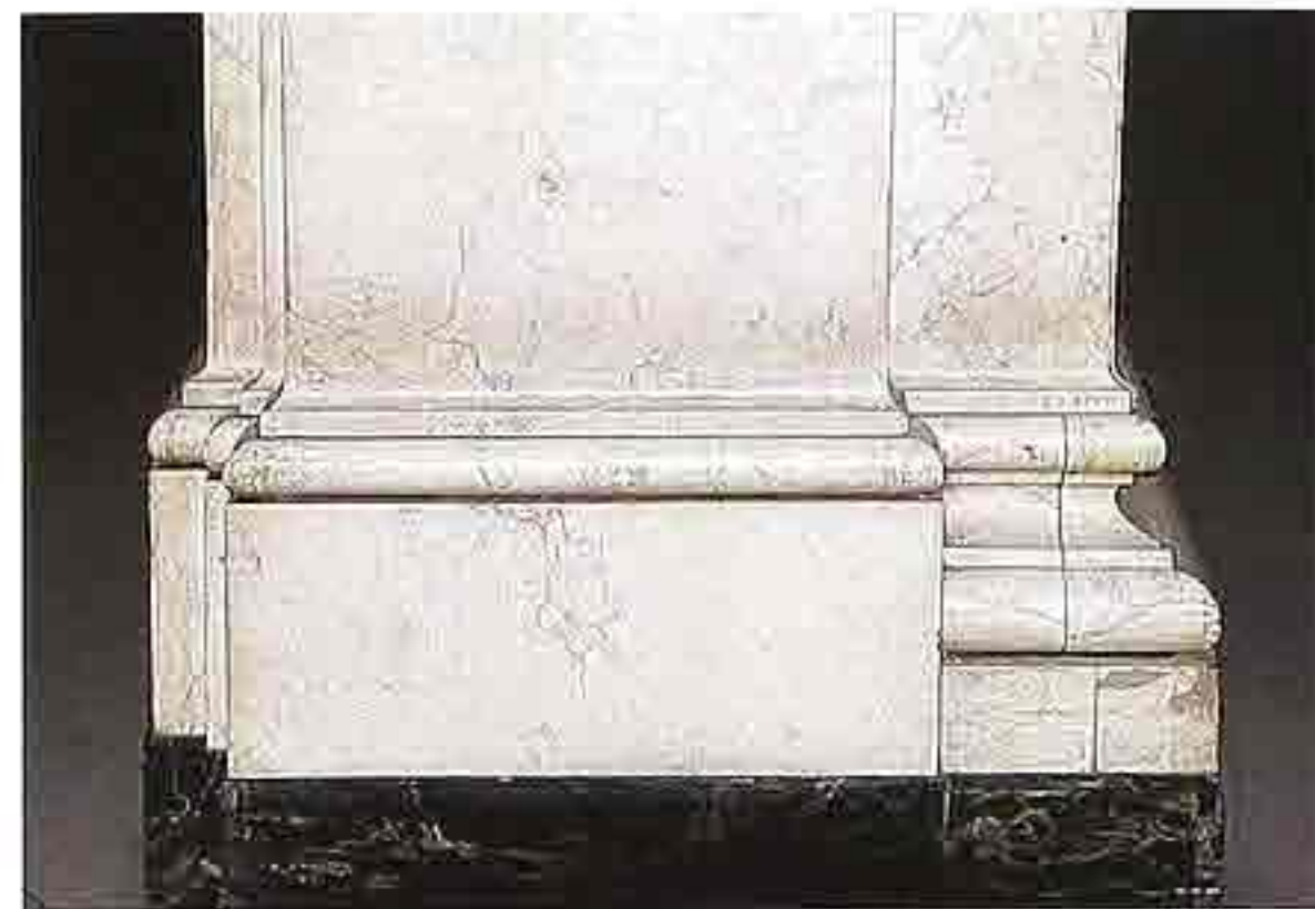
CP-50 Marble column with compound square base. Left: Attic profile base on a high plinth; right: Attic profile
