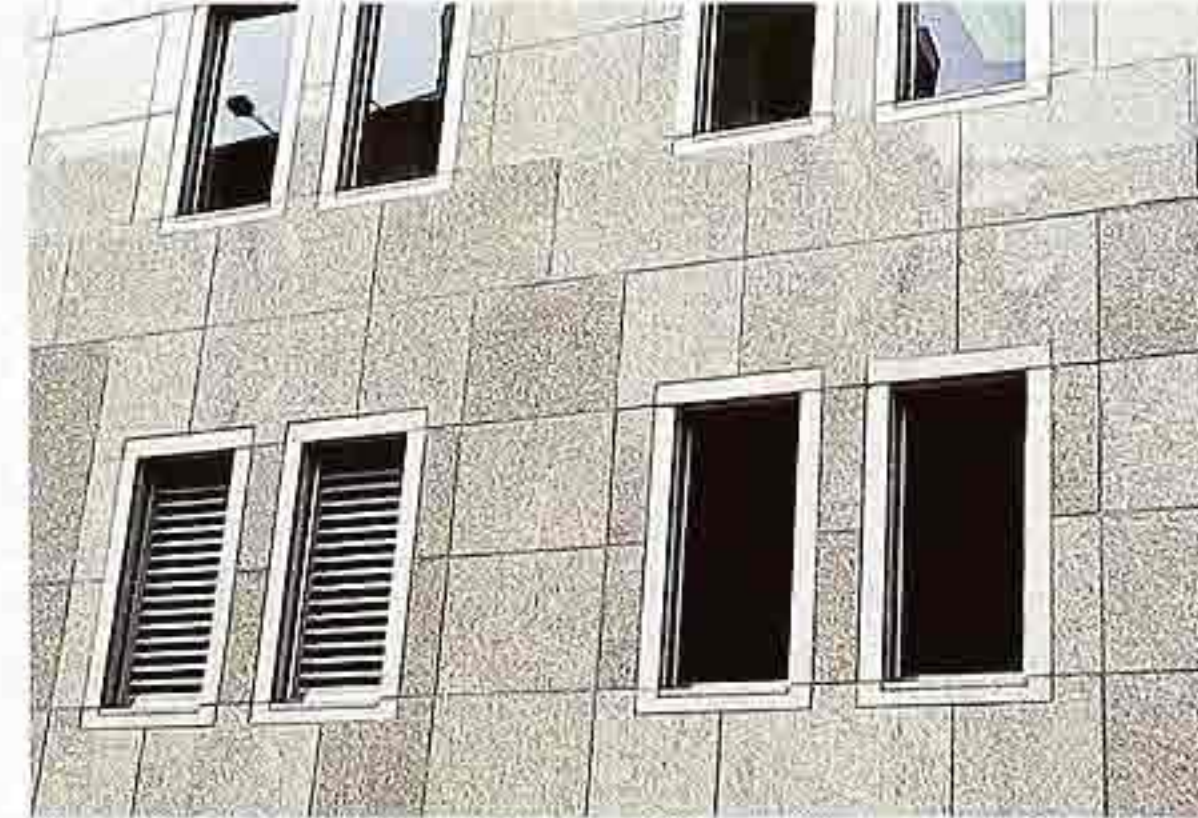
WI-161 Group of fixed windows with two louvered ventilation panels in stone surround, modern commercial building
