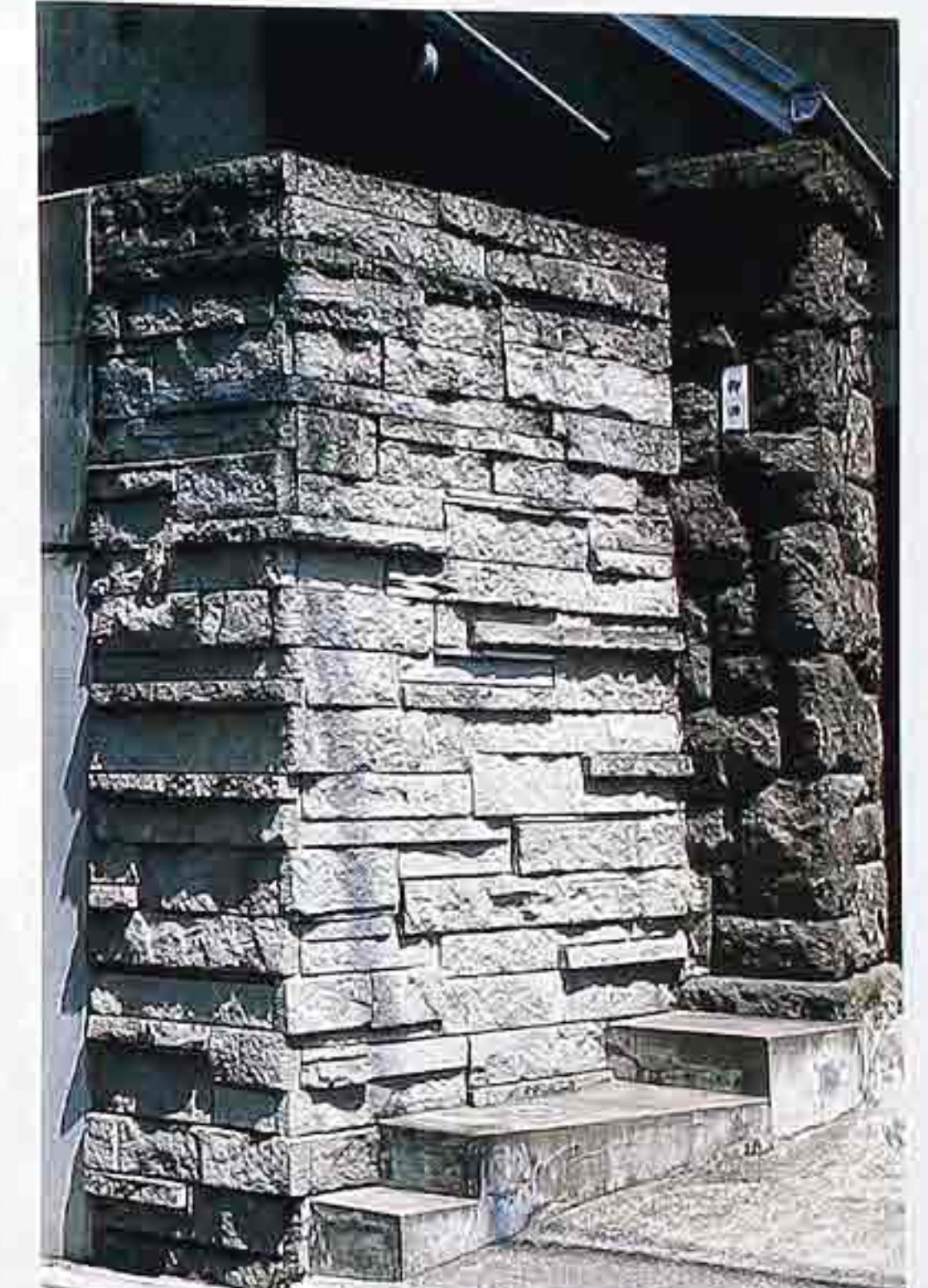
WA-94 Split-faced granite wall in shelf, random ashlar with roughly squared rubble pillar (right)
