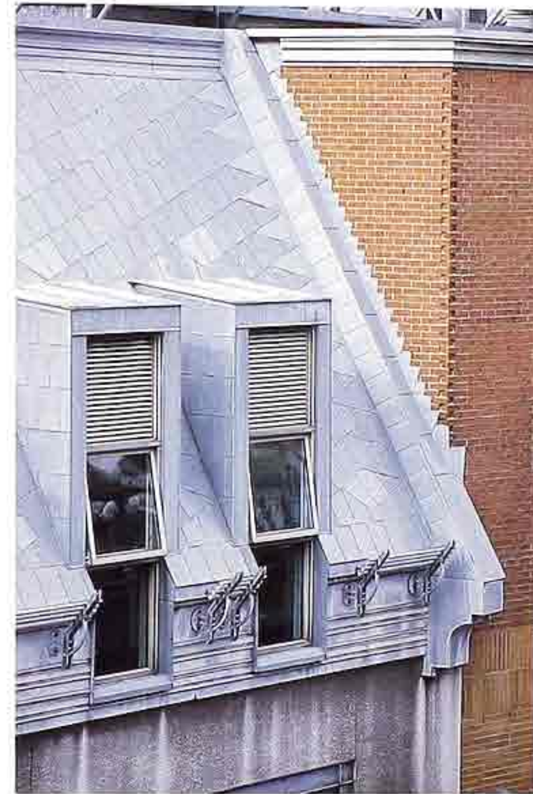
CR-99 Flat-roofed wall dormers on metal roof
