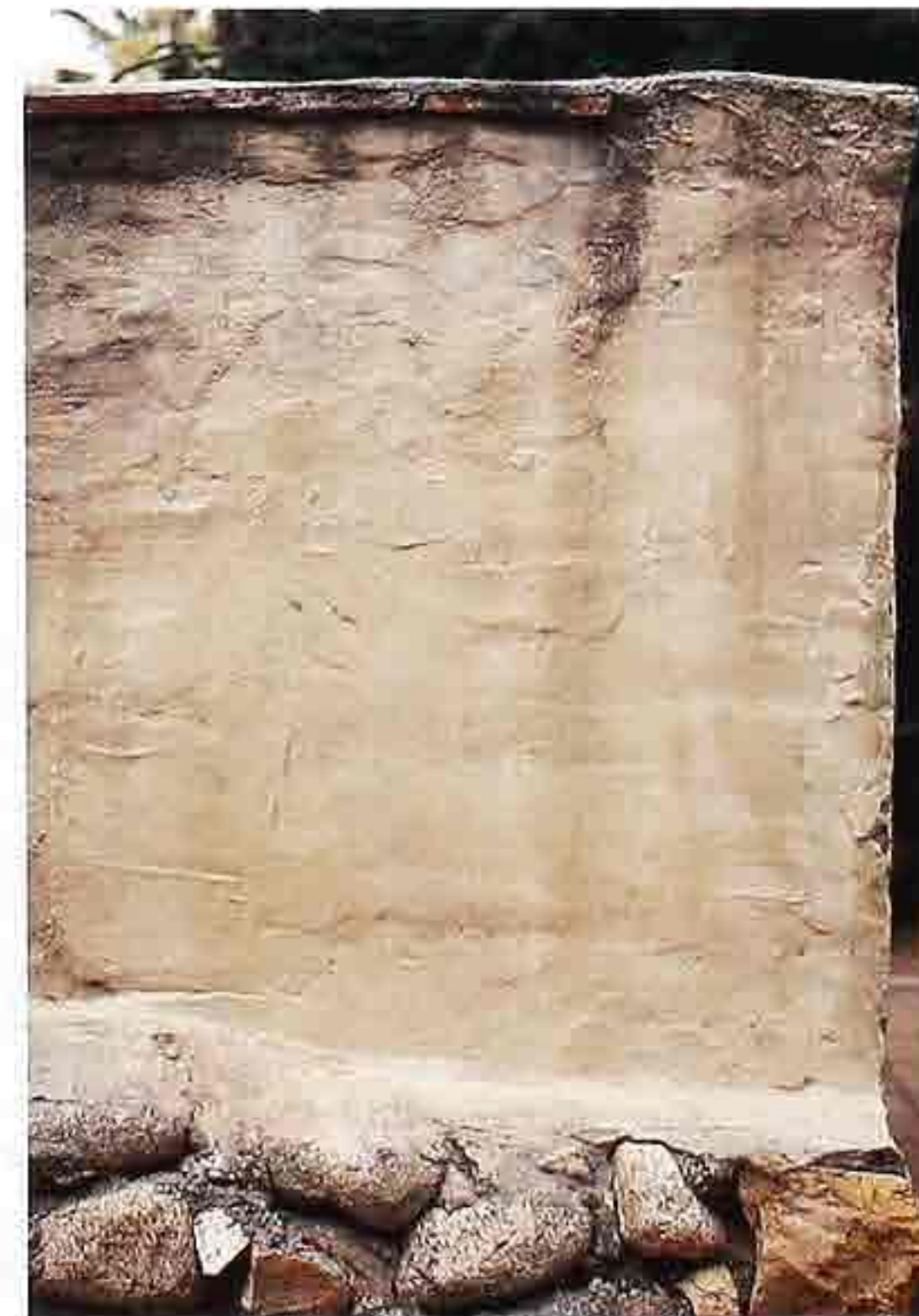
WA-233 Smoothed and whitewashed mud plaster over adobe brick on a base of fieldstone, courtyard wall
