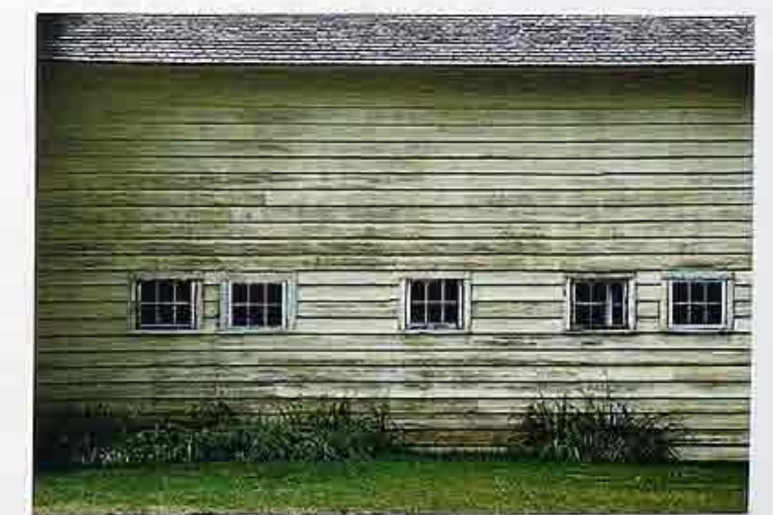
WA-25 Weathered painted clapboard wall with windows
