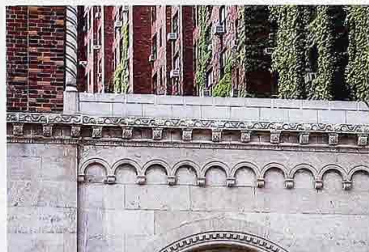
OM-88 Cornice. Top to bottom: serpentine band; modillion band; Gothic cornice. Dentilated archivolte at bottom
