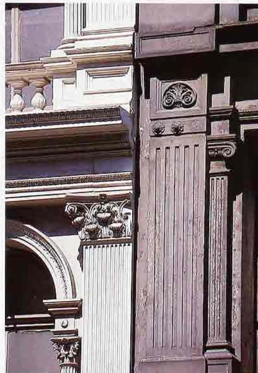
CP-83 Antae of adjacent cast-iron buildings. Left: Corinthian pilaster with fluting; right: fluted shaft with eclectic capital and adjacent jamb-shaft
