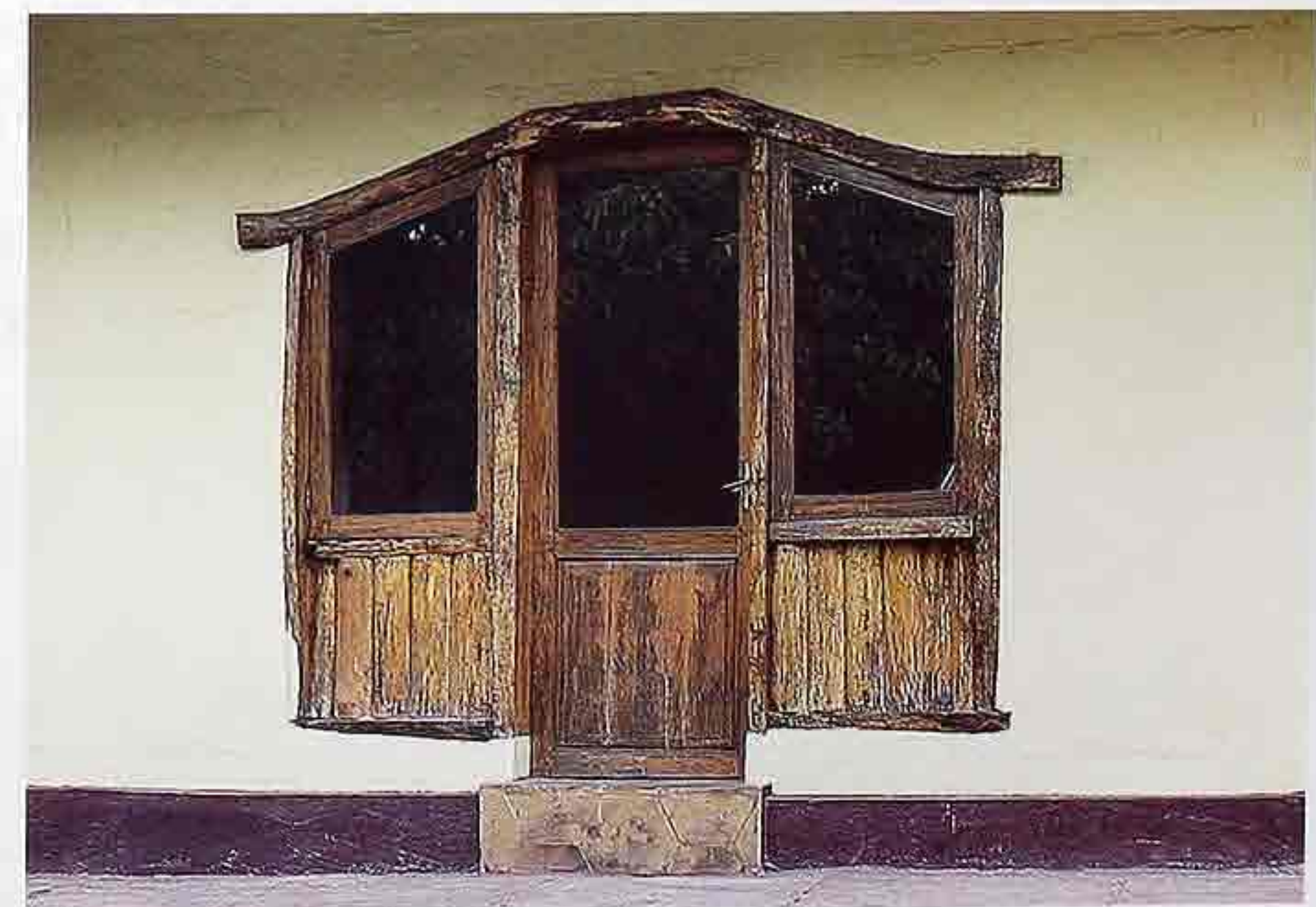
DW-71 Single-light door and side lights in rustic wood with curved timber eyebrow lintel
