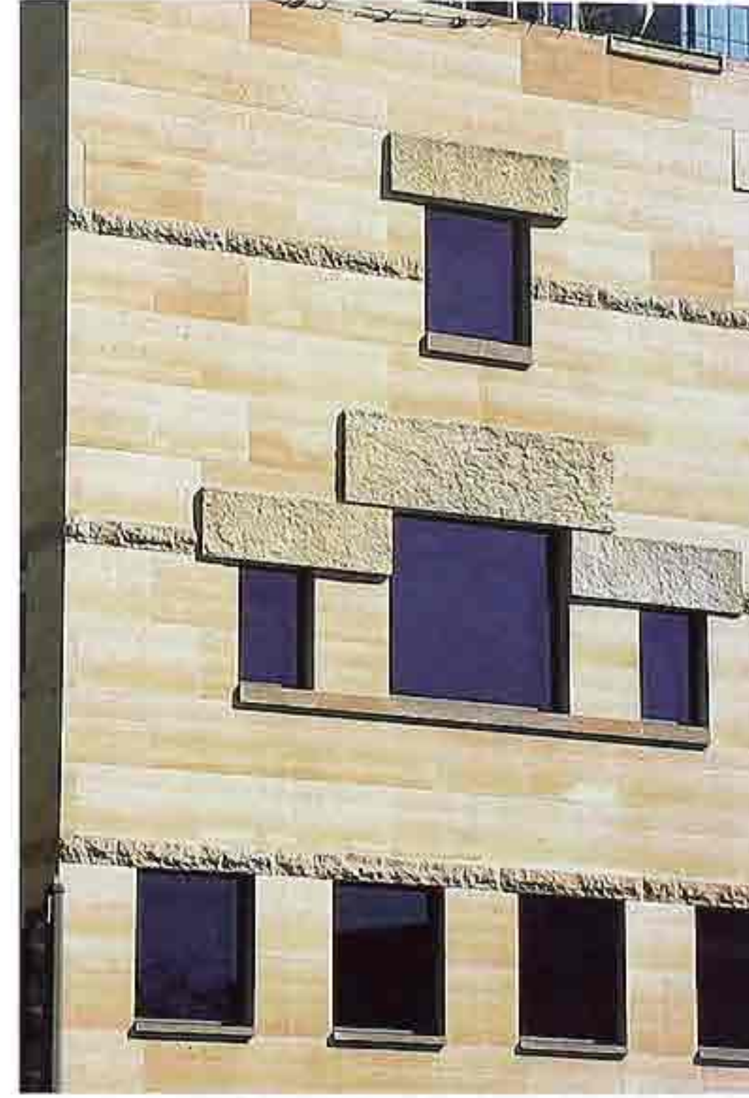
WI-154 Variety of fenestrations of rectangular, probably fixed, windows, modern commercial building
