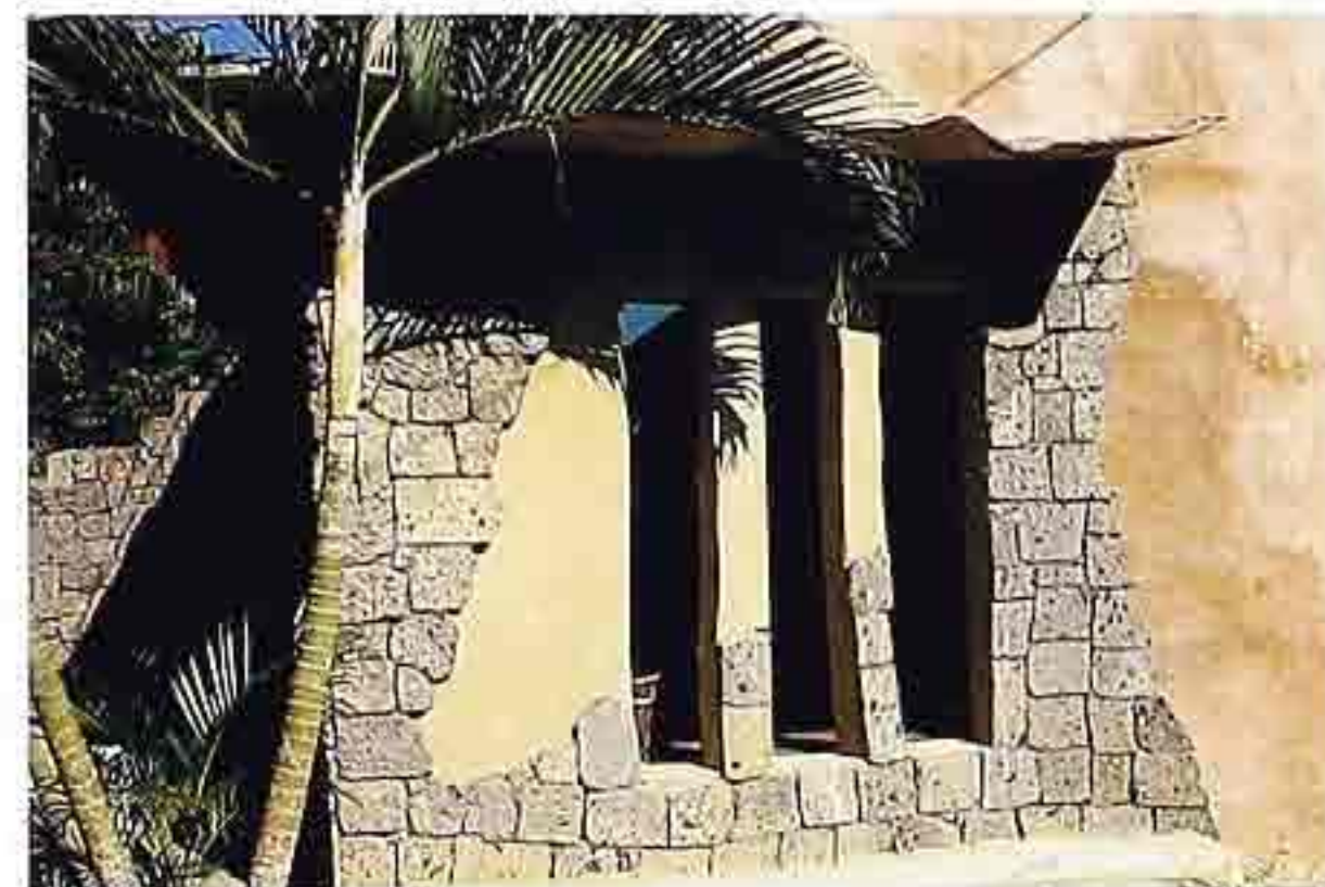
WA-241 Stucco over random ashlar stone
