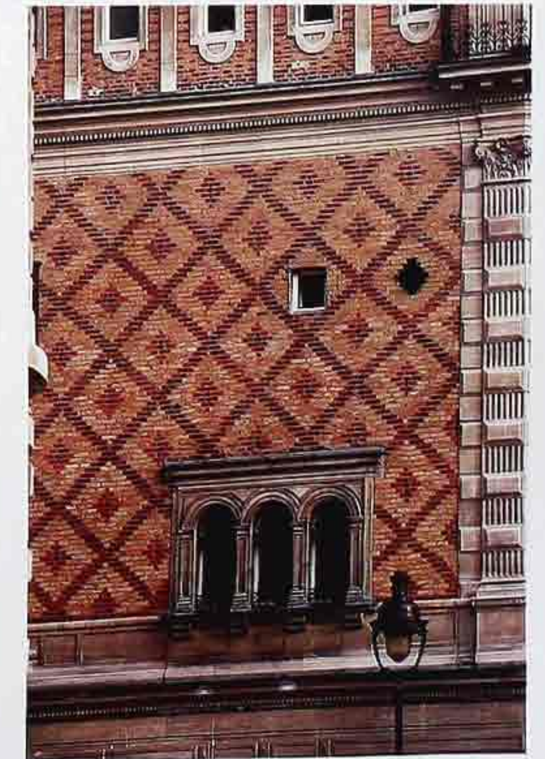
FA-111 Diamond-patterned brick facade with window arcade, framed by a rusticated corner pilaster and cornice
