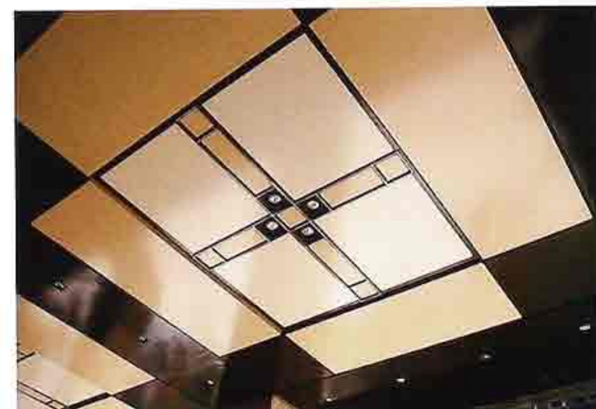
CR-13 Ceiling of contrasting colored enameled panels in Art Deco design on portico
