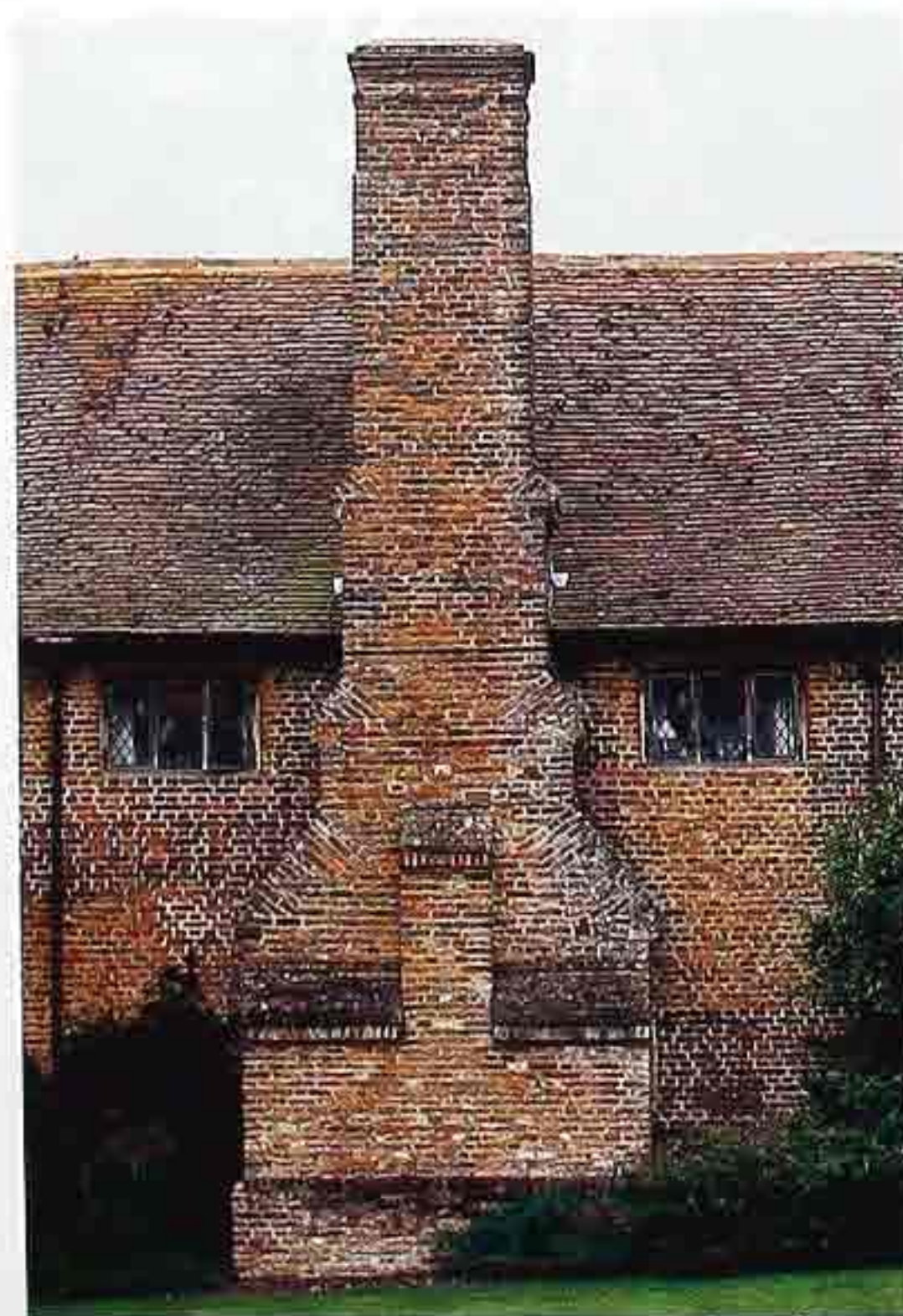
CR-149 Brick chimney
