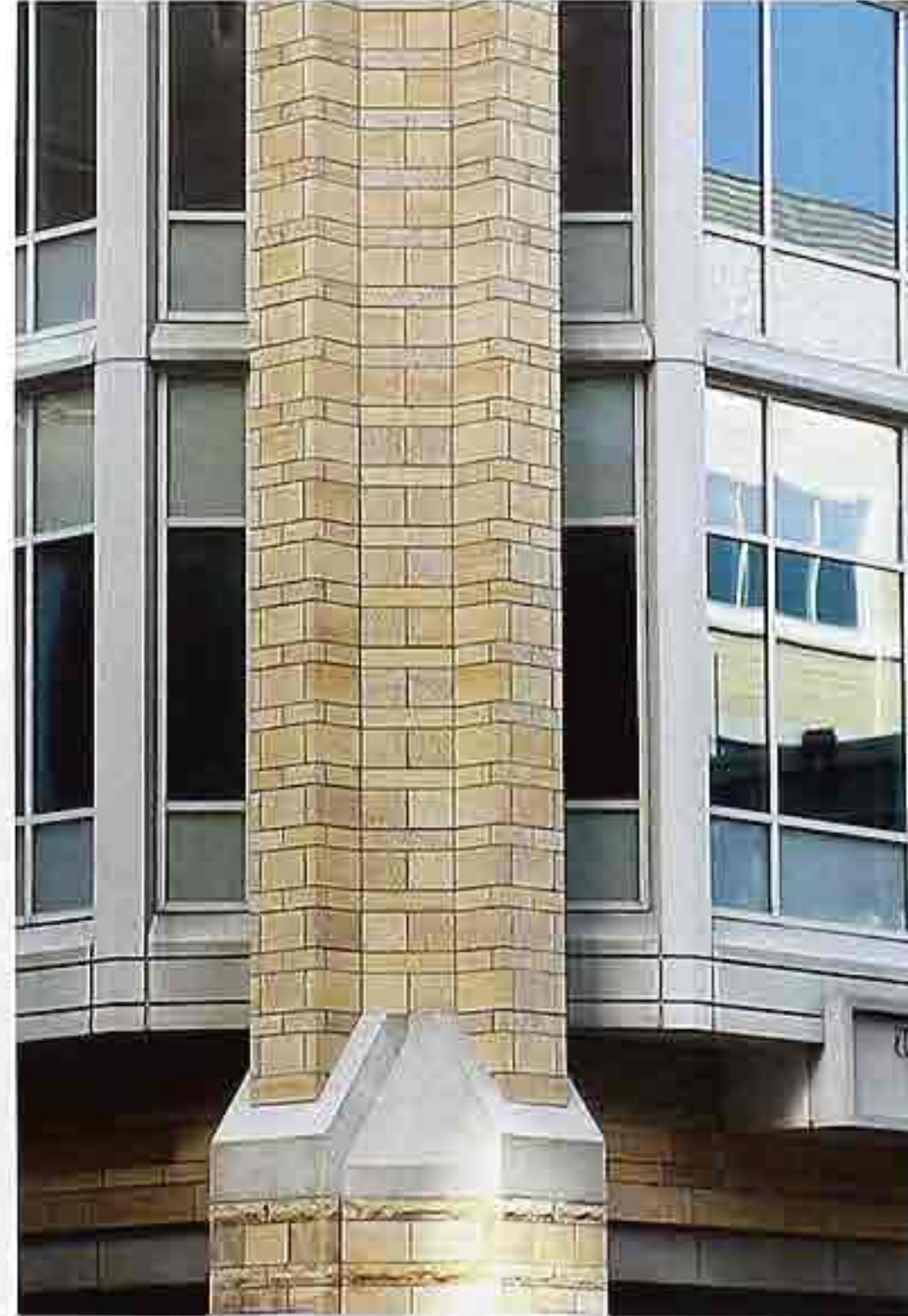
CP-81 Compound corner pier, modern commercial building
