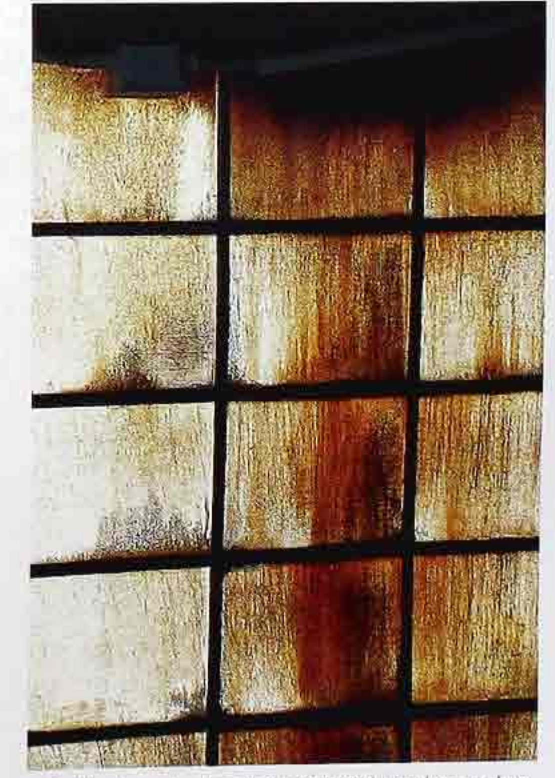
WI-8 Metal muntins holding weathered translucent glass, industrial building
