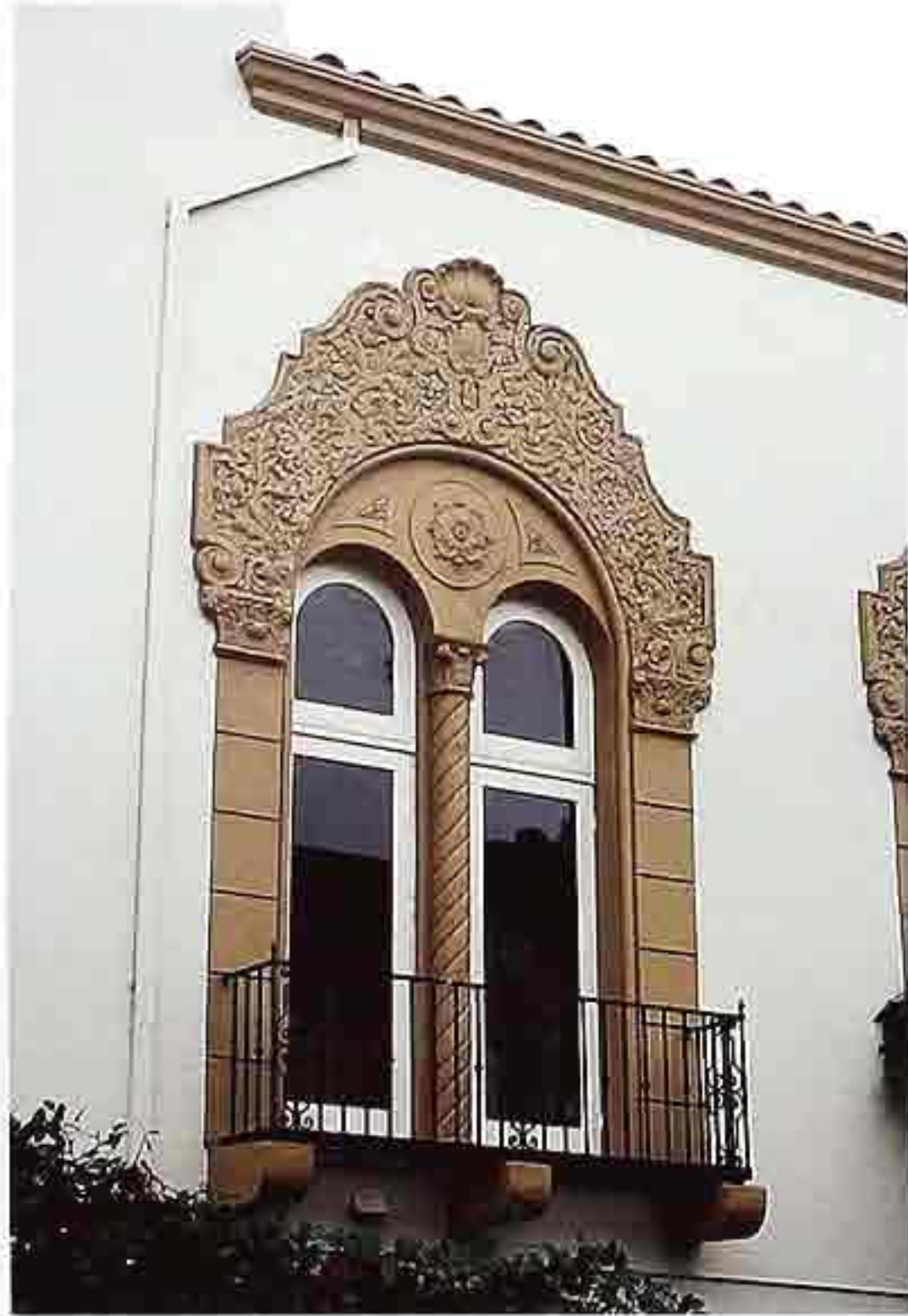
WI-150 Relief ornamental panel and pilasters around variation of Venetian-style window with balcony; 20th-c. apartment house
