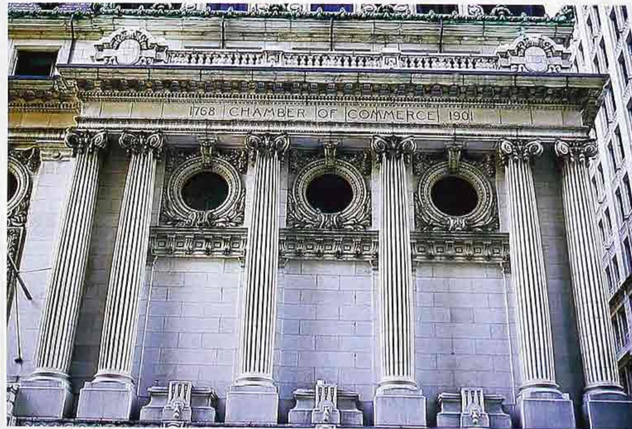
CP-75 Marble Ionic columns with fluted shafts; wall with bull's-eye windows; marble entablature
