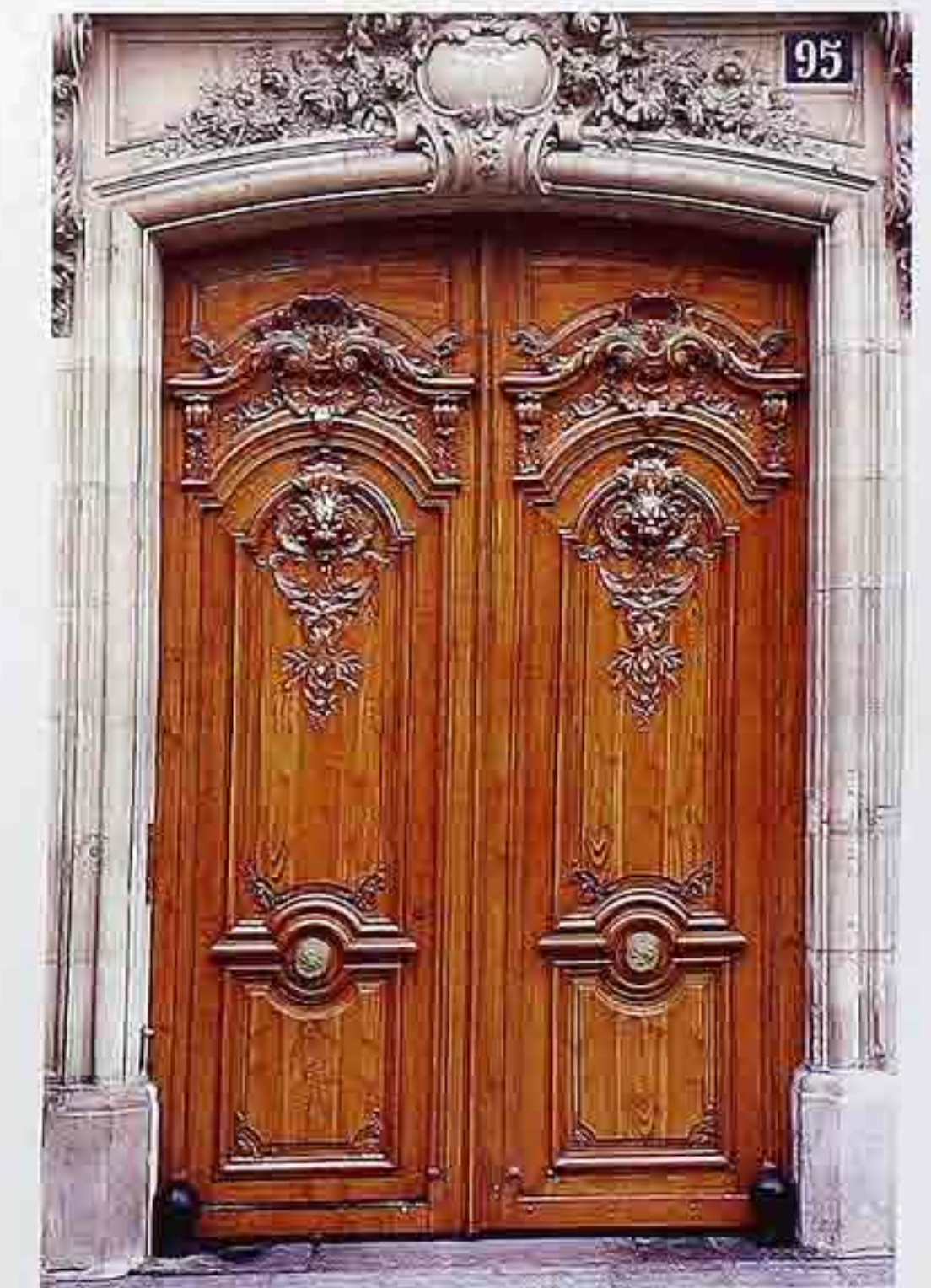
DW-8 Two panels, double doors with carved bas-relief ornament and trompe l'oeil wood finish. Cambered stone arch doorway with cartouche keystone
