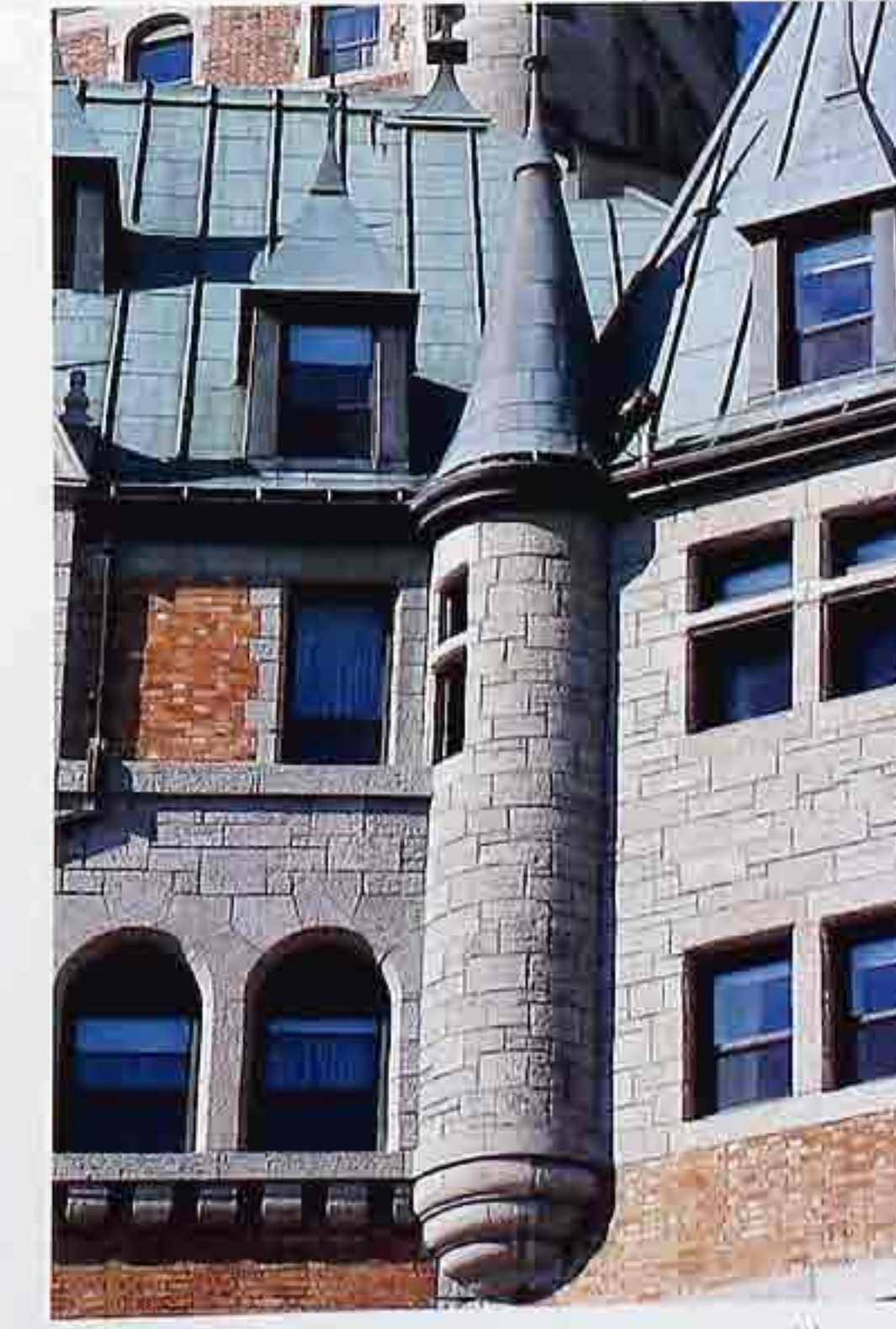
WA-289 Coursed ashlar on inside-corner turret with corbelled jetty and adjacent upper story; remaining walls of brick
