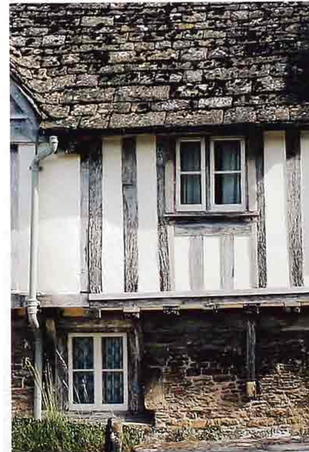
WA-280 Half-timbering; fieldstone under jetty, 16th- or 17th-c. English house
