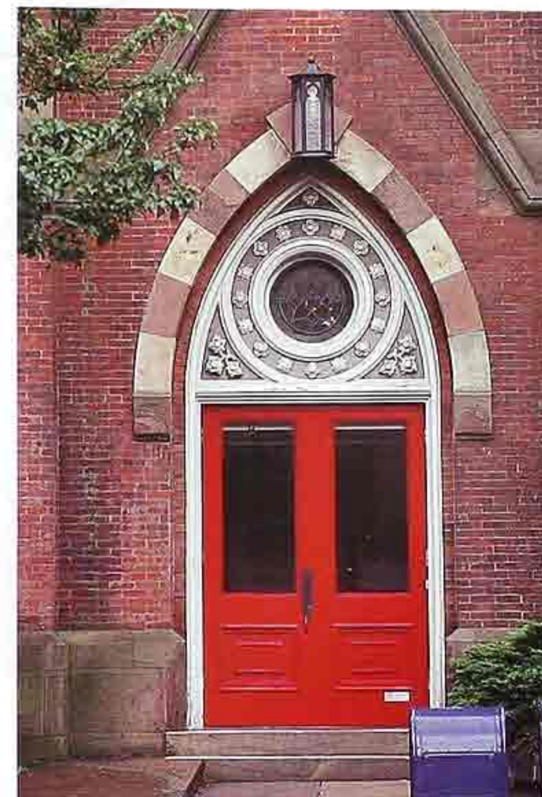
DW-76 Pointed arch in banded stone over carved stone transom panel with bull's eye window; two-paneled single-light double doors, brick church
