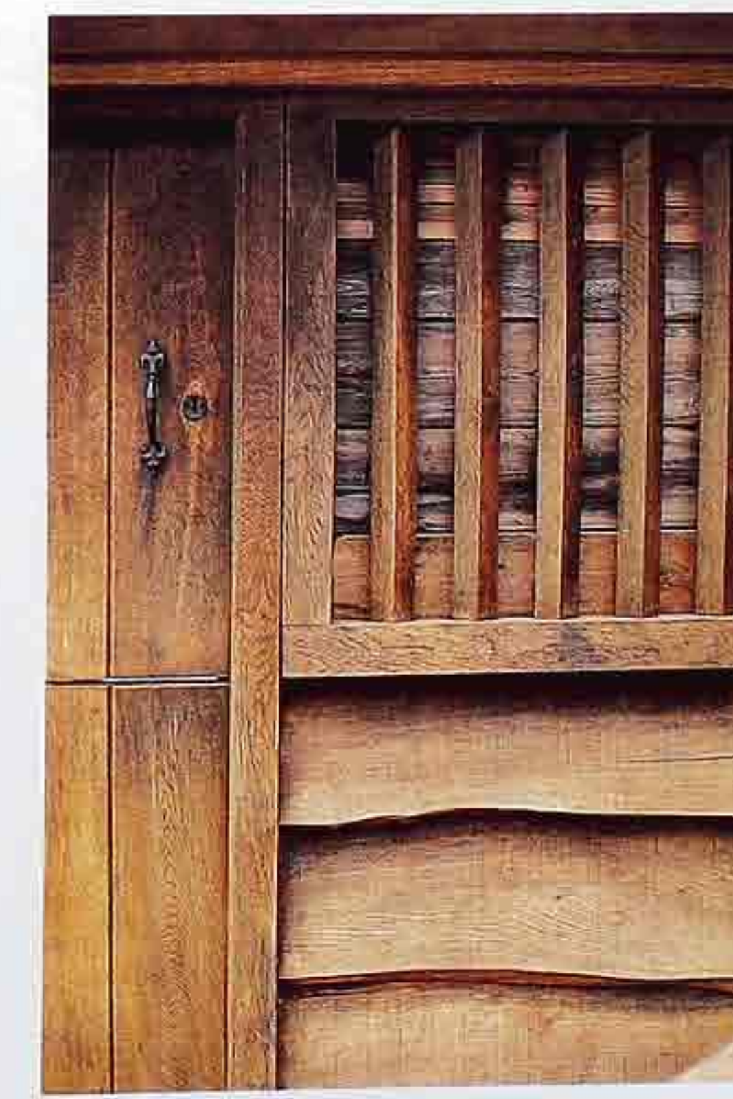
WA-8 Batten door (left); shutter behind diagonally split square-stock wood bars (upper right); elm waney-edged clapboard bottom (lower right) on an outbuilding
