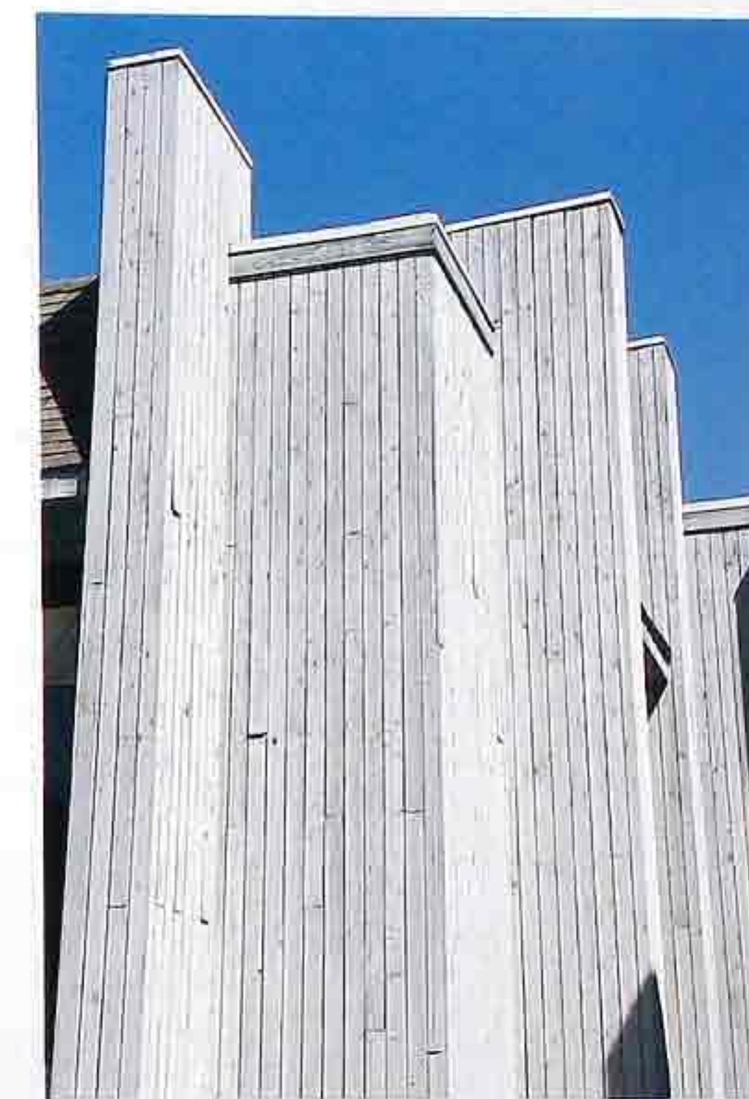
WA-48 Flush board siding, modern commercial building
