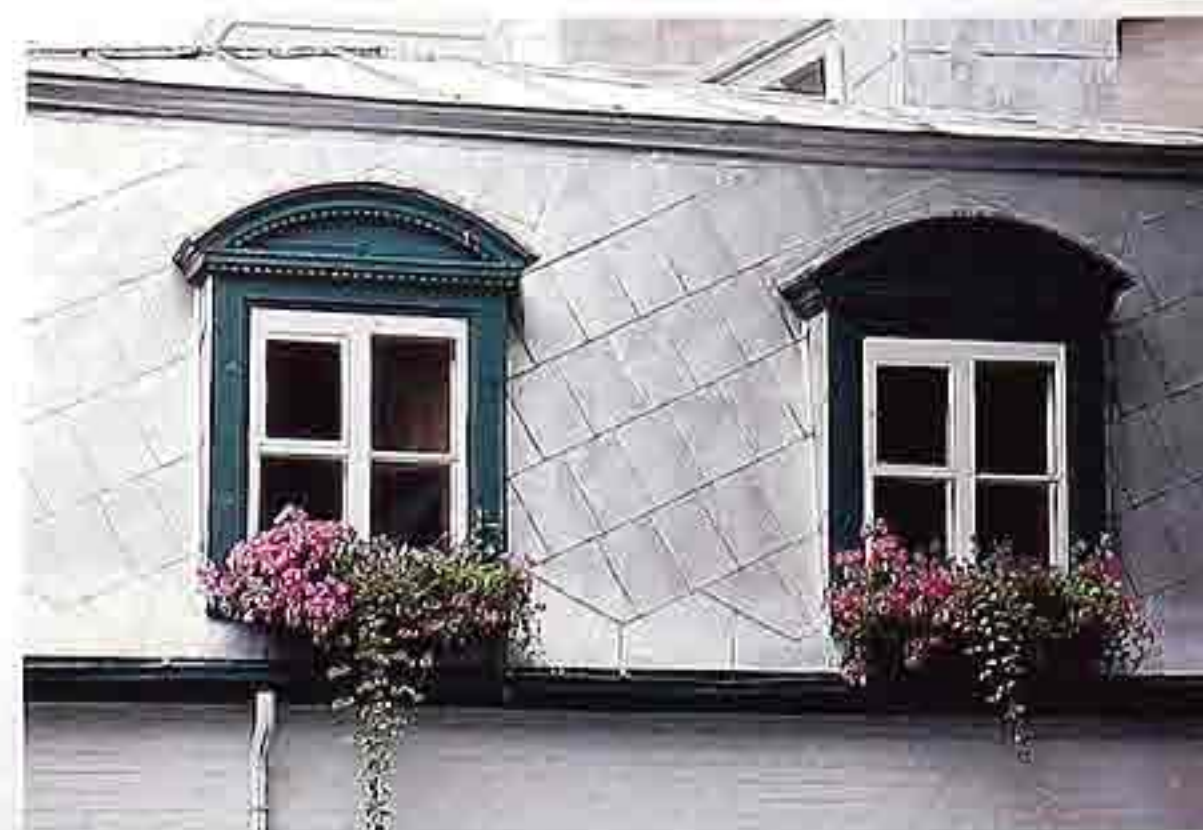
CR-98 Segmental-arch roof dormers on mansard roof with metal shingles
