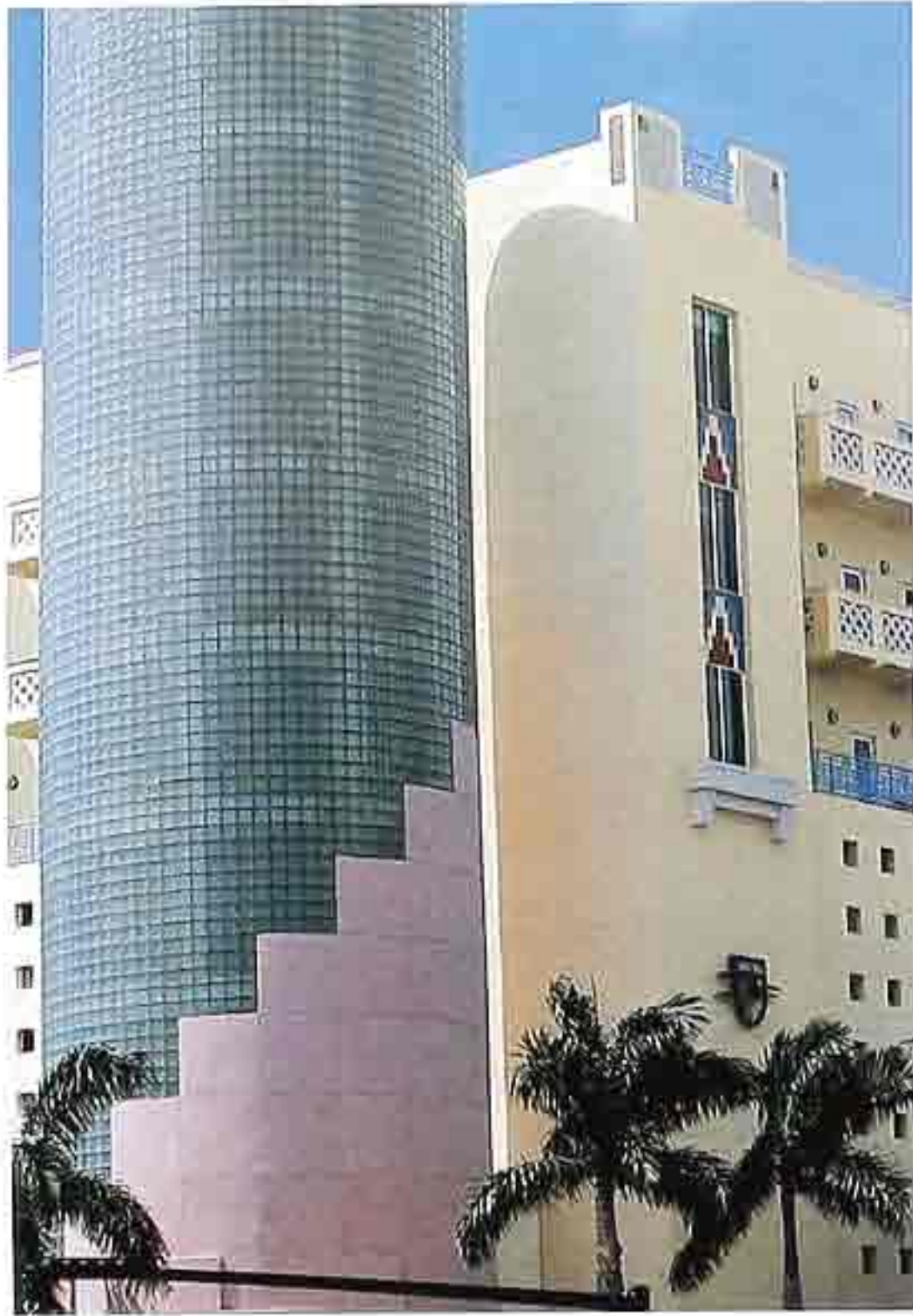
WA-306 Glass-block tower with stepped cast concrete at base next to cast-concrete Art Deco-style modern residential building
