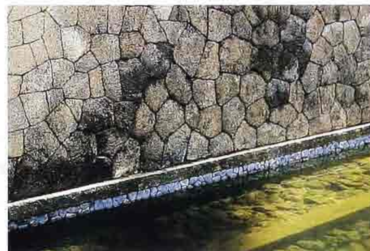
WA-63 Pool wall in hammered-finish sandstone with mosaic bond and water-line courses of roughly squared stone and beach pebbles
