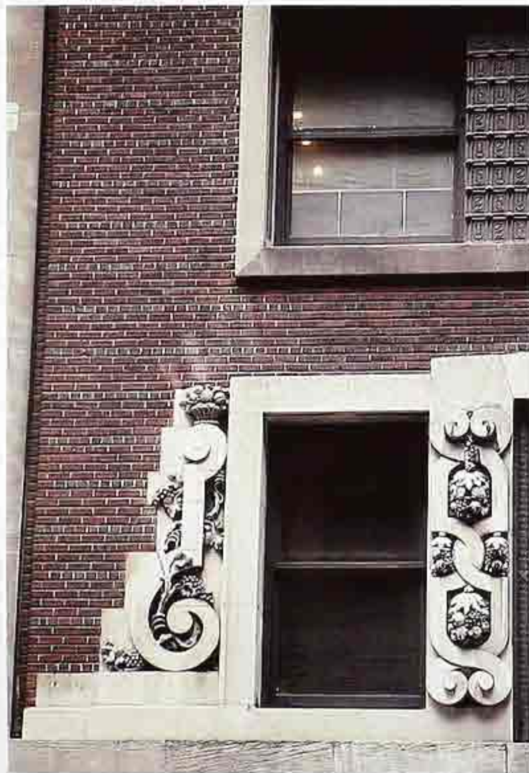
WI-134 Stone eclectic ornament flanking metal replacement window, apartment house
