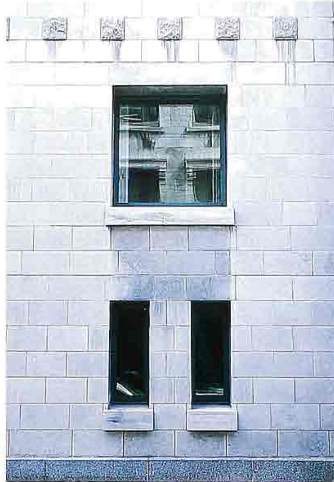
WA-139 Stone in running bond with projecting window sills and rock-faced decorative blocks, modern commercial building
