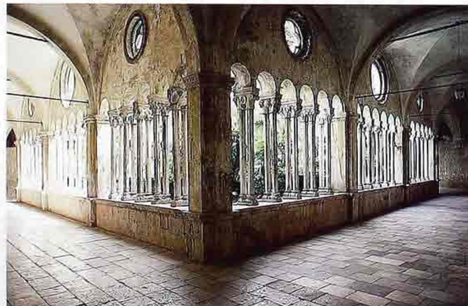
CP-166 Groin-vaulted arcade with multipart vaults and arches
