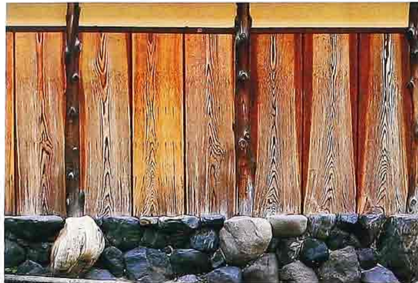
WA-44 Weathered unfinished plain-sawn planks with vertical undressed timbers on rubble foundation
