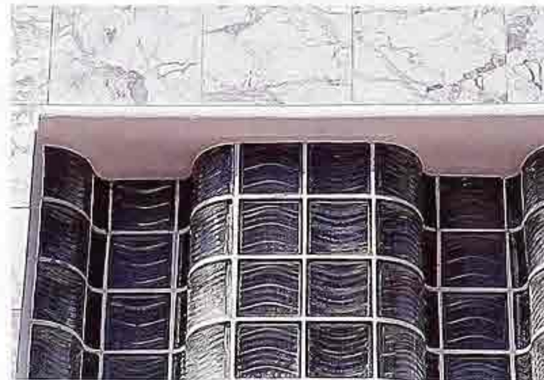
WI-22 Undulating window: flat and curved glass block with wavy texture, Art Deco apartment building
