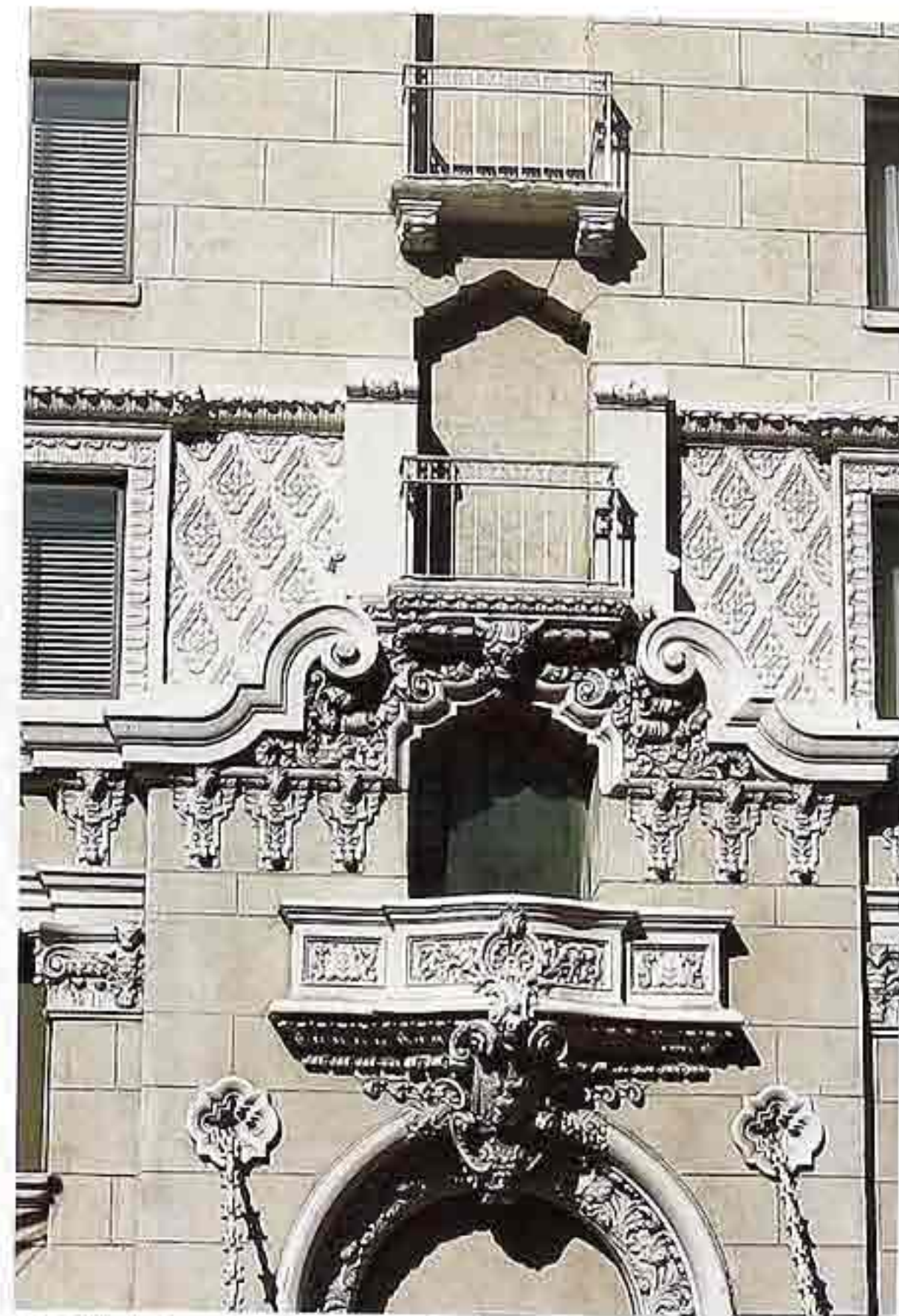
FA-113 Balconies over portal, broken pediment, and ornate details on multistory masonry facade
