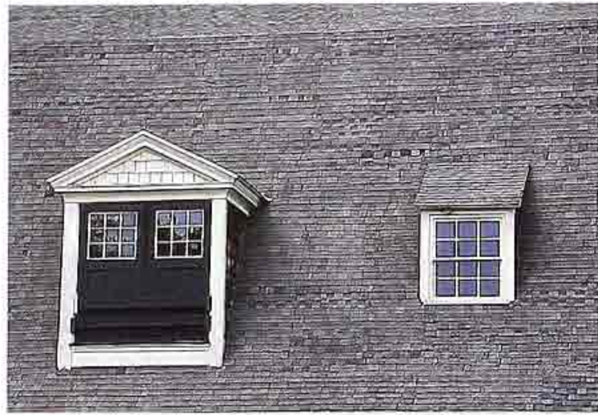
CR-93 Pedimented gable roof dormer and shed-roof dormer
