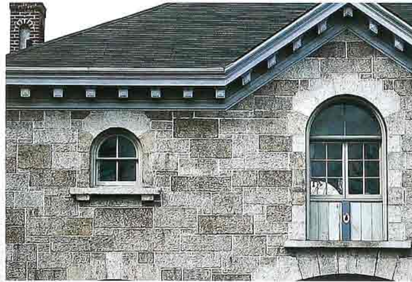
WA-123 Gable-end wall in random ashlar; block modillion cornice; quoins around arched windows; corbelled window sill (left)
