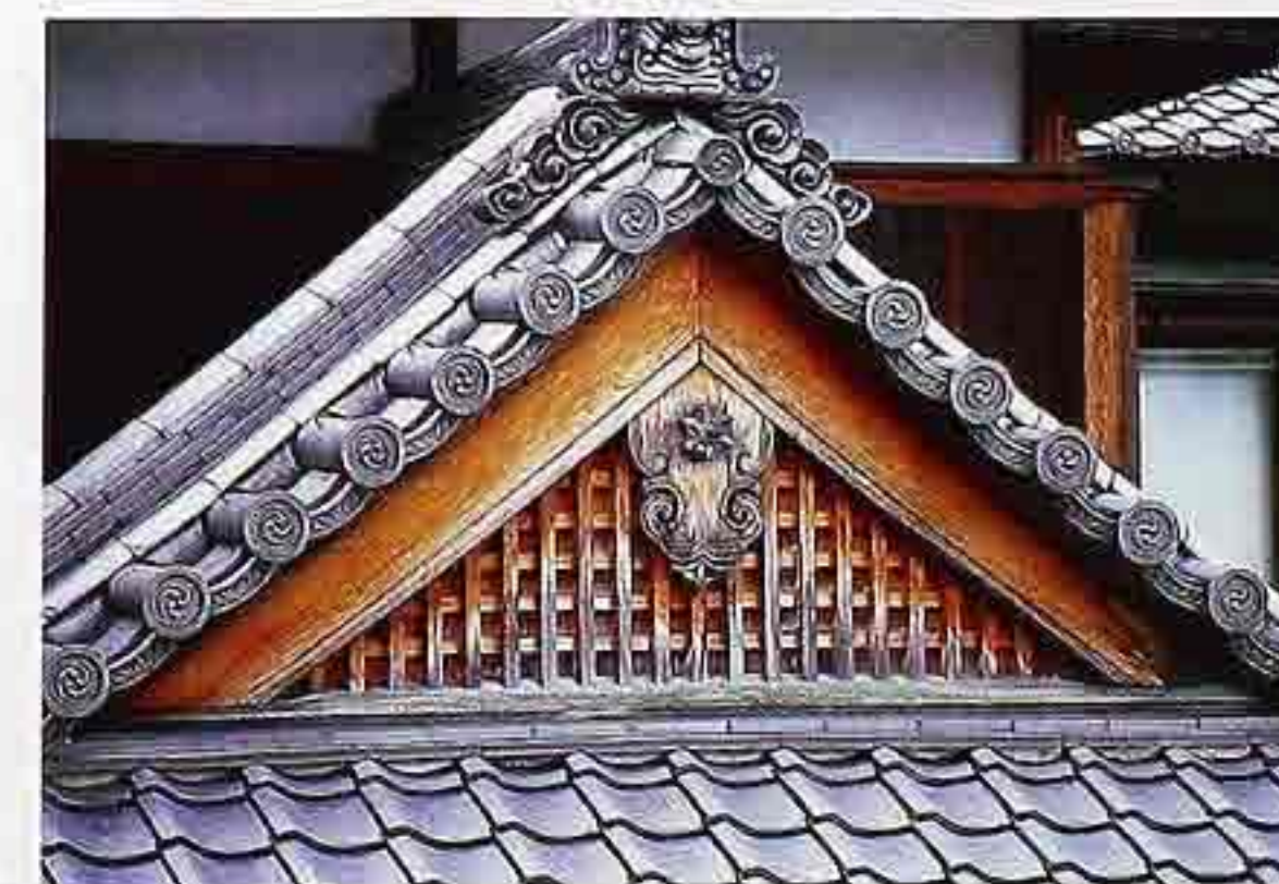
CR-84 Wood gable with lattice; ceramic tiles on gable roof and adjoining shed roof (bottom), Japanese temple
