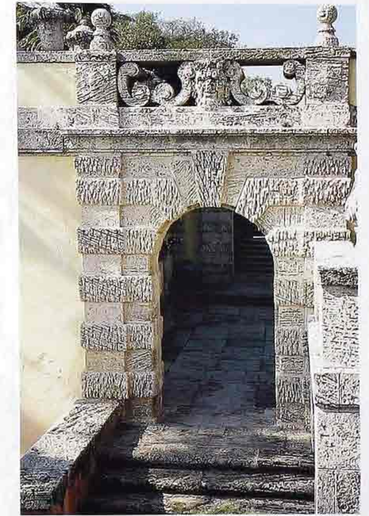
CP-168 Rusticated coquina garden portal with semicircular stepped arch, crossettes, banding, and ornamented balustrade with a mascarón
