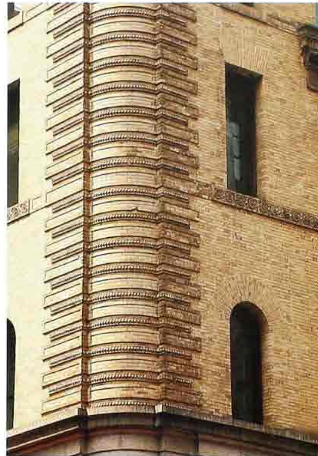
WA-190 Curved corner banded with courses of stretcher bricks and sculpted brick or architectural terracotta
