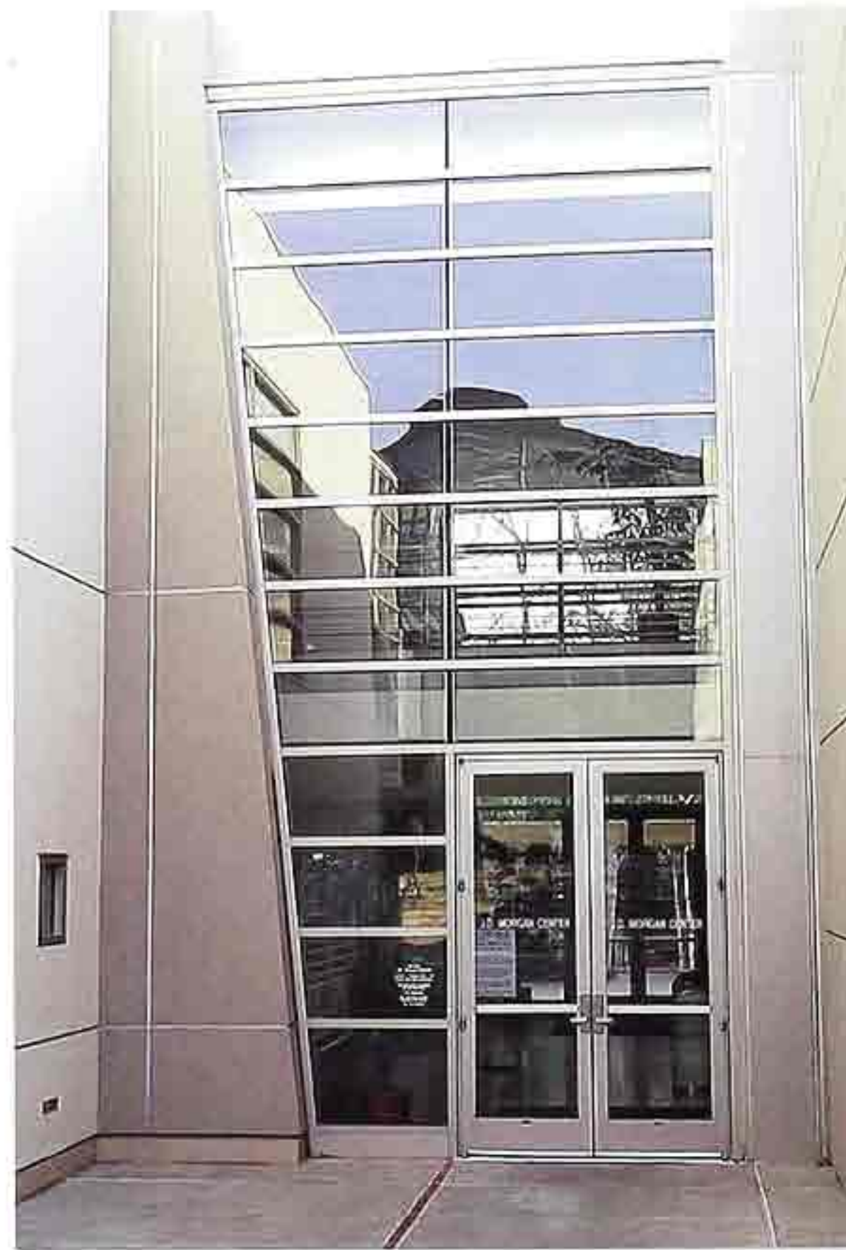
DW-102 Covered entryway: stainless steel double doors with full glass set in glass-paneled wall; masonry surround, modern commercial building
