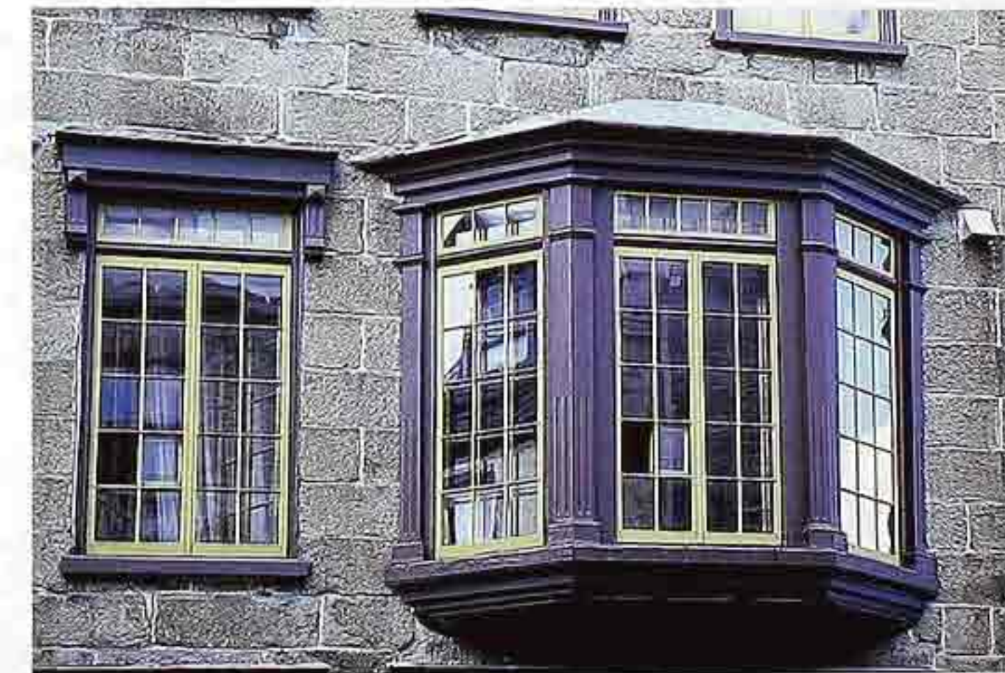
WI-84 Left: double-casement window; right: cant-oriel with fixed side and transom lights and center casement window, 19th-c. mixed-use building
