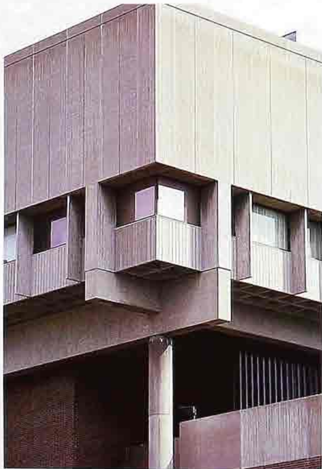
CP-132 Concrete column and beams, possibly pre-cast, supporting waffle slab
