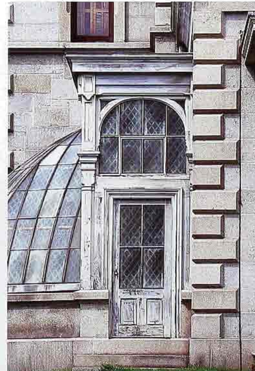
DW-78 Victorian conservatory entry: painted wood four-light door and transom light with etched glass; wood pilasters and crown molding; stone base
