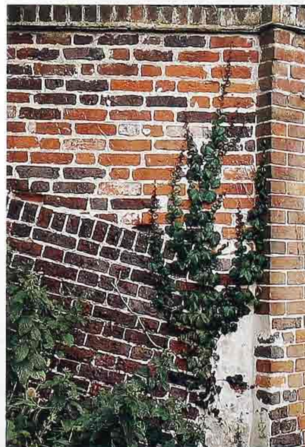
WA-151 Erratic Flemish bond with a sloping course and rowlock-course coping
