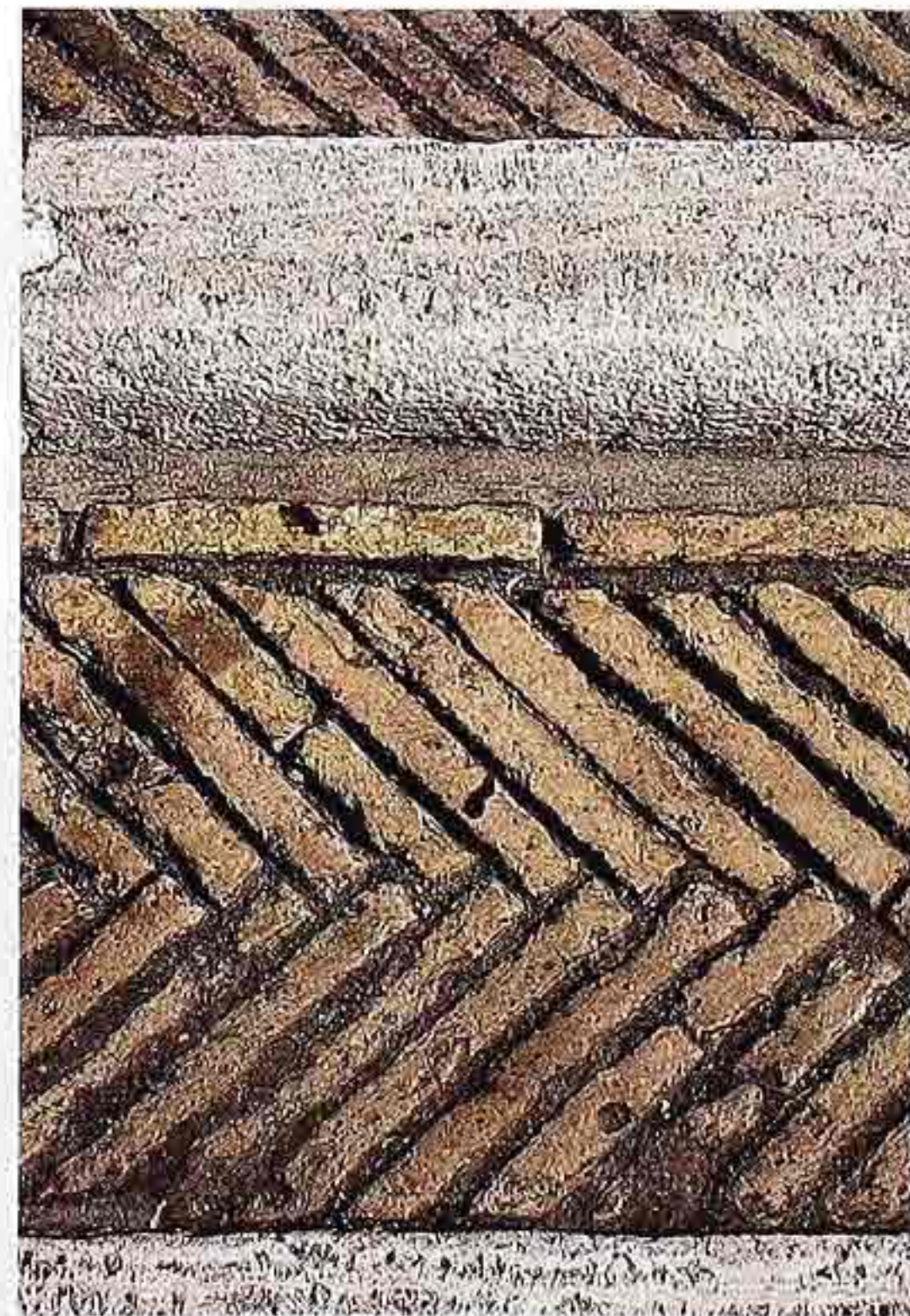
FP-63 Stone curb and Roman brick in herringbone pattern on ancient sidewalk
