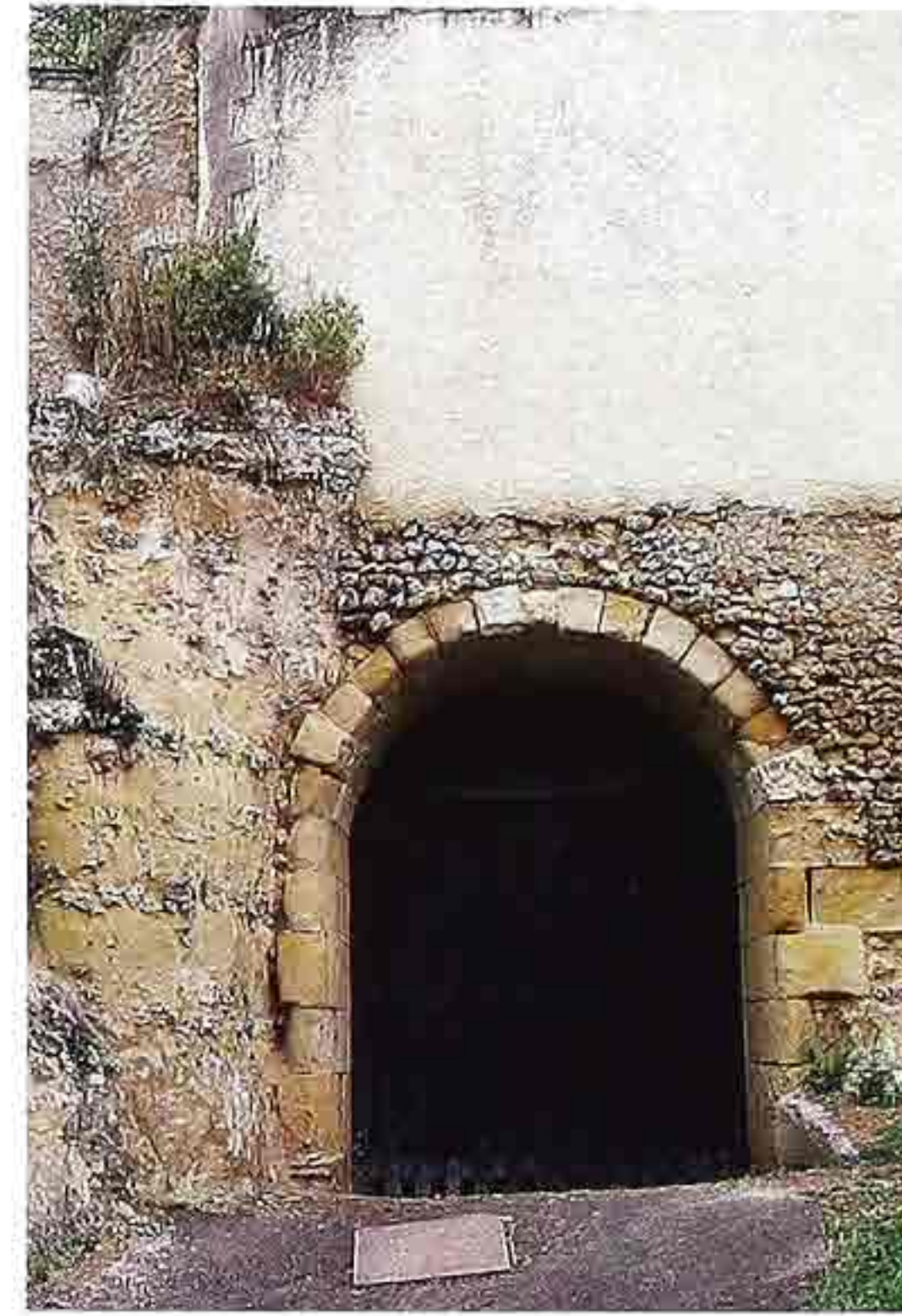
CP-150 Rustic semicircular masonry arch in rubble wall in natural rock formation
