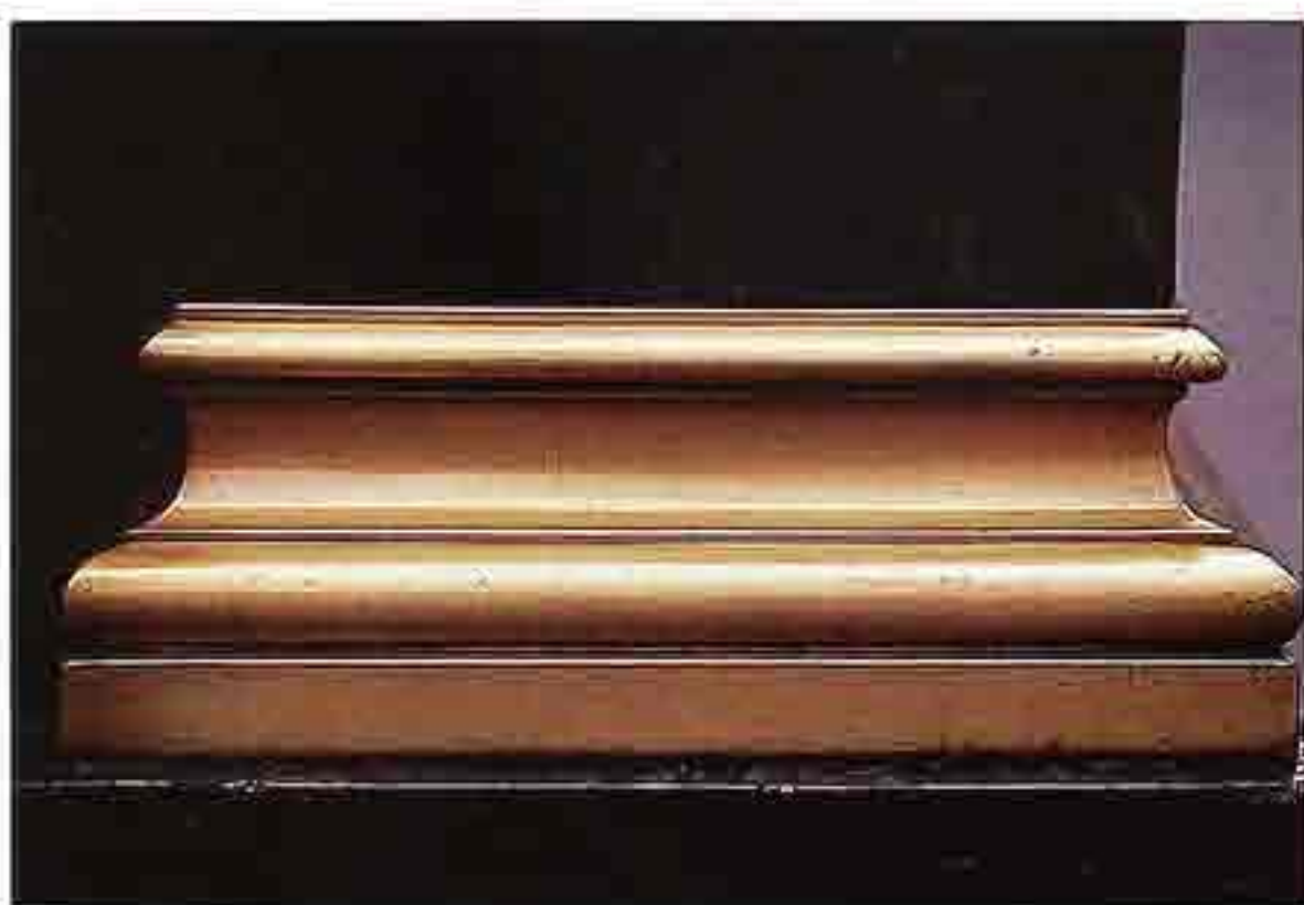
CP-51 Square metal base, Attic profile with enlarged scotia and diminished upper torus
