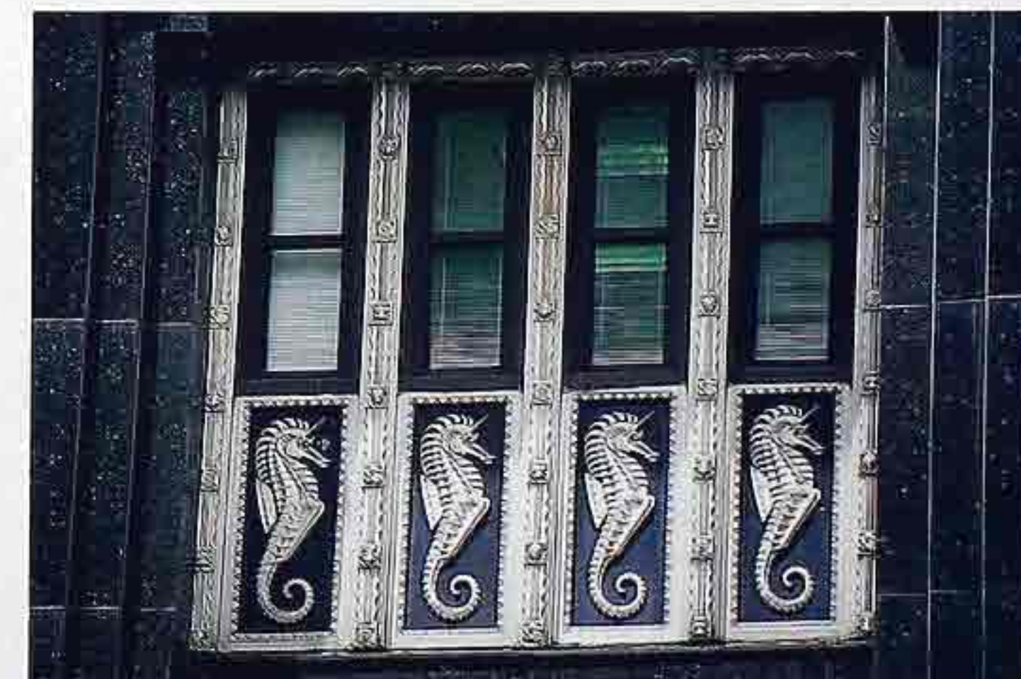
OM-8 Nickel-silver-plated bronze or cast stainless steel spandrel panels with seahorse ornament
