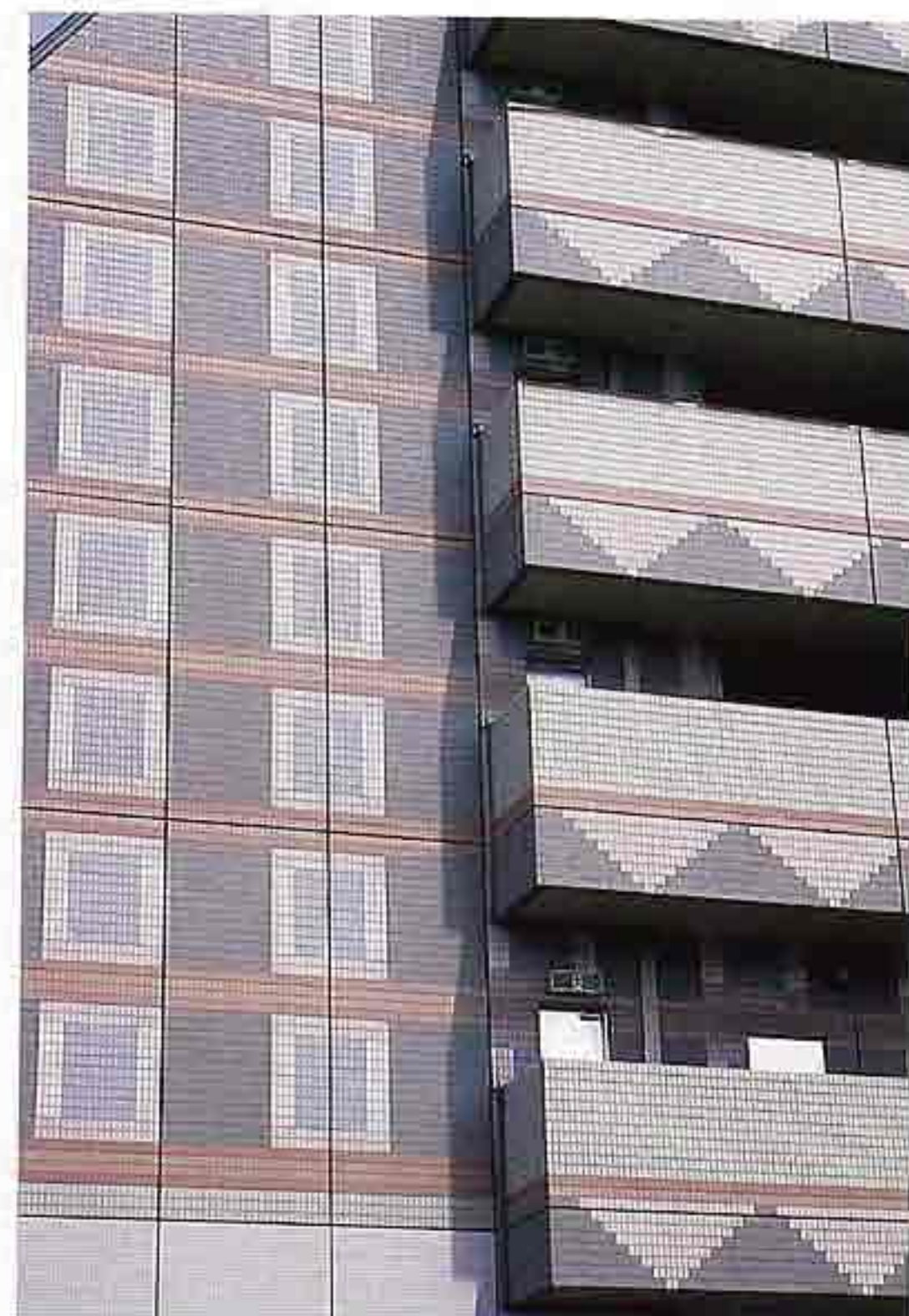
FA-71 Polychrome tiles in geometric patterns on walls and balconies of modern apartment house
