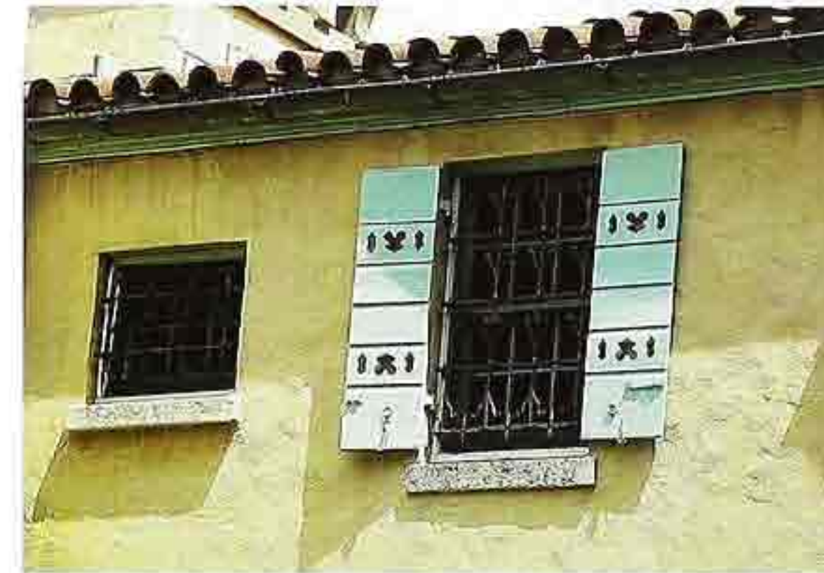
WI-191 Horizontal-board shutters with pierced design
