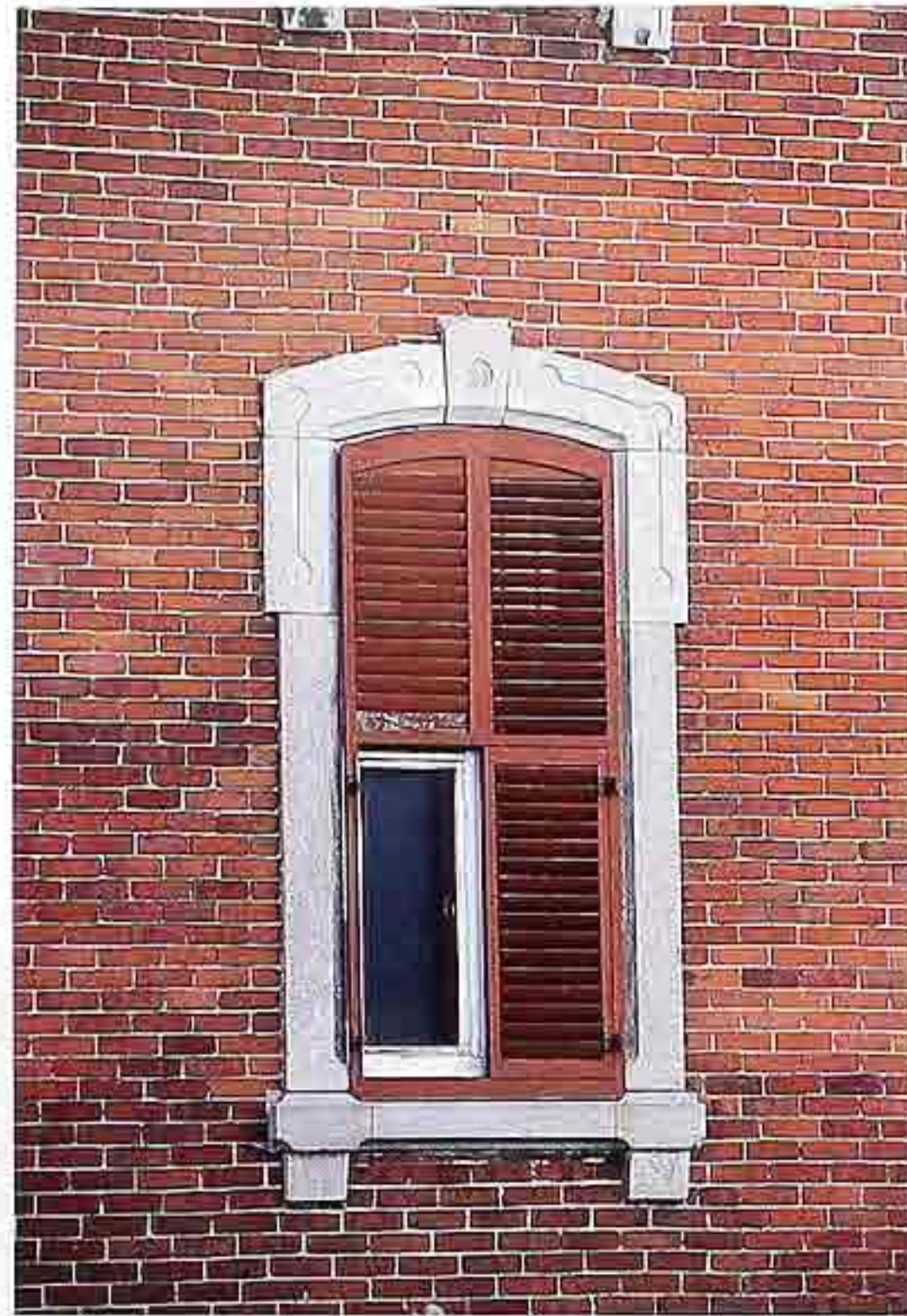
WI-183 Louvered shutters with fixed top shutters
