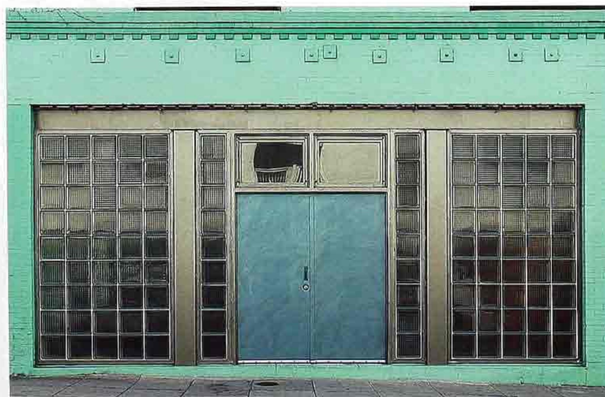
DW-103 Painted metal double doors flanked by side lights, stainless steel panels, and window wall
