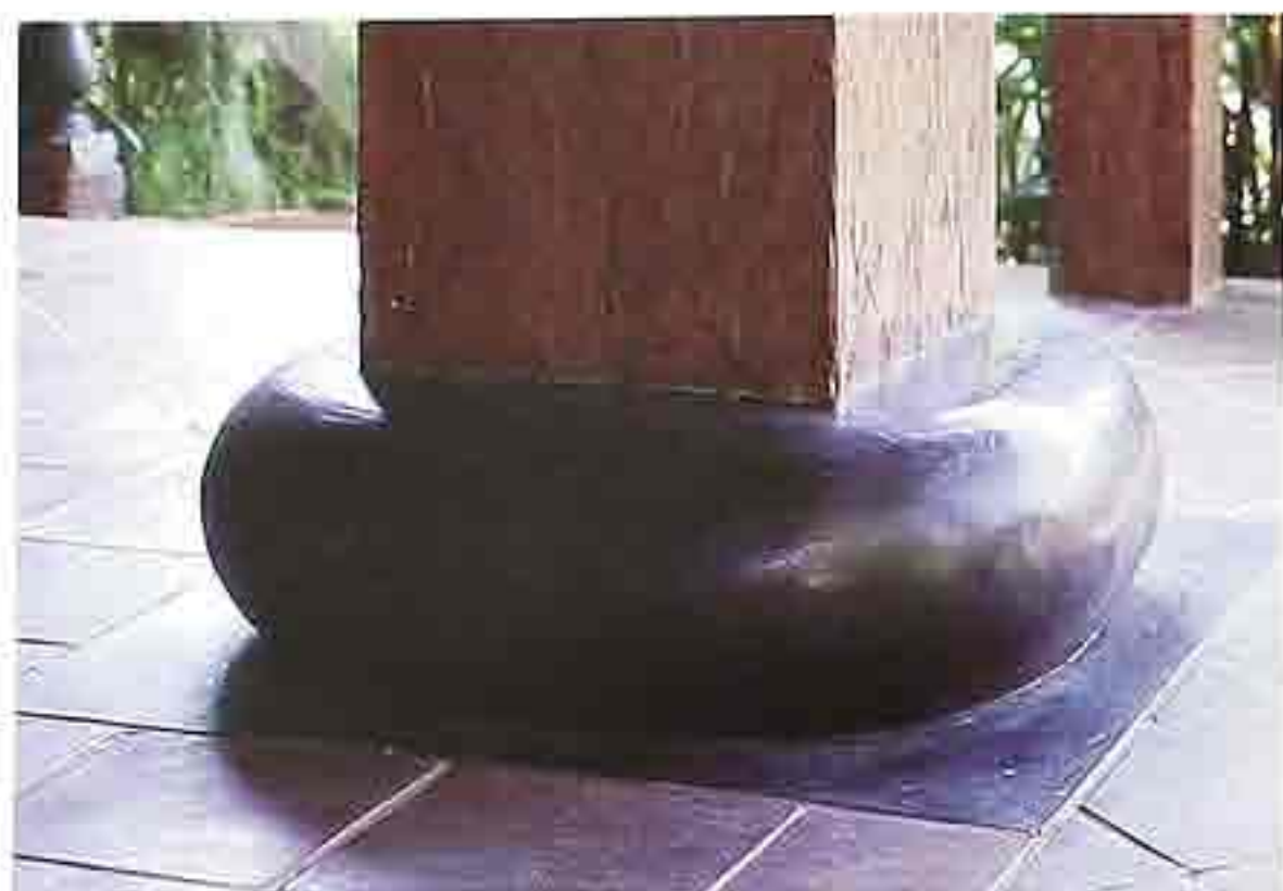
CP-49 Hand-hewn beveled timber post on a honed stone base with rounded edge
