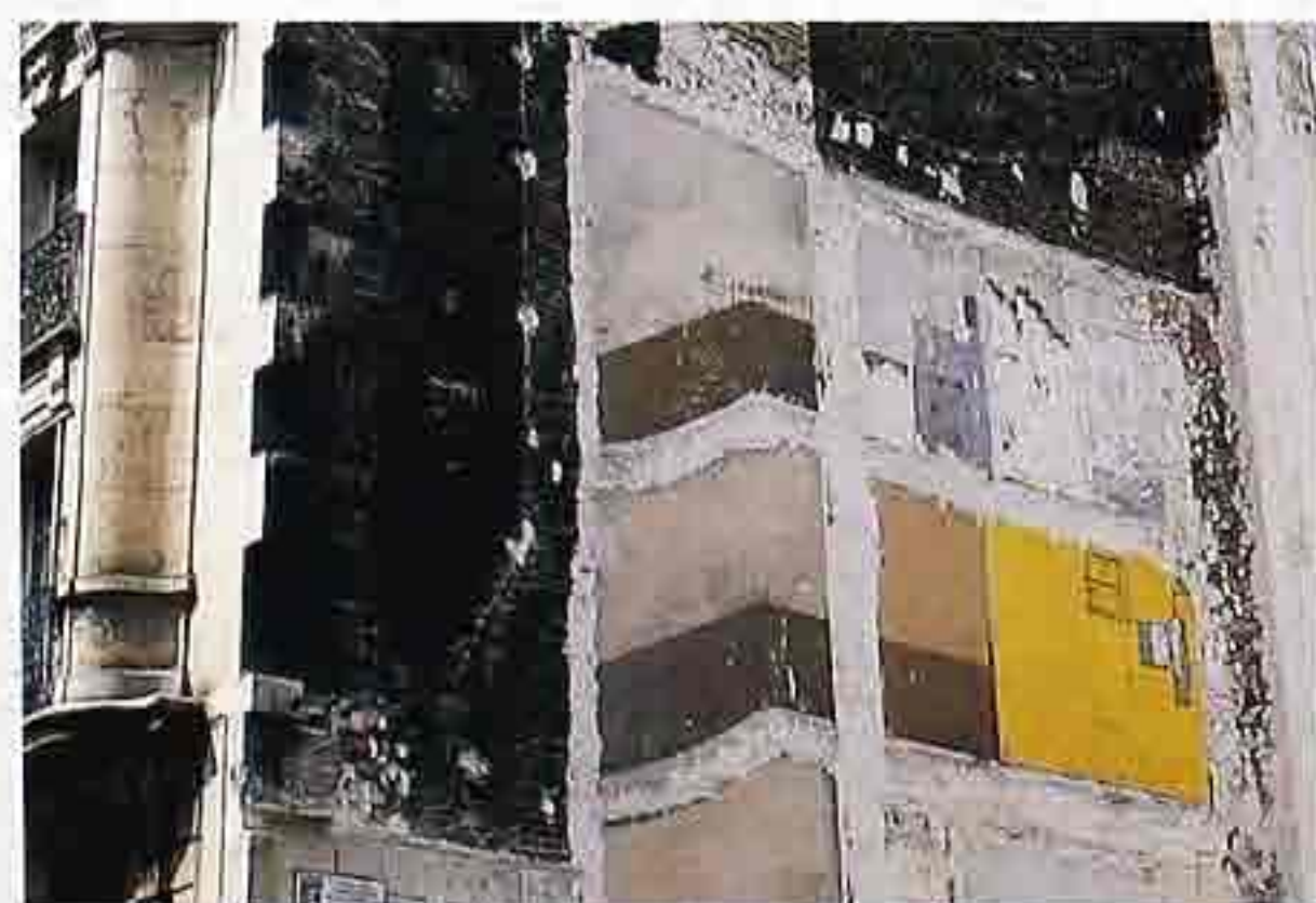
WA-258 Walls of plastered interior apartment walls exposed by demolition
