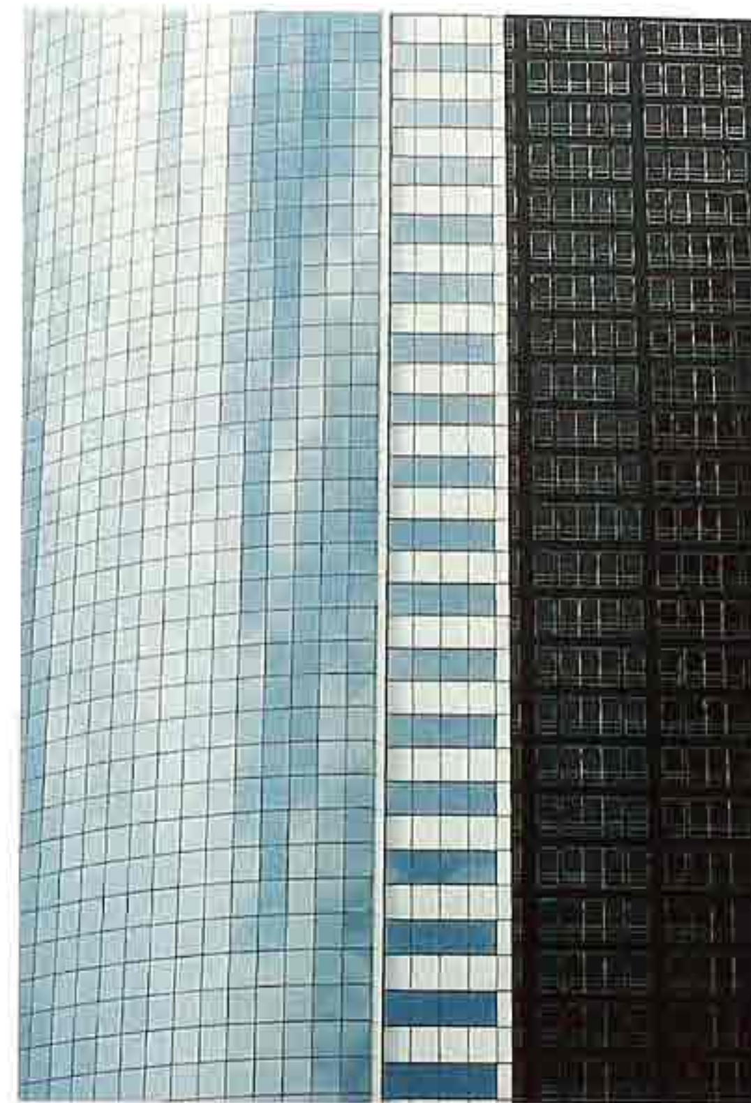
FA-36 Left to right: fully glazed; alternating solid spandrel panels and glazing; curtain-wall system with column covers and glazed units
