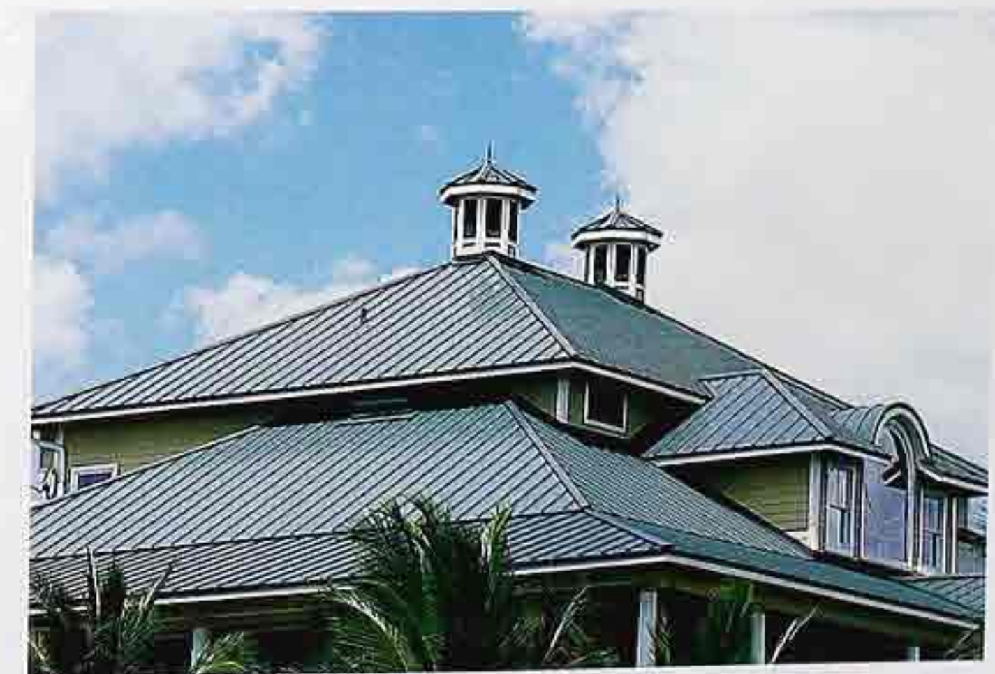
CR-139 Hipped roof with octagonal cupolas, metal with standing seams
