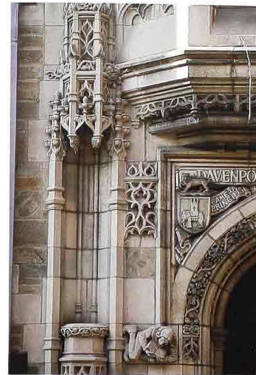
OM-43 Niche covered by a baldachin on Gothic-style entry
