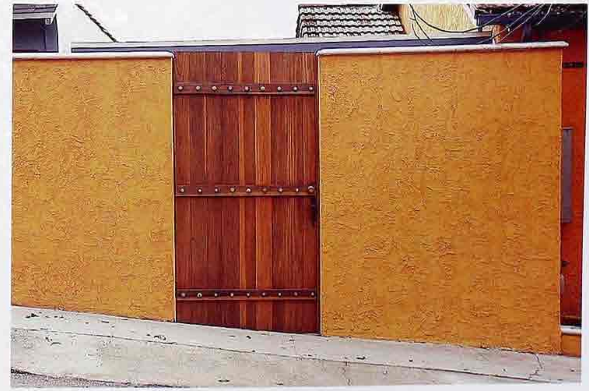
DW-29 Stained wood courtyard gate with horizontal braces, set in painted stucco wall
