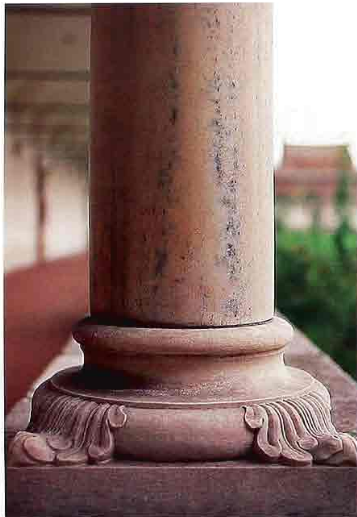
CP-31 Idiosyncratic marble Attic base with foliated ornament draped over torus on plinth
