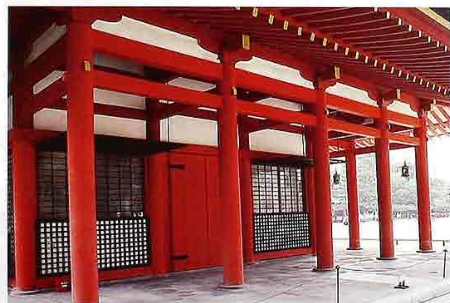
CP-140 Post-and-beam construction, Japanese temple
