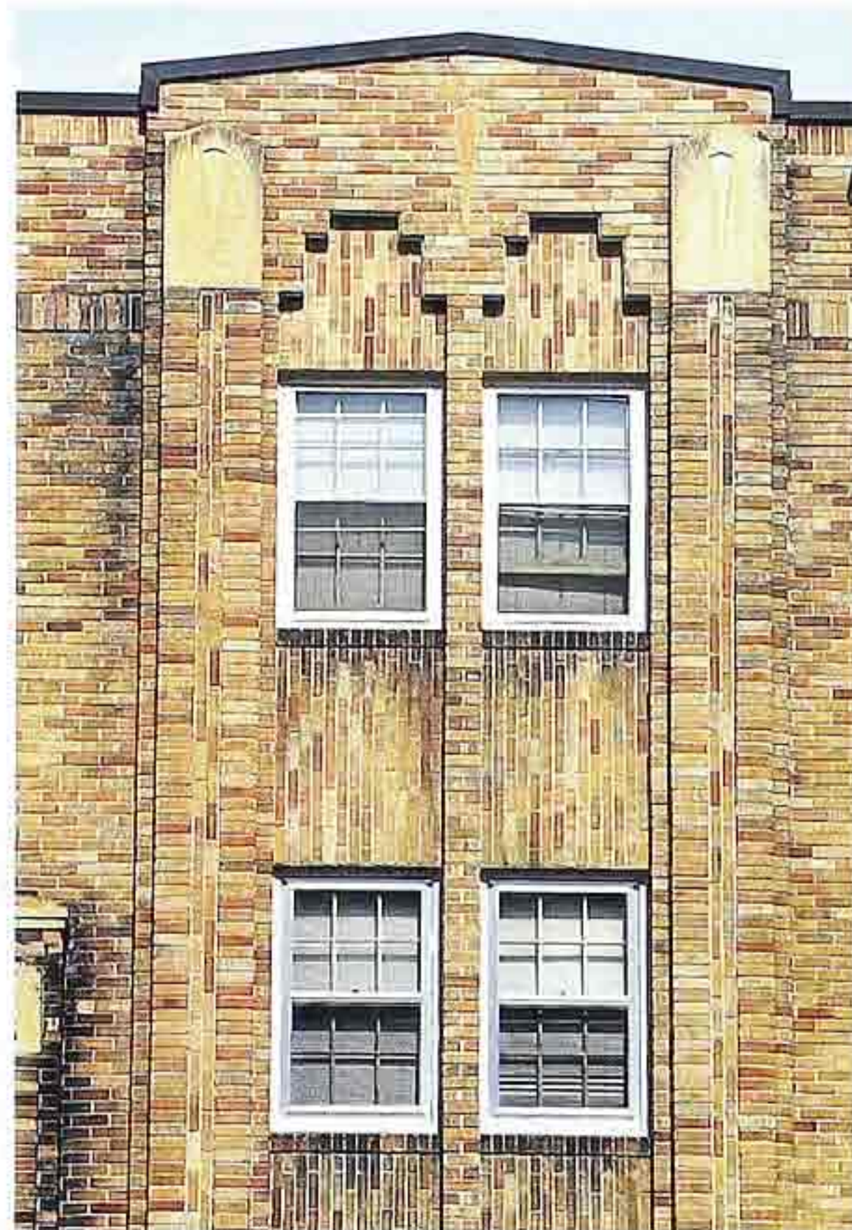
WA-184 Idiosyncratic collection of stacked bond and horizontal and vertical running bonds on pilasters and spandrels; rowlock window sills
