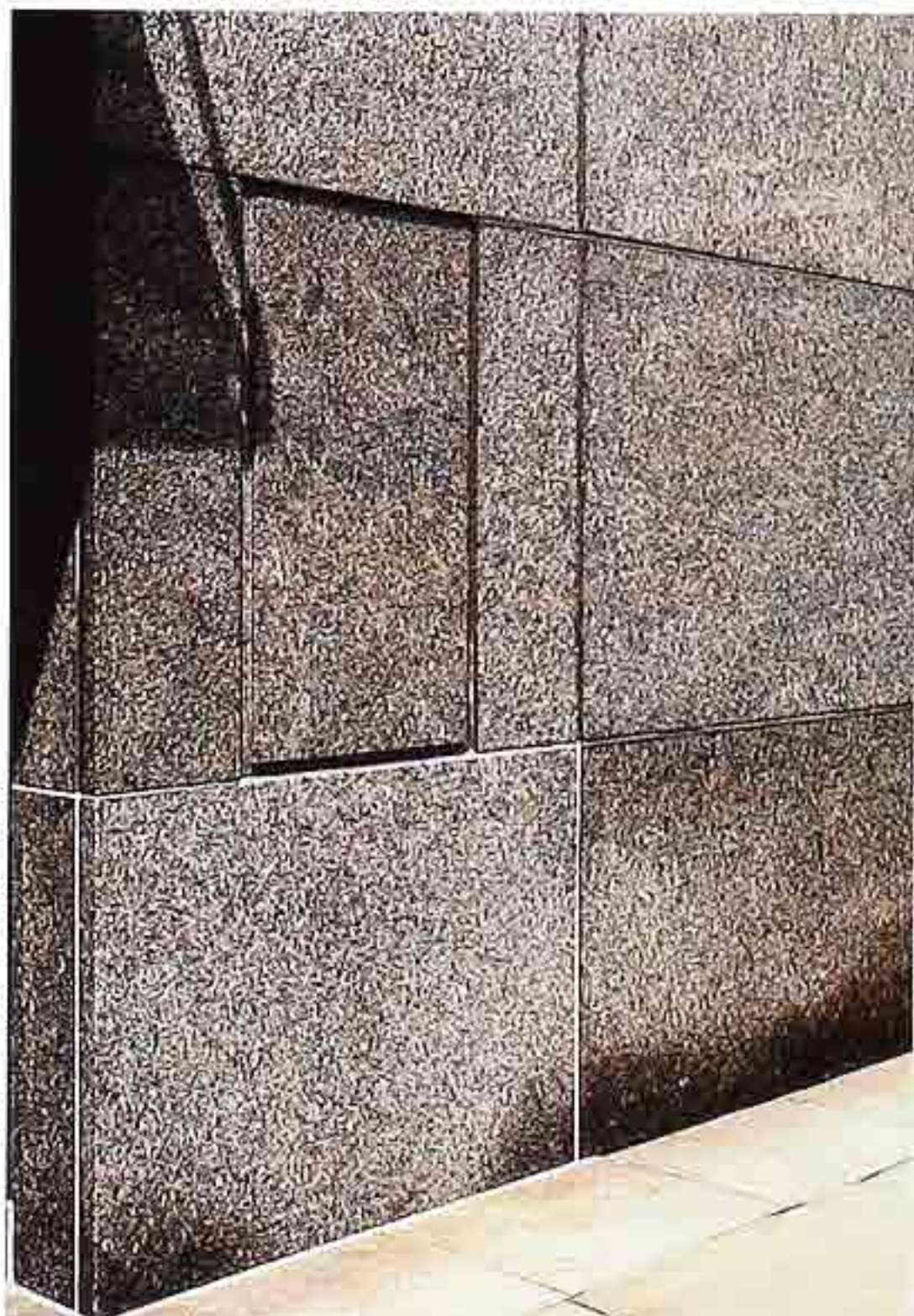
WA-85 Honed granite veneer in stack bond with grouted joints
