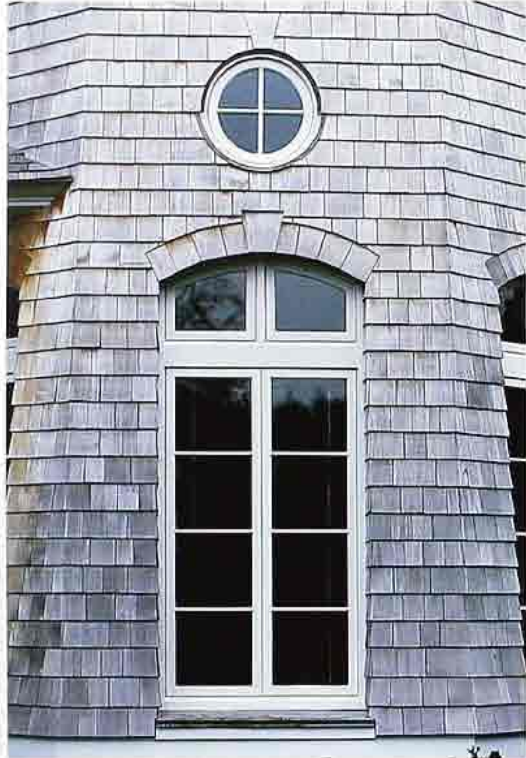
WI-94 Segmental-arch transom light with shingle "voussoirs" and "keystone" above French door, modern shingle house
