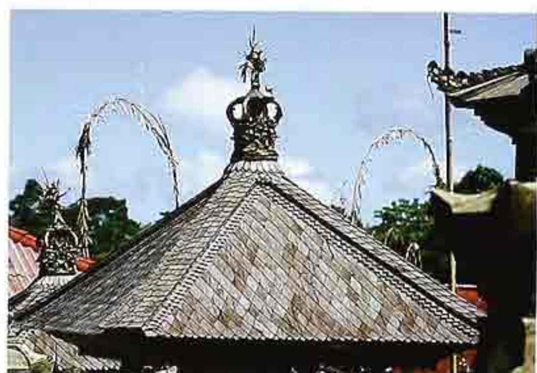
CR-67 Wood shingles on hipped roof with antefix, Balinese shrine
