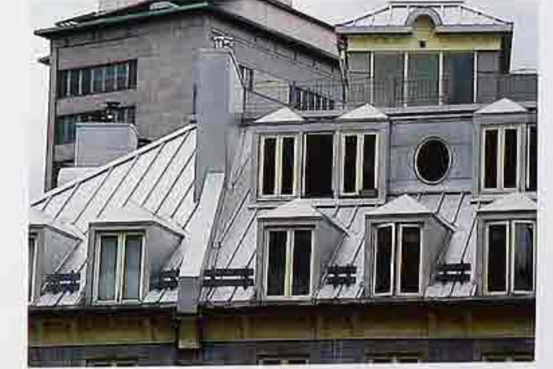
CR-102 Hipped-roof dormers on metal hipped roof with pipe snow guards, modern apartment house
