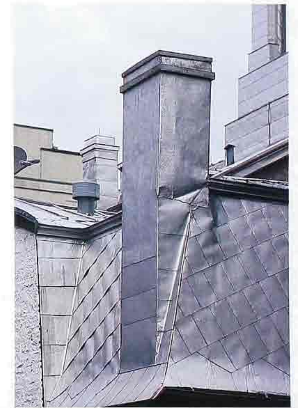
CR-152 Flat-seamed metal chimney on diagonal flat-seamed metal roofing
