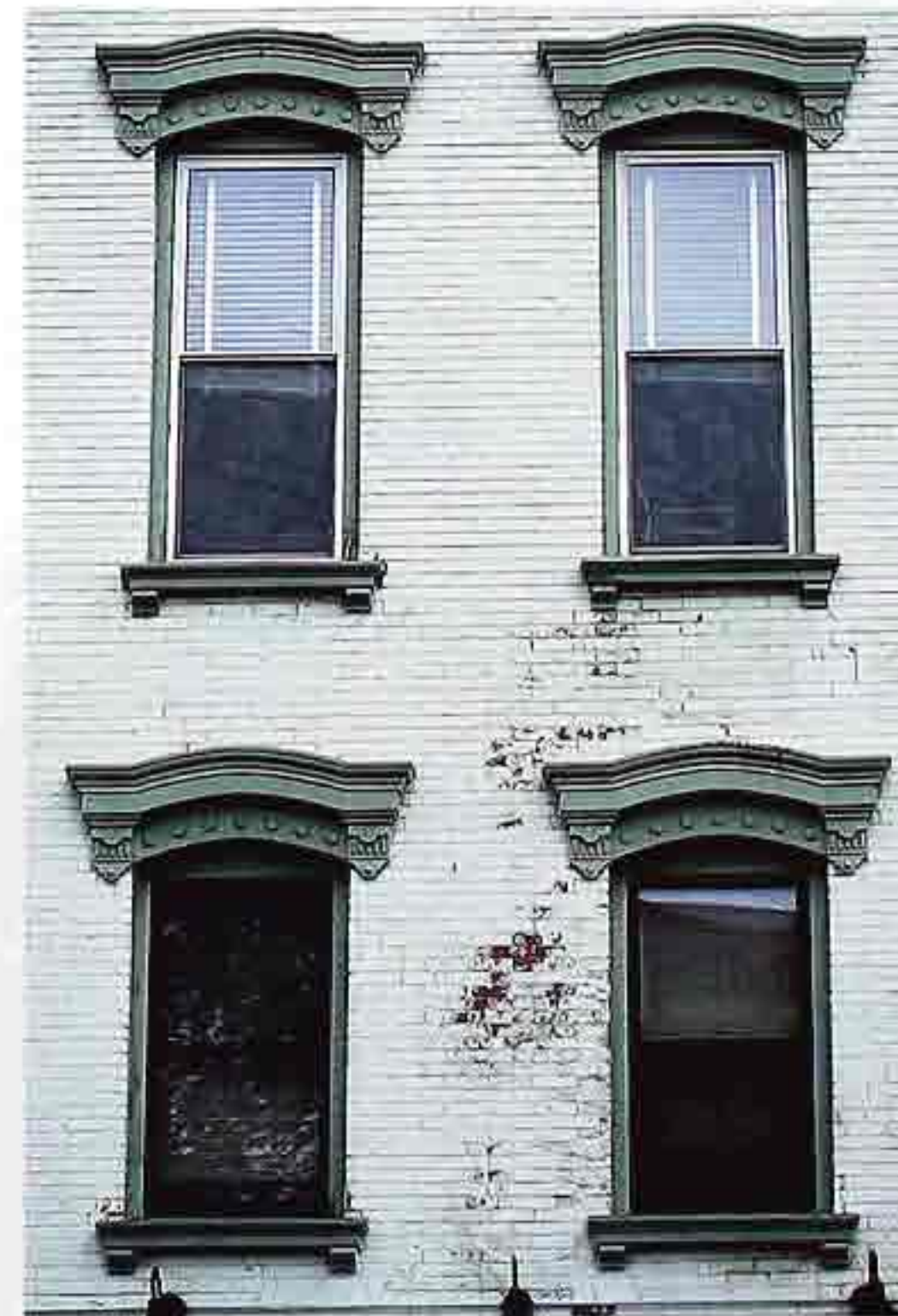
WI-109 Flat trim echoing arch profiles of window openings, 19th-c. American mixed-use building
