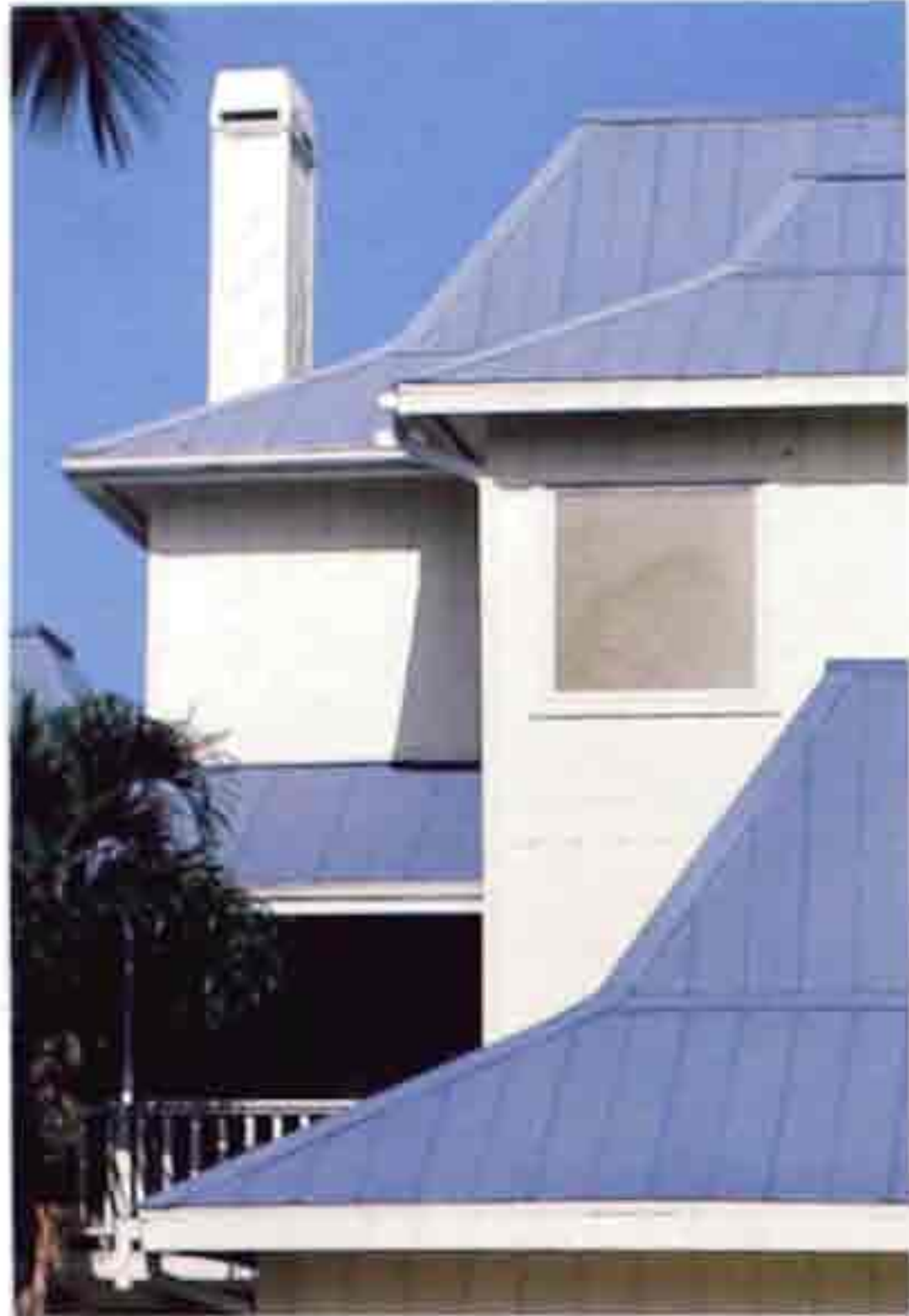
CR-30 Anodized aluminum or coated sheet steel with standing seams, variation of hipped roof, modern house
