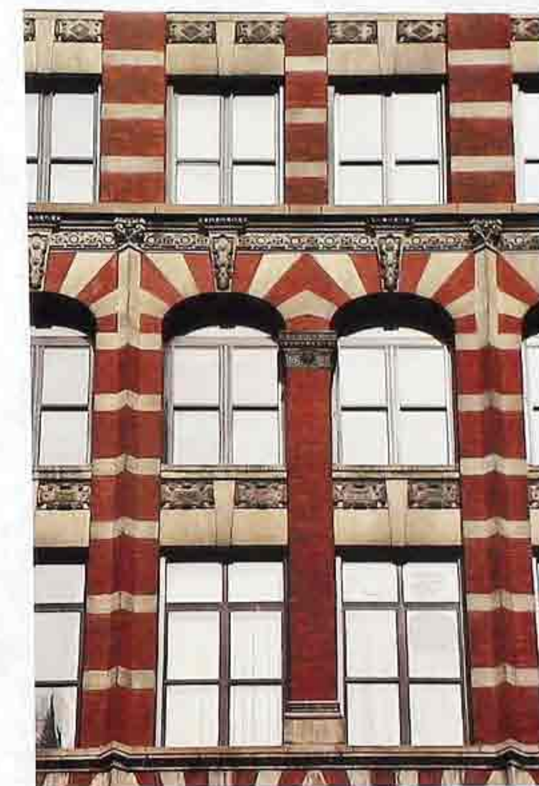
WA-287 Banded brick-and-stone arches with carved ornament in keystones and spandrels
