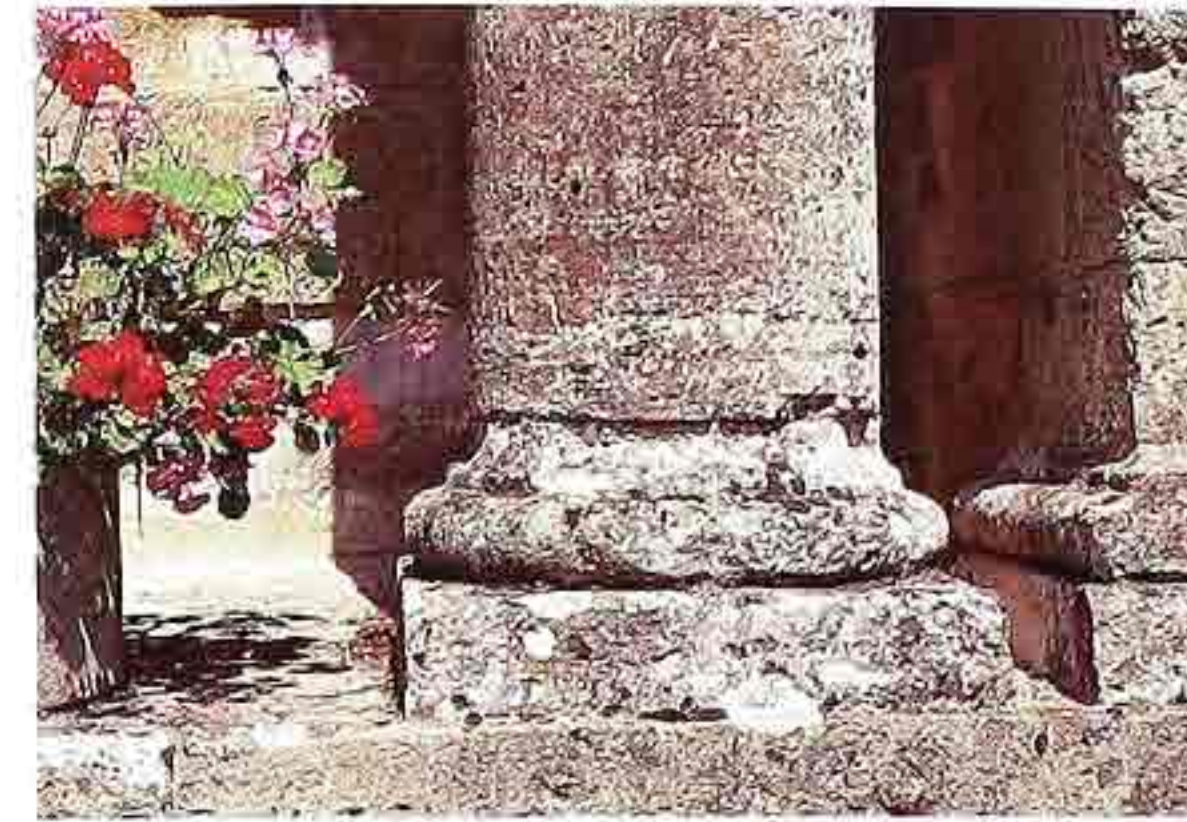
CP-35 Doric base of heavily weathered volcanic stone column on square plinth
