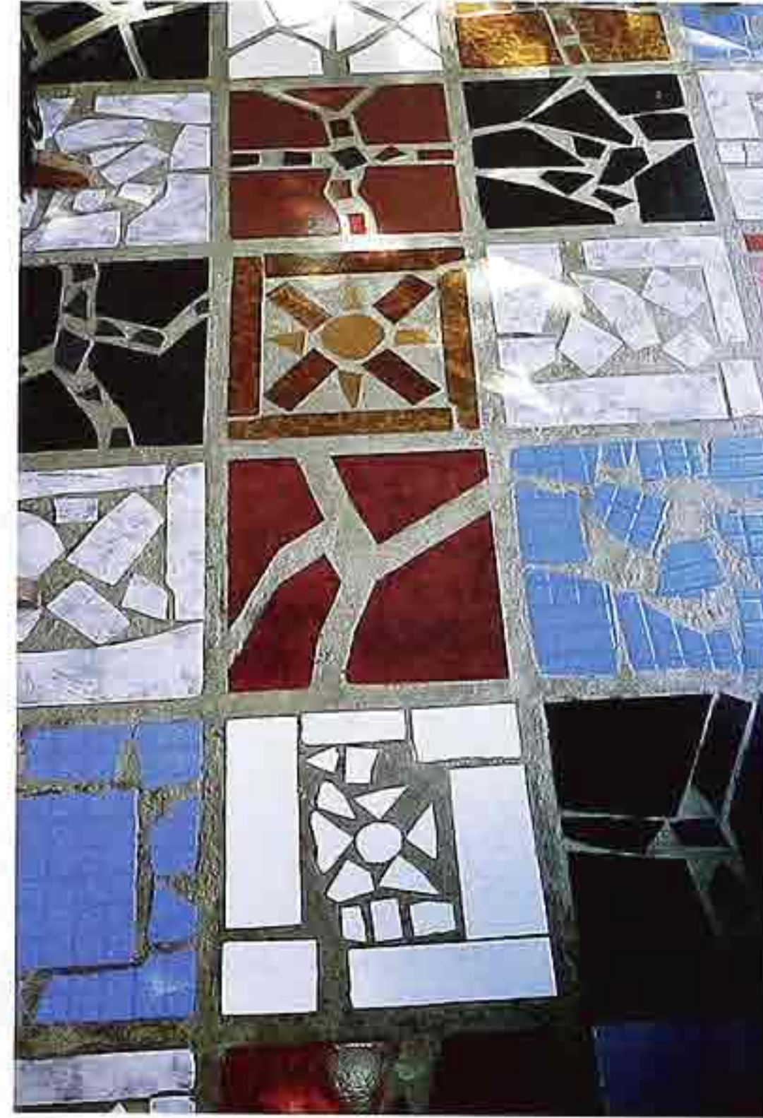
FP-104 Random-shaped tile pieces used as tesserae in mosaic grid design set in concrete
