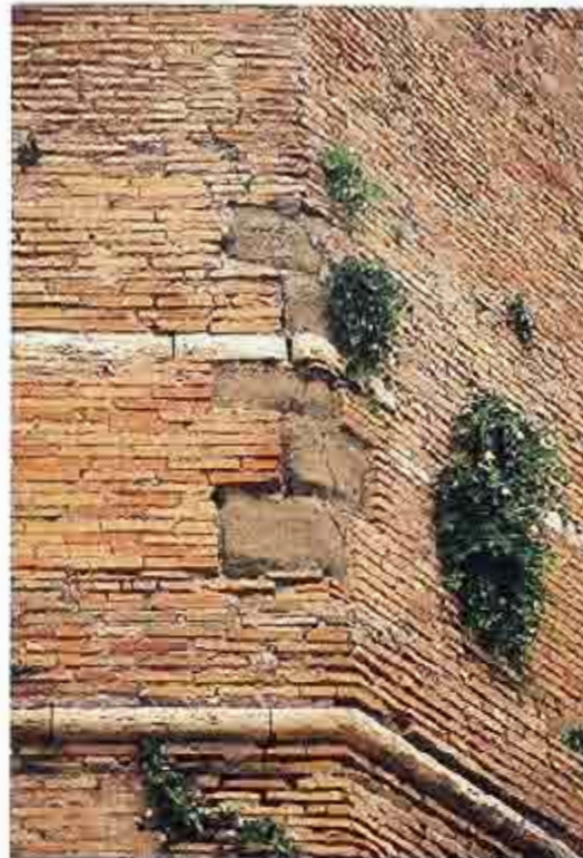
WA-159 Ancient Roman brick running-bond wall with stone quoins, banding course, and bead molding
