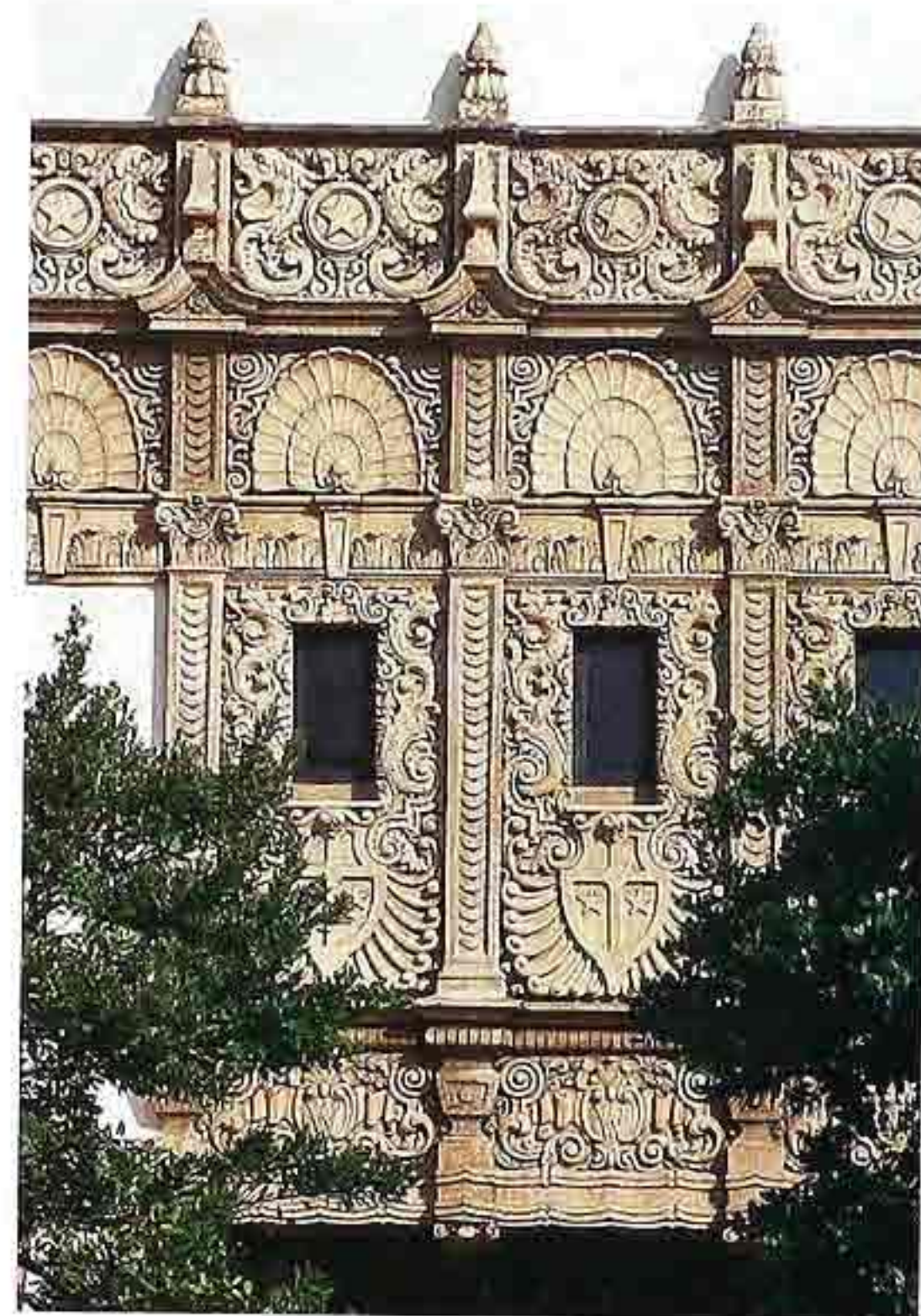
FA-60 Ornate banded stone-finish architectural terracotta facade with pilasters
