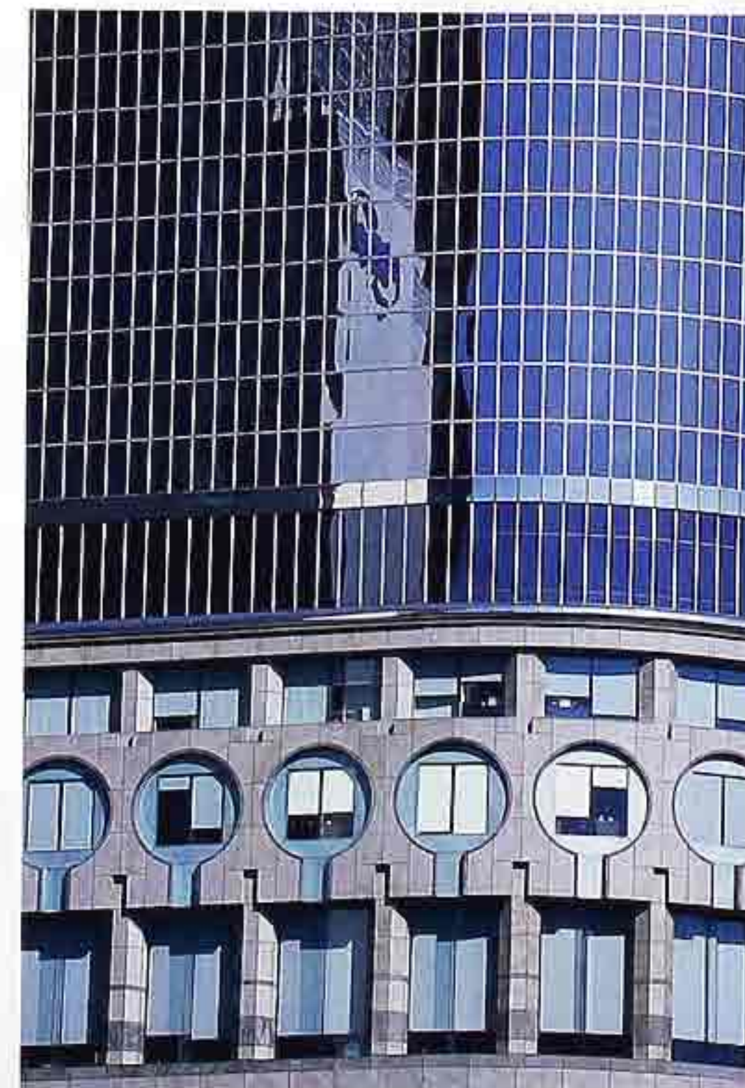
FA-126 Curving glass curtain wall above stone-veneer facade with expressed piers and keyhole window surrounds, modern commercial building
