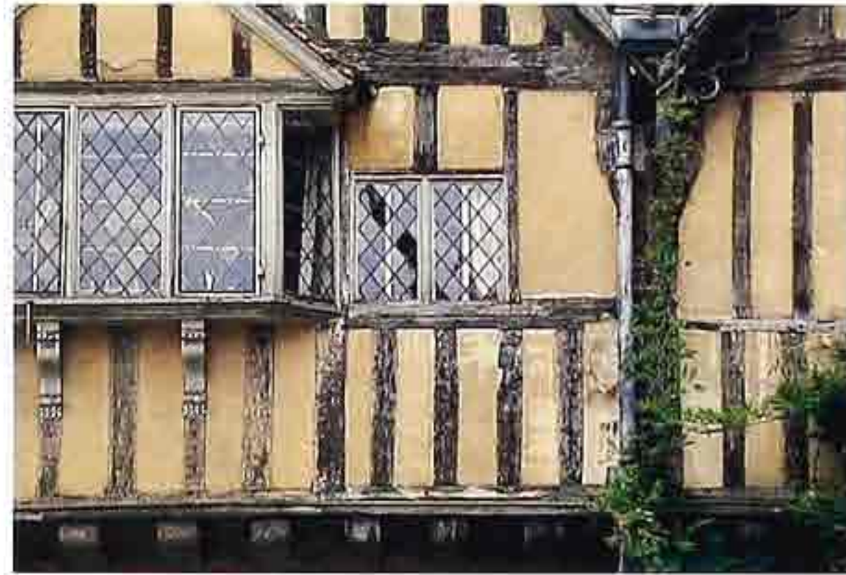
WA-276 Half-timber construction with corbels under jetty; leaded windows, and console supports under oriel, 16th- or 17th-c. English house
