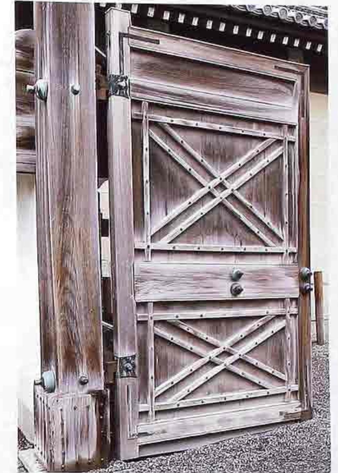
DW-13 Weathered two-panel wood with double cross-braces, brass hardware, and doorknob in center stile, Japanese courtyard gate
