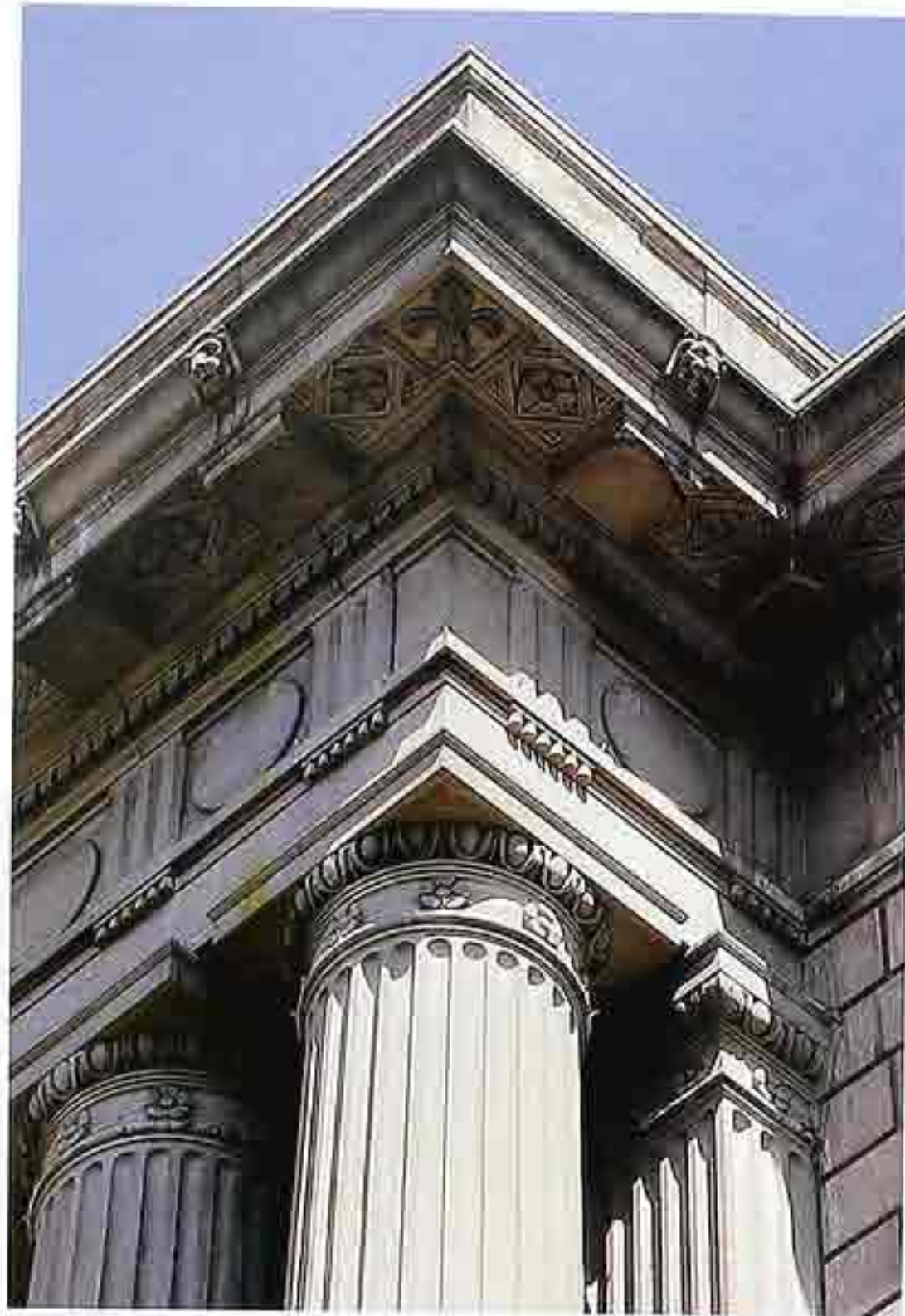
OM-105 Roman Doric-style entablature; discs in metopes; rosettes in coffers alternating with plain mutules in the soffit
