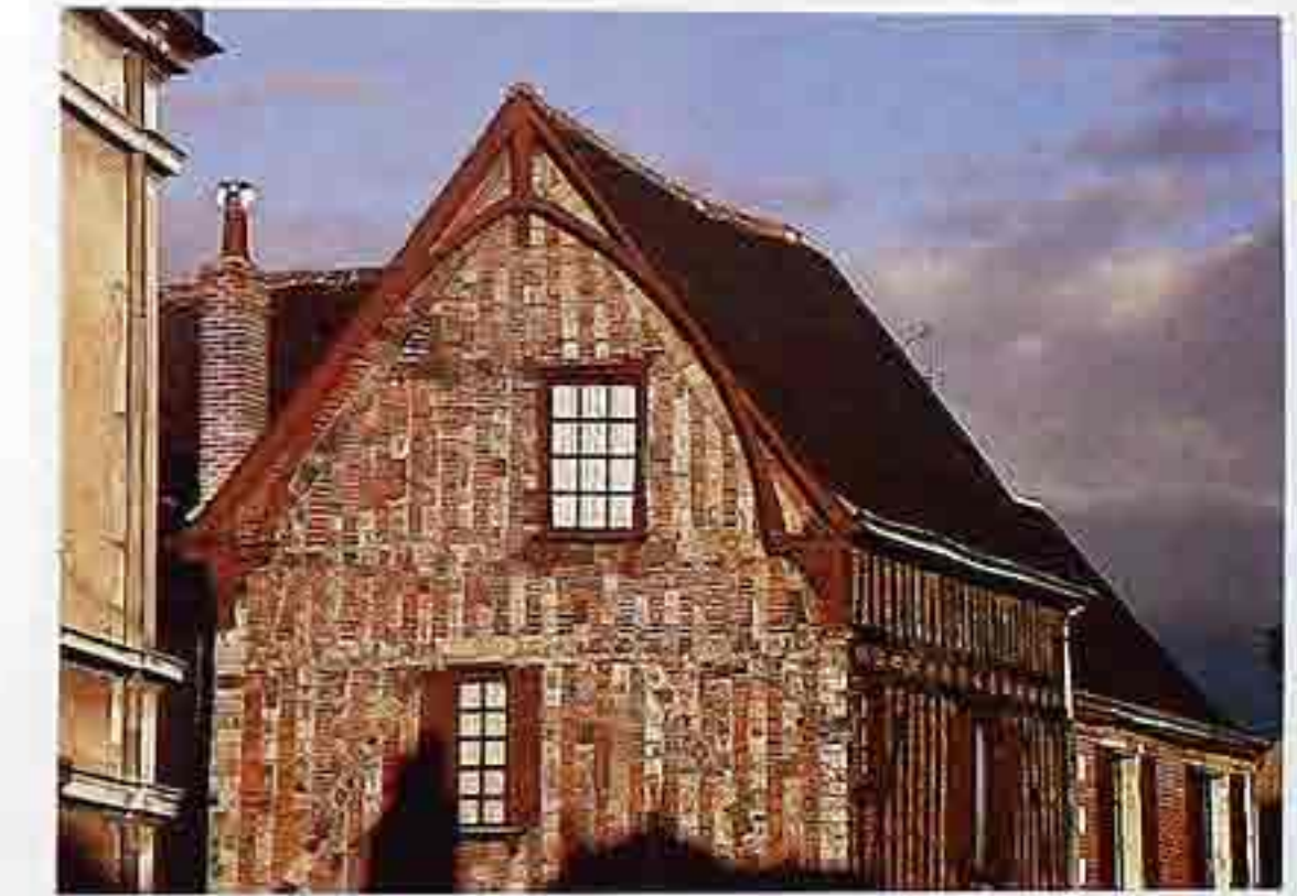
CR-123 Half-timbered gable, with surface arch
