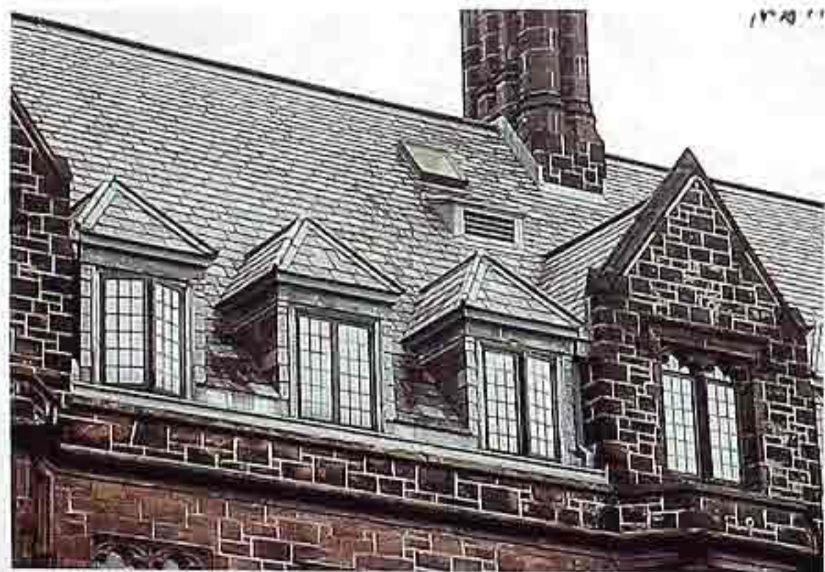
CR-97 Three hipped-roof dormers and a gabled wall dormer; slate cladding on roof dormers and roofs
