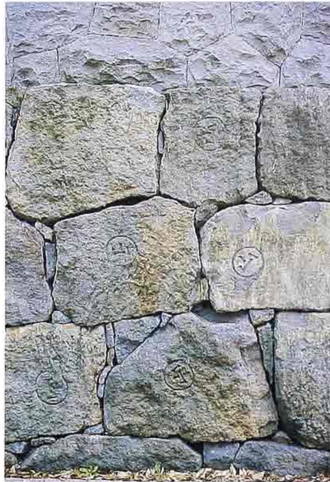
WA-73 Coursed rubble with gallets and rock-face cap
