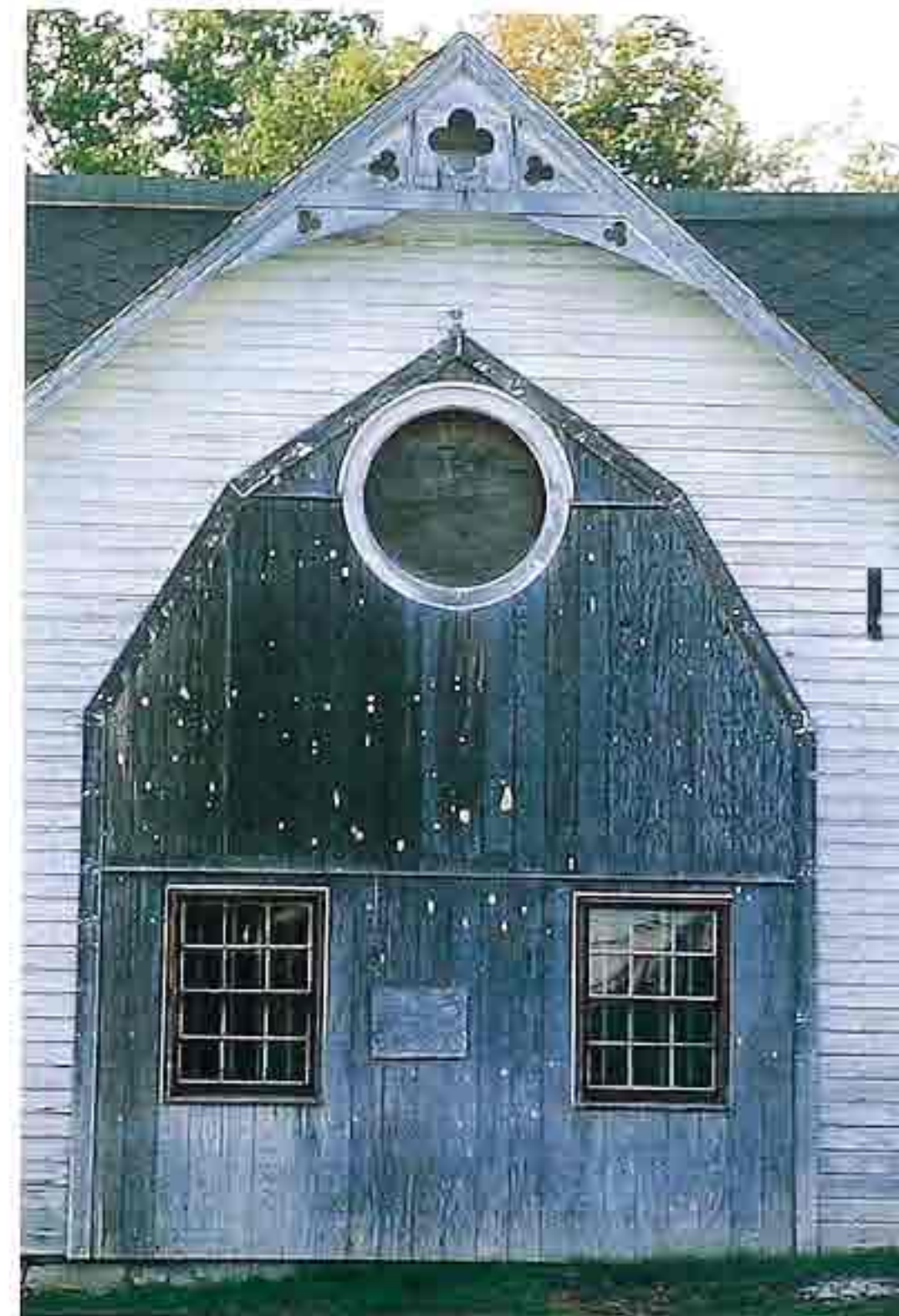
WA-22 Painted clapboard gable-end wall with gable ornament and exposed vertical board cladding
