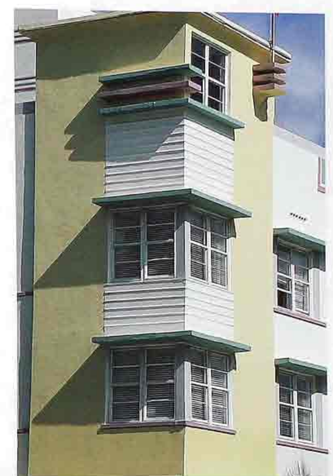
WI-91 Corner windows: single-hung sashes with fixed upper lights, Art Deco apartment house
