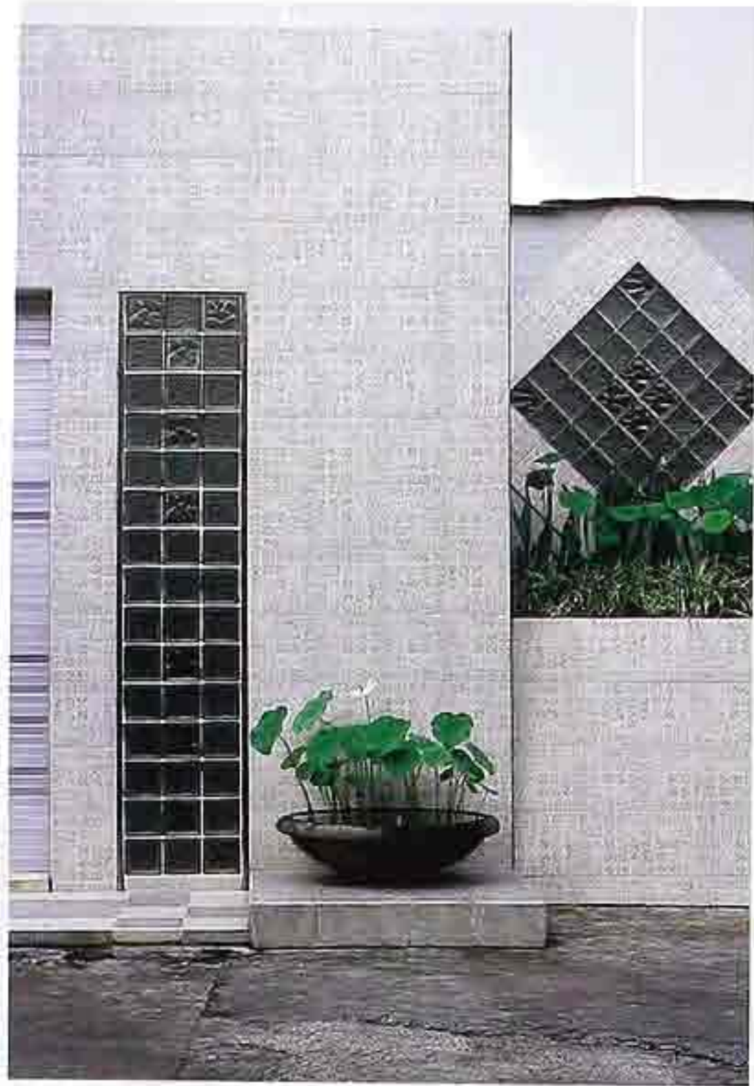
FA-68 Textured matte tiles with glass-block windows, entry of modern house
