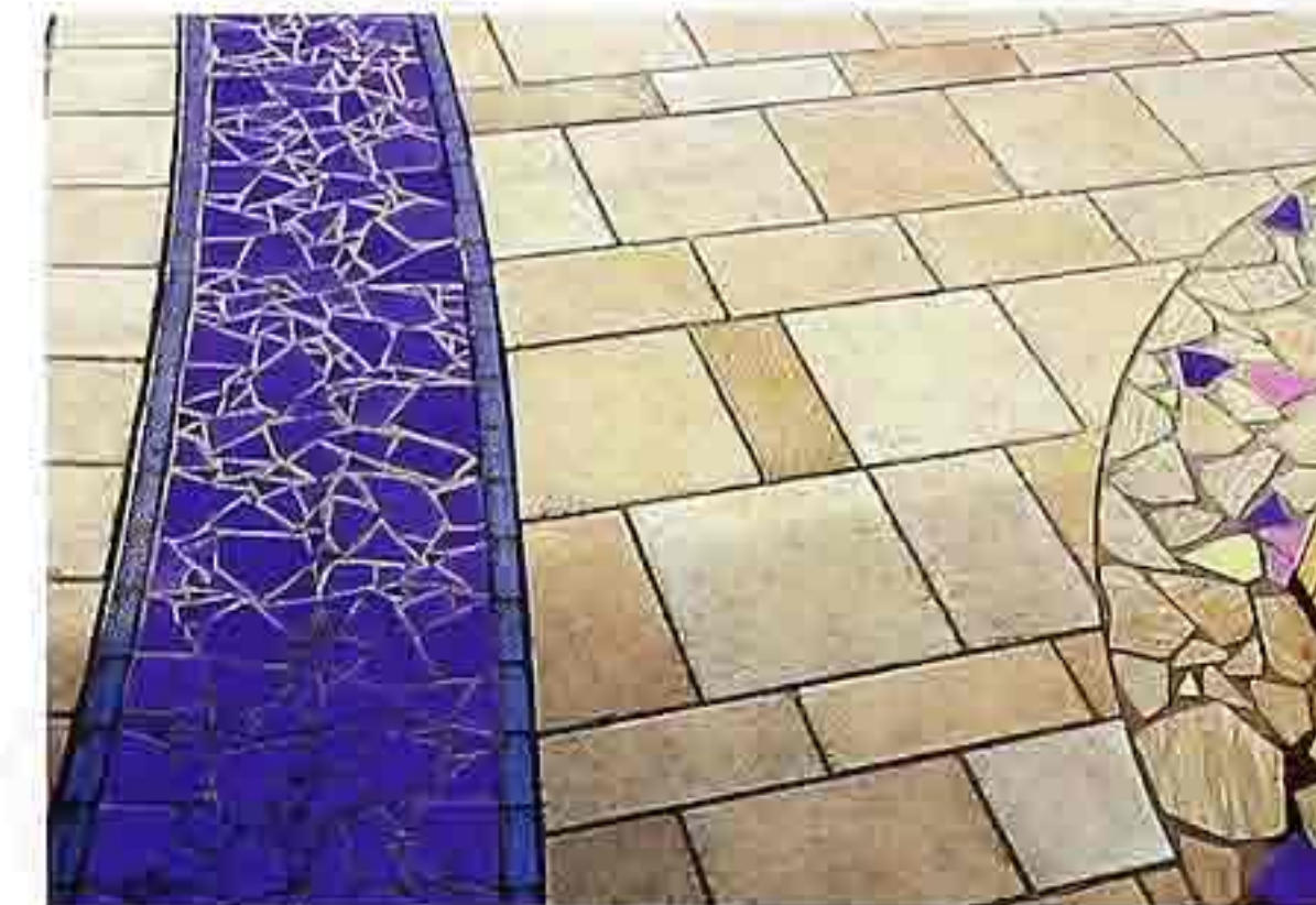
FP-87 Random-shaped ceramic and stone tiles in mosaic pattern surrounded by random-ashlar pavers, urban public space
