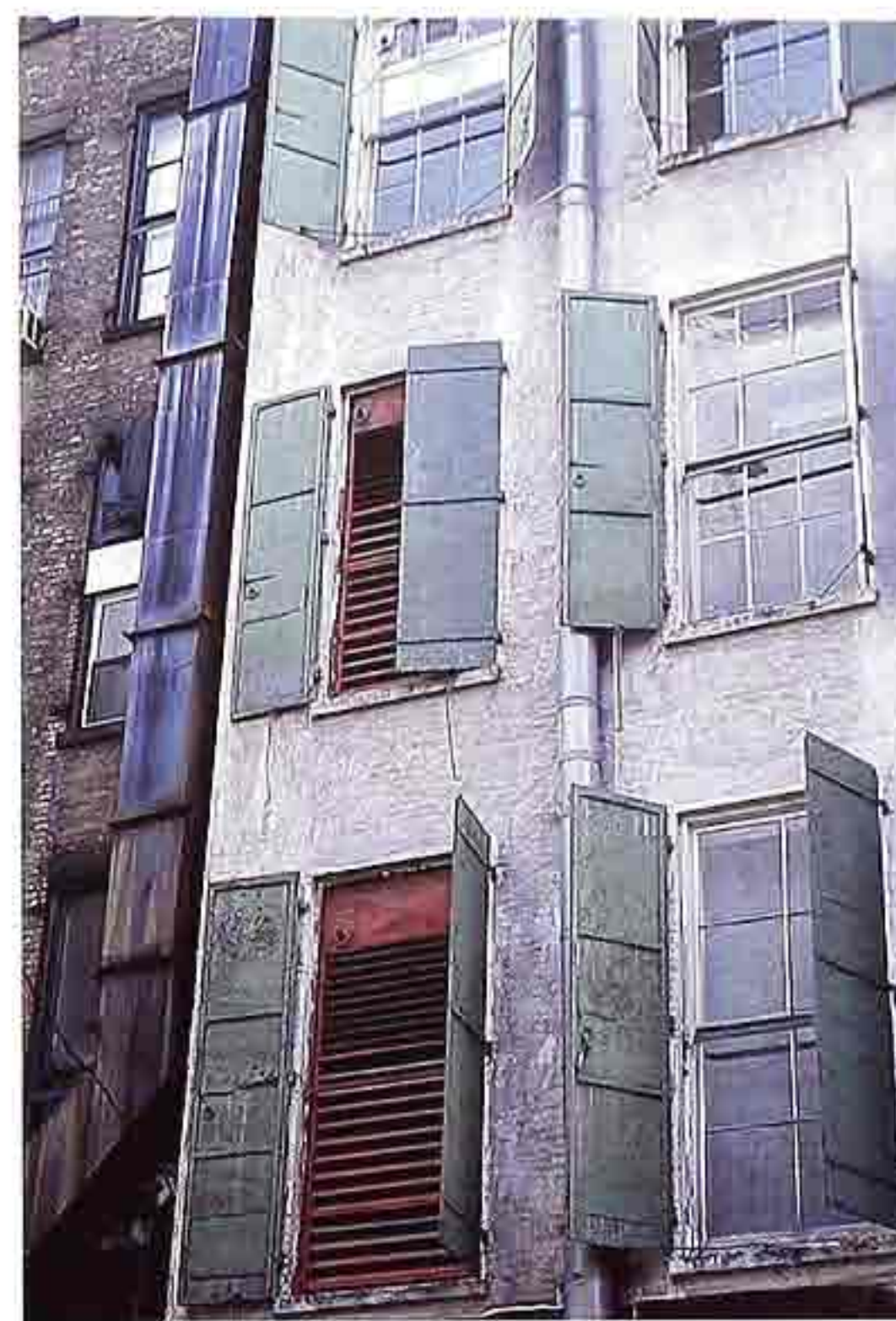
WI-179 Metal shutters, 19th-c. industrial building
