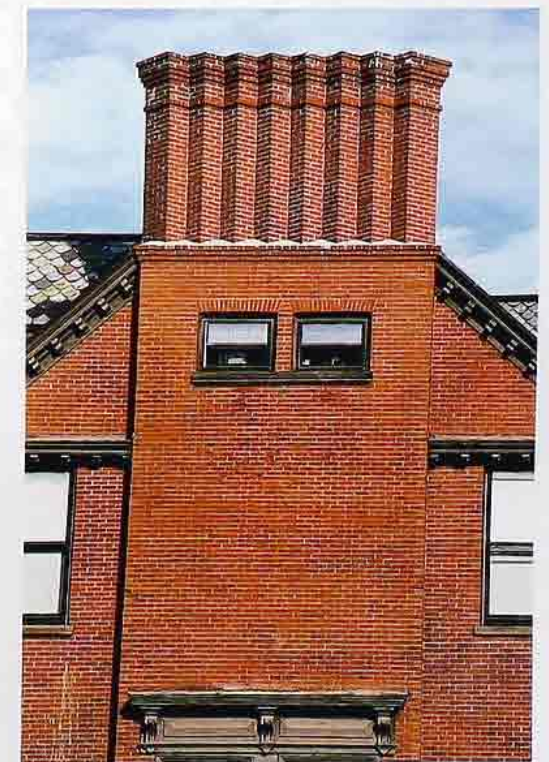
CR-146 Engaged rectangular chimney stack
