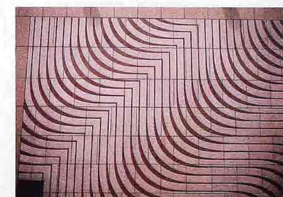
WA-69 Pink granite in running bond with polished and flamed finishes forming supergraphic, modern commercial building
