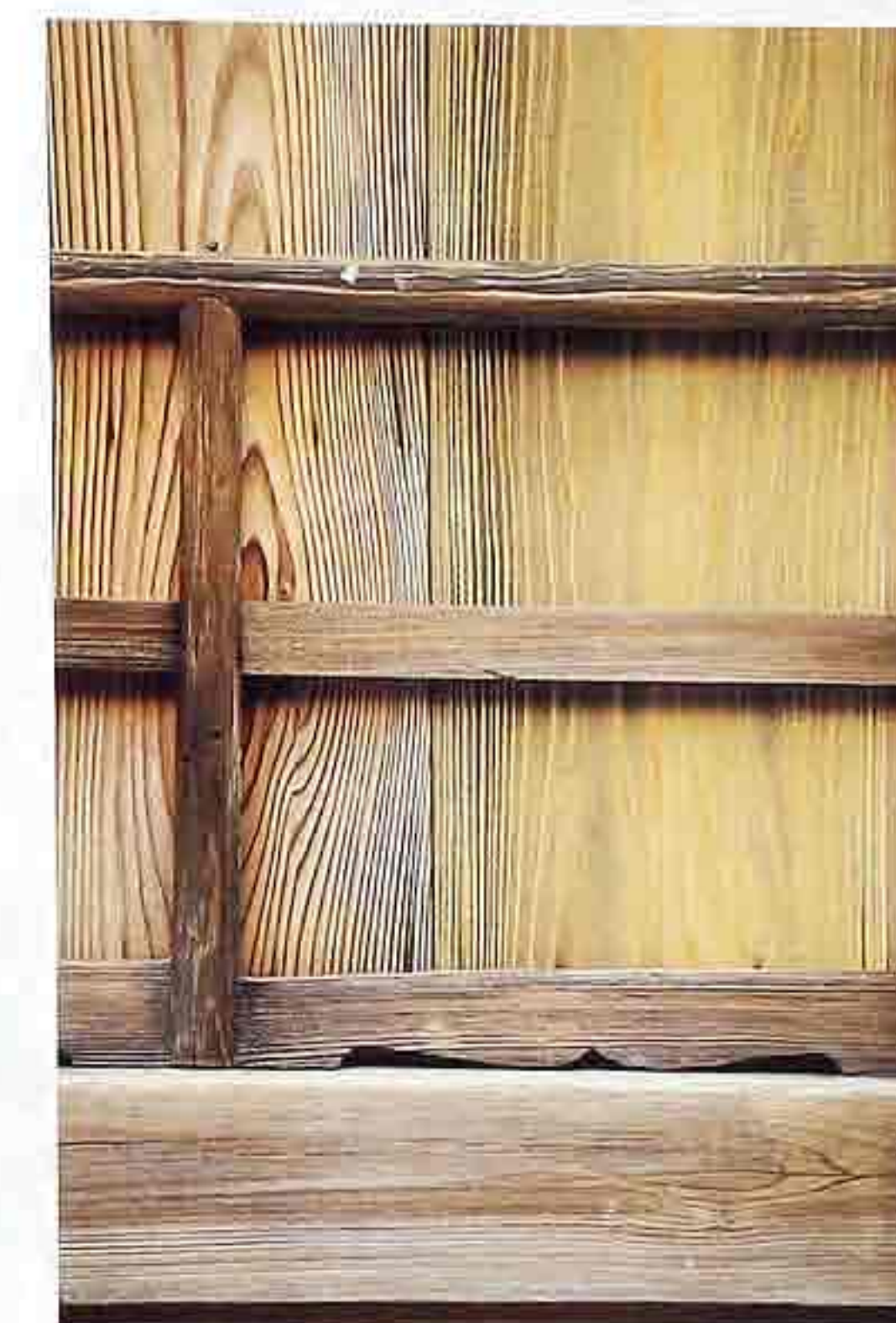
WA-6 Plain-sawn vertical planks with decorative battens
