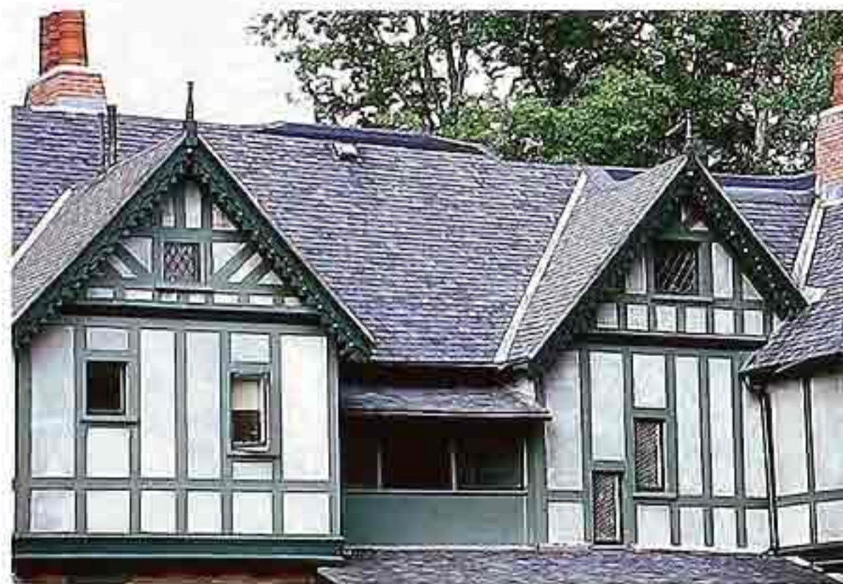
CR-95 Half-timber wall gables with scalloped bargeboard flanking shed roof and flashing in roof valleys
