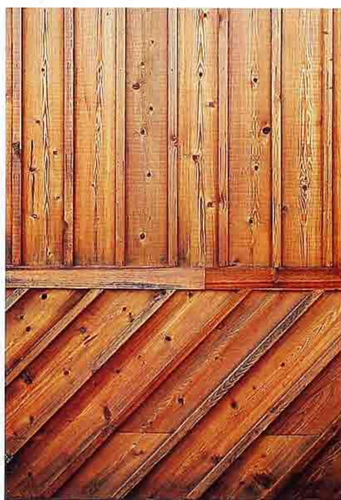
WA-4 Stained and sealed board-and-batten siding
