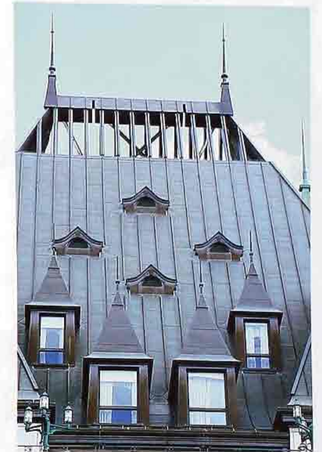
CR-100 Four flared-gable roof dormers above flared pyramidal roof dormers on metal hipped roof
