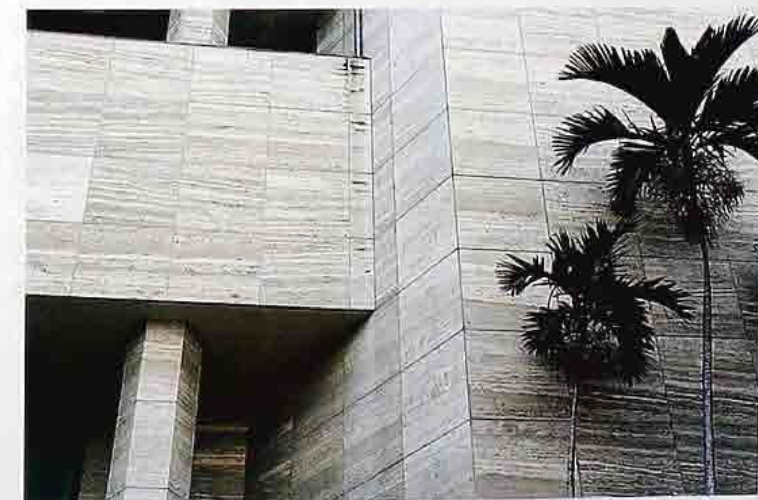
WA-130 Inside and outside corners of end-matched travertine veneer on walls and post, modern commercial building
