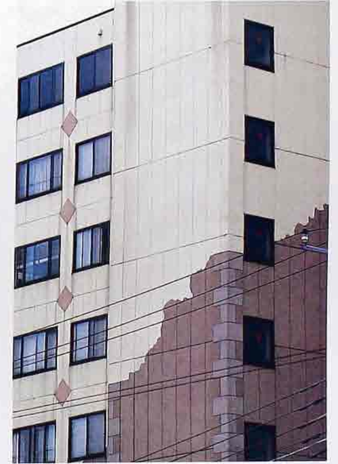
WA-247 Colored smooth stucco supergraphic with stucco quoins in lower section, modern apartment house
