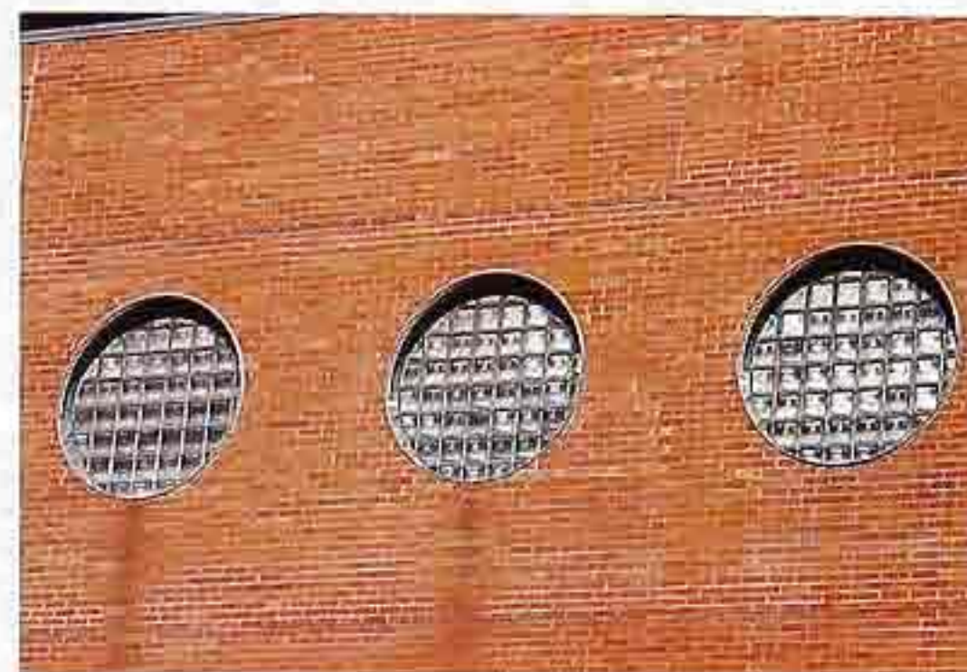
WI-24 Circular windows with glass block, modern commercial building
