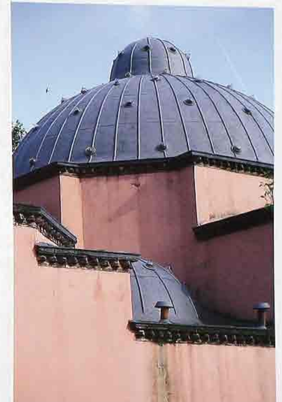
CR-131 Composite dome, metal with standing-seam
