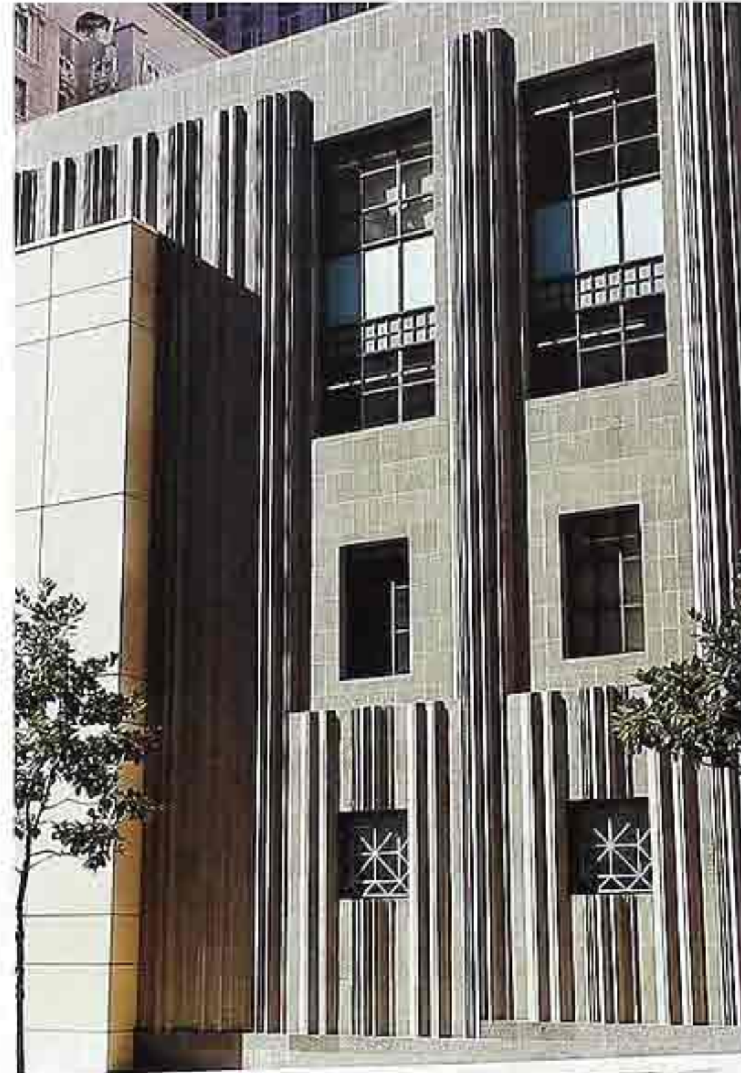
CP-97 Fluted and reeded pilasters on Art Deco facade
