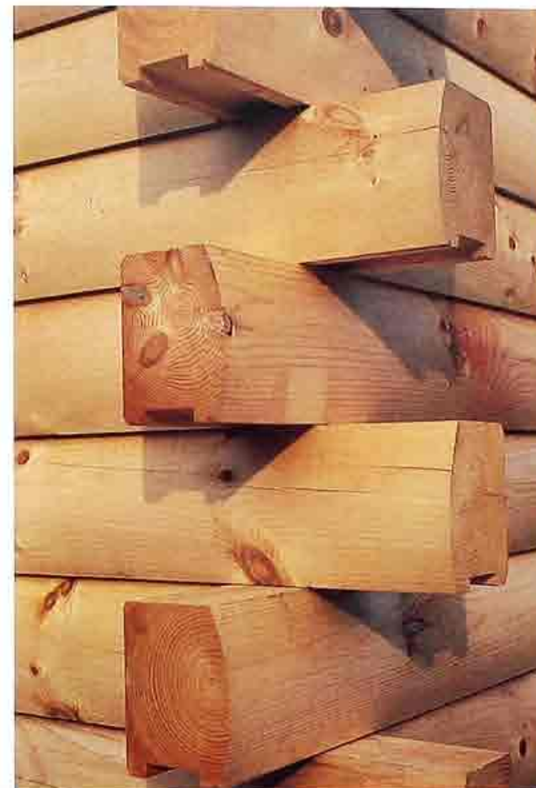
WA-5 Pine log house construction, corner detail
