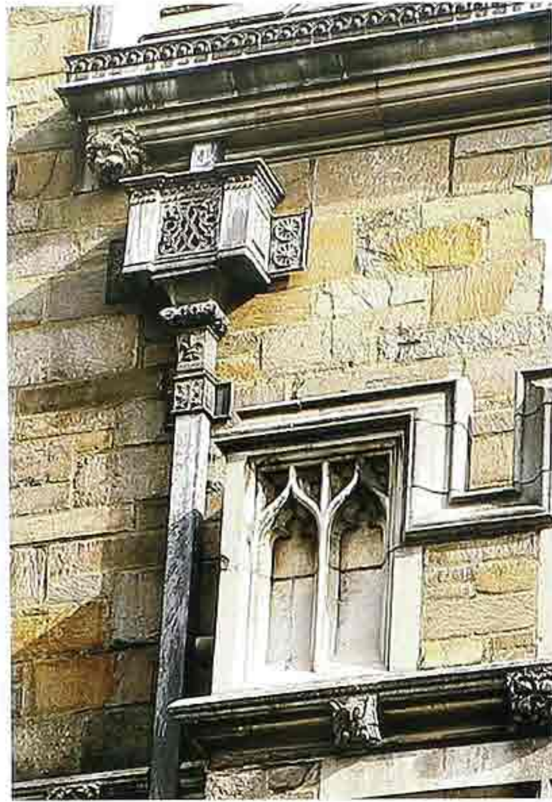
CR-156 Metal decorated gutter, rainwater head, and drainpipe
