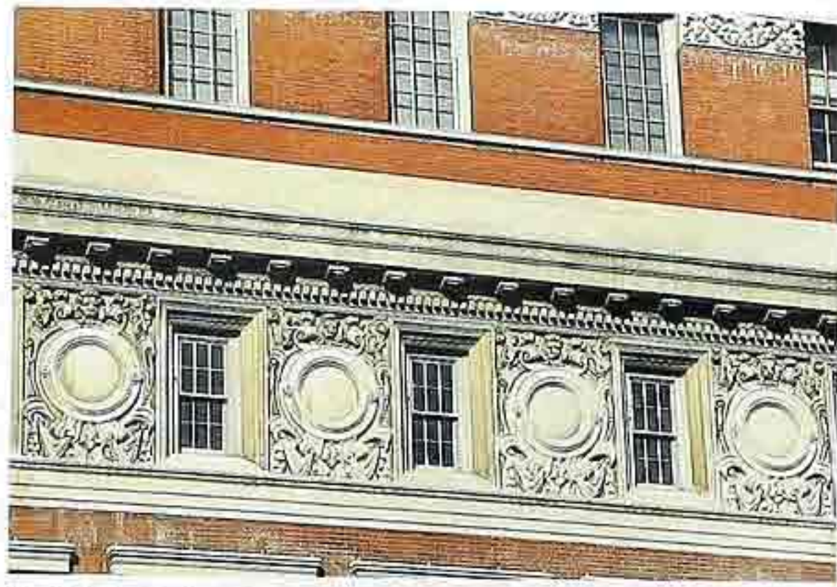
FA-119 Brick facade with decorative masonry frieze of sculpted spandrels between windows
