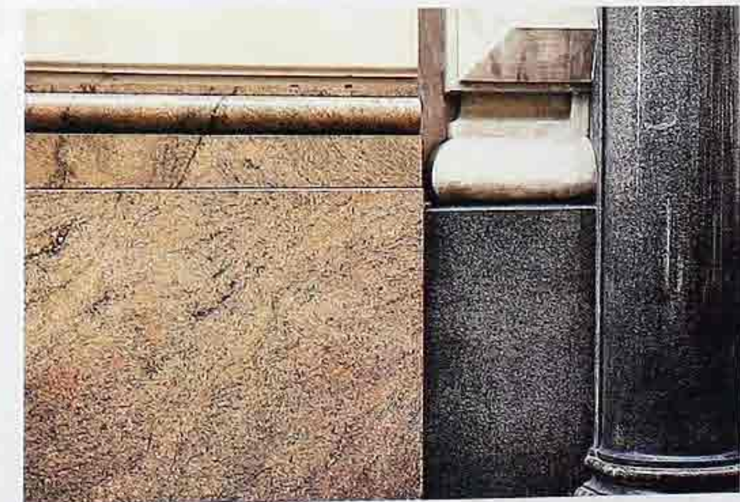
WA-88 Polished granite and marble. Left to right: granite-veneer base with bead molding; granite plinth with marble ovolo molding on base; polished granite engaged column
