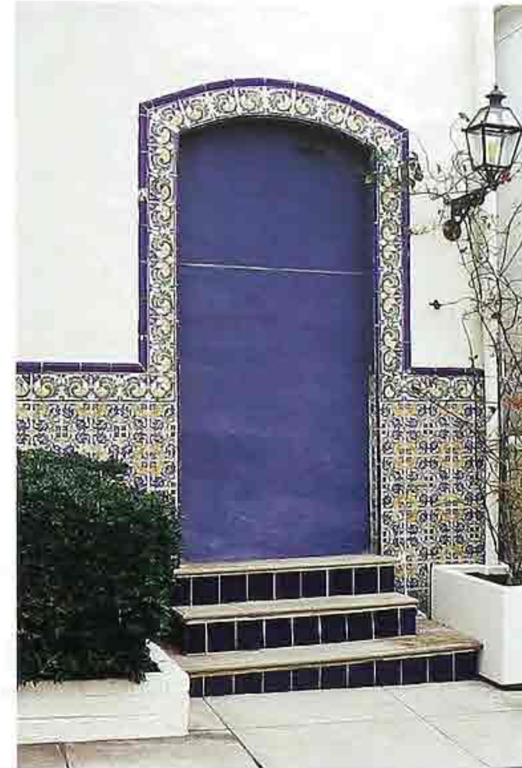
DW-90 Spanish-colonial-style recessed door in segmental arch framed with decorated glazed tiles on stucco wall; Mexican tile steps
