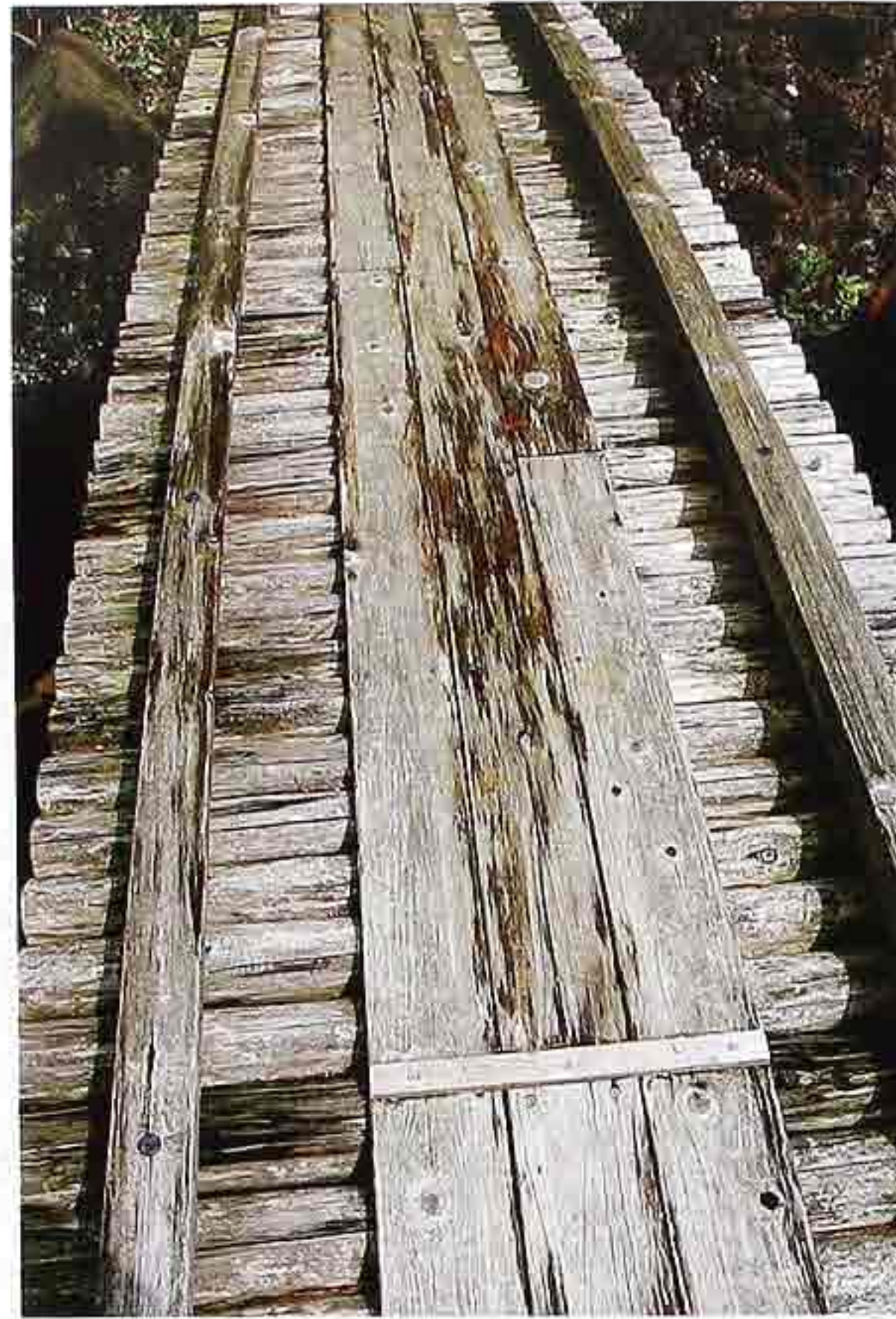
FP-2 Dressed logs with center-sawn planks and wood-peg construction, rustic garden bridge
