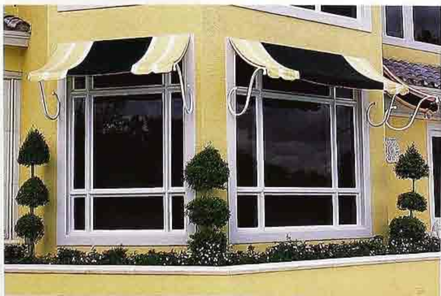
WI-75 Fixed windows and sidelights; awnings with brackets, patio wall of modern house
