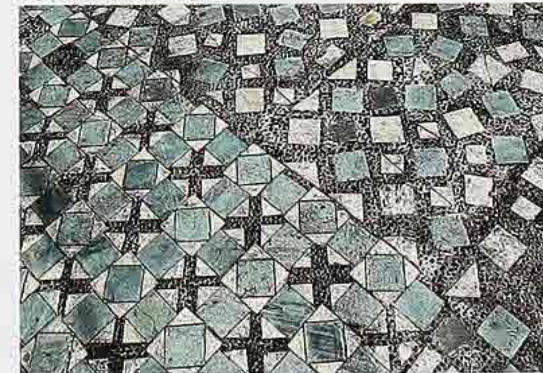
FP-101 Square and triangular ceramic tiles set in exposed-aggregate field in geometric and random patterns, entryway
