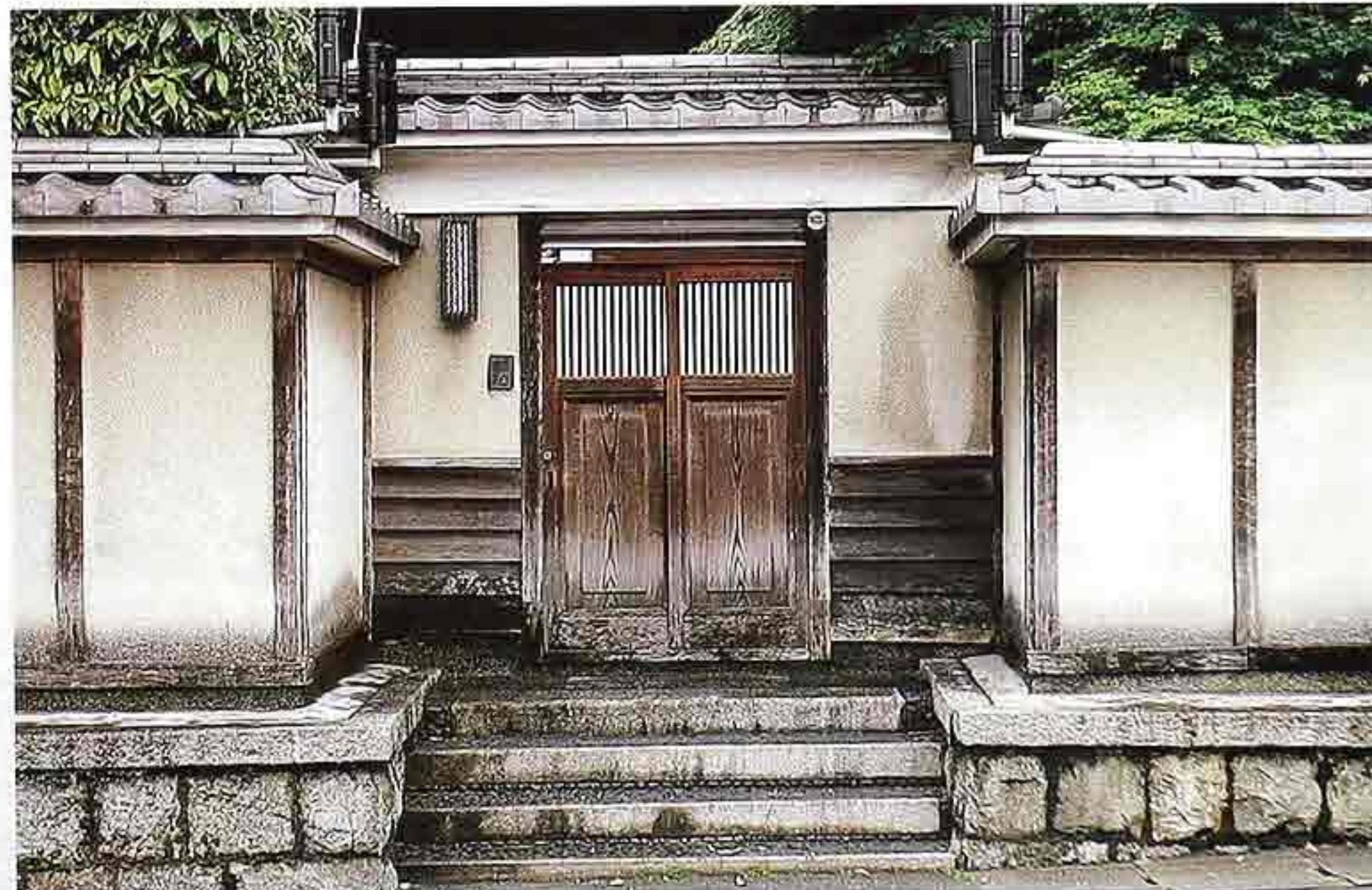
DW-96 Traditional Japanese entry: double wood doors and stone steps
