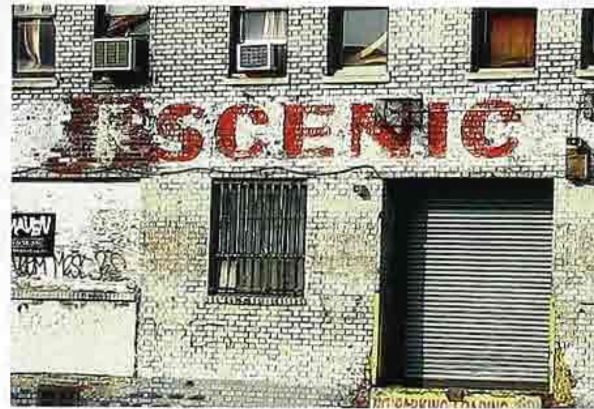
FA-105 Painted sign on brick facade with loading door
