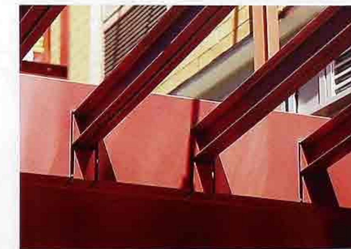
CP-119 Steel beams built up of two C-channels of weathering steel
