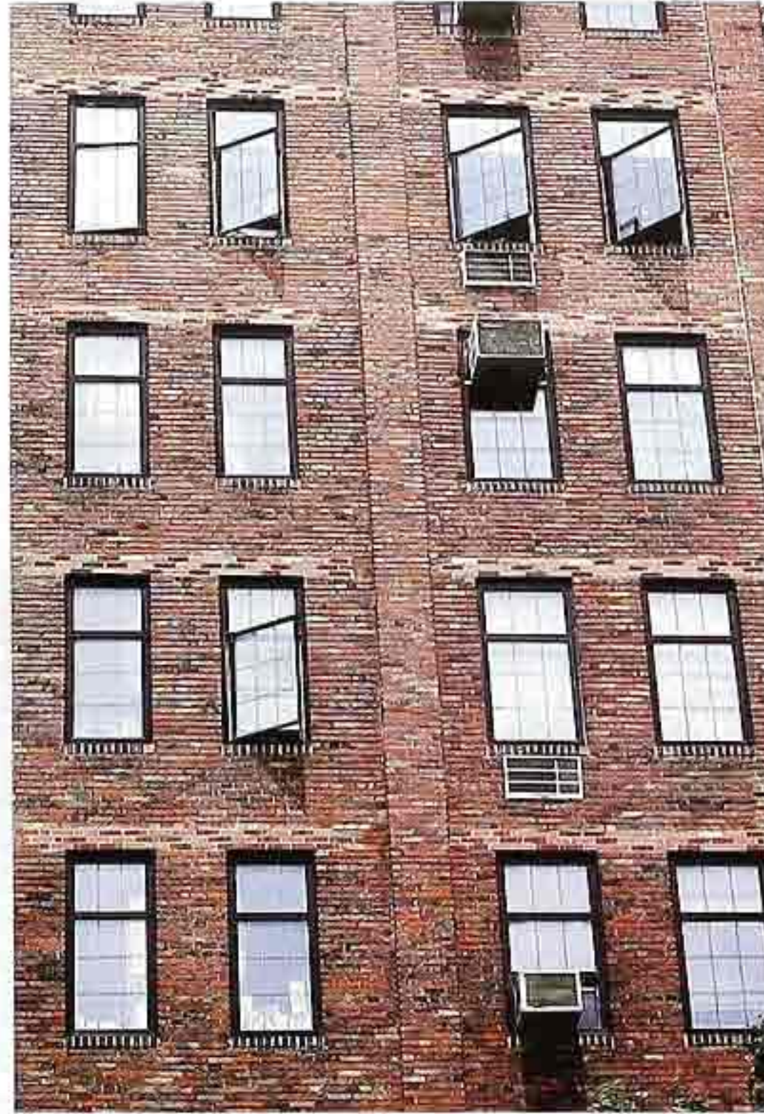
WI-31 Casement windows with internal muntins and fixed light above, modern metal replacement windows in older apartment house
