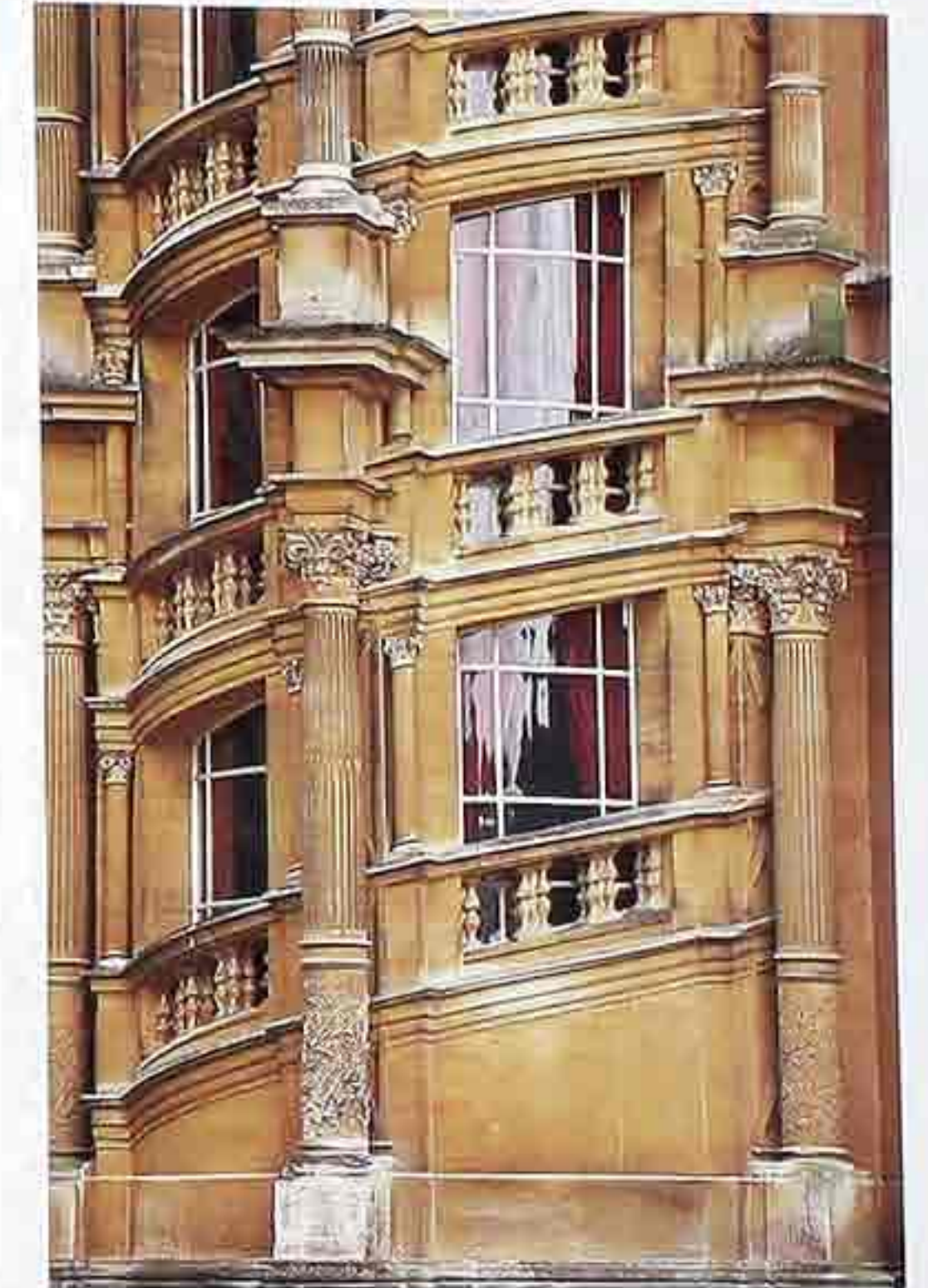
FA-109 Stair tower with engaged columns and spiral balustrade
