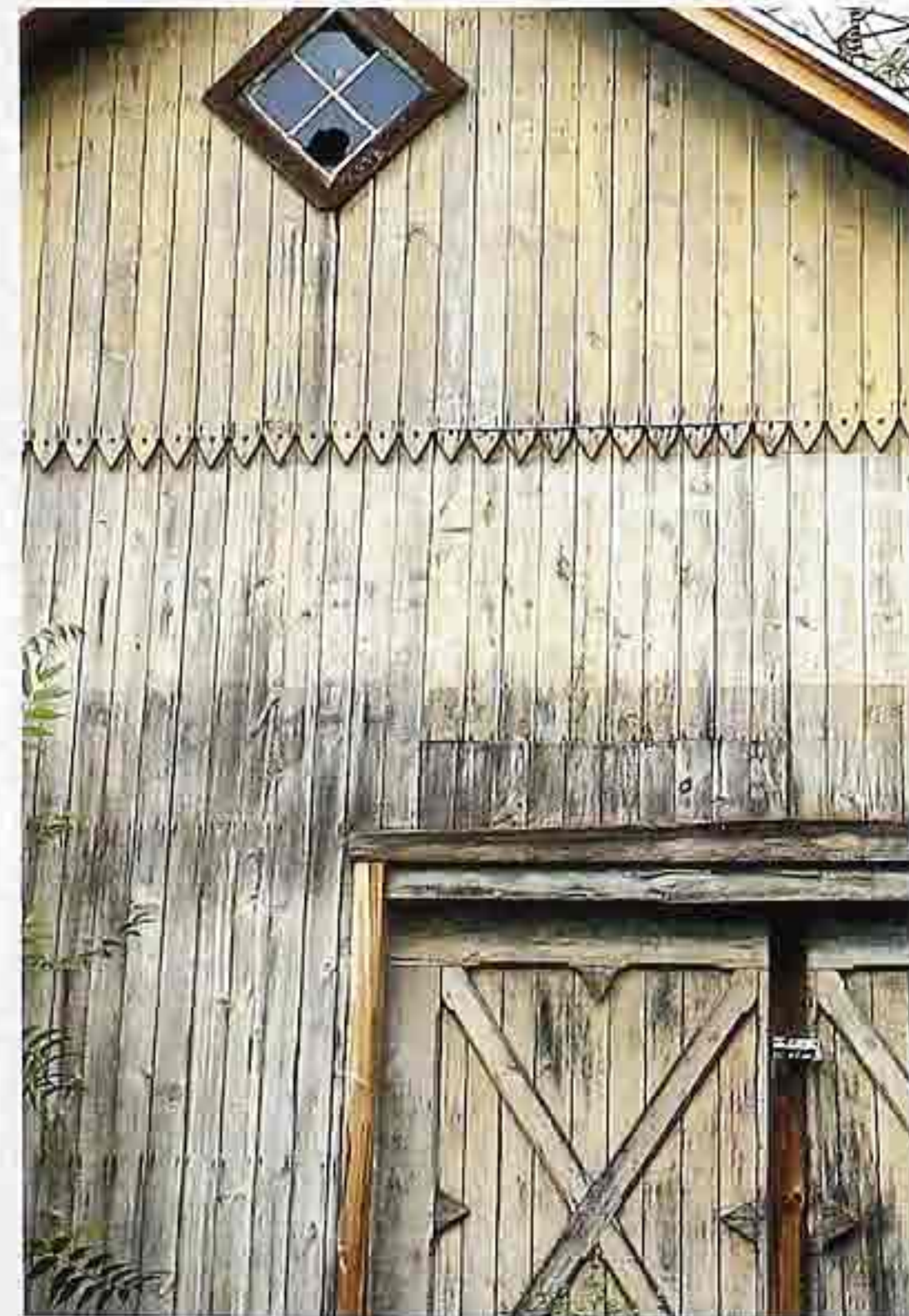
WA-30 Weathered painted flush vertical board cladding on barn gable end with diamond-shaped window and vertical scallop-edged siding
