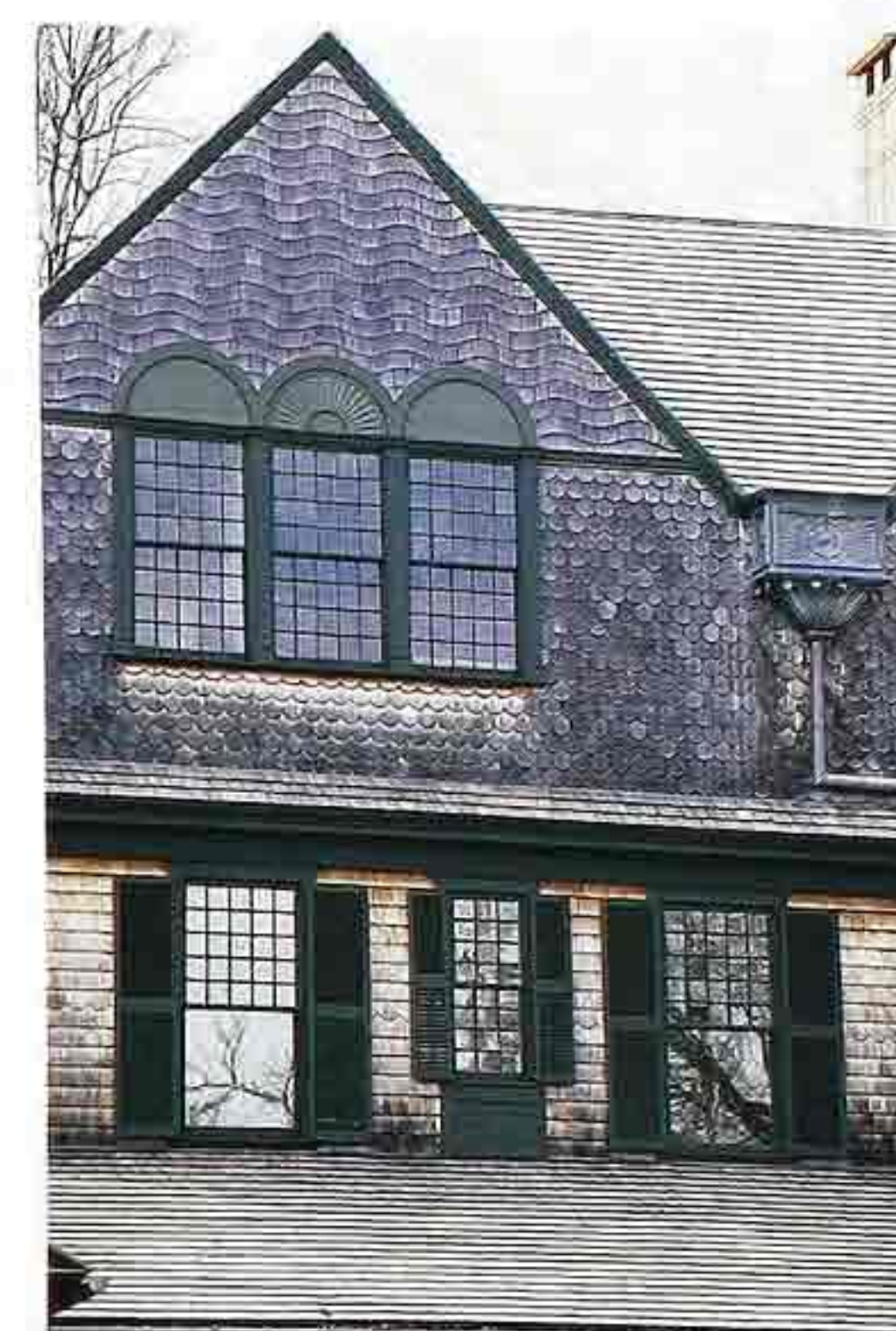
WI-52 Double-hung windows: twenty-over-twenty with plaster mullions (top); twenty-over-ones flanking twelve-over-twelve, 20th-c. shingle house
