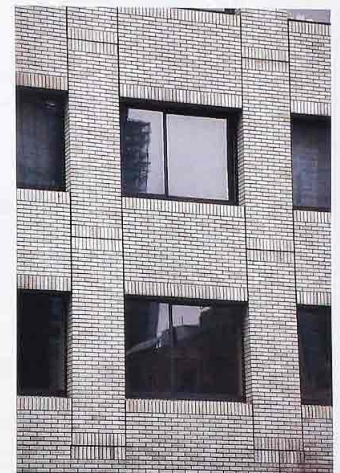
WA-180 Brick panels in running bond articulated by joints and soldier courses; soldier courses top and bottom of windows, modern commercial building
