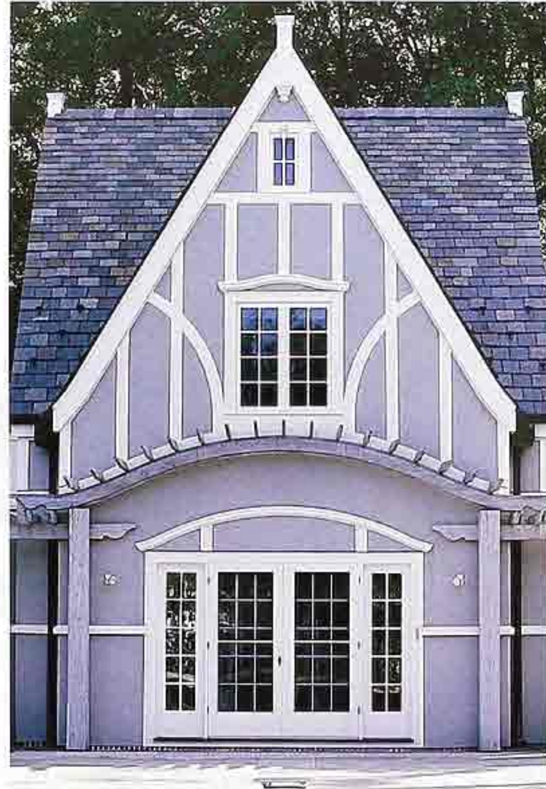
CR-127 Half-timber-style cross gable with variegated slate roofing
