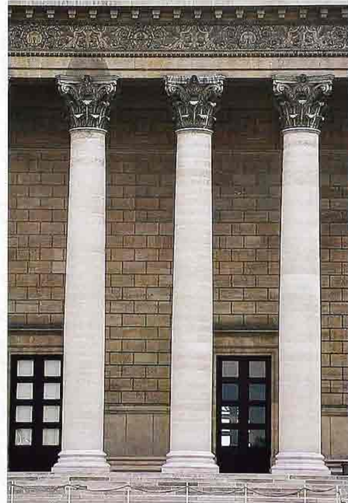
CP-74 Corinthian columns supporting portico
