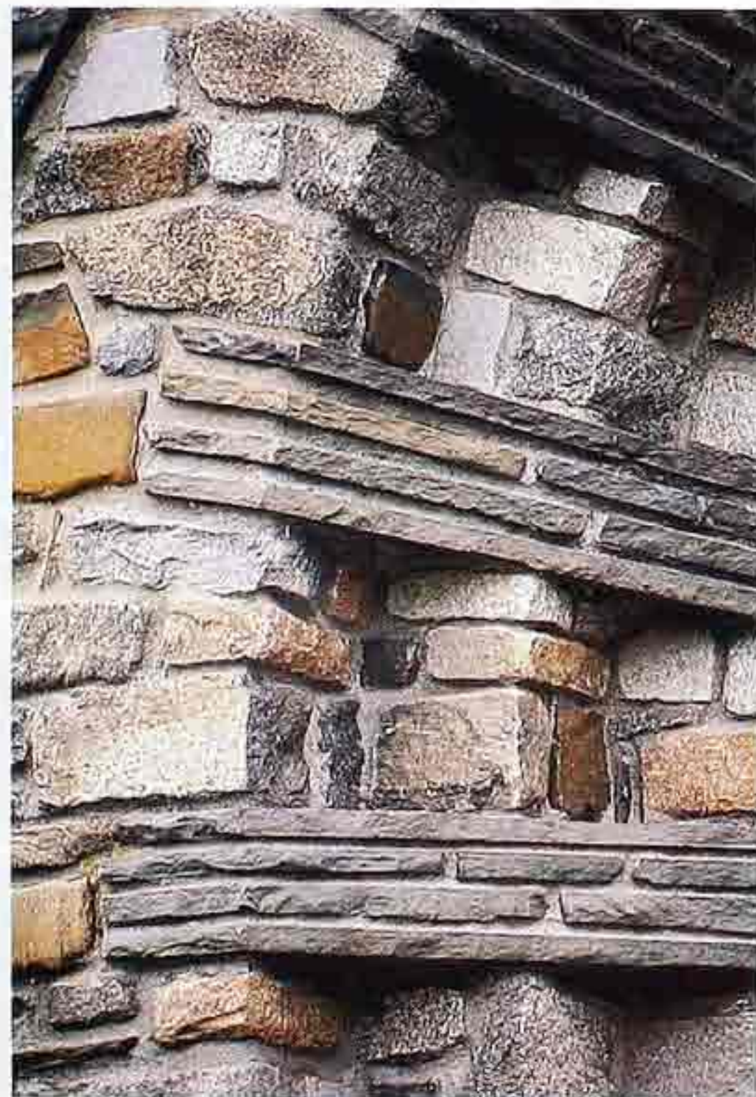
WA-91 Roughly squared stone in random ashlar wall with flagstone voussoirs in compound arch
