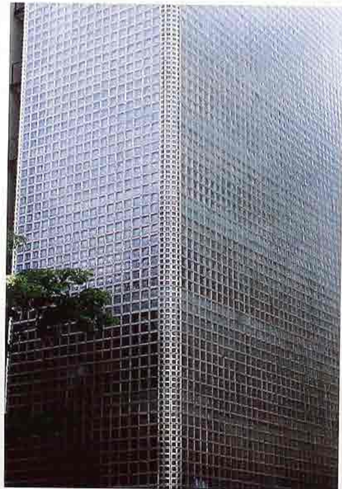
FA-35 Glass-block curtain wall with rounded corner
