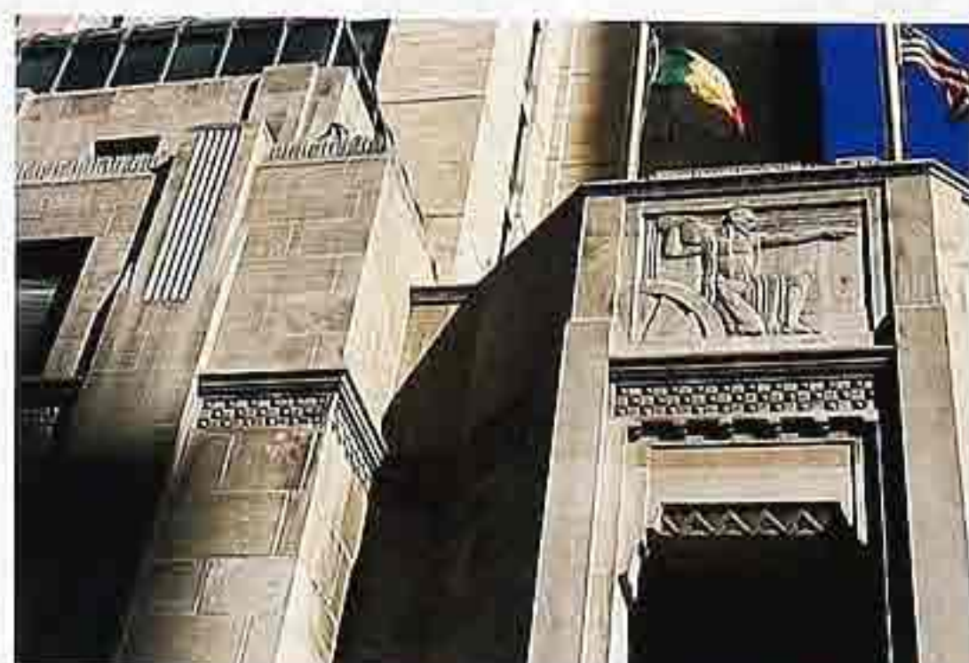
WA-119 Sand-finish limestone veneer with Art Deco bas-relief cartouche and molding
