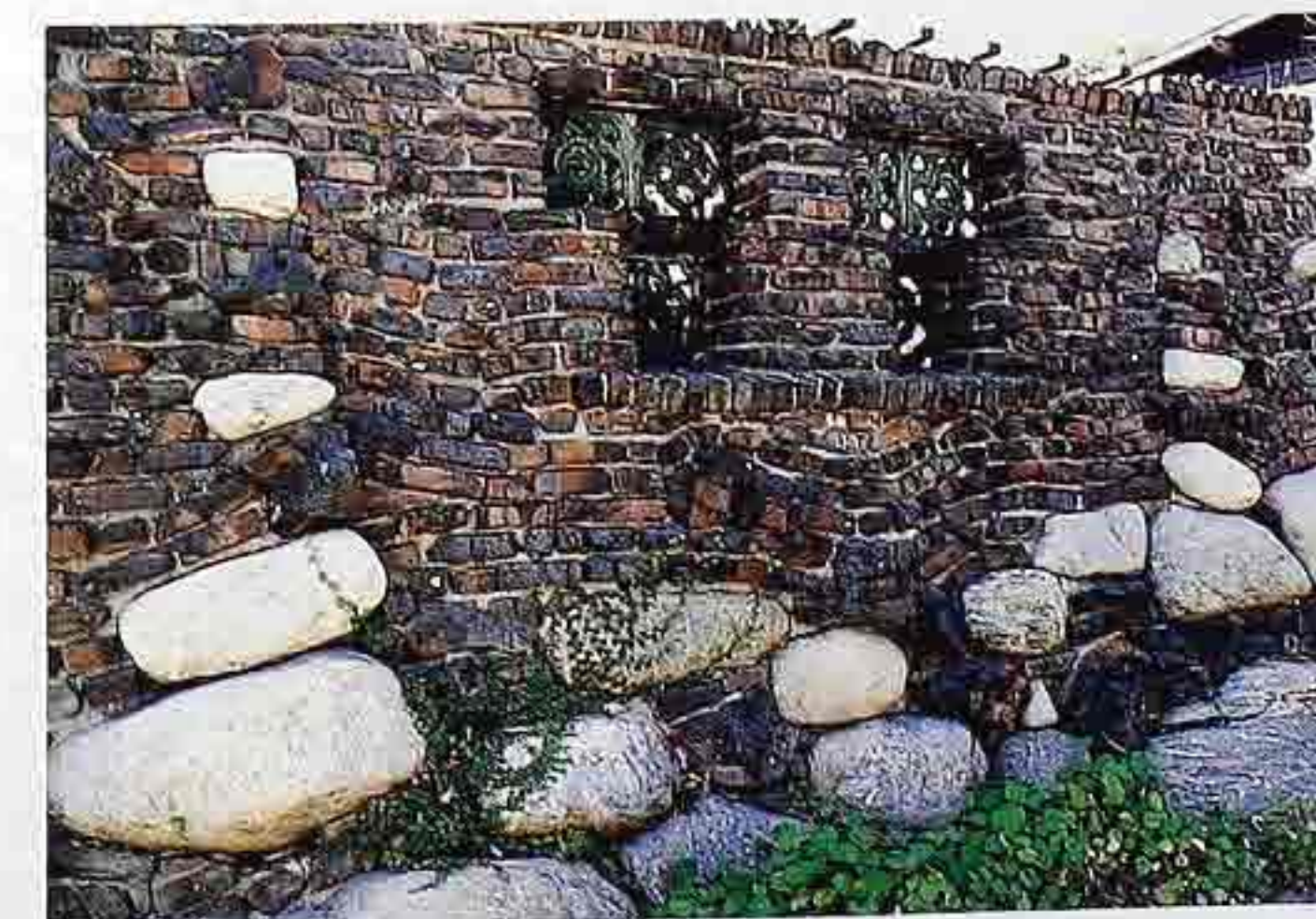
WA-272 Boulders and large cobbles randomly interspersed with custom-bond brick, openings filled with grillework or screen blocks, battered garden wall
