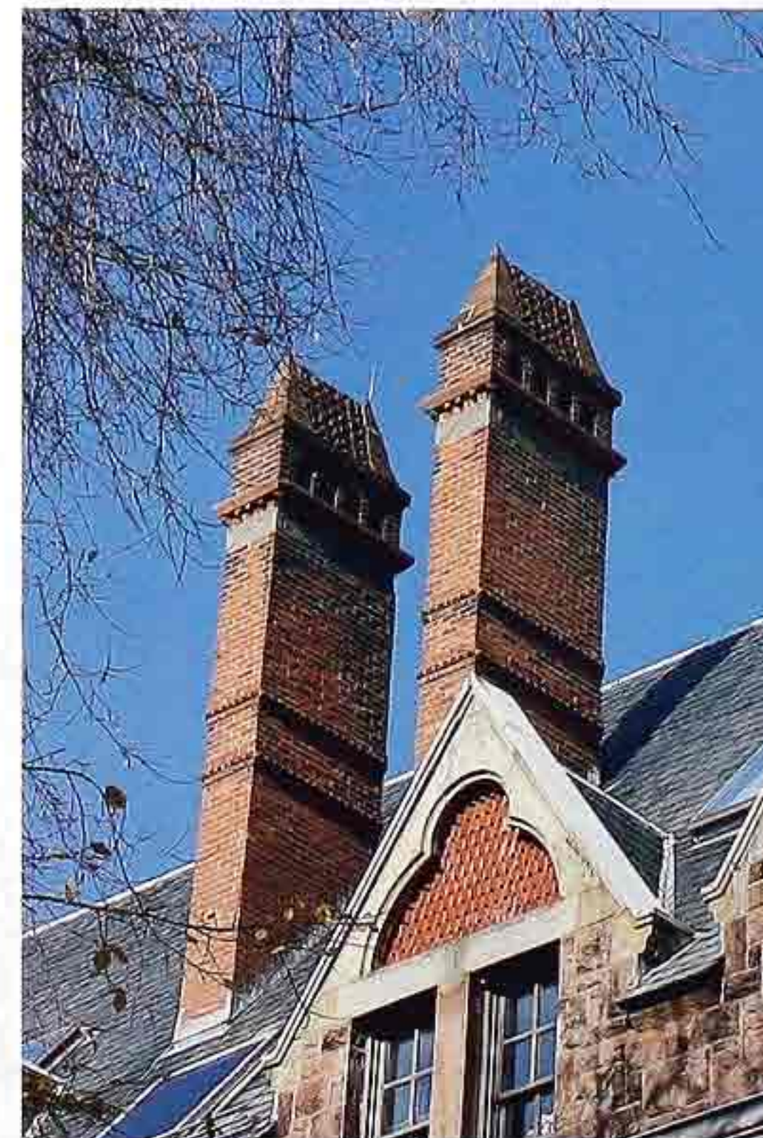
CR-145 Brick chimneys with hipped chimney hoods
