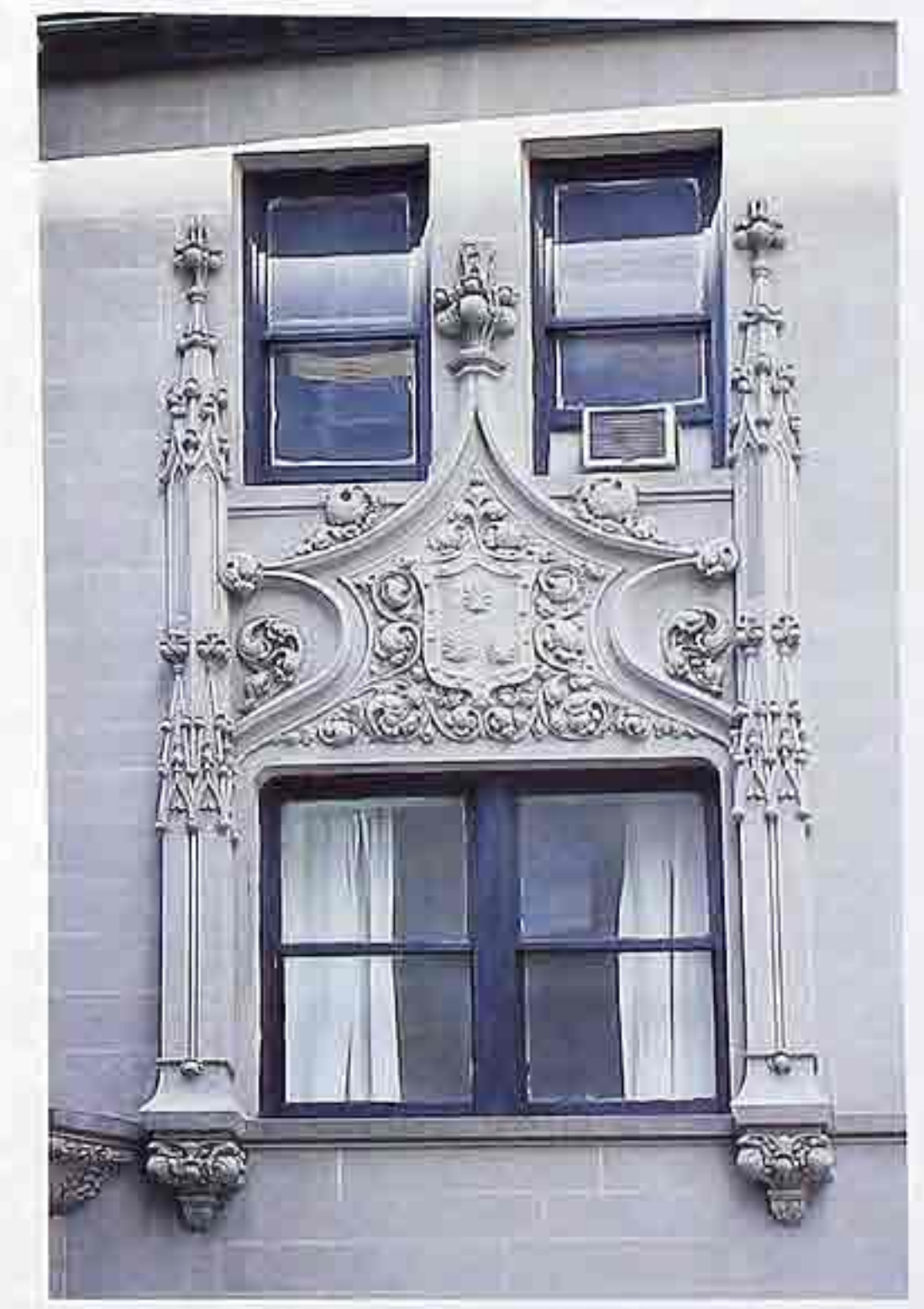
WI-137 Fanciful neo-Gothic spandrel with cartouche flanked by corbelled pilasters, apartment building
