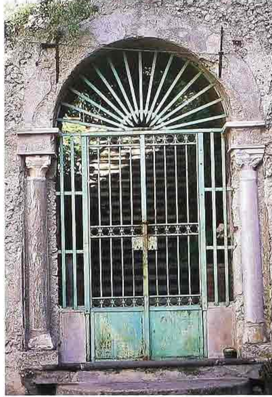
DW-115 Metal double gate with open bars and fan-shaped top panel in rustic stone arch with impostes on engaged columns
