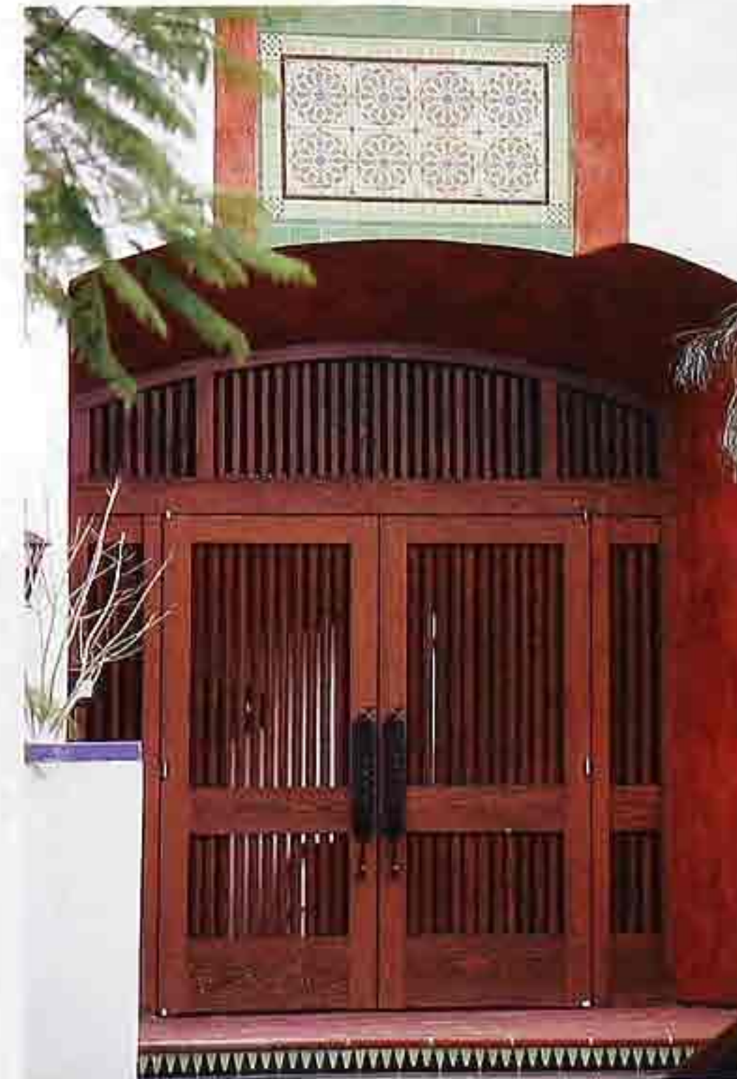
DW-92 Spanish-colonial-style hotel entry with recessed wood gate under cambered arch
