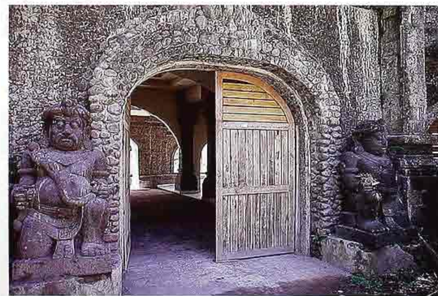
CP-158 Shallow surbated arch in rubble masonry with wood door
