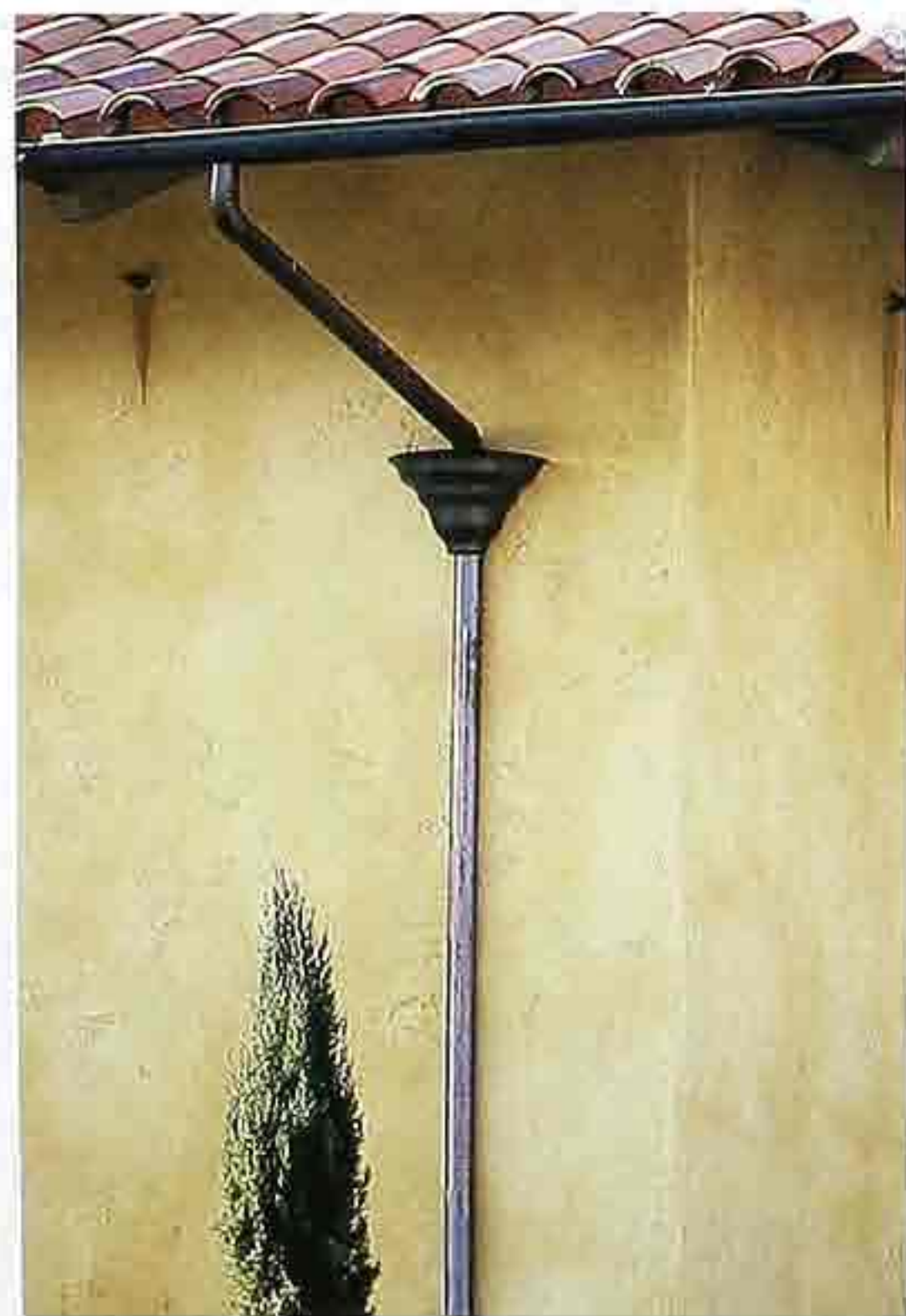
CR-157 Metal gutter, drainpipe, and rainwater head
