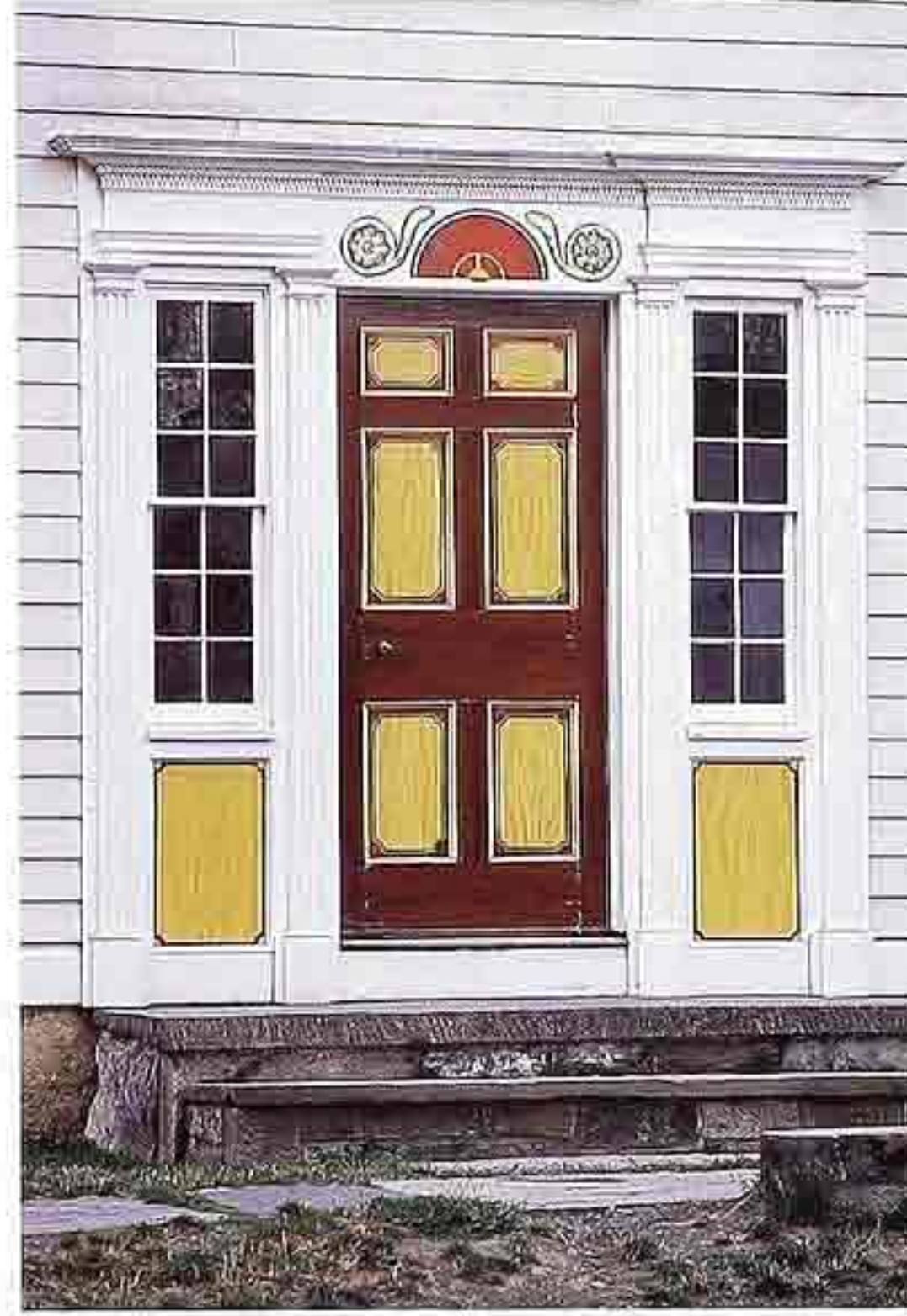
DW-38 Six-panel American Colonial-style door with flush molding, painted ornament on transom, and double-hung side lights
