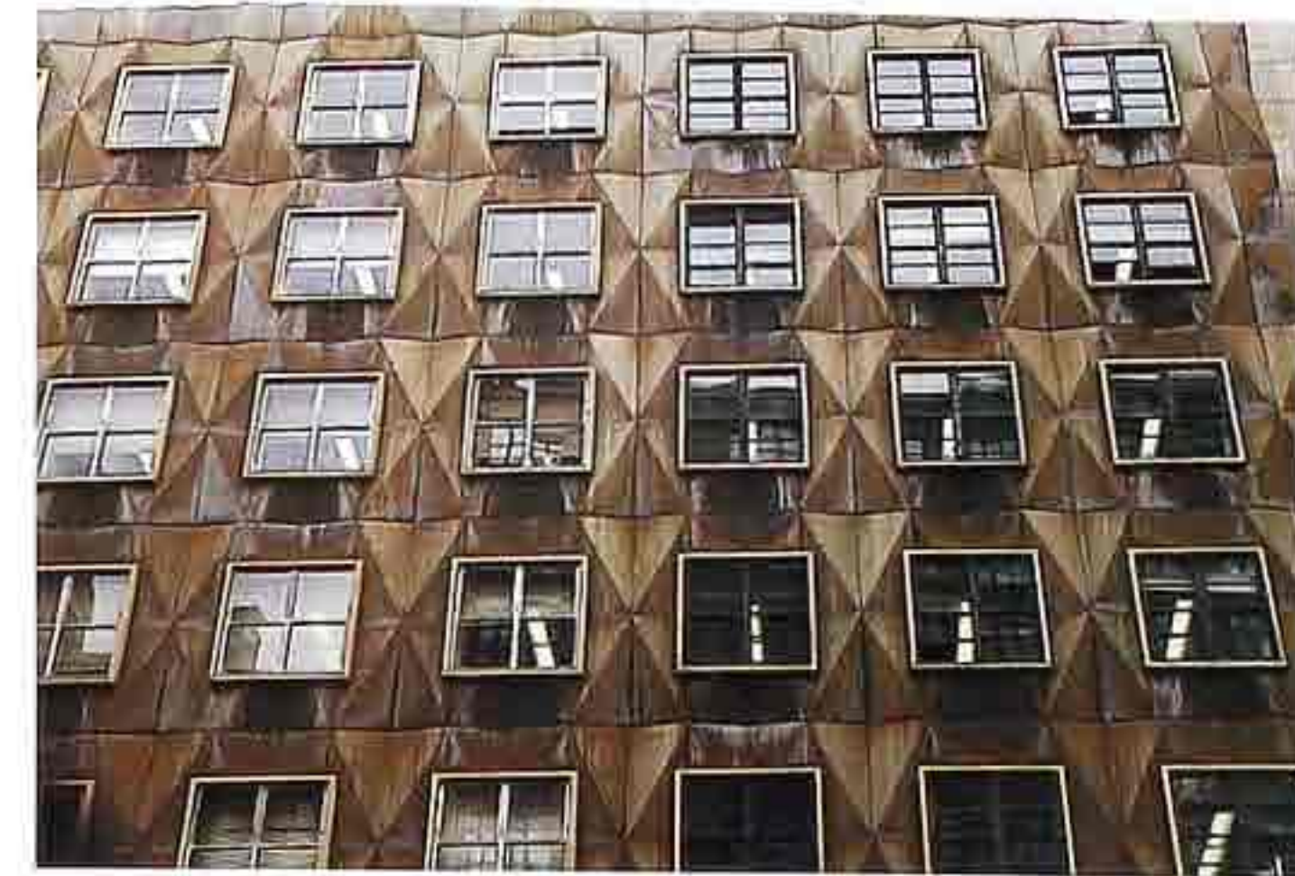
FA-23 Weathered panelized wall system with stamped diamond pattern, modern apartment house
