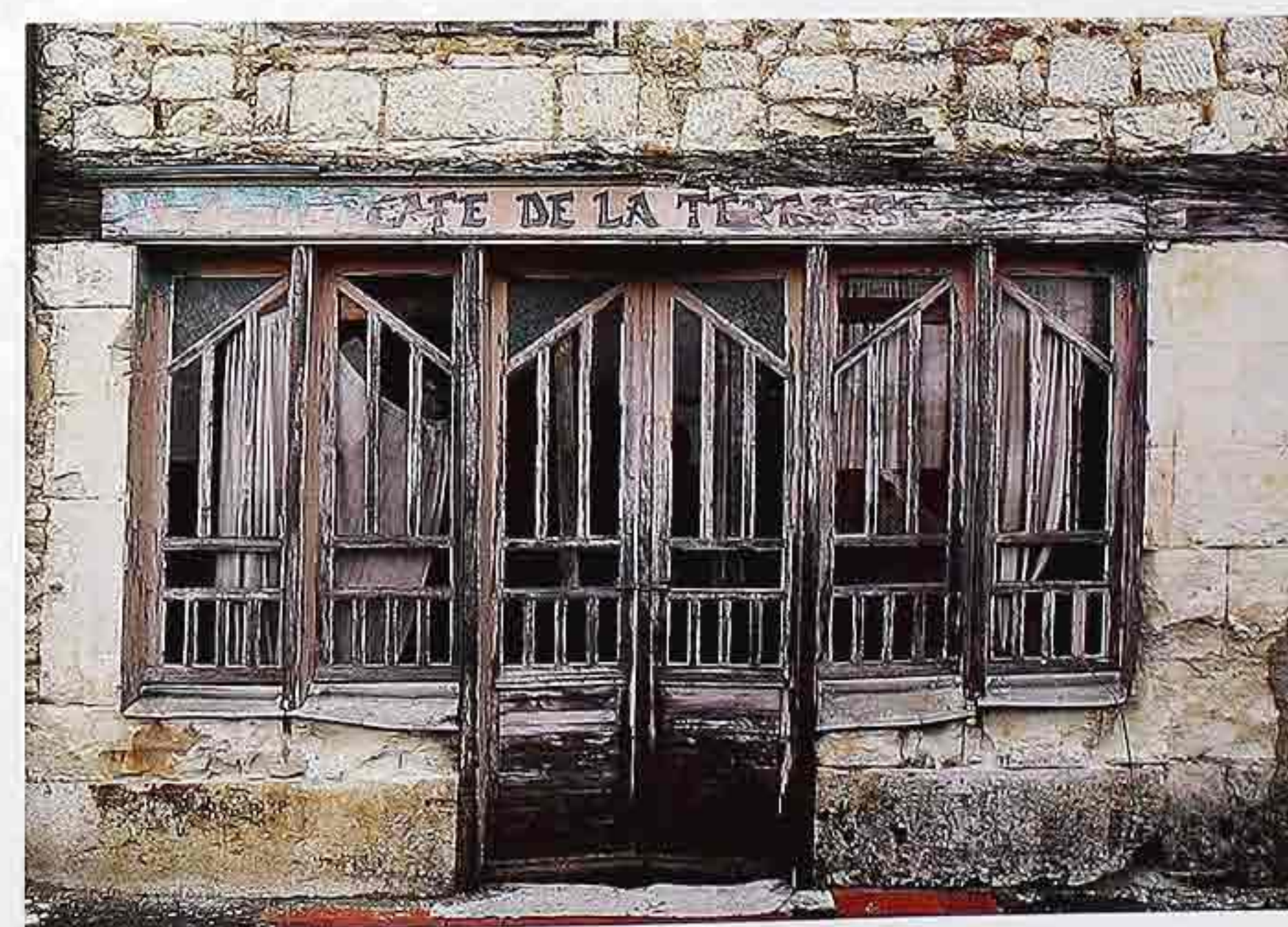
DW-106 Café entry in ruins: wood-paneled double doors with lights flanked by wood-framed windows
