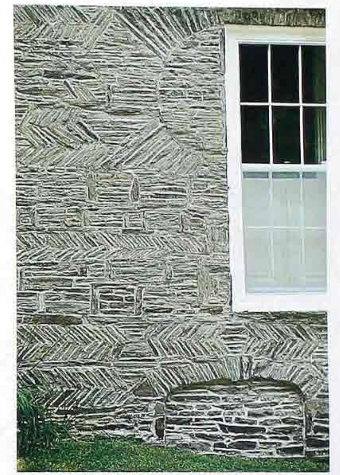
WA-111 Shale fieldstone in coursed roughly squared rubble and herringbone pattern
