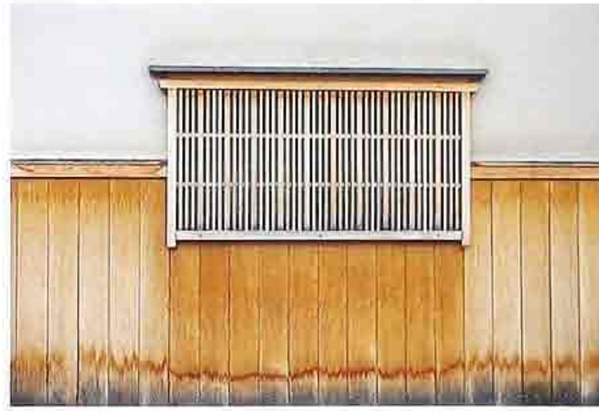
WA-274 Stucco and wood-planked infill; timber-frame construction; traditional Japanese wood lattice window
