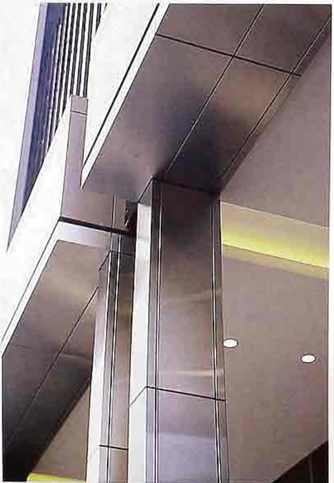
CP-124 Steel frame clad with possibly stainless steel panels, modern commercial building
