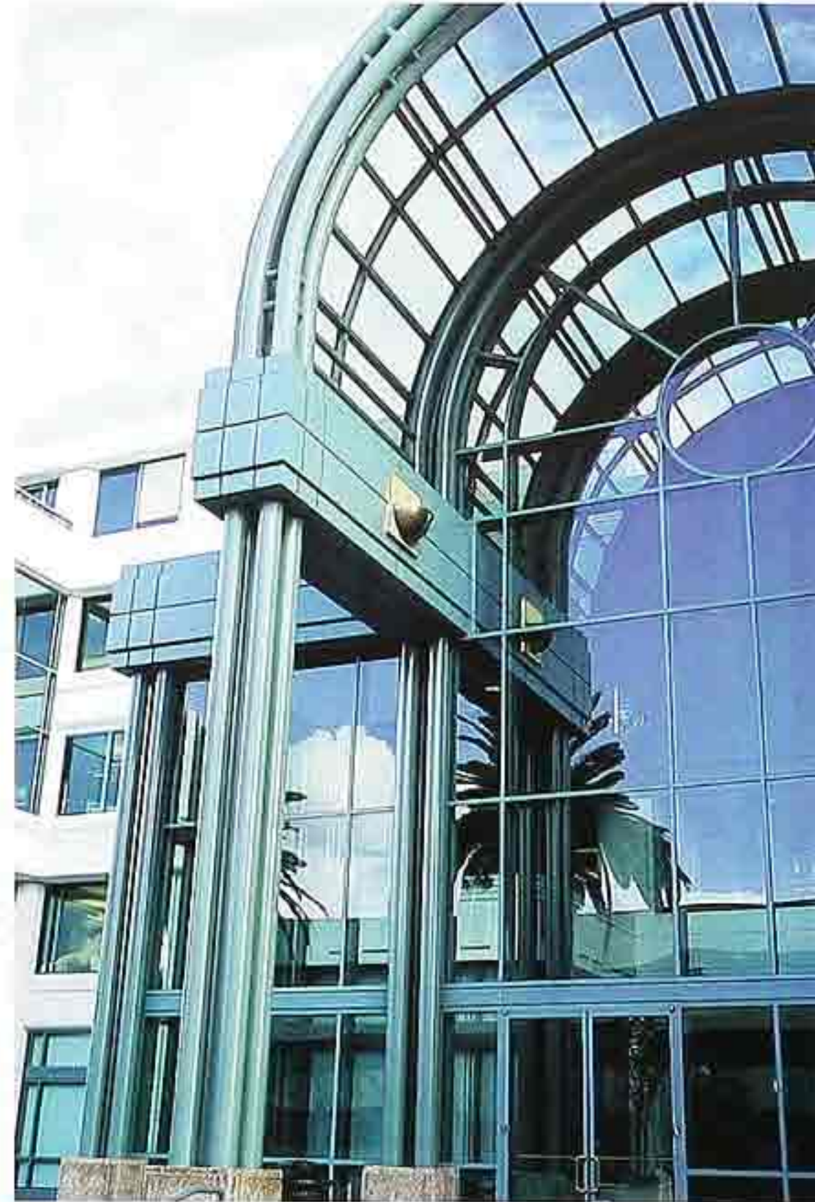
CP-177 Barrel-vaulted tubular-steel-frame-and-glass entry, modern commercial building
