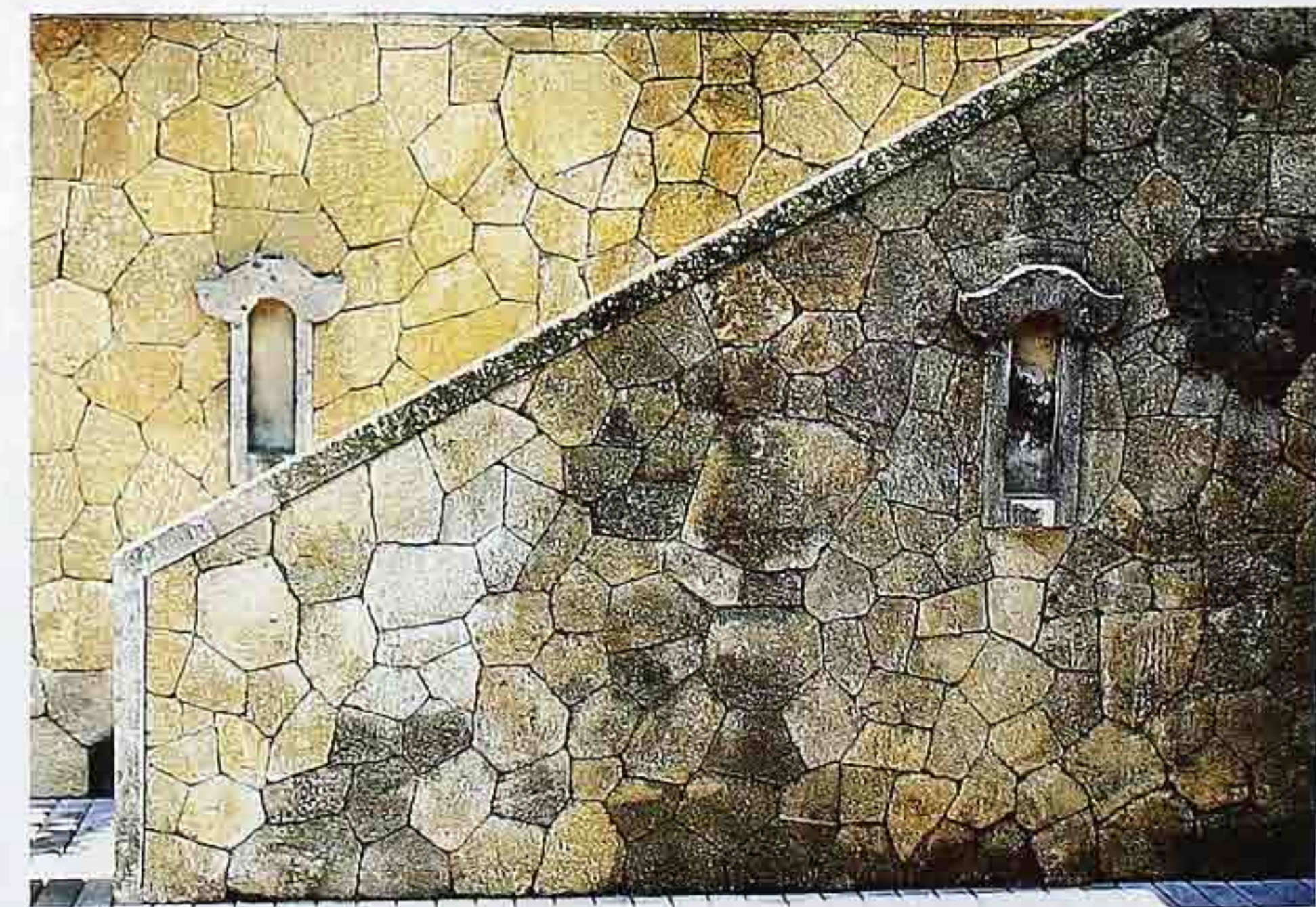
WA-122 Staircase wall in mosaic-bond rubble with niches and stone coping
