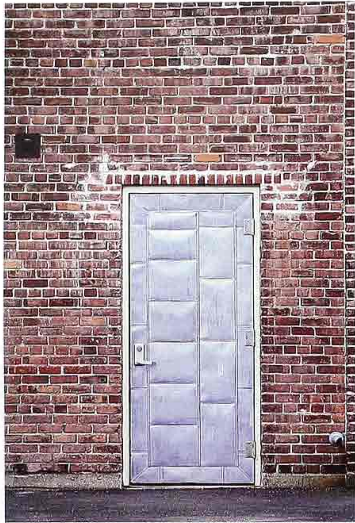
DW-52 Metal-clad door with "quilted" panels; brick surround with rowlock course above door opening
