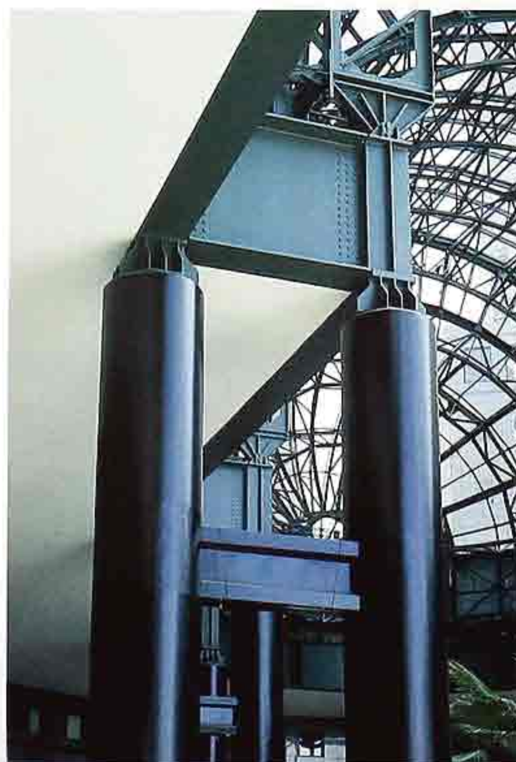
CP-115 Poured-in-place concrete piers supporting deep steel plate girders
