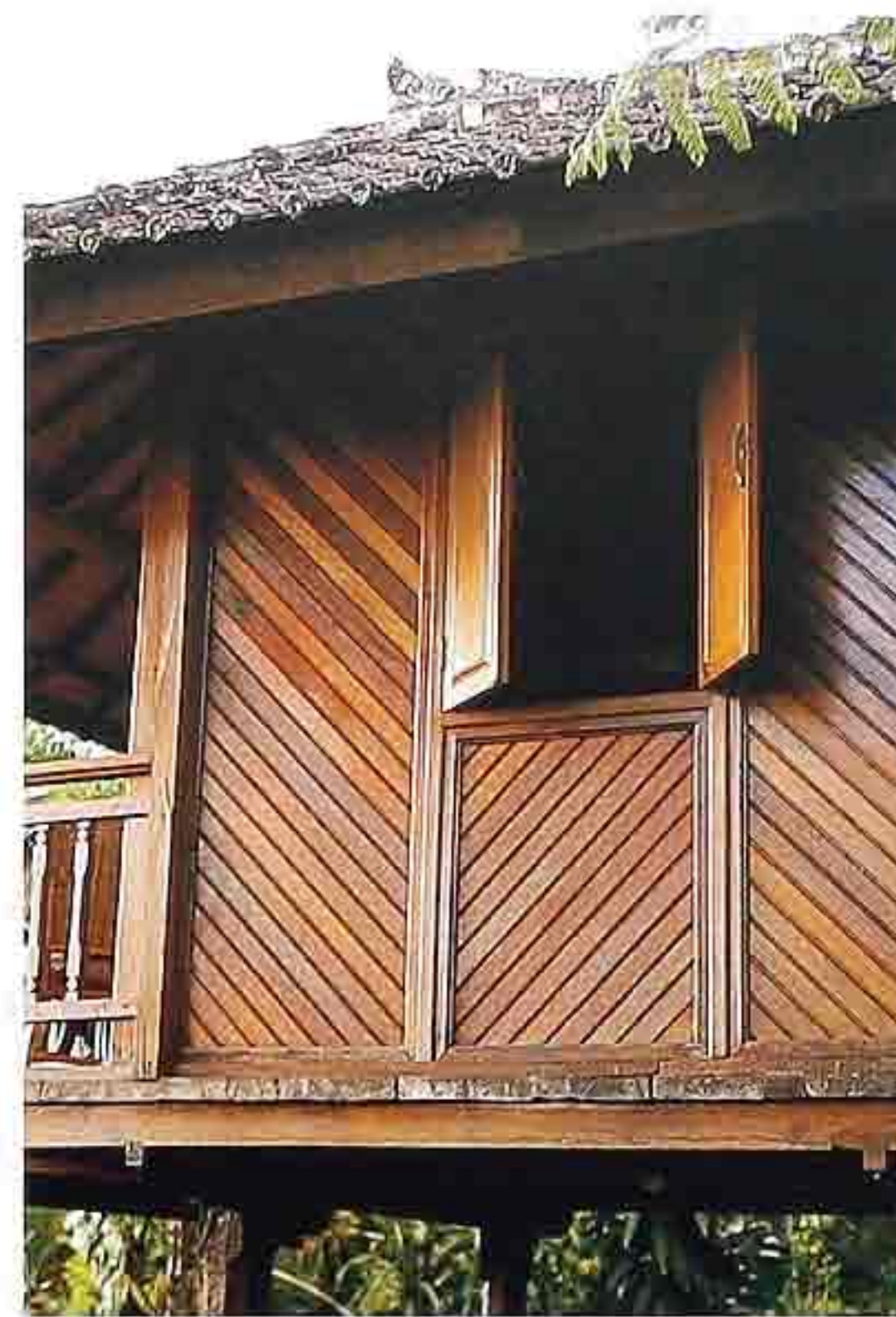
WA-40 Tongue-and-groove panels in alternating diagonal patterns, Indonesian house on stilts
