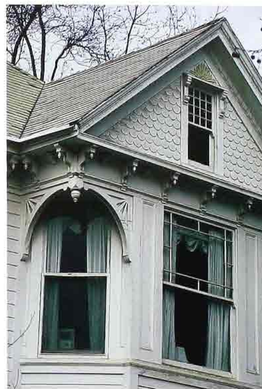
WI-51 Double-hung windows: one-over-one (left); six-over-one (gable); one-over-one decorative-lights (right), 19th-c. clapboard house
