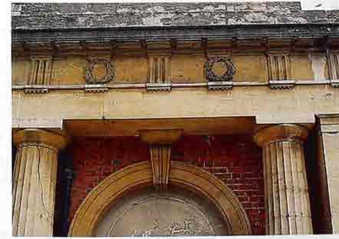
OM-96 Doric entablature: wreaths substituted for two triglyphs in the frieze; plain mutules in the soffit
