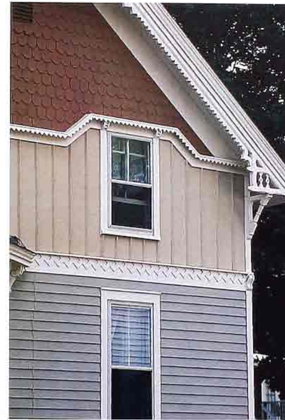
WA-32 Painted siding divided by molding. Top to bottom: scalloped wood shingles; board-and-batten; clapboard. Bargeboard with saw-tooth motif
