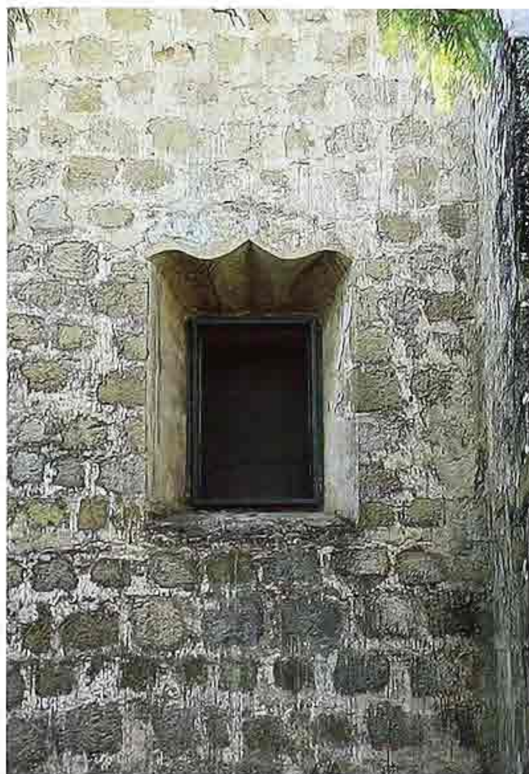
WI-121 Shaped embrasure in coursed-rubble wall, 19th-c. American Southwestern mission
