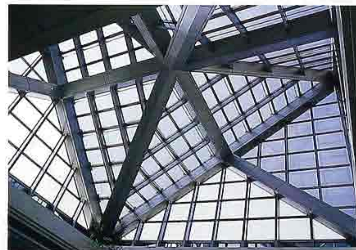
CR-18 Metal-framed glass atrium ceiling, modern commercial building
