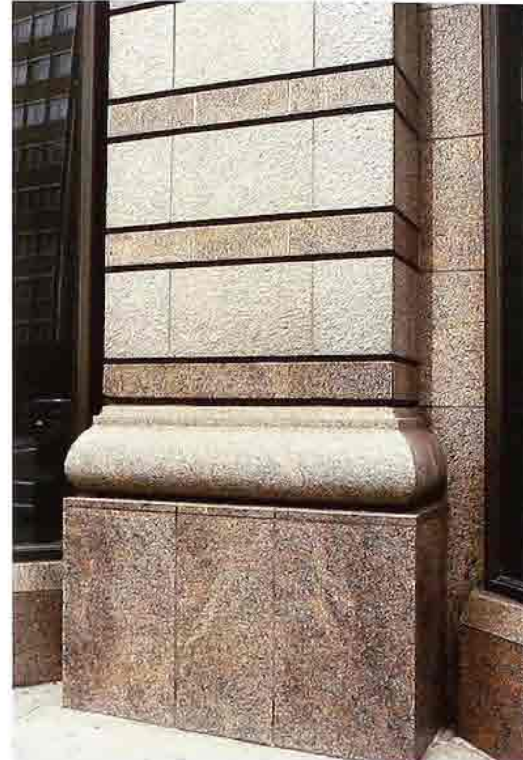
CP-45 Banded granite veneer pilaster on Tuscan-style base, entry of modern commercial building
