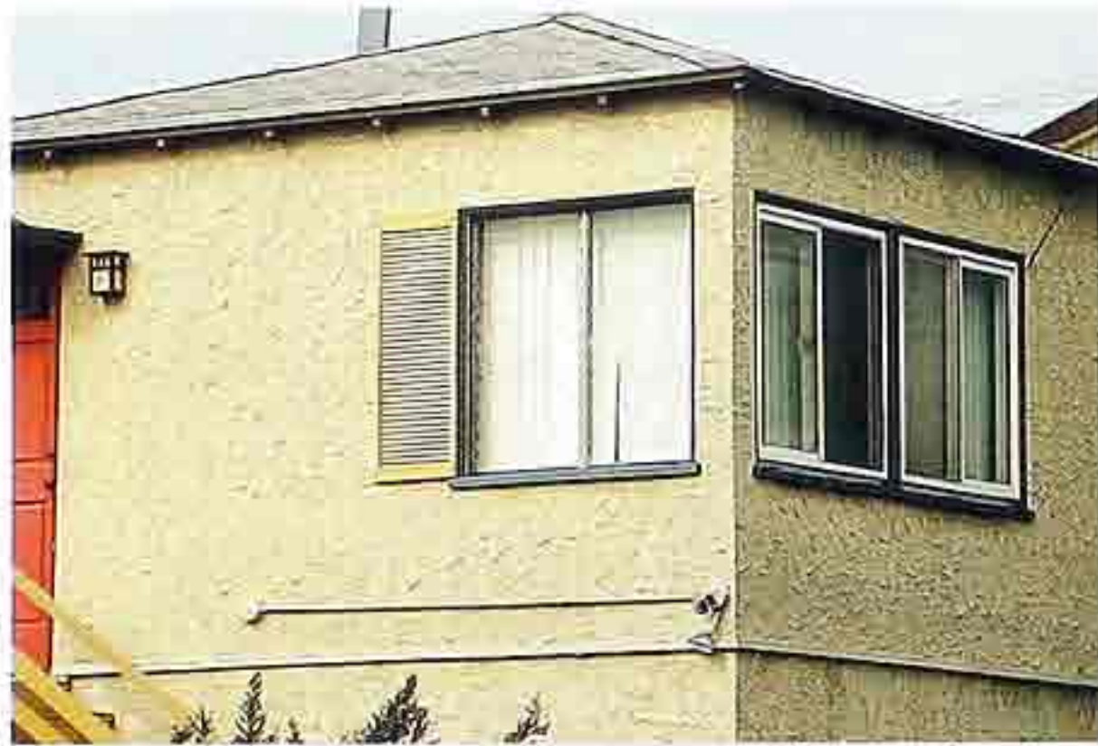
WA-238 Knocked-down skip-troweled stucco finish on beach house
