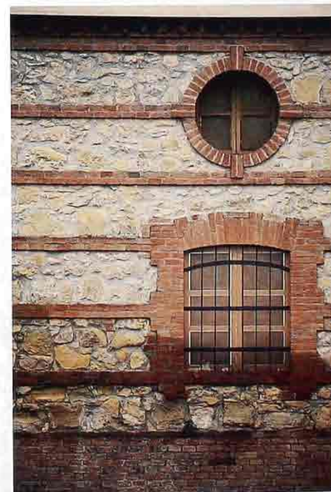
WA-288 Uncoursed rubble wall with brick-framed windows and brick belt courses; cambered arch window with trompe l'oeil grille and shutters
