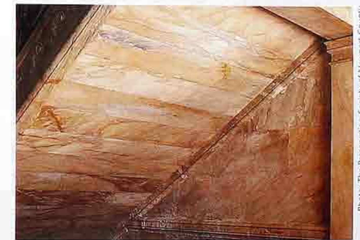
WA-104 Siena marble veneer on staircase soffit, molding and pilaster
