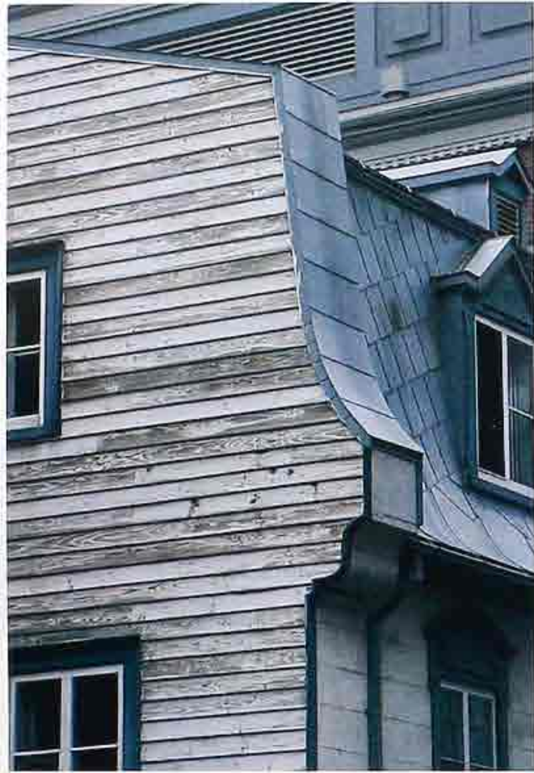
WA-36 Weathered untreated clapboard on gambrel-end wall rising from corbel detail
