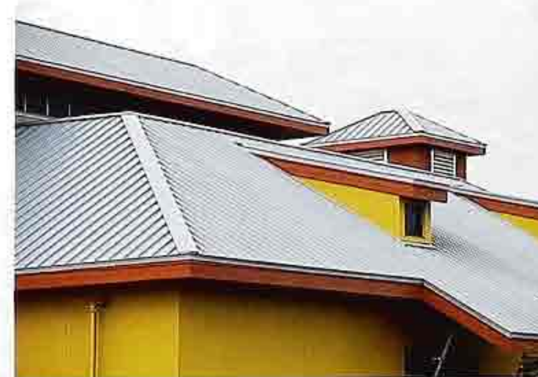
CR-101 Shed-roof dormer on metal hipped roof with standing seams, modern house
