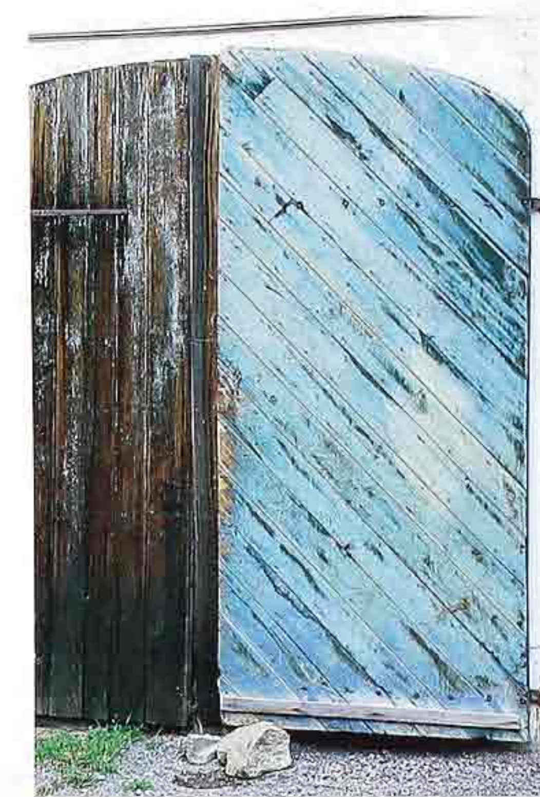
DW-34 Weathered wood double doors with rough-sawn vertical planks and painted diagonal planks
