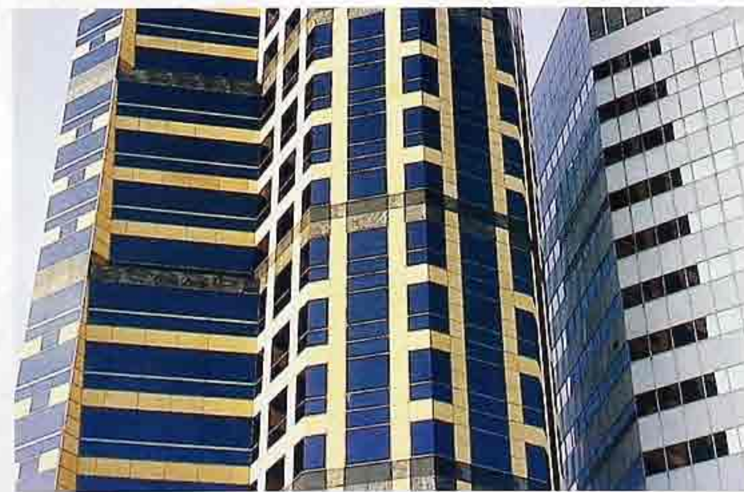
WA-301 Glass and stone curtain walls, modern commercial building
