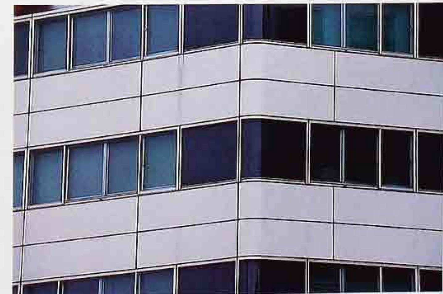
WI-166 Ribbon windows separated by solid panels, modern apartment building
