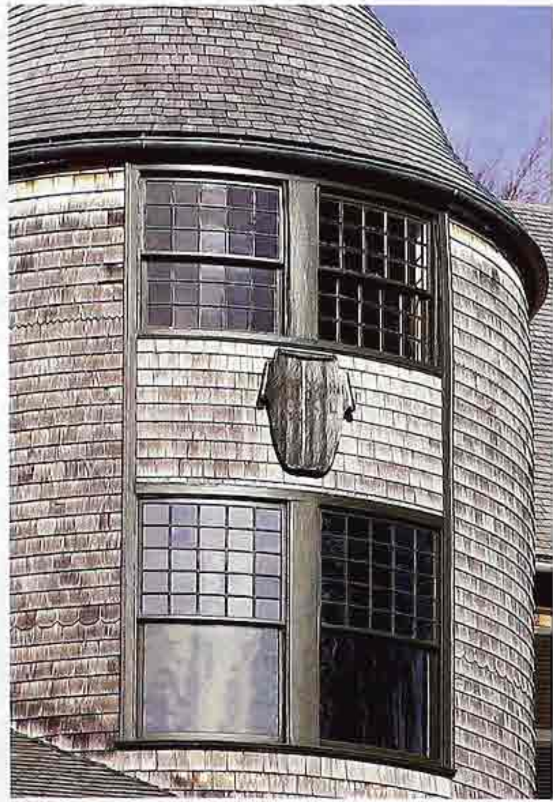
WI-55 Curved double-hung windows with slumped glass. Top: fifteen-over-fifteen; bottom: twenty-five-over-one, 20th-c. American shingle house
