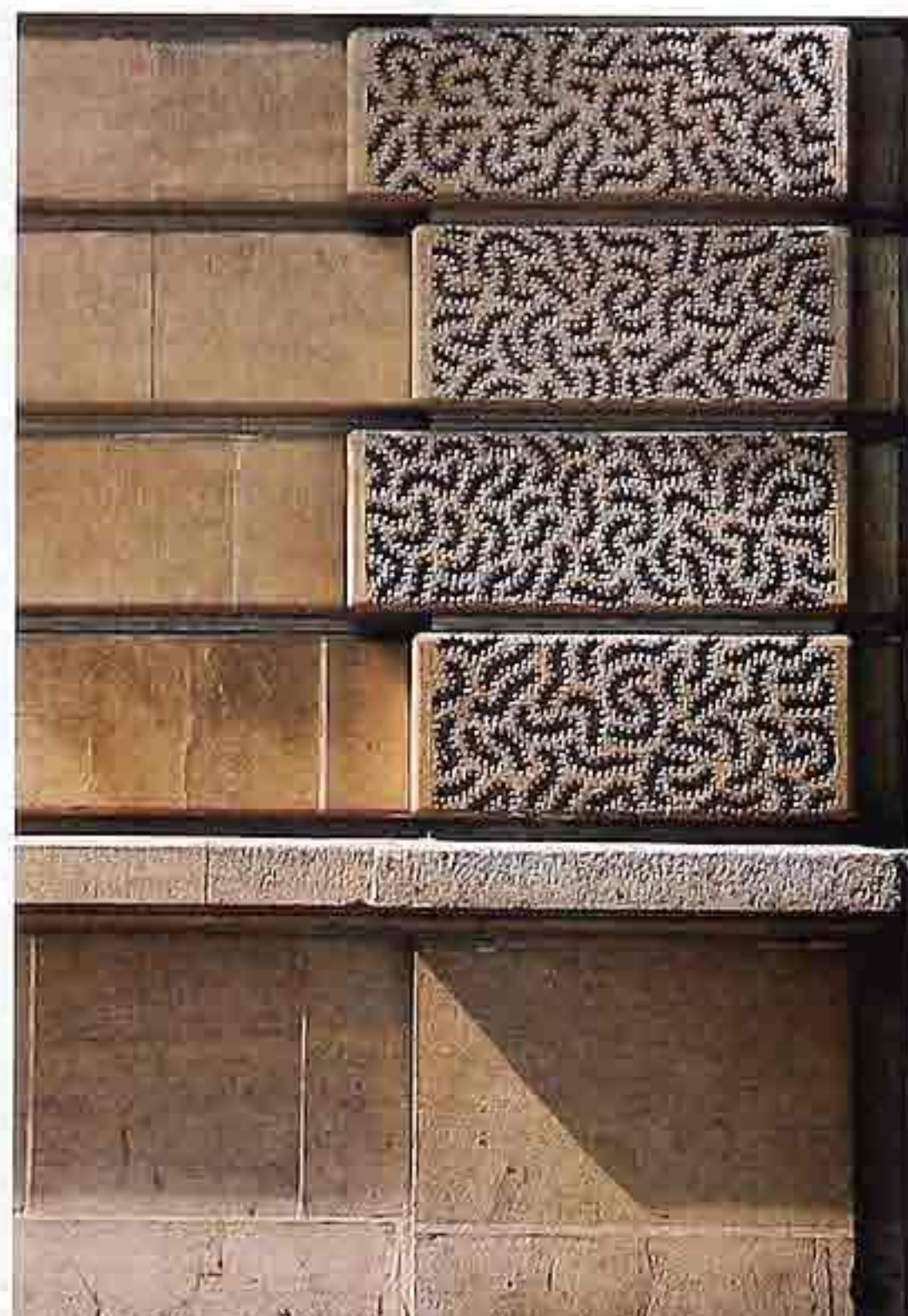
WA-92 Sawn ashlar sandstone courses, quoins with vermiculated finish
