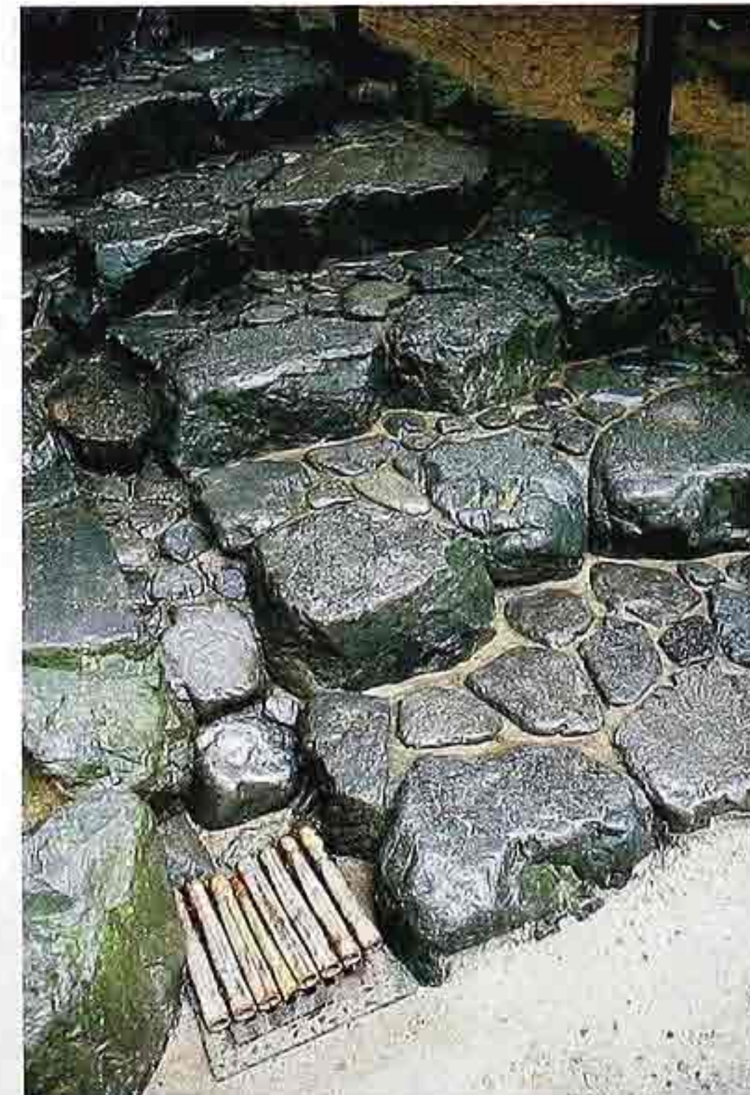
FP-46 Steps made from roughly squared split, polished fieldstone set in concrete. Bottom left: bamboo drain cover
