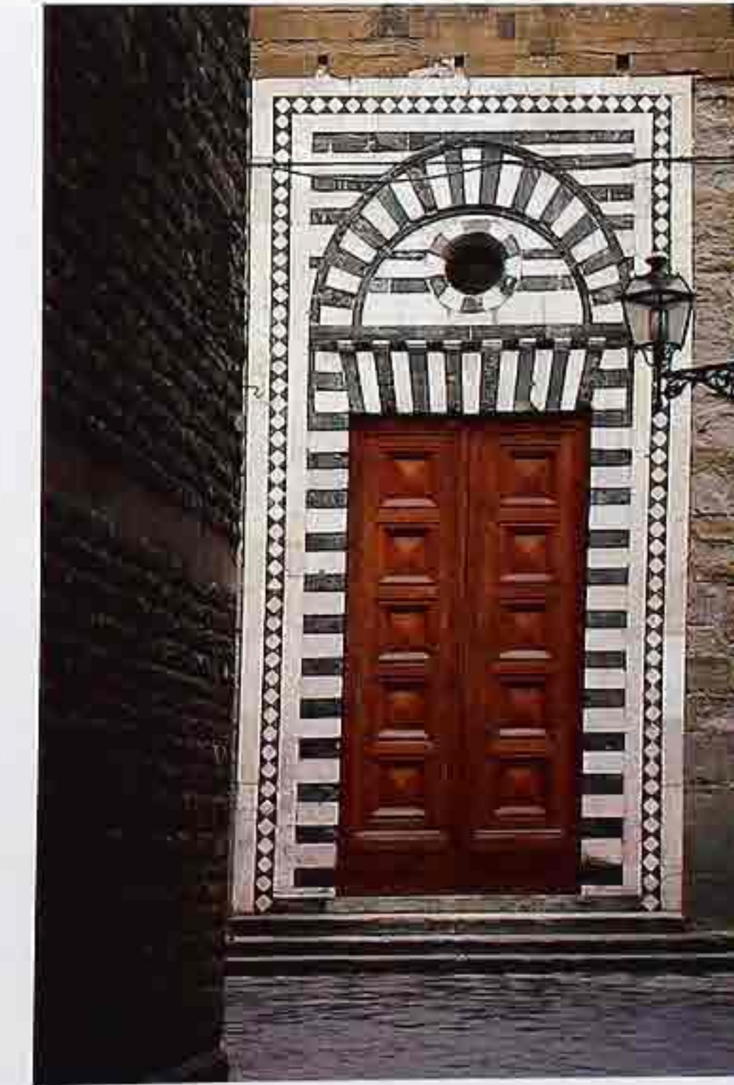
DW-79 Marble entry with diamond band, Florentine arch, and gauged-block jack arch over carved wood double doors, 16th-c. Italian church
