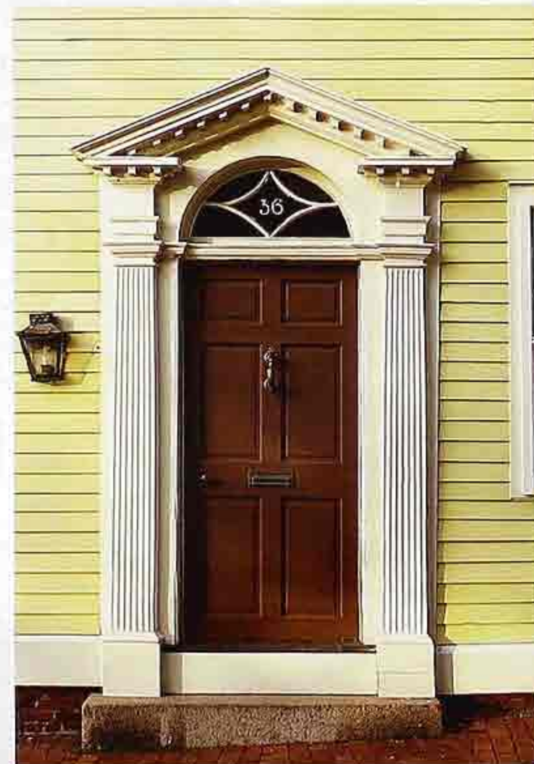
DW-83 Neoclassical pedimented door hood over pilasters and arched doorframe; wood panel door with fanlight
