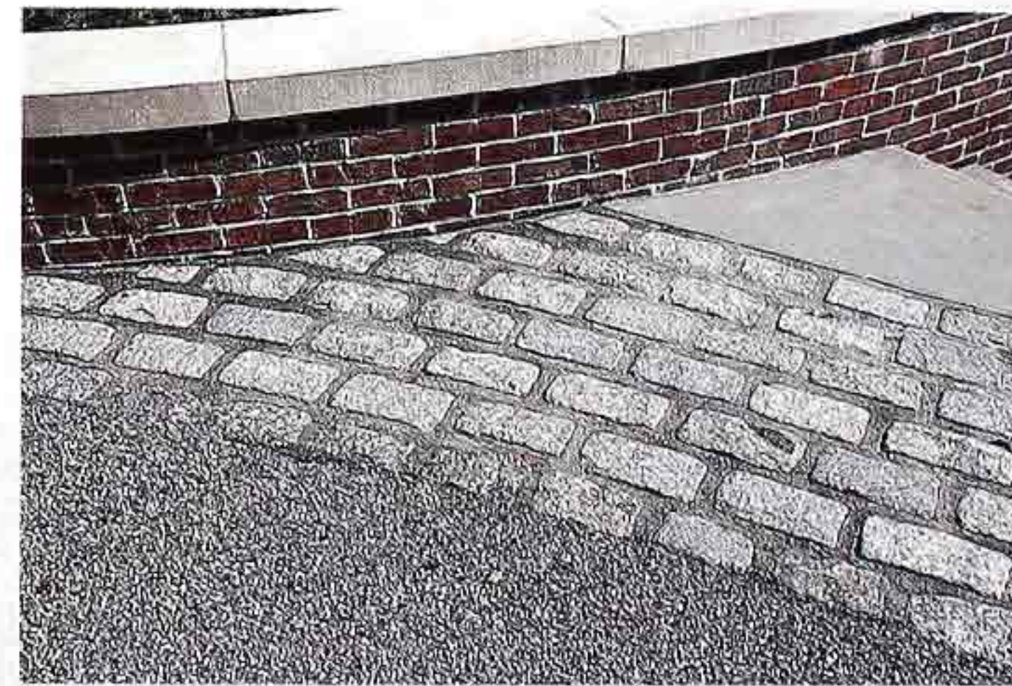
FP-56 Left to right: oiled stone gravel on asphalt paving; mortared running-bond cobblestones; New York bluestone step, residential driveway
