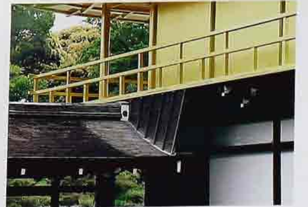
CR-114 Eave of shed roof connected to balcony to shelter courtyard walkway, traditional Japanese house
