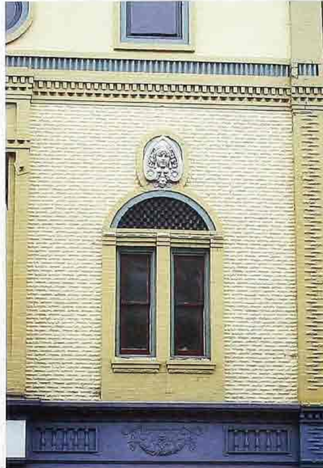
WA-176 Painted rock-face brick with dentil molding, pilasters, and double window under arch in recessed panel with cartouche
