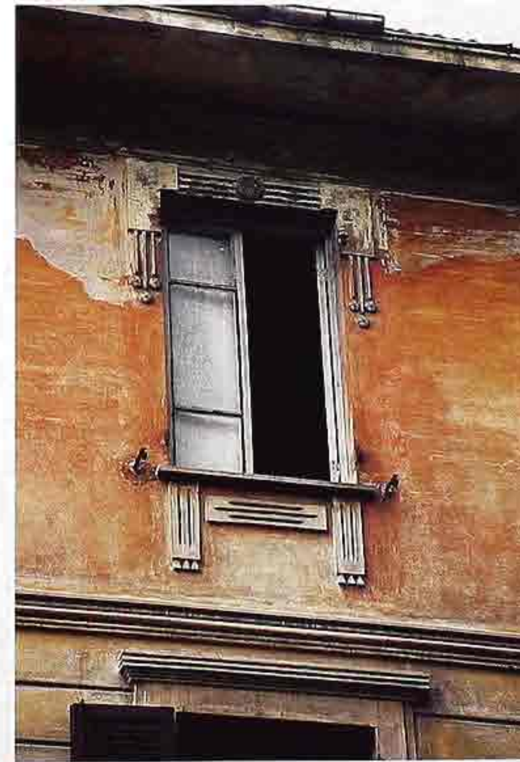
WI-36 Double-casement window in stucco wall
