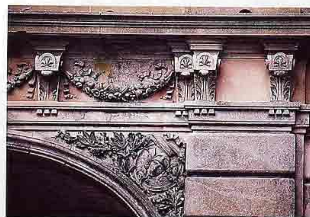
OM-52 Arch with sculpted spandrel. Entablature with frieze and festoons between consoles terminating in guttae below molding
