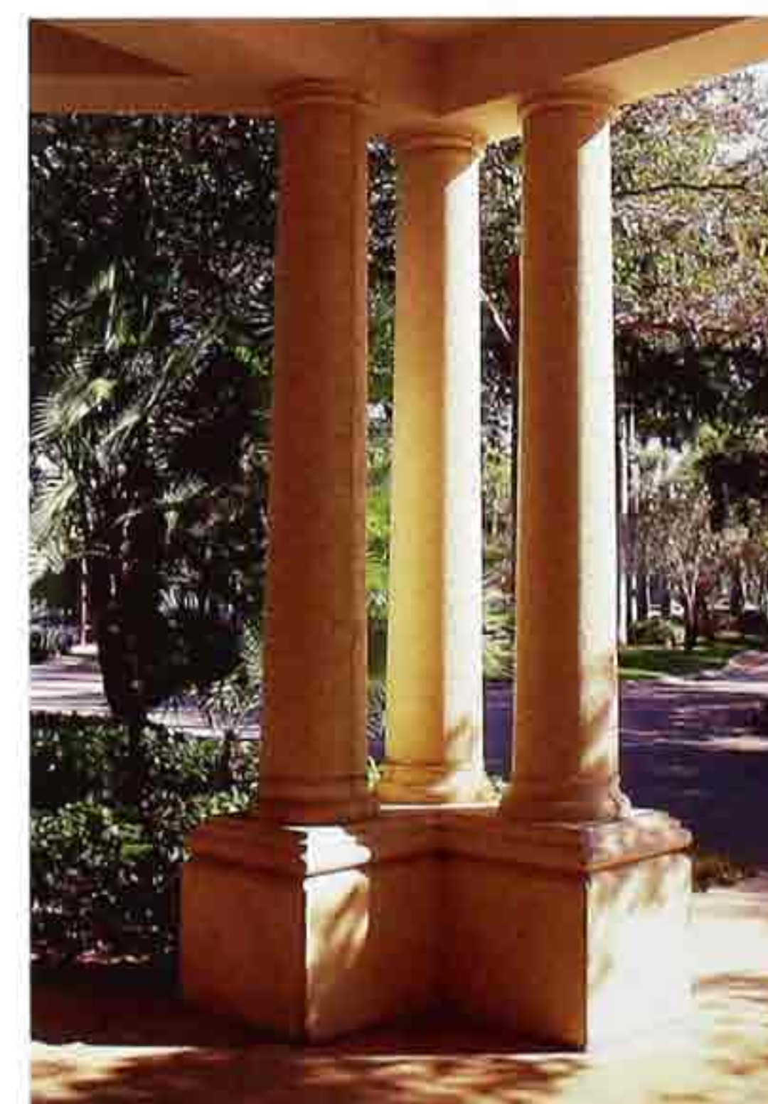
CP-71 Corner cluster of three columns with unresolved capitals
