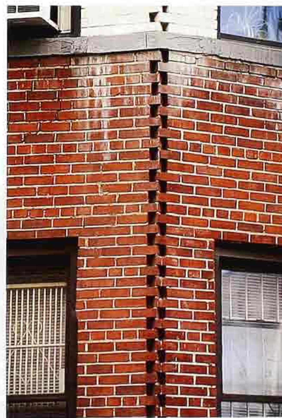
WA-195 Corner detail of common bond, sixth-course header, with dog's-tooth corner
