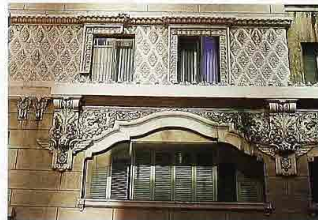
WI-145 Assortment of moldings and ornament around square casement windows over profiled fixed window
