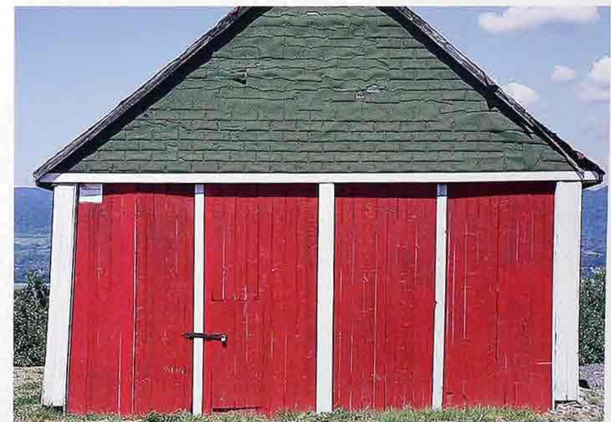
FA-81 Painted garage with shingles on gable end, vertical tongue-and-groove siding and door
