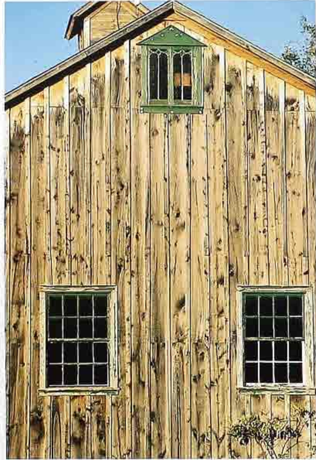
WA-28 Gable-end wall with unpainted board-and-batten siding and gable window
