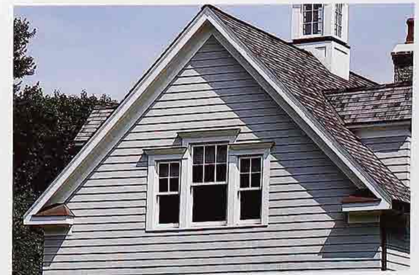
WI-117 Set of three gable wall double-hung windows; flat wood casings, with crown molding caps
