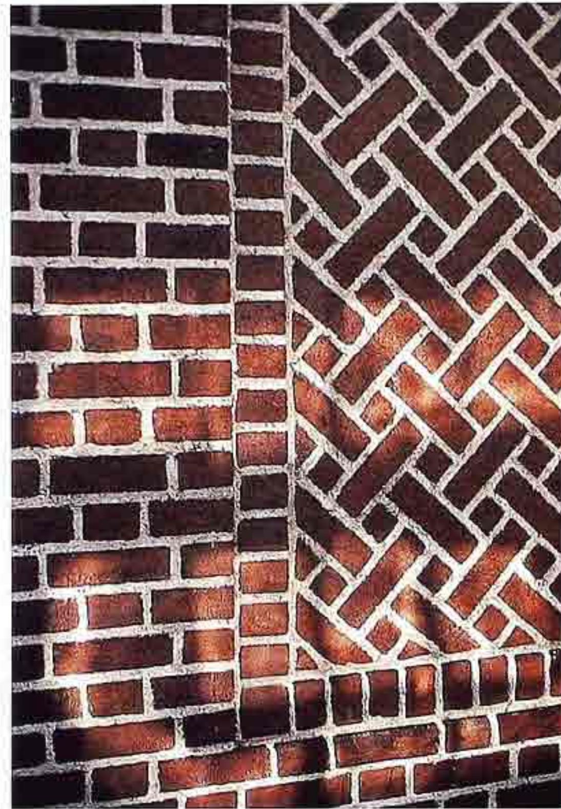
WA-166 Multiple bonds. Left to right: Flemish bond; rowlock and header frame; basket-weave
