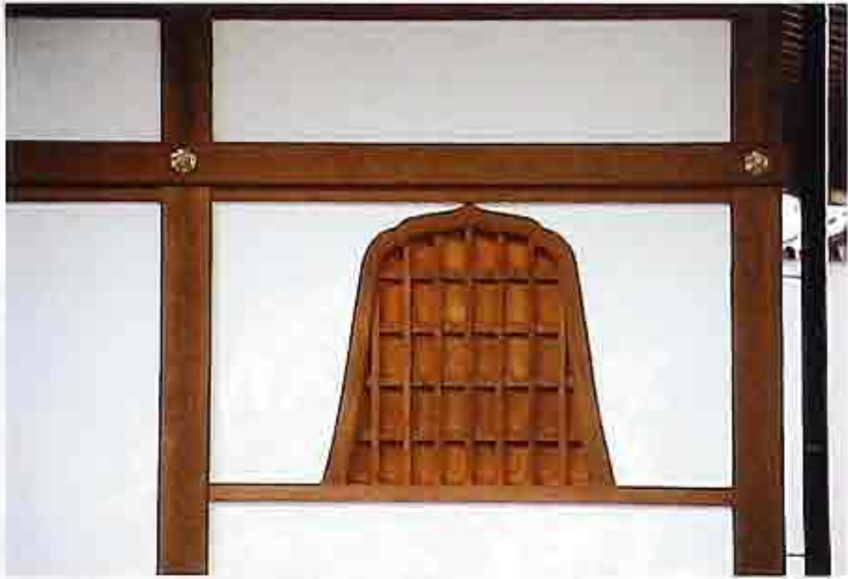
WA-275 Stucco infill; post-and-beam wall with decorative metal tie-irons at intersections of posts and beams, bell-shaped sliding shutter
