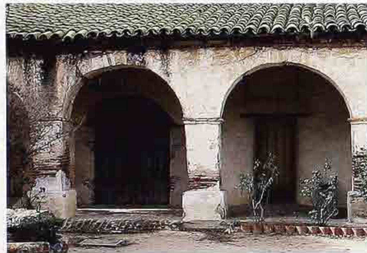
CP-164 Arcade with semicircular arches with molding at springing, stucco over adobe brick, late-18th-c. American Southwestern mission
