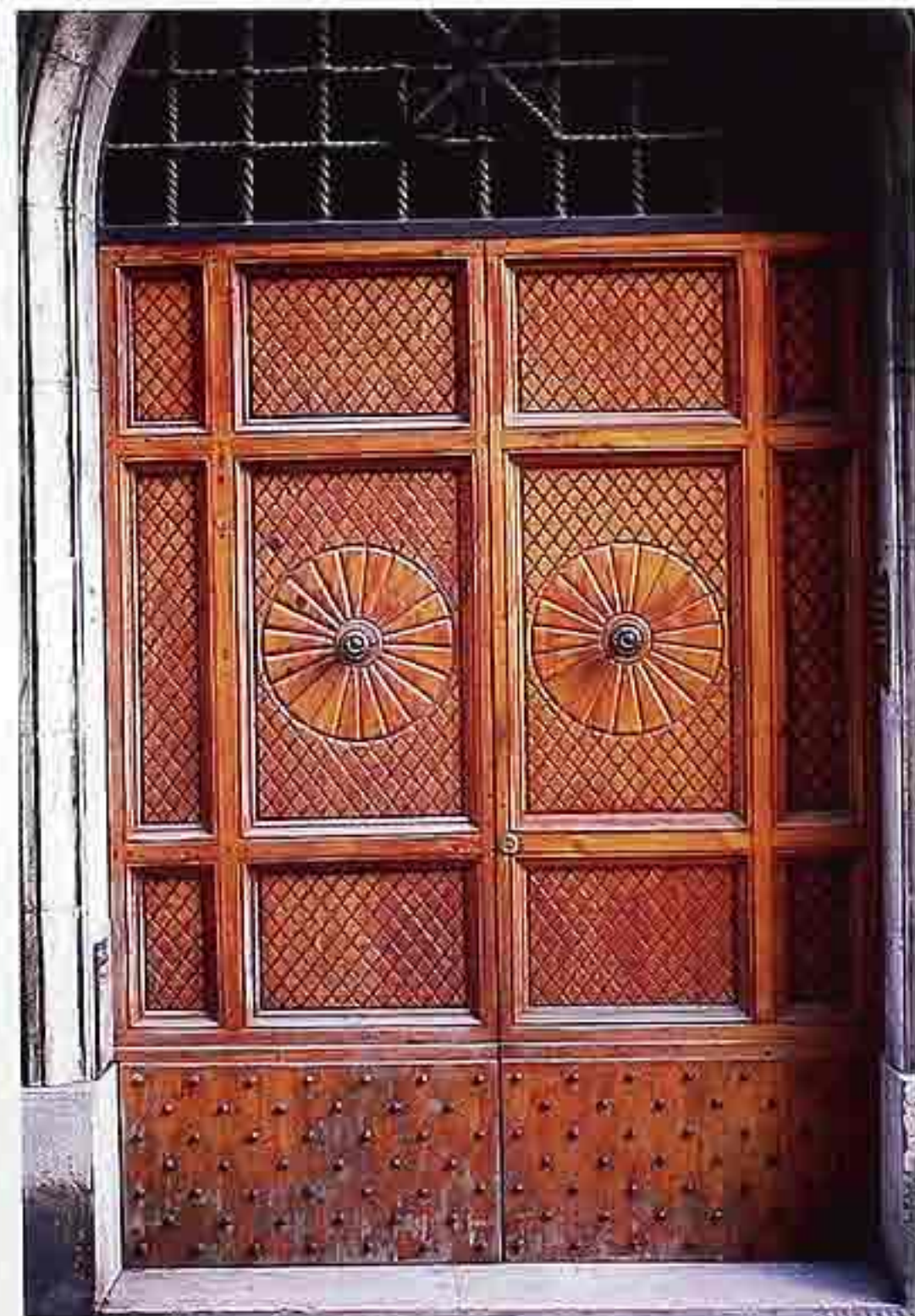
DW-3 Six panels, wood; double doors with carved diamond pattern in panels, ornament framing handles, studded bottom panel, and transom grille
