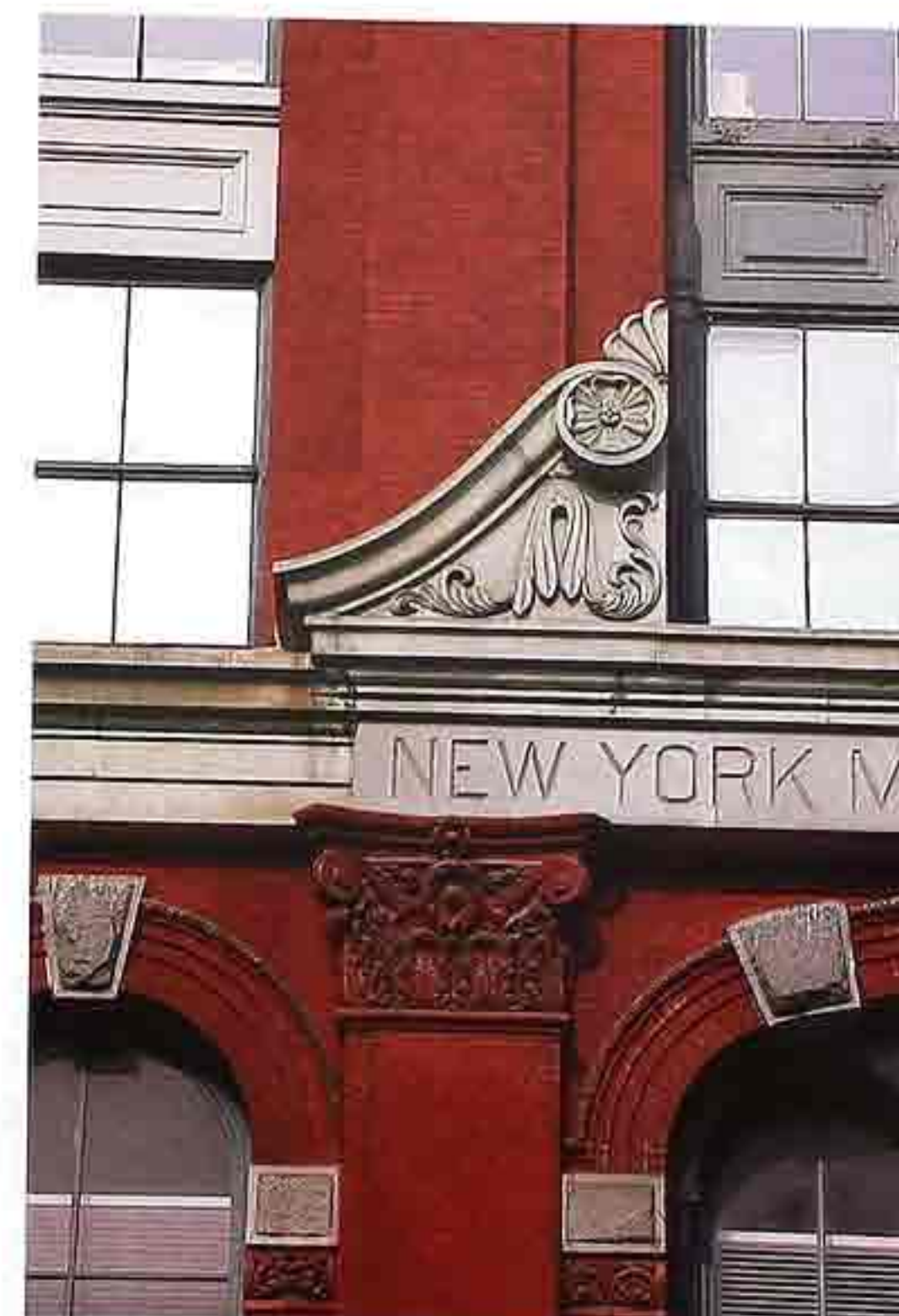
OM-53 Stylized broken scrolled pediment over a plain cornice and inscribed architrave
