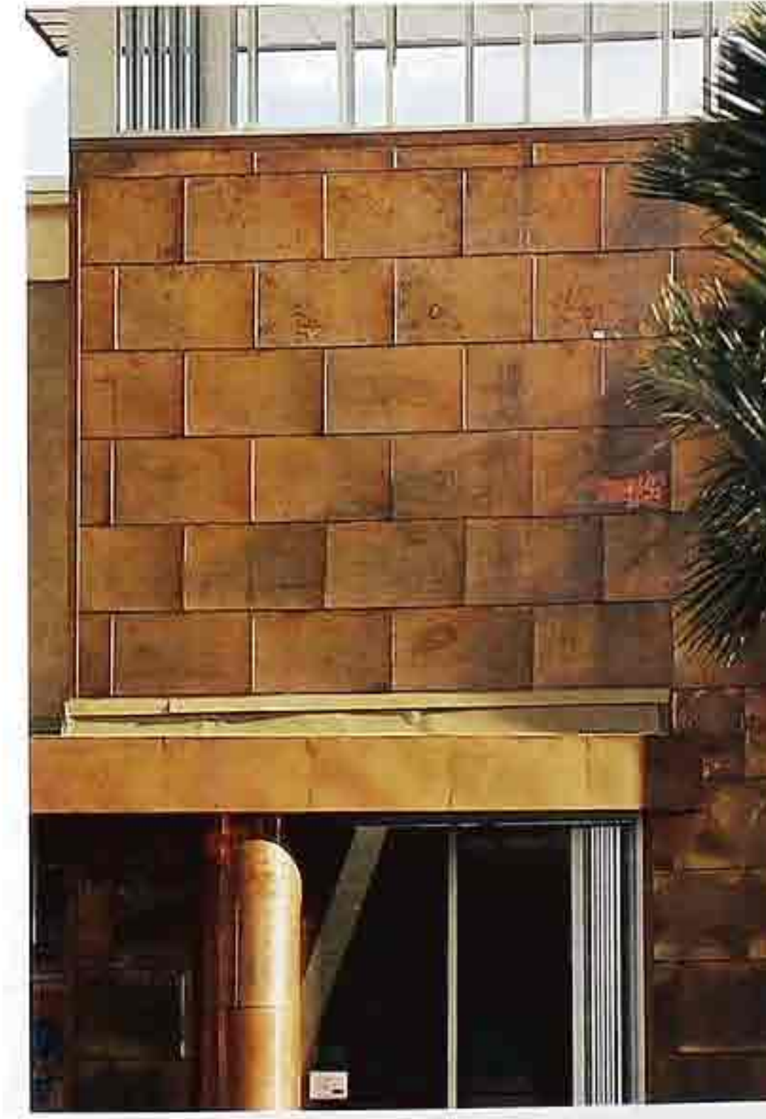
FA-17 Copper panels, possibly with standing vertical seams, lapped horizontally
