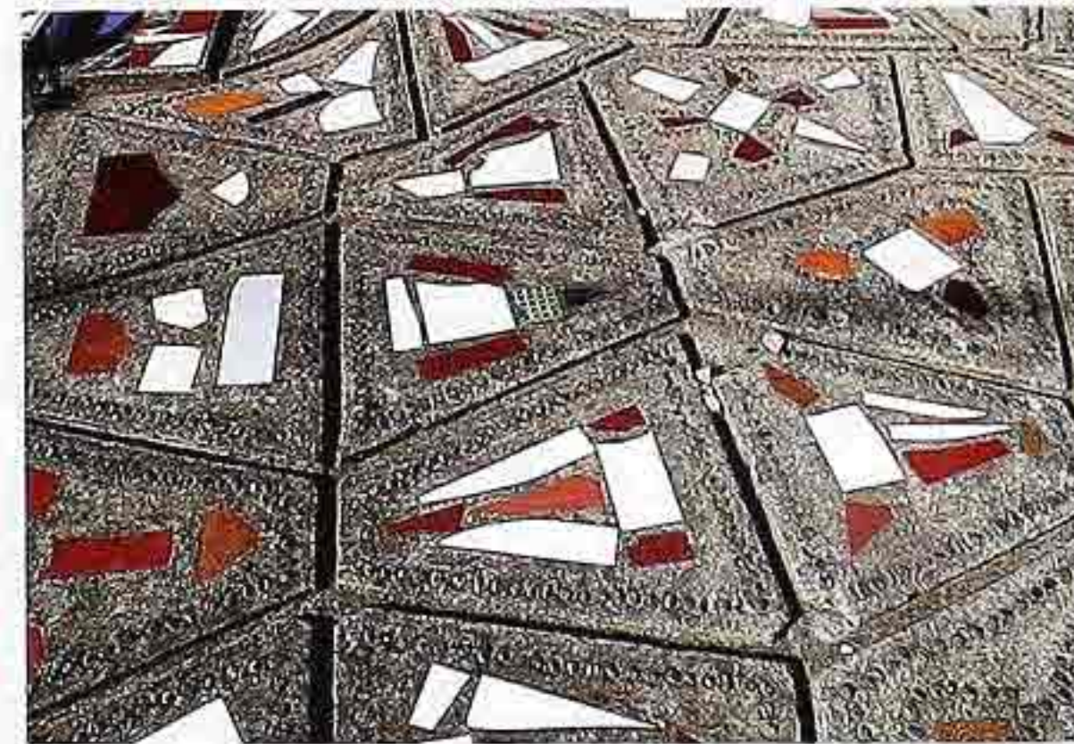
FP-94 Trapezoidal concrete pavers inlaid with ceramic tiles and pebbles, patio
