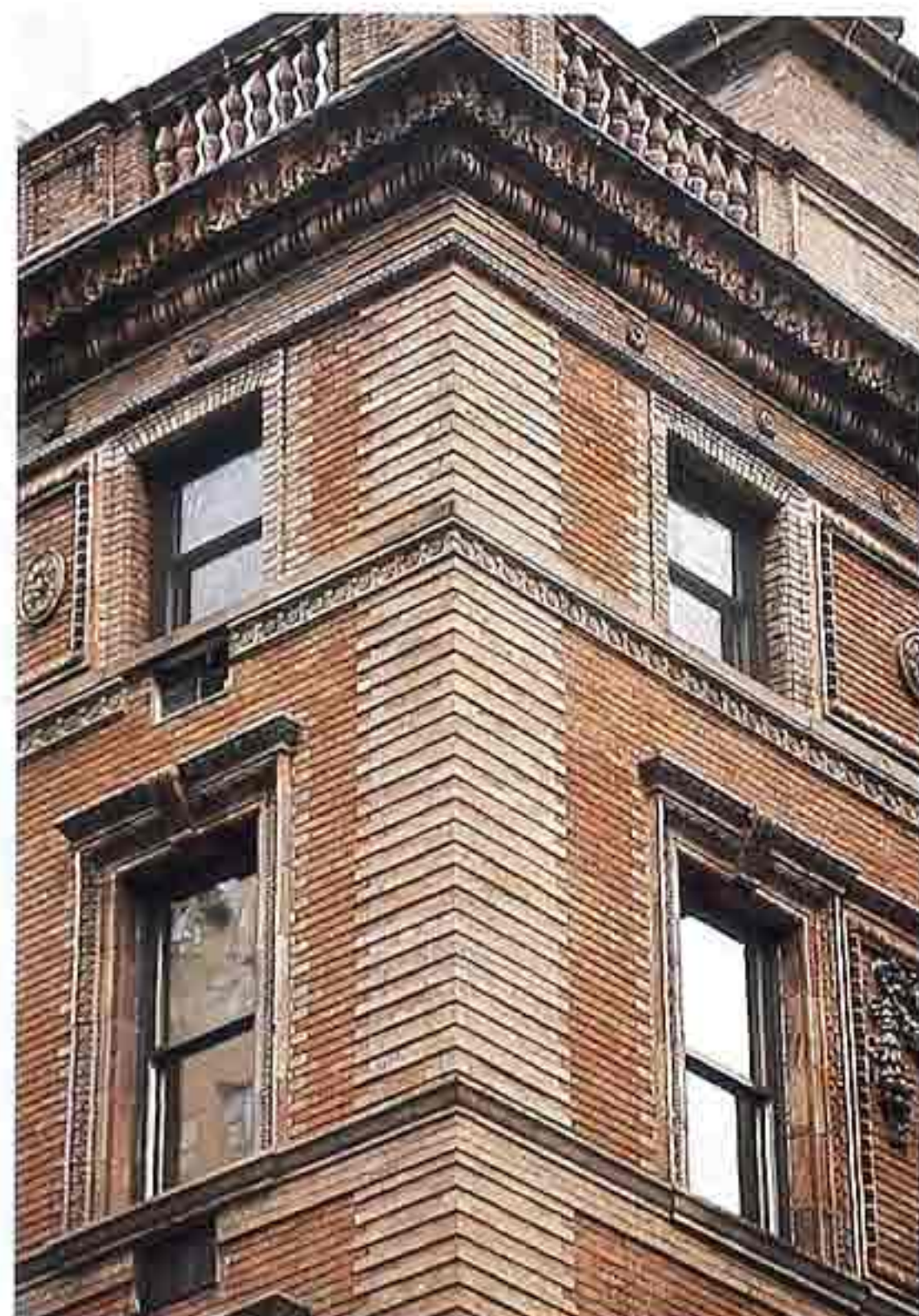
WA-192 Corner detail of brick and molded decorative brick or terracotta, 19th-c. apartment house
