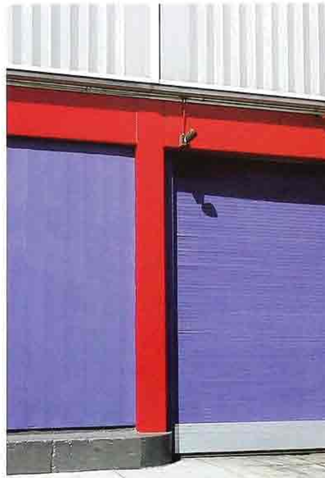
CP-113 Painted metal beam with welded connections; painted corrugated metal walls
