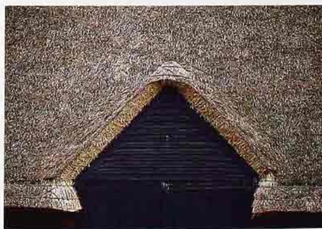
CR-74 Detail of thatching around gable, English barn
