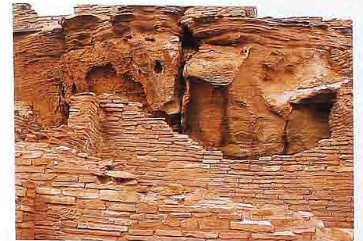
WA-77 Roughly squared sandstone in random ashlar attached to natural stone wall
