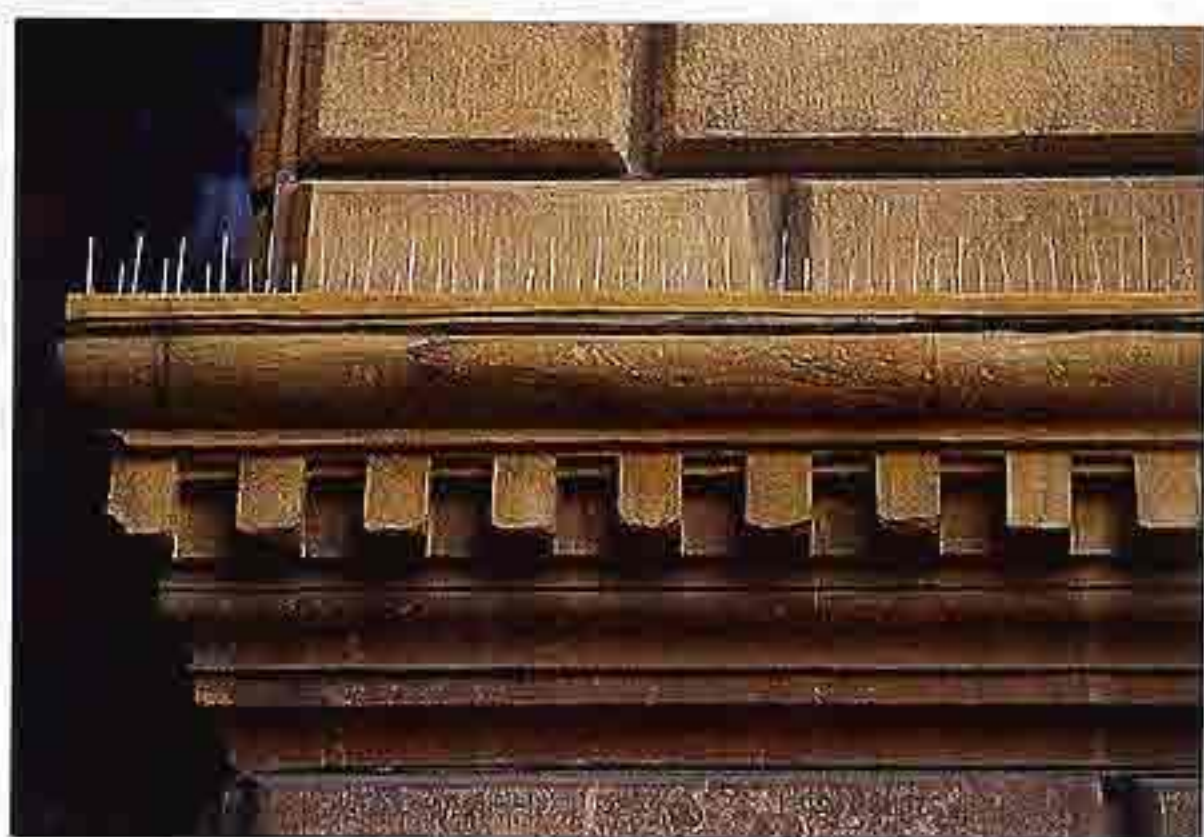
OM-70 Cornice. Top to bottom: plain ovolo molding, dentil band, plain cyma reversa, plain cyma recta
