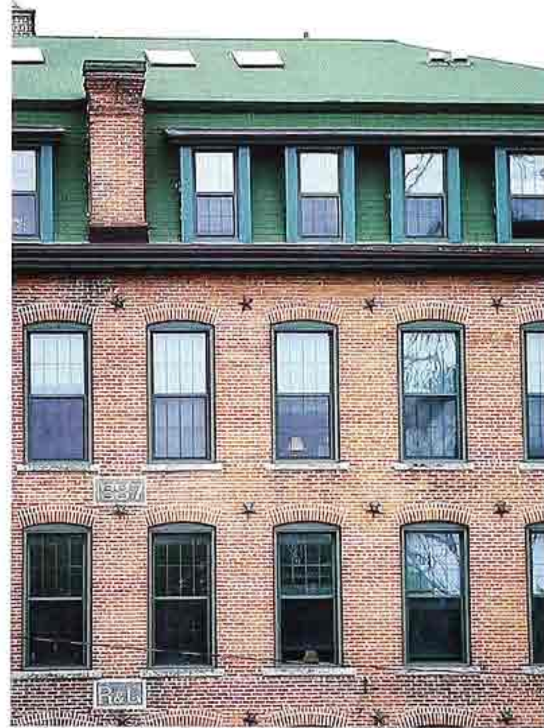
WI-56 Double-hung metal or vinyl replacement windows with internal muntins, 19th-c. brick industrial building
