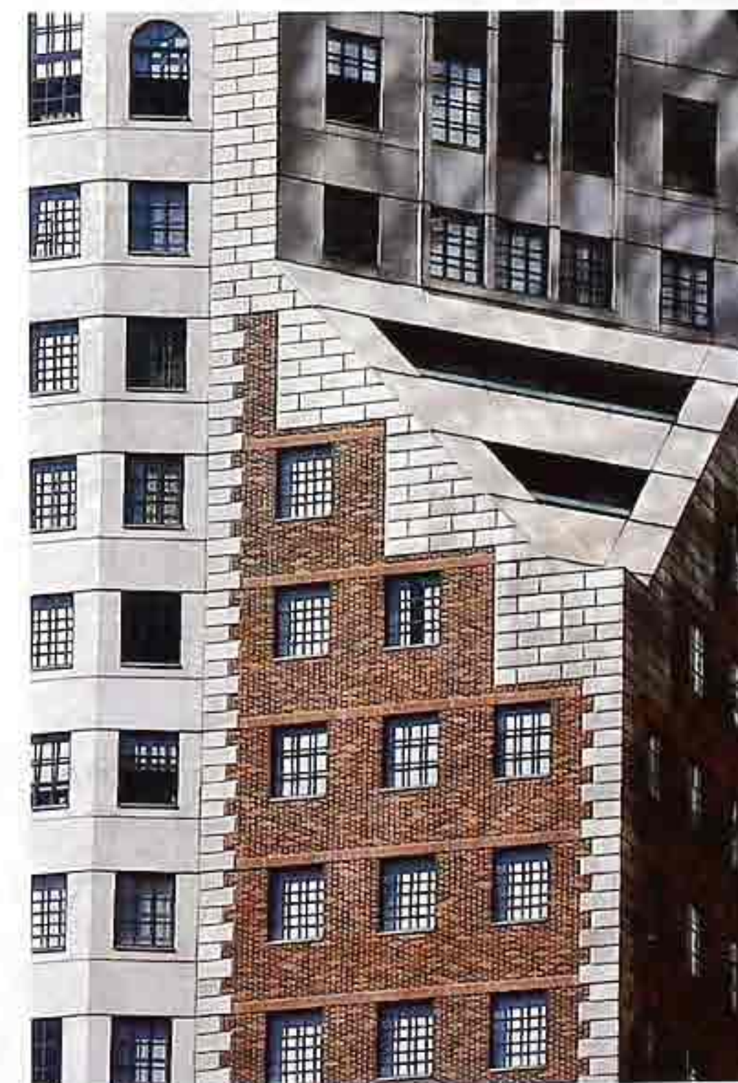
WA-304 Stone veneer and brick wing with stone-veneer quoins, modern commercial building
