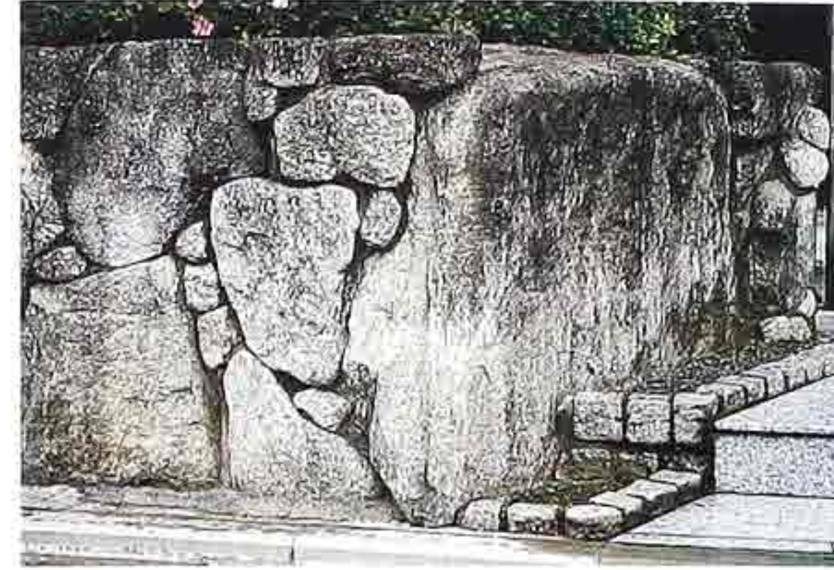
WA-76 Massive rubble with gallets, garden wall
