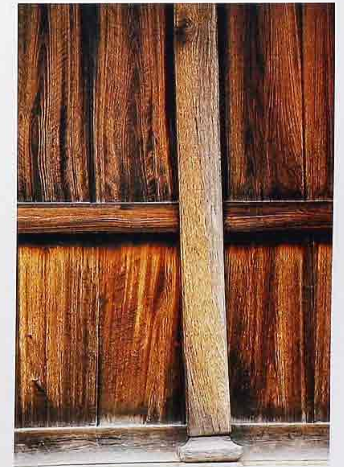
WA-43 Plain-sawn vertical planks with horizontal batten on shaped stone foundation; timber post with wood base
