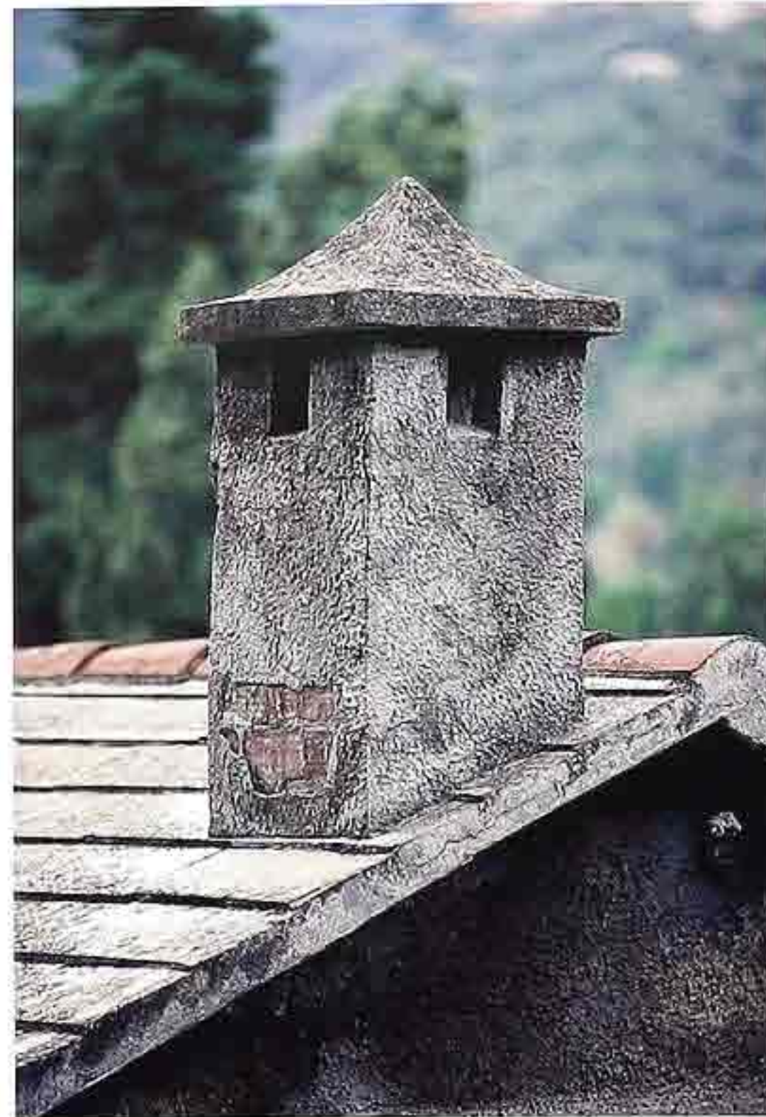
CR-148 Stucco-over-brick chimney with pyramidal hood
