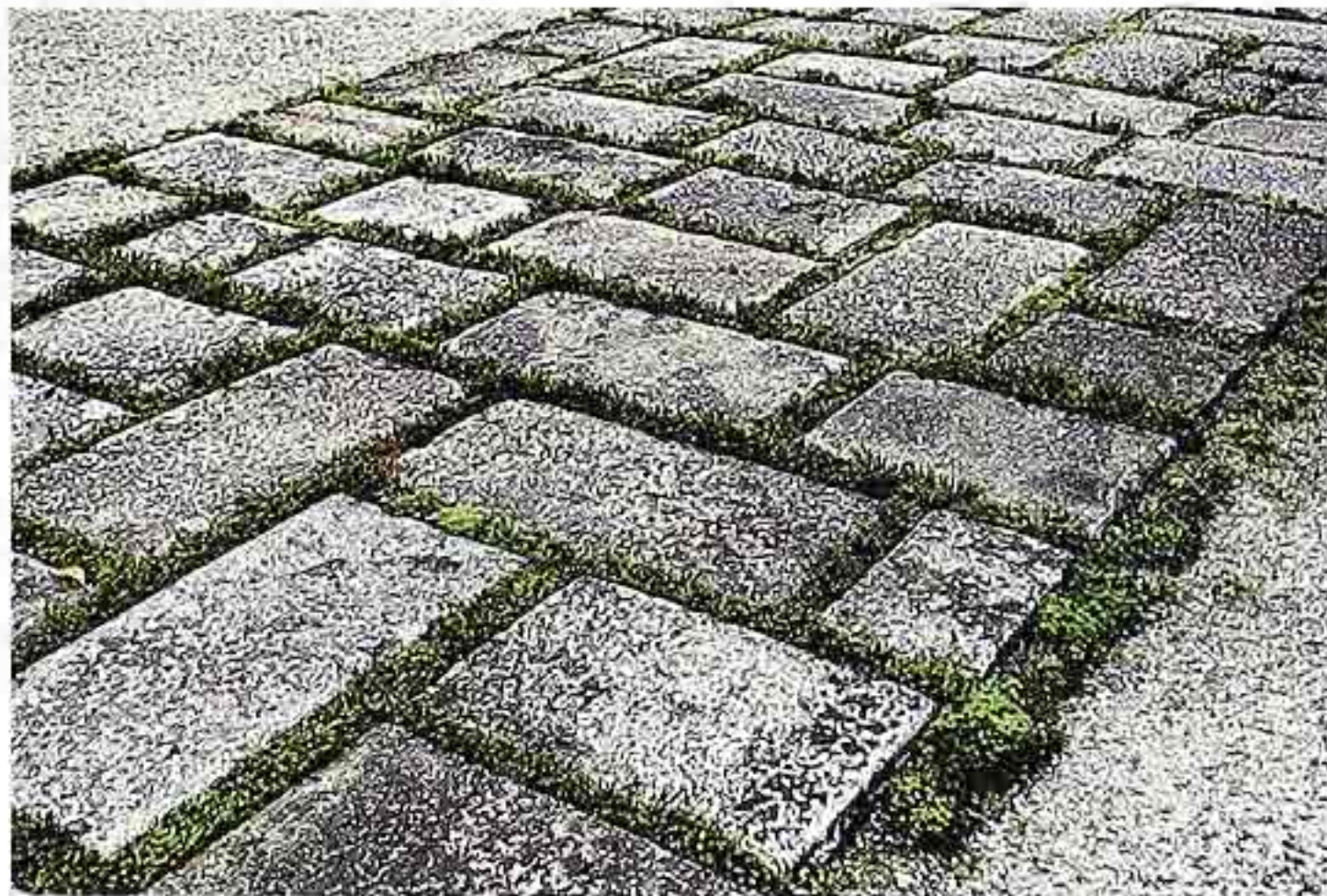
FP-29 Roughly squared paving stone in random-ashlar pattern with moss on sidewalk
