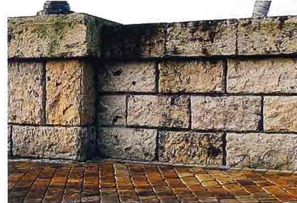
WA-78 Split-faced and rusticated Mexican volcanic stone in running bond, footbridge wall
