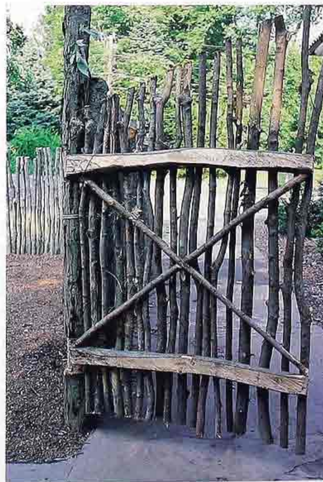
DW-112 Rustic garden gate of vertical branches attached to horizontal battens
