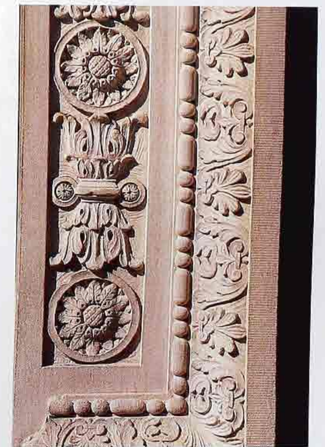
OM-66 Corner detail of enriched ovolo molding with trailing foliated pattern; bead-and-reel framing foliated design flanked by rosettes
