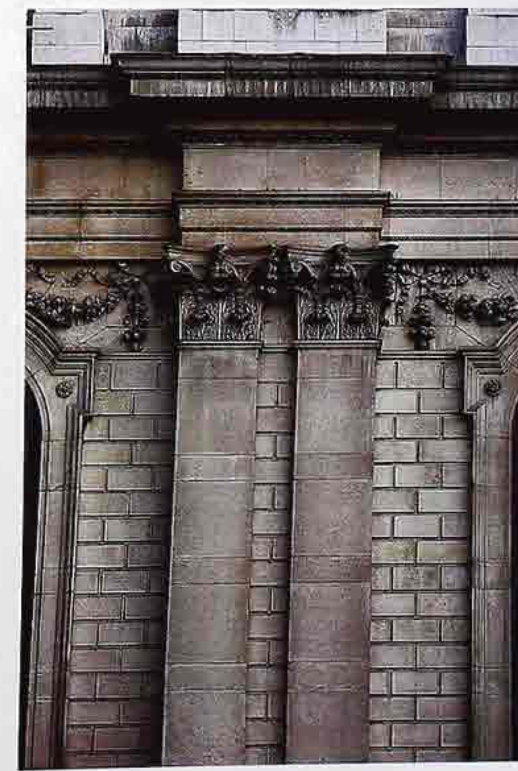
OM-104 Two-banded architrave, festooned frieze flanking Corinthian pilasters
