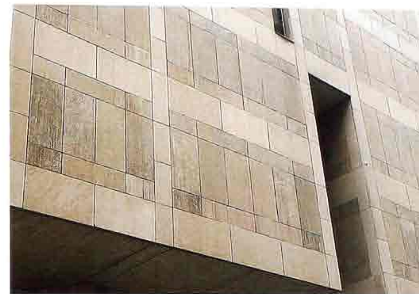
WA-135 Limestone-veneer panels framed by contrasting stack-and-running-bond courses, modern commercial building
