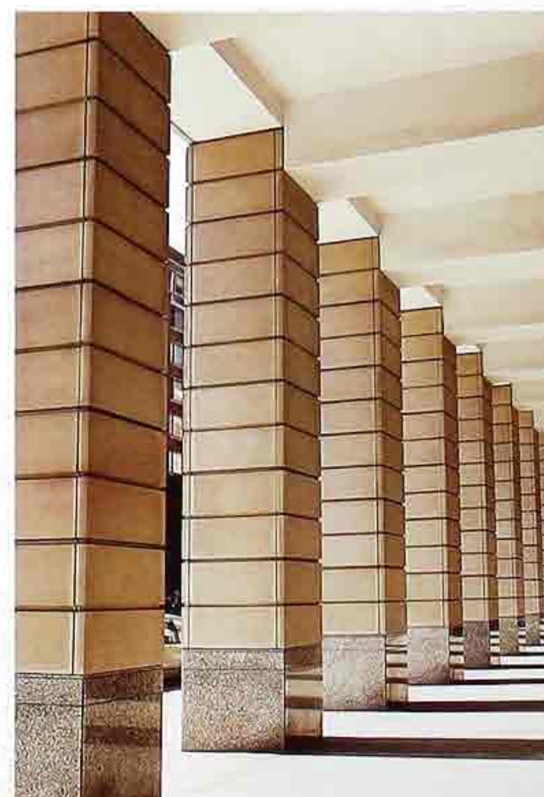
CP-136 Polished rusticated granite-veneer piers with adjoining boxed beams in arcade, modern commercial building
