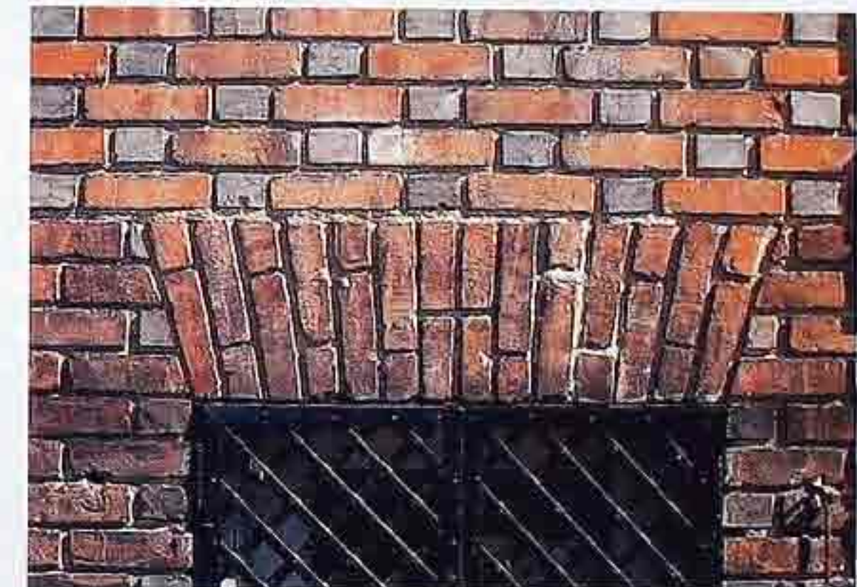
WA-172 Jack arch surrounded by Flemish bond in alternating colors
