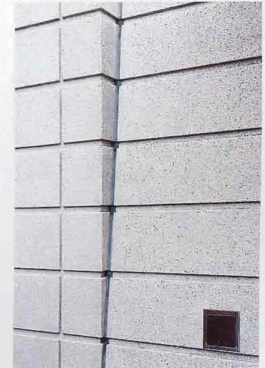
WA-220 Pre-cast coarse-aggregate concrete, modern commercial building
