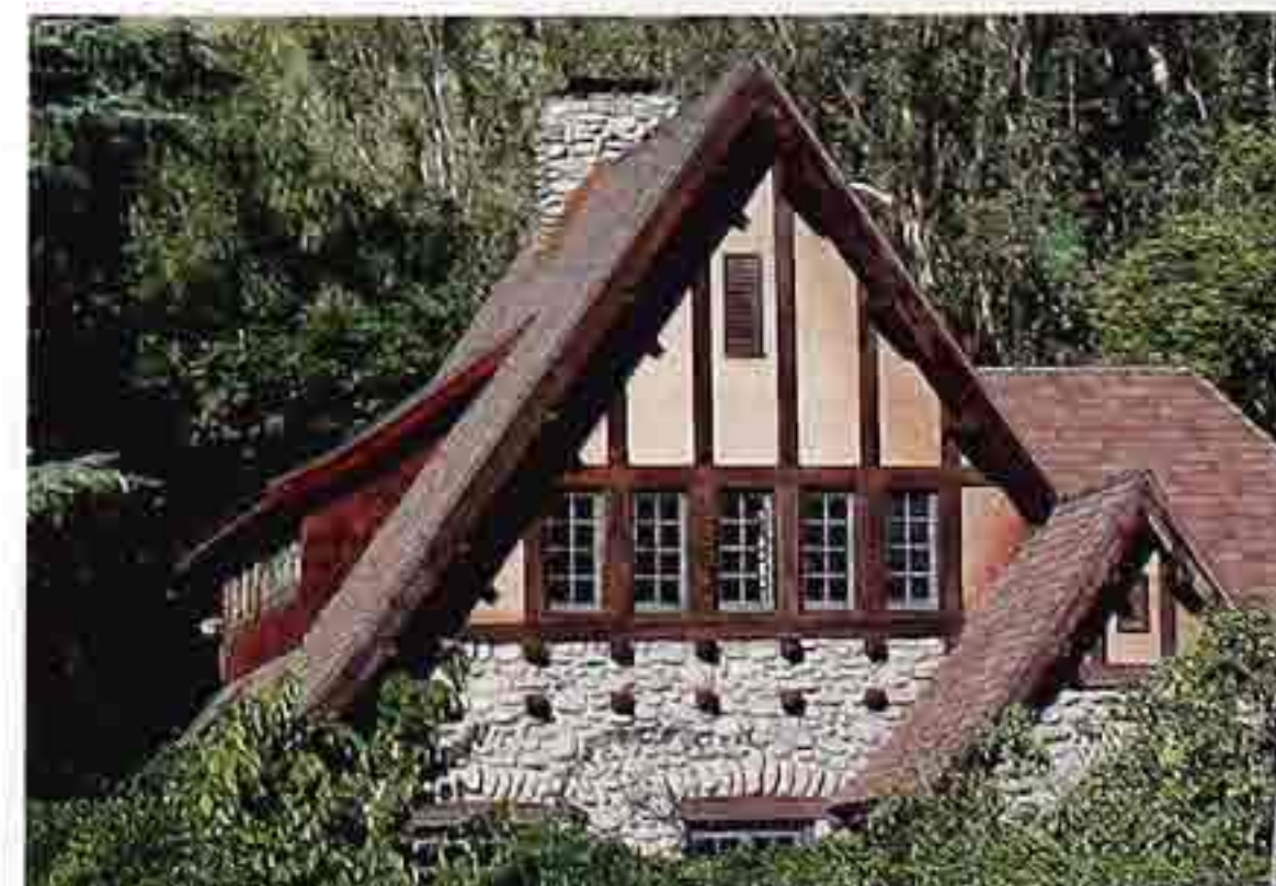
CR-124 Steep half-timbered gable with shed dormer
