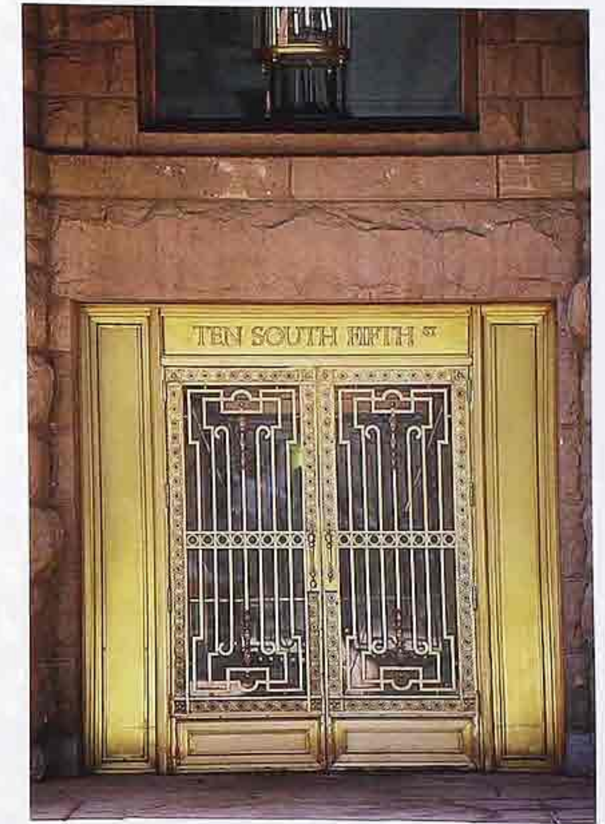
DW-50 Brass double doors; full glass behind ornate brass grille; brass panels flanking doorframe
