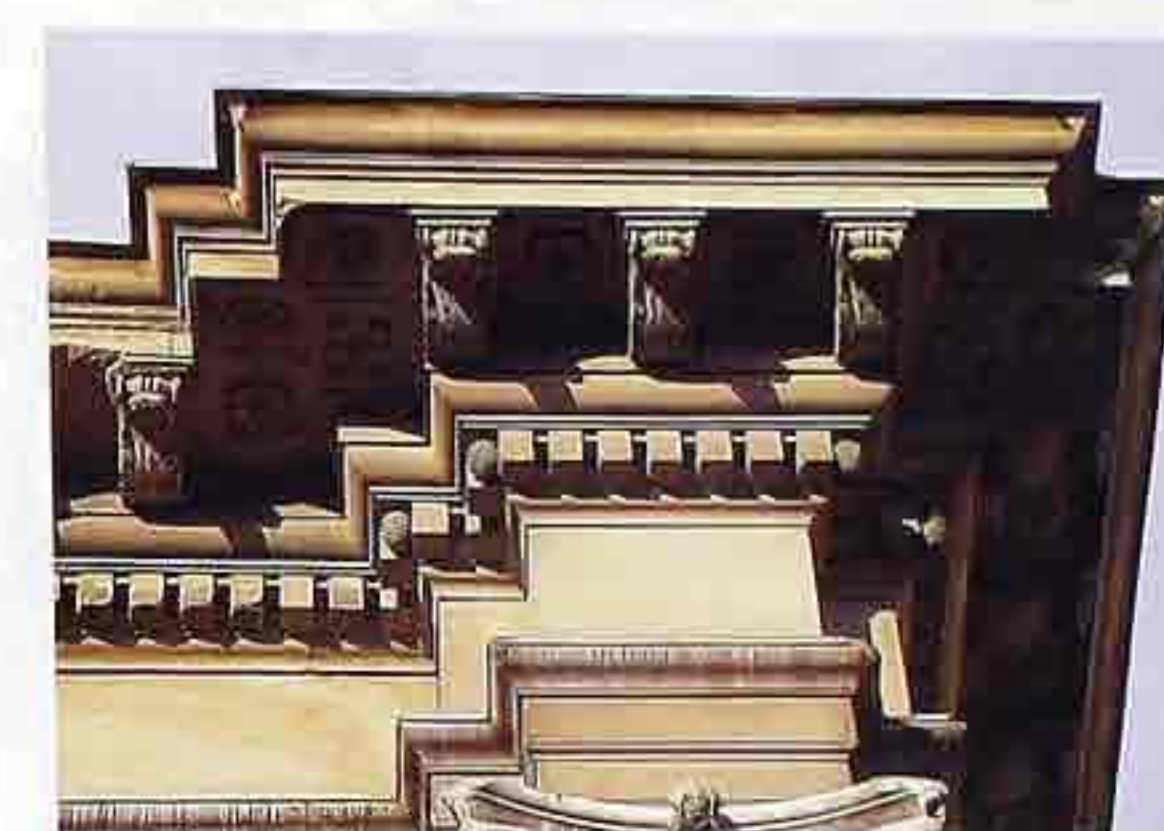
OM-93 Corner detail of Corinthian entablature: plain frieze and moldings; rosettes in coffers and in the soffit between the modillions
