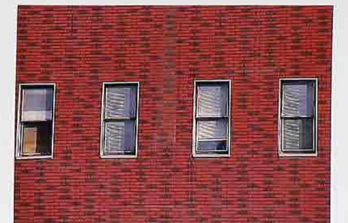
FA-58 Bituminous shingles in faux brick pattern
