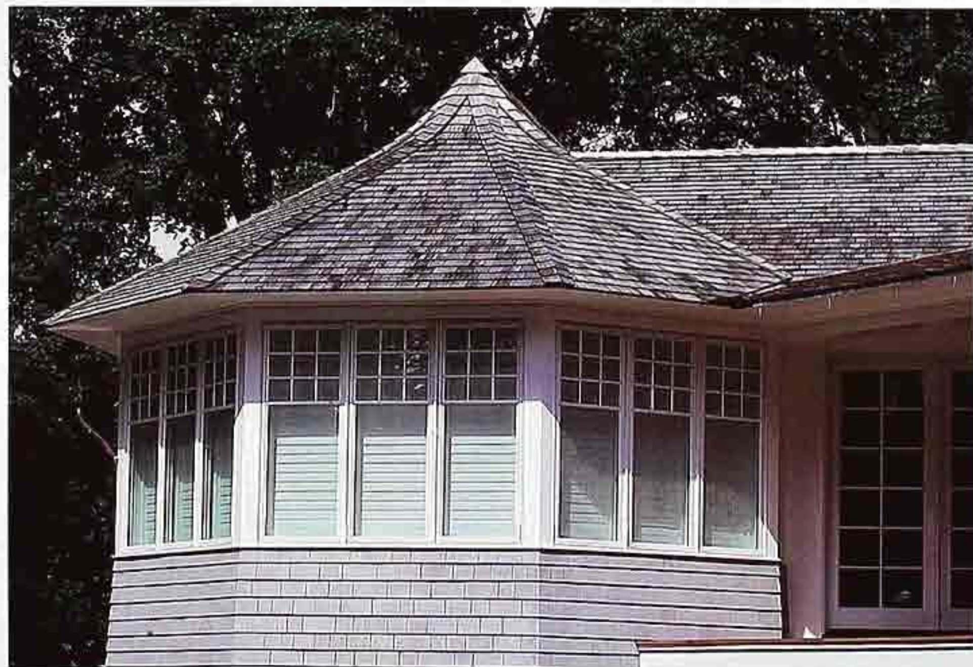
WI-82 Cant-sided bay with three windows per side, conical shingle roof, modern house
