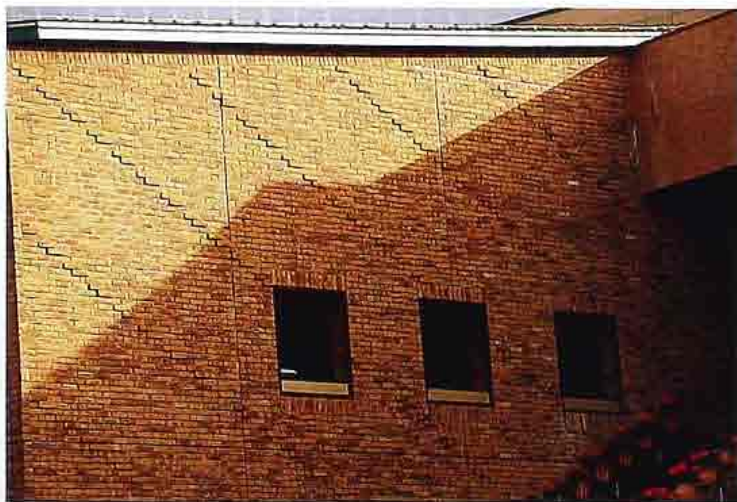
WA-206 Brick in random tones with projecting diagonal pattern and soldier courses above square windows, modern commercial building
