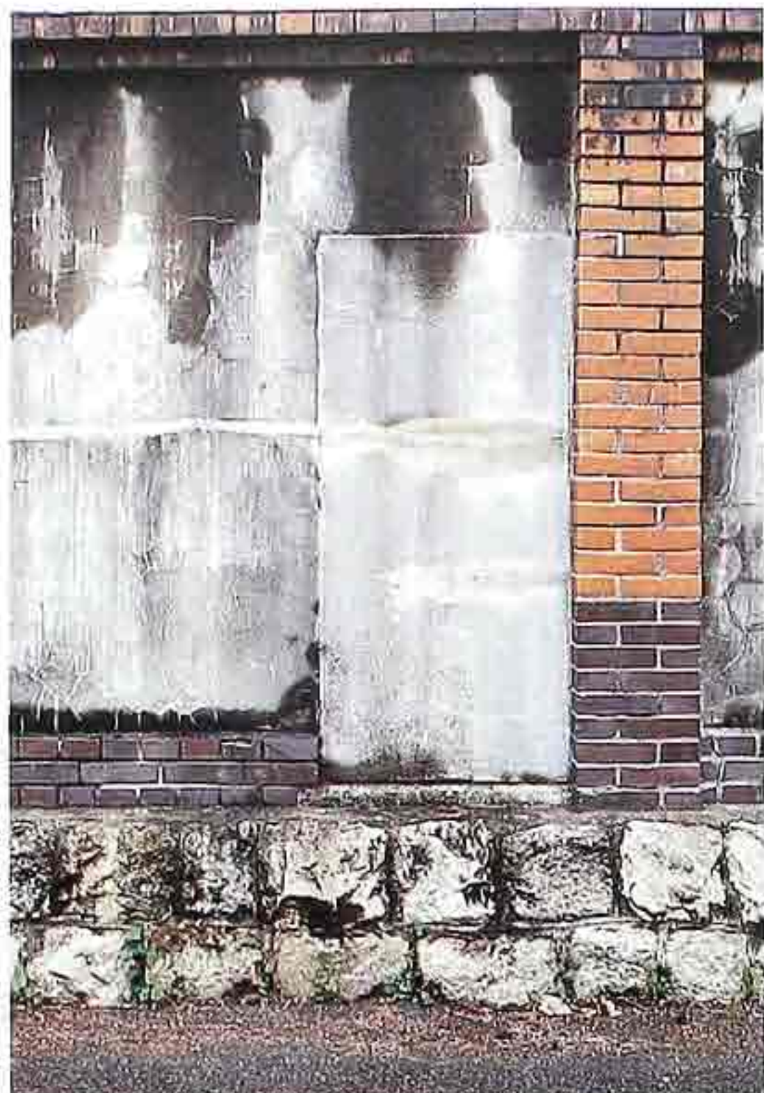
WA-264 Courtyard wall. Top to bottom: rowlock and header brick coping; cast concrete (left); running-bond brick pilaster; roughly squared fieldstone base
