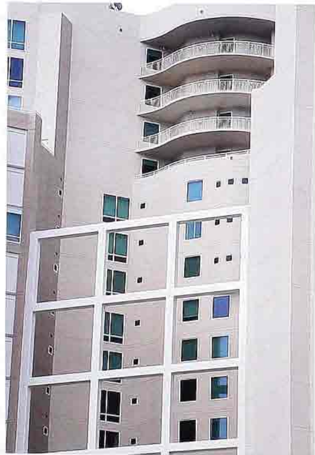
FA-130 Facade of simple punched windows, curvilinear balconies, and large-scale open grid, modern apartment house
