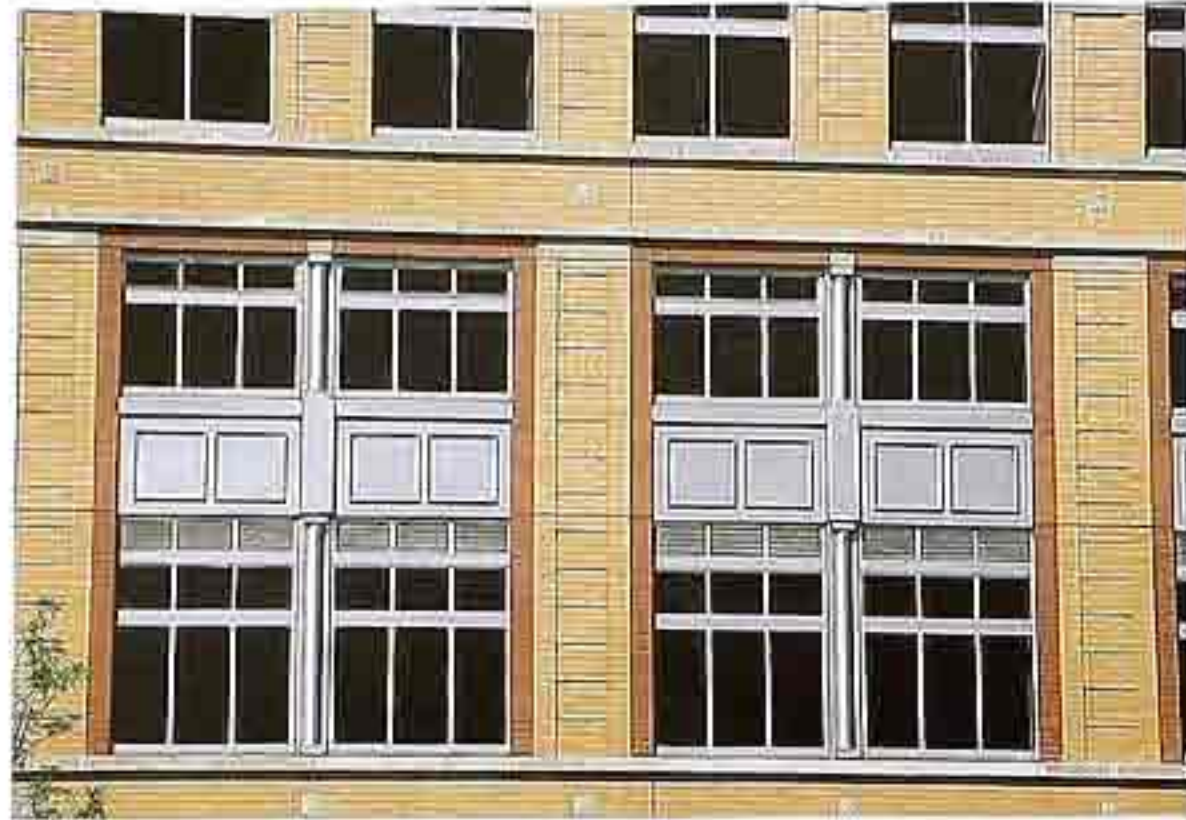
WI-158 Repetitive fenestration of three-mullion windows with raised panel spandrels, modern commercial building
