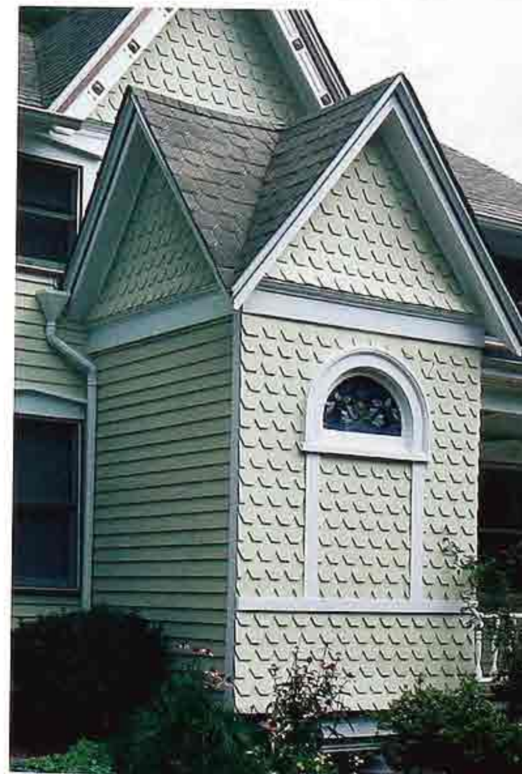
FA-45 Clapboard and sawn siding in fish-scale pattern with corner board, flat applied trim, and lunette window
