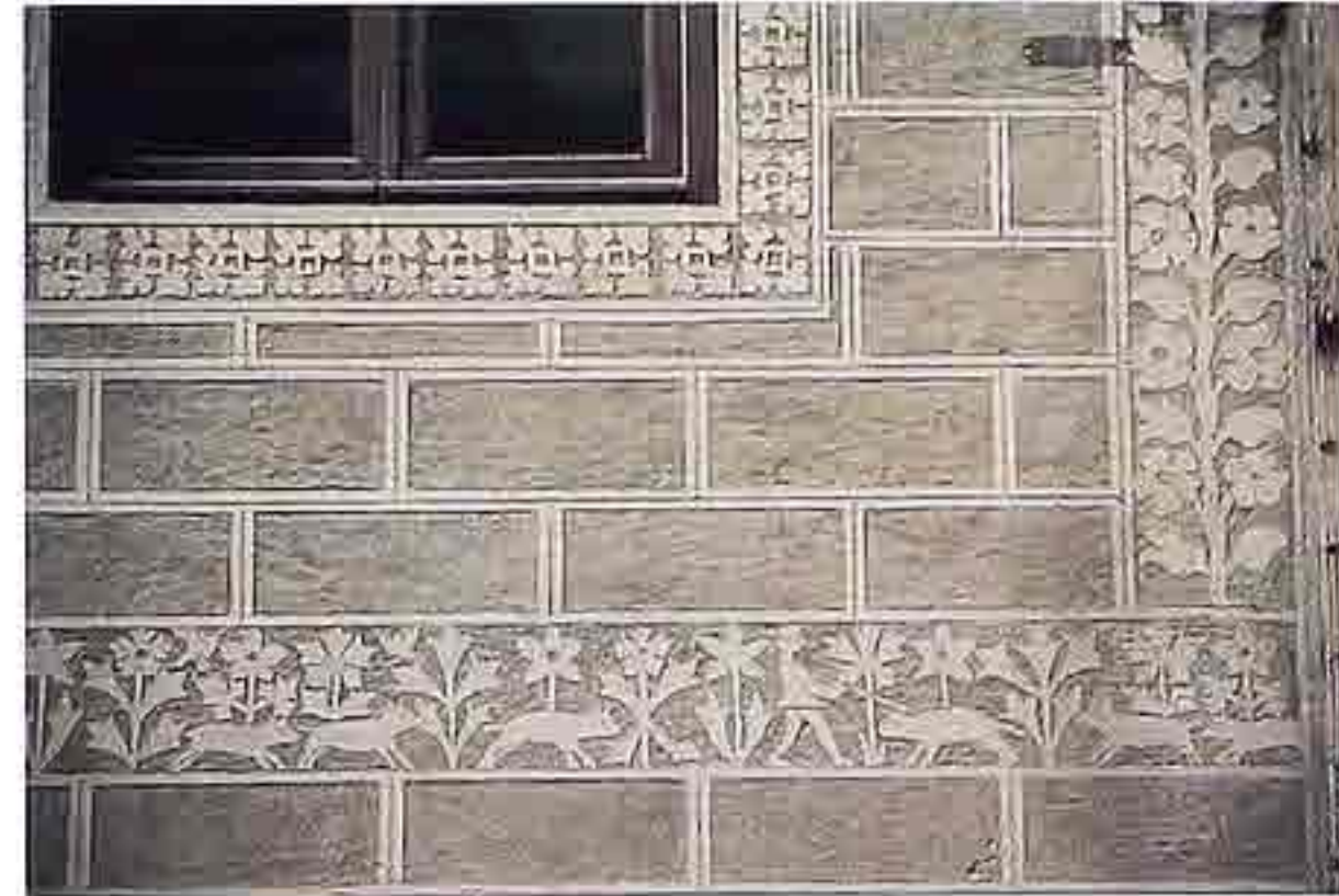
WA-239 Textured and inscribed stucco, foliated and pictorial designs mixed with imitation split-face stone in running bond
