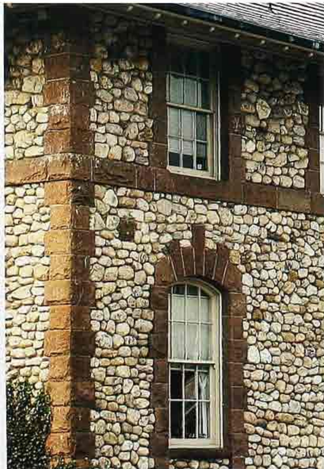
WA-108 Random rubble of cobbles with rusticated dimension-brownstone quoins, belt course, and voussoirs around arch window
