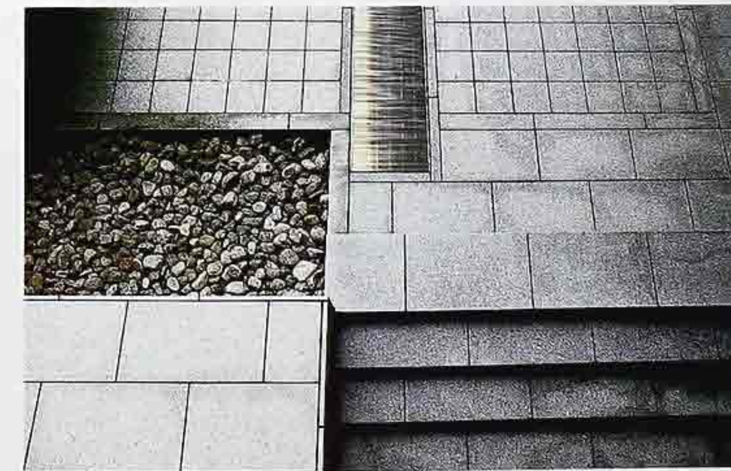
FP-27 Textured dimension paving stone with straight joints (top), and running bond (bottom), metal grates, and river rocks in courtyard of modern commercial building
