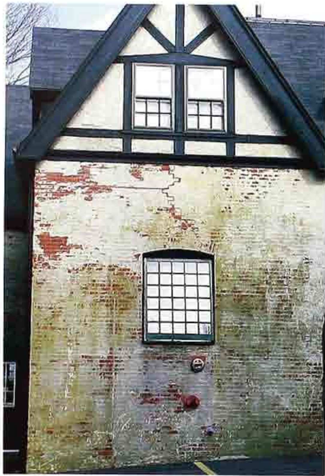
FA-92 Weathered painted stucco over exposed brick with half-timber gable above
