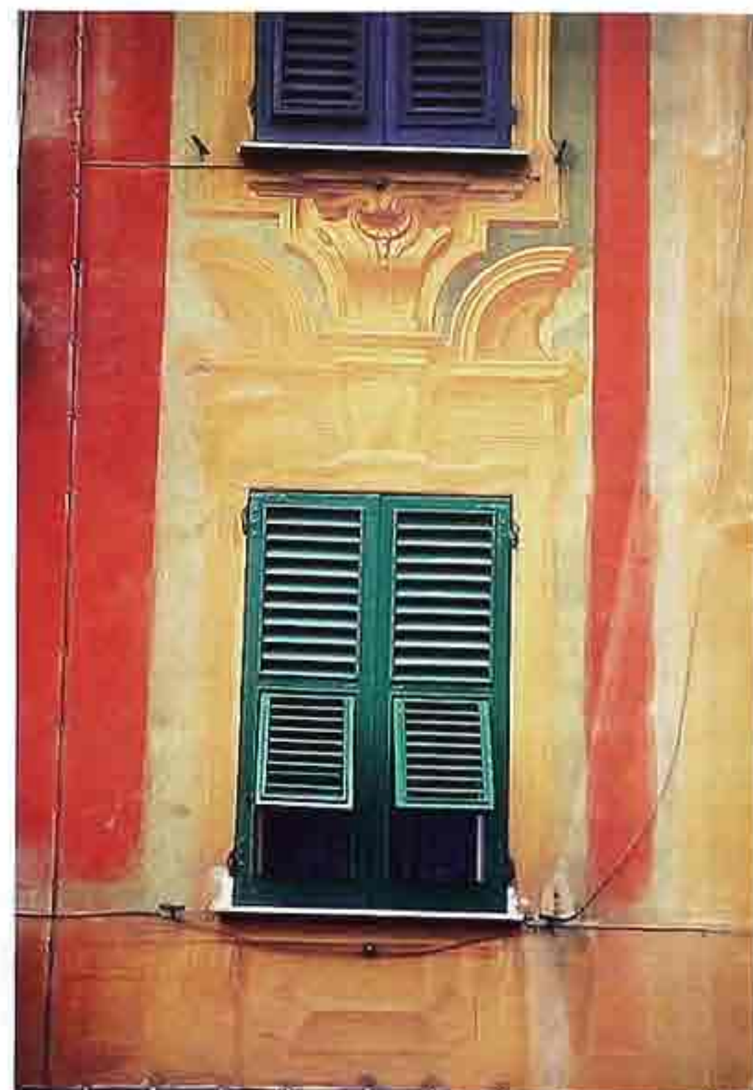
FA-83 Weathered trompe l'oeil moldings and pediment around shuttered windows on Tuscan wall
