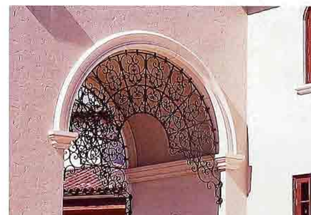
CP-143 Semicircular arch in stucco wall with molded impost blocks, archivolt, and inset wrought-iron tracery
