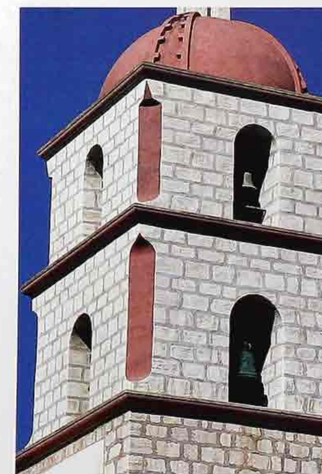
FA-91 Trompe l'oeil stucco simulating adjacent masonry on belfry, dome with chamfered corners, 19th-c. mission
