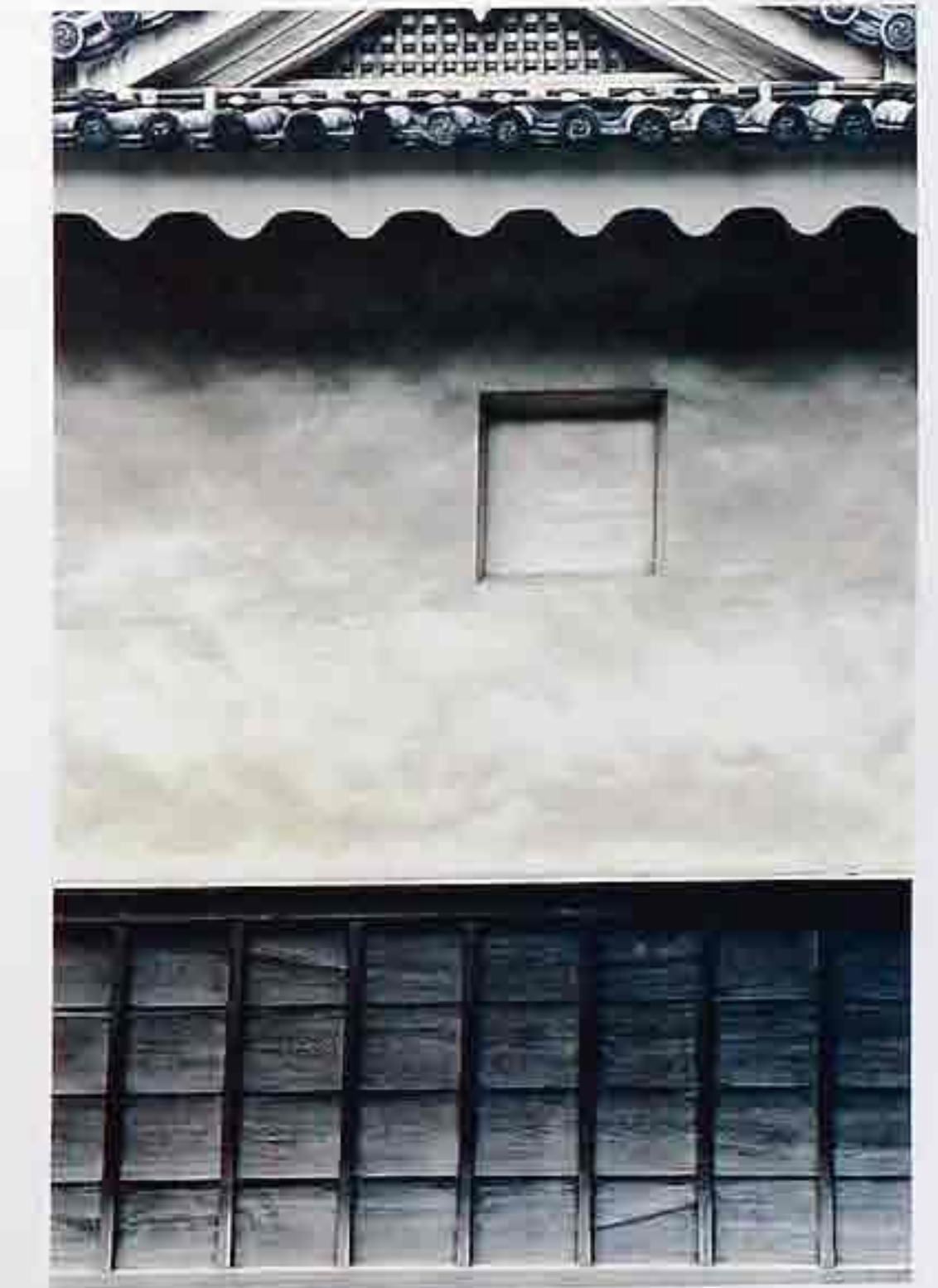
WA-281 Timber frame with infill of undulating stucco and framed planks, traditional Japanese building
