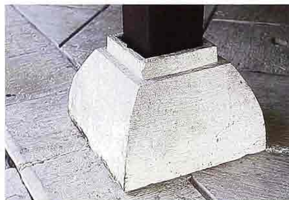
CP-52 Timber post on a square chamfered stone base
