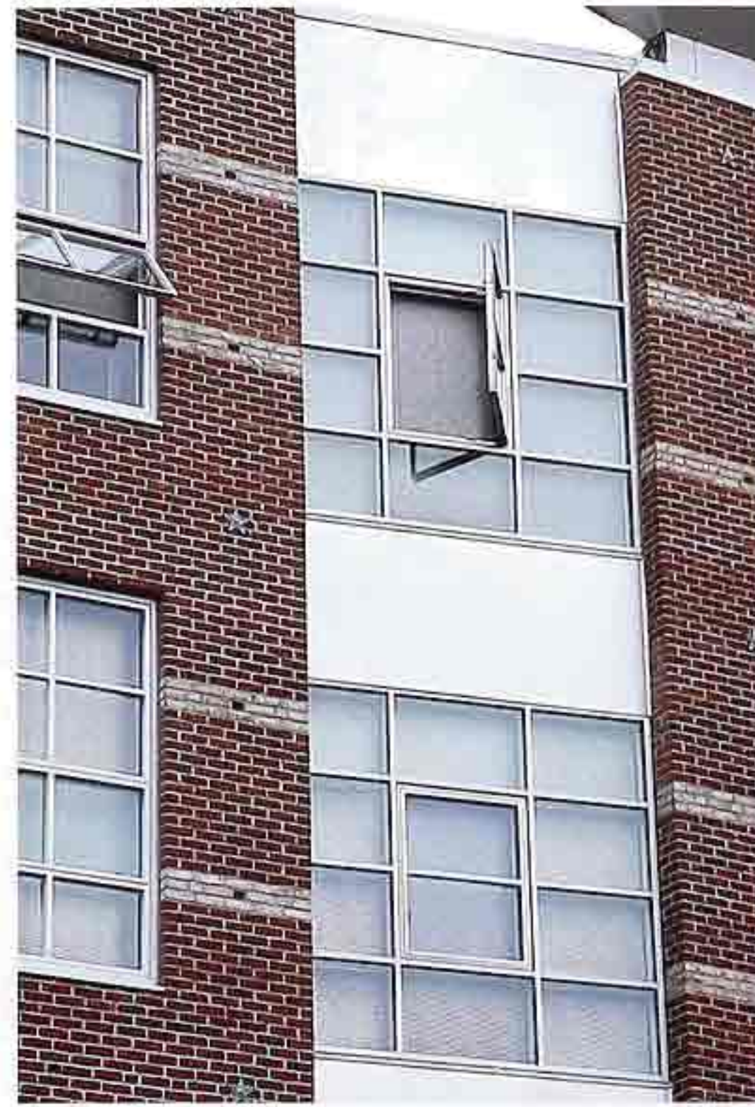
WI-39 Casement windows (center) and awning window (left) set in fixed lights; extruded aluminum mullions, modern apartment house
