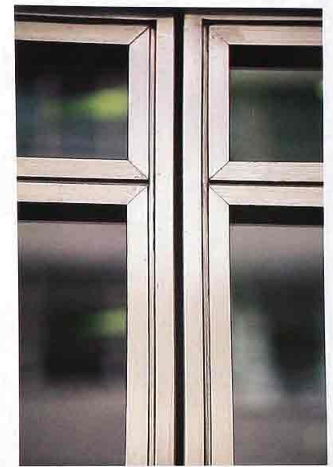
WI-6 Fixed window with stainless steel muntins and mullions, modern commercial building
