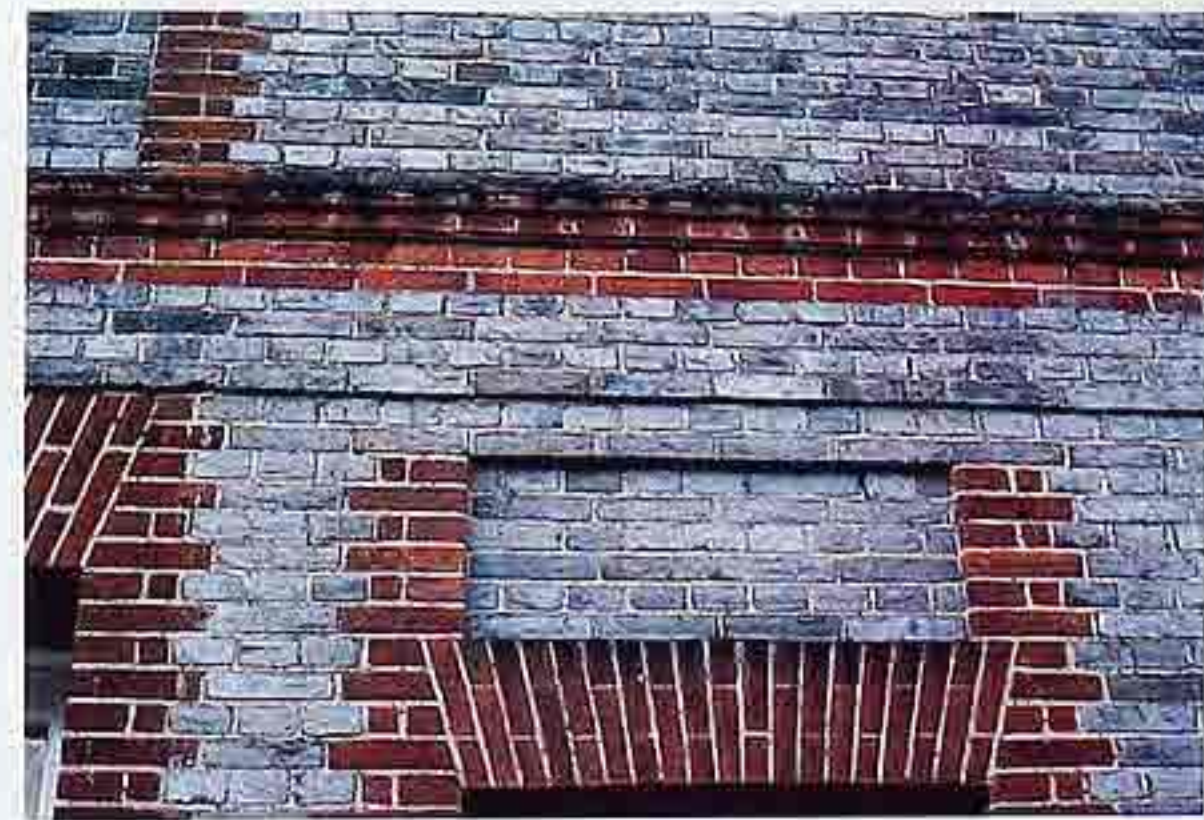
WA-173 Jack-arch window and dog-tooth course of contrasting brick in English bond wall with recessed panel
