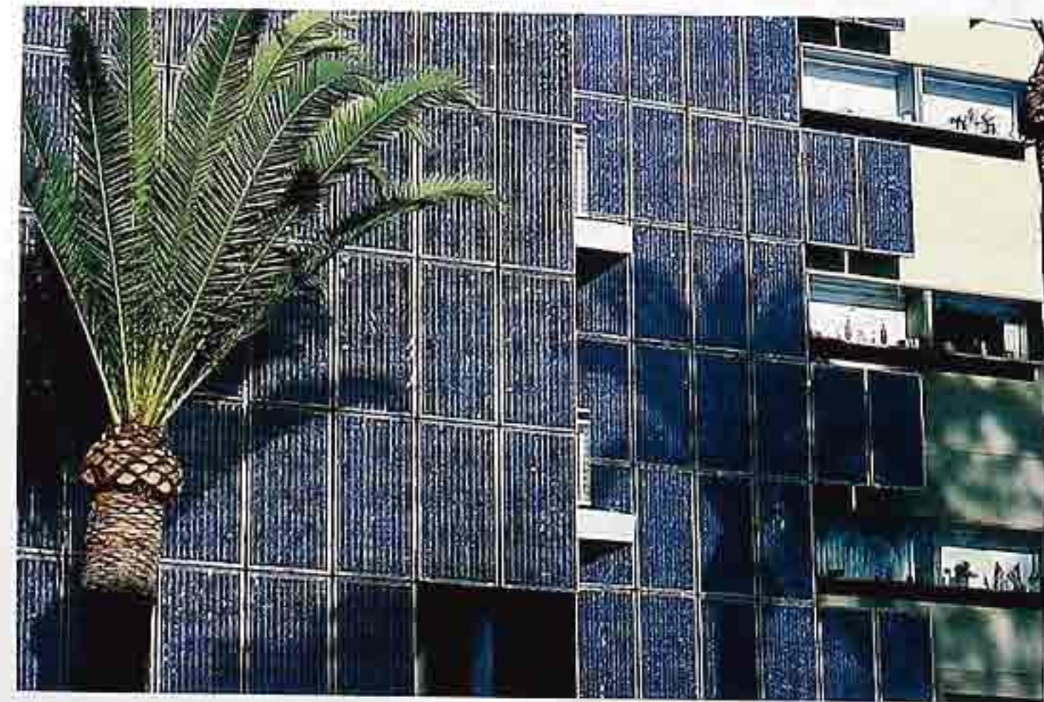
FA-42 Photovoltaic-panel cladding, modern commercial building
