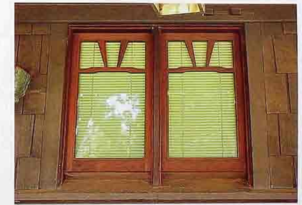
WI-28 Wood-framed awning windows with shaped wood muntins, Arts and Crafts house
