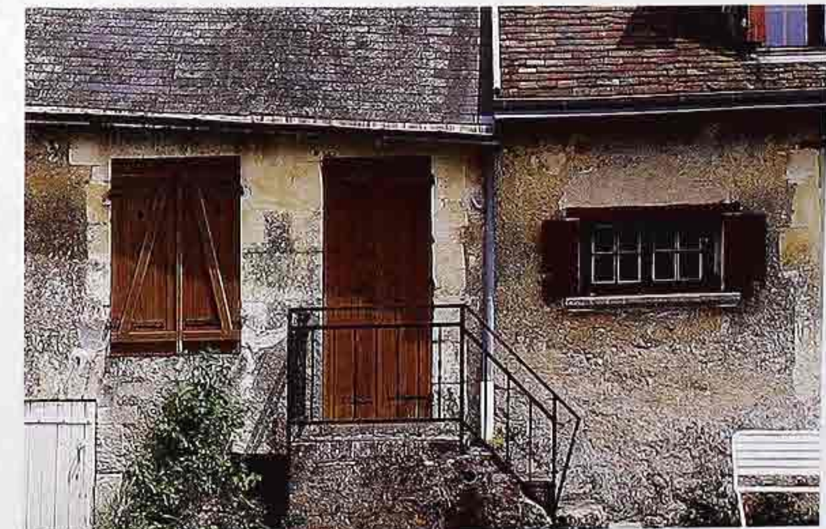
WI-193 Batted shutters and door
