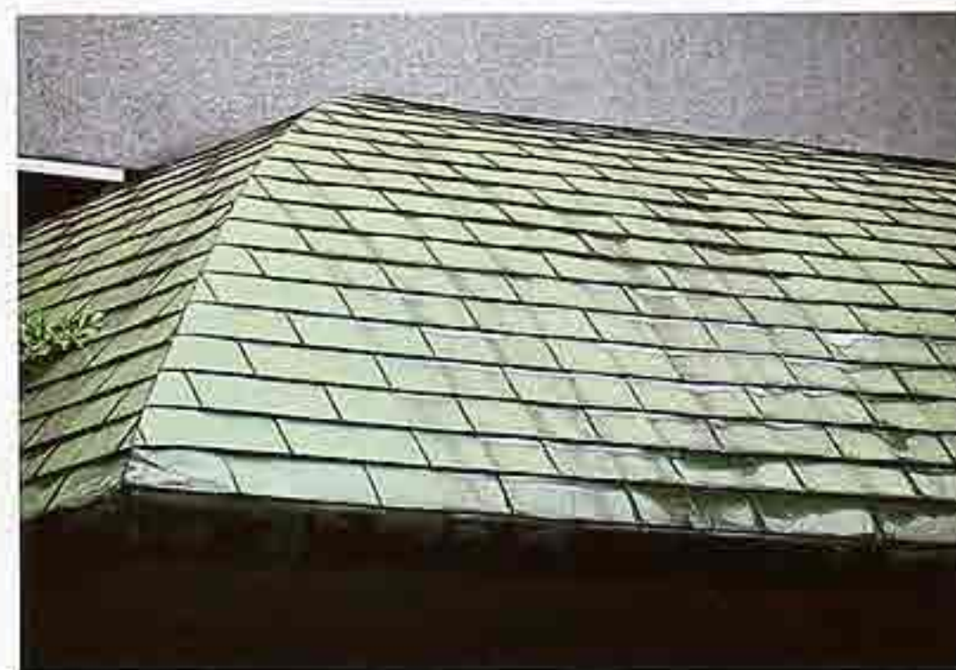
CR-23 Copper shingles on curved hipped roof
