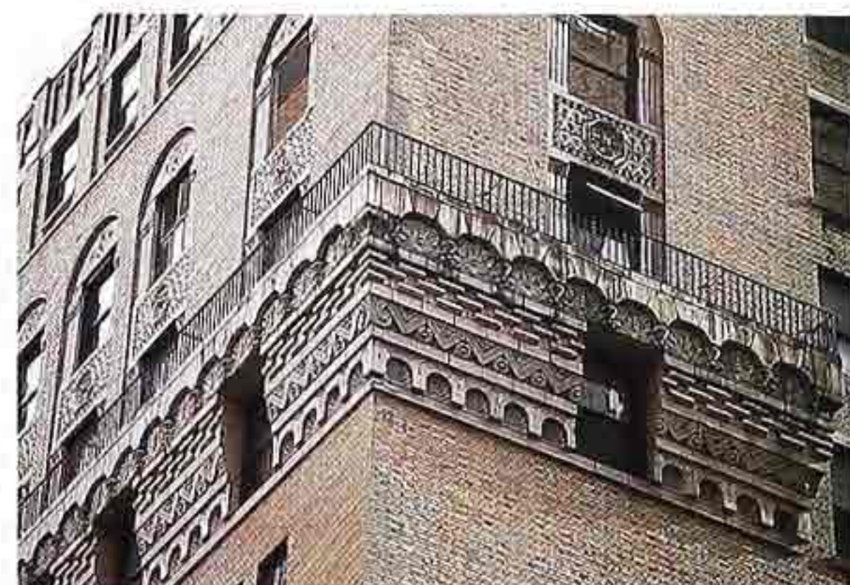
OM-87 Ornamented corbelled courses. Top to bottom: Gothic cornice, three rows of biliet molding, zigzag band, Gothic cornice
