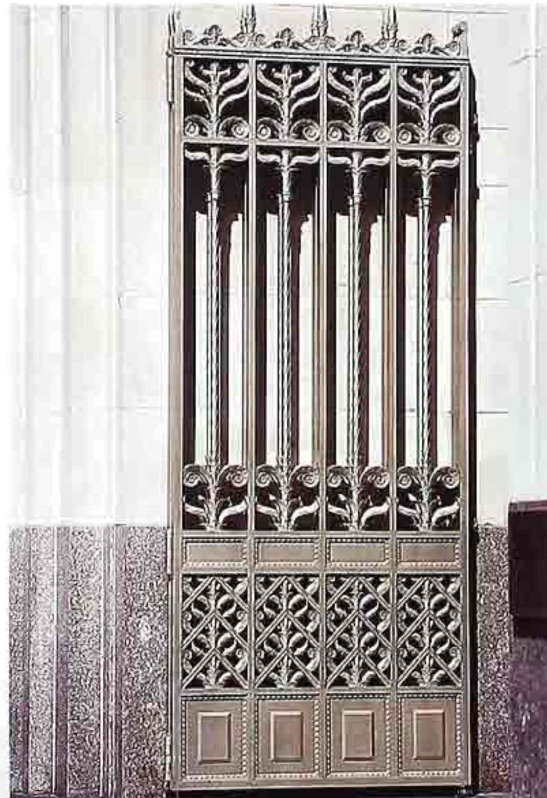
DW-117 Cast-bronze gate coated with sealant to prevent patination, commercial building
