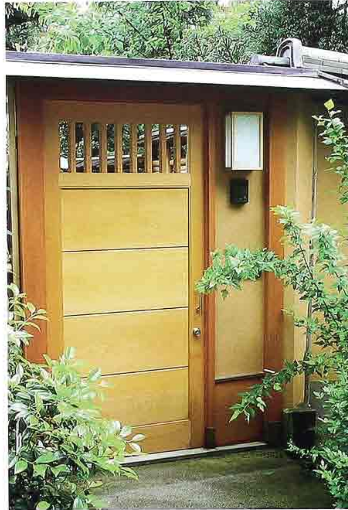
DW-95 Courtyard entry to modern house: door hood over natural wood paneled door with wood grille
