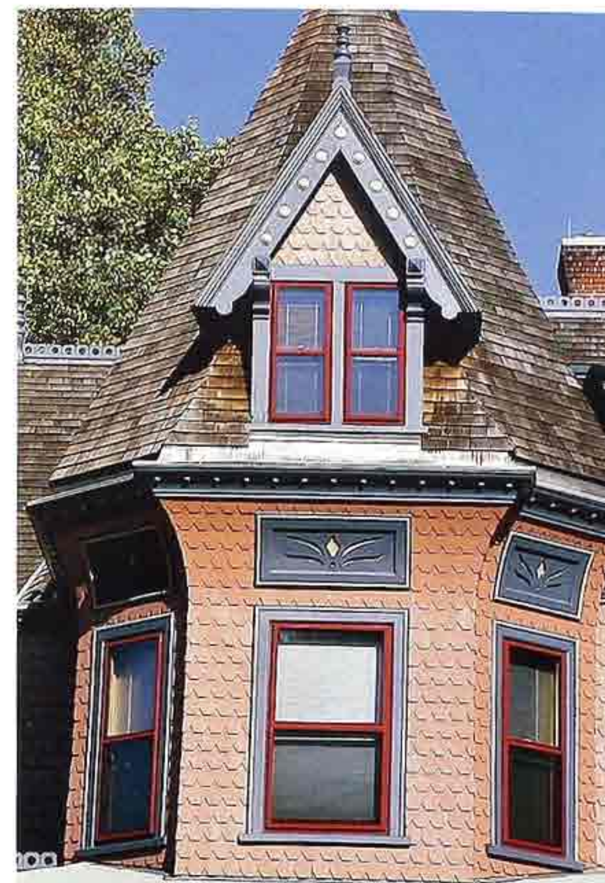
FA-79 Polychrome house with octagonal turret, steep gable dormer, prominent bargeboards, fish-scale cut siding, and modillion cornice, 19th-c.
