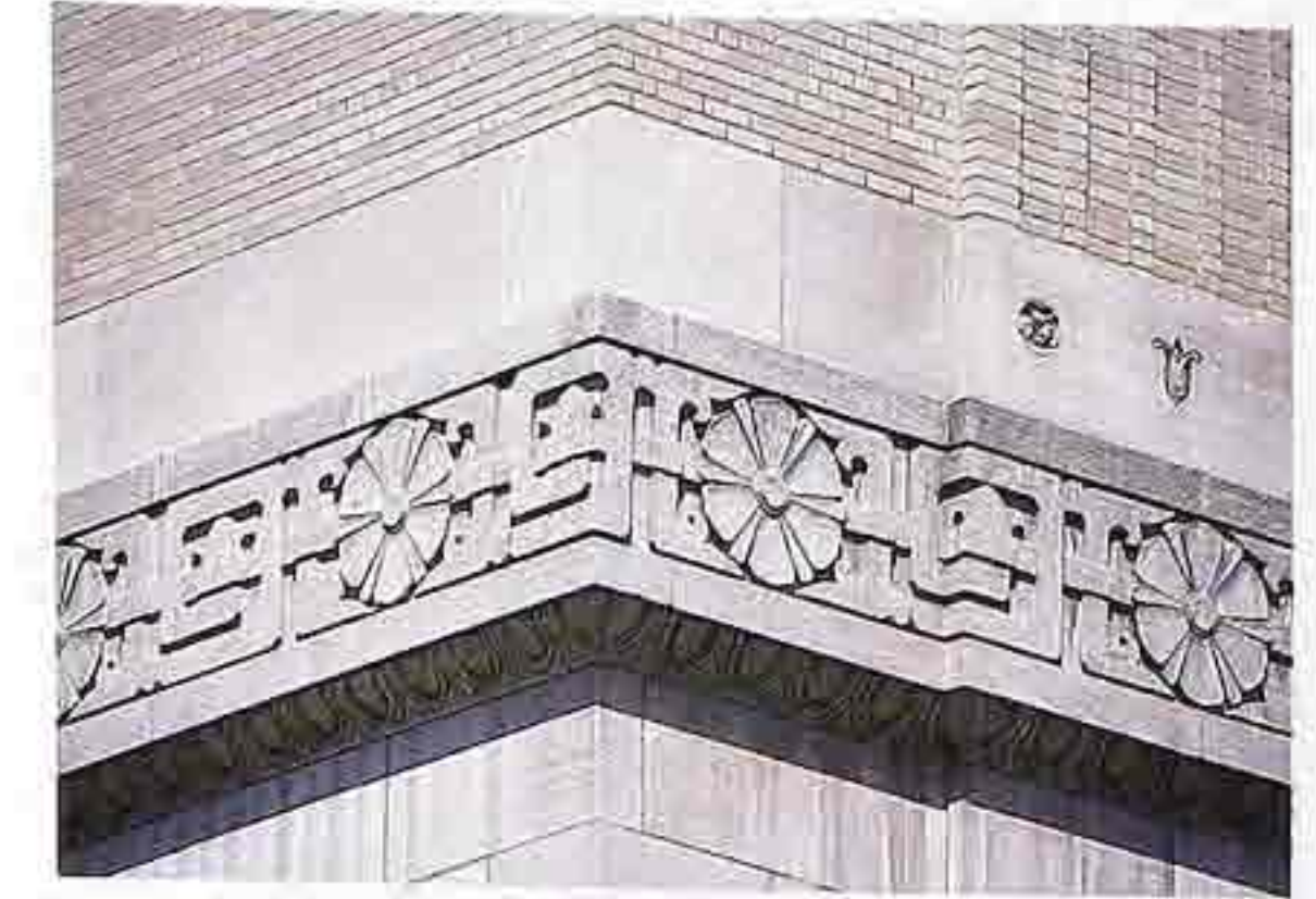
OM-34 Ornamental band with rosettes in a Greek-key motif, over egg-and-dart molding
