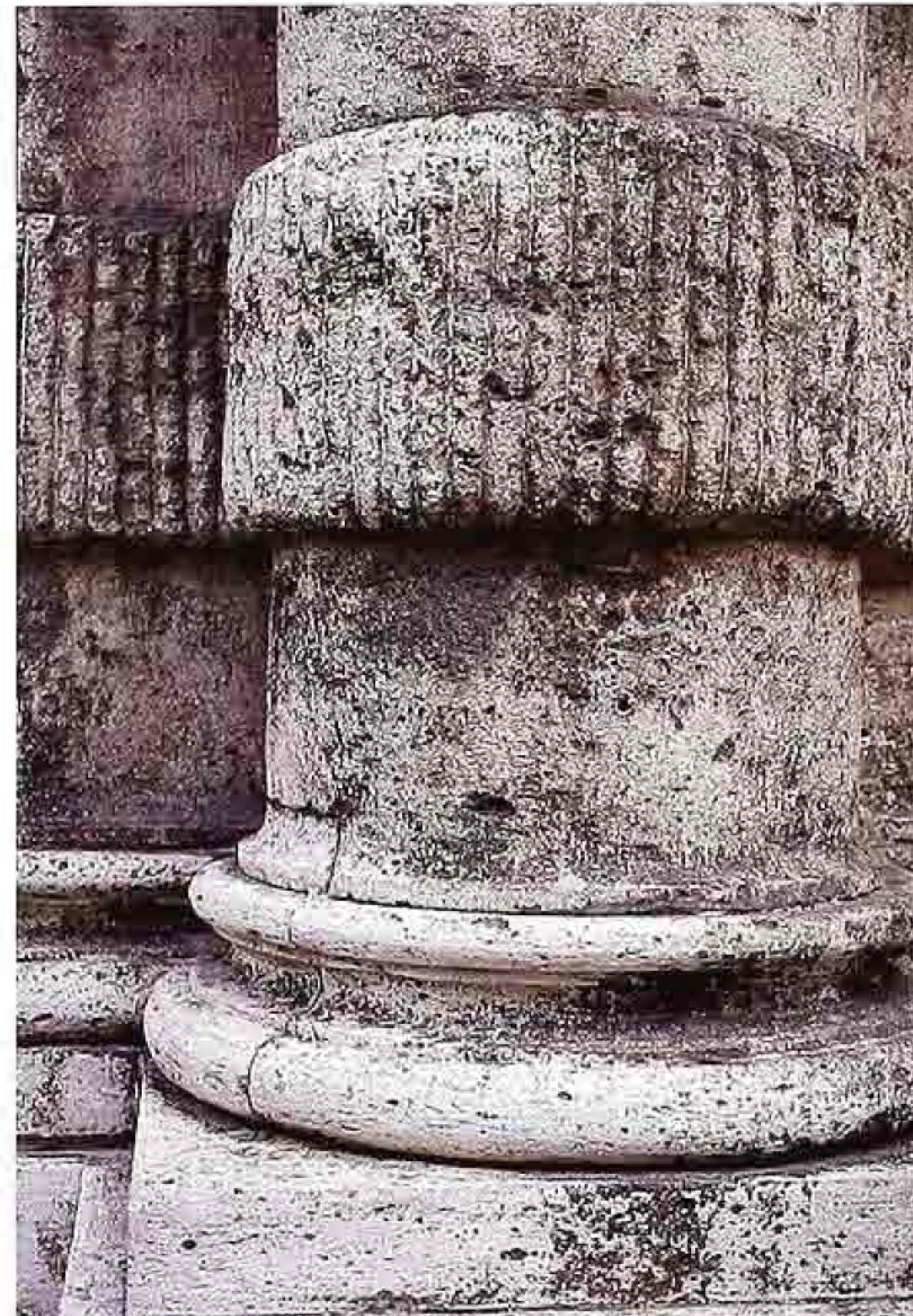
CP-32 Attic base of weathered column in volcanic stone with banded rusticated shaft
