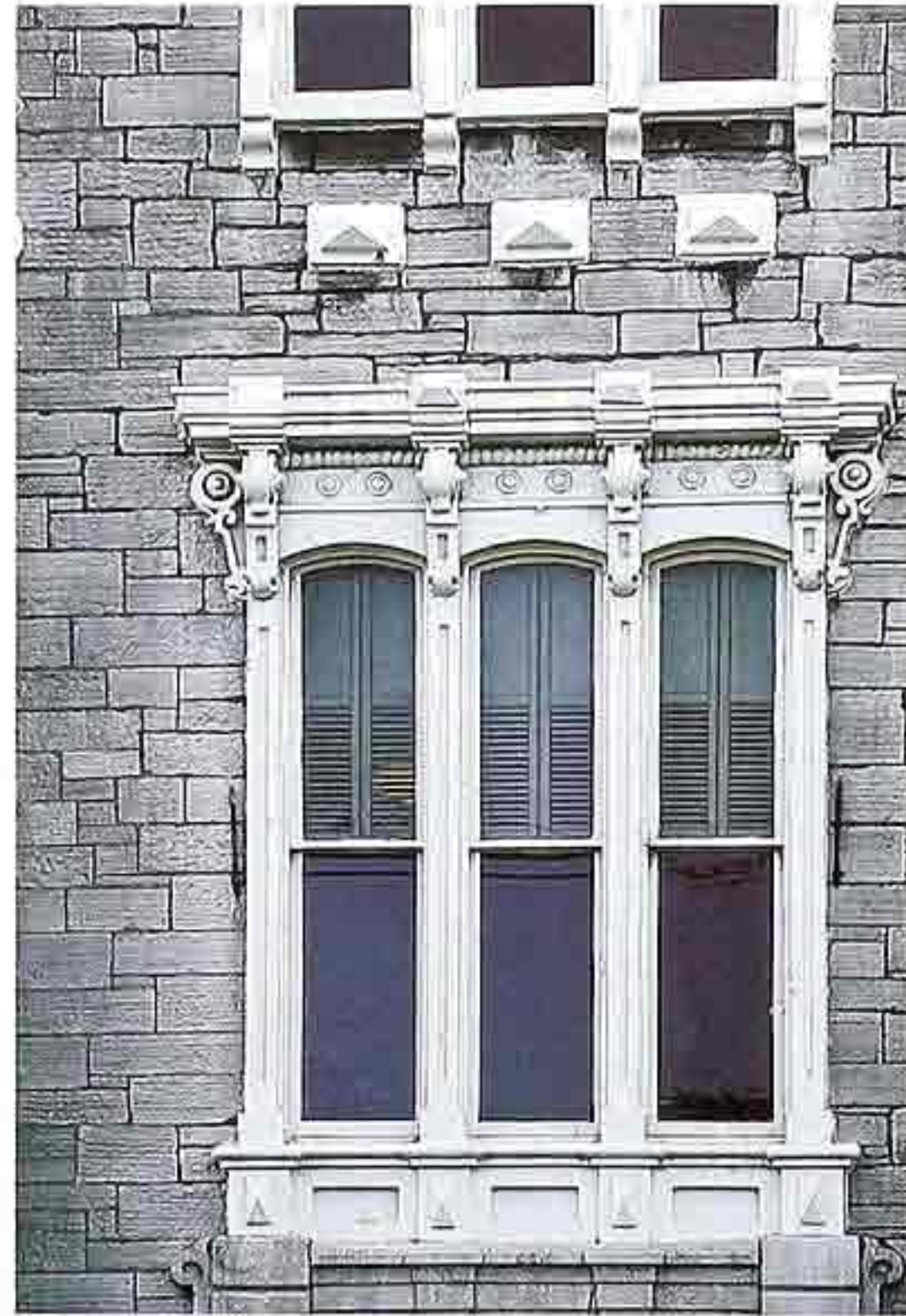
WI-112 Ornament and molding around group of three double-hung windows; consoles supporting cornice, 19th-c. American stone commercial building
