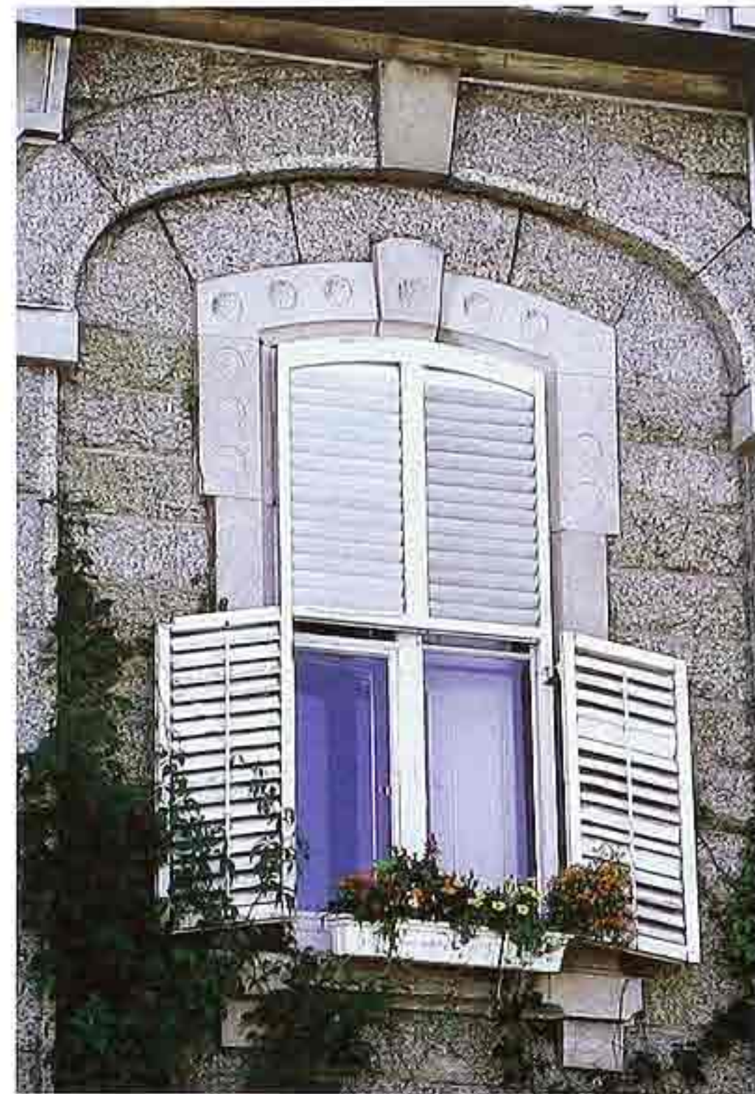
WI-184 Louvered shutters with fixed top shutters
