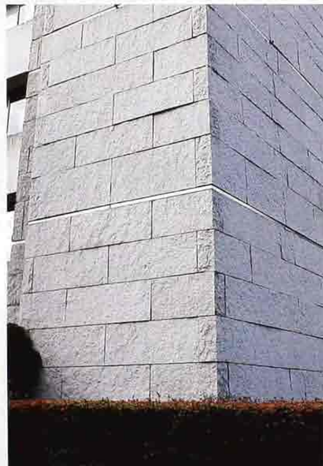
WA-133 Corner of split-face granite in shelf, running bond with metal banding, modern commercial building
