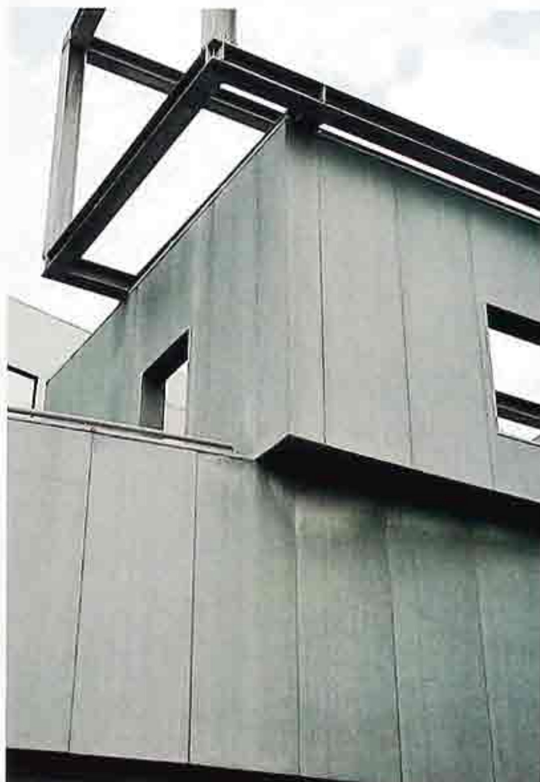
FA-22 Flush galvanized panels, modern commercial building
