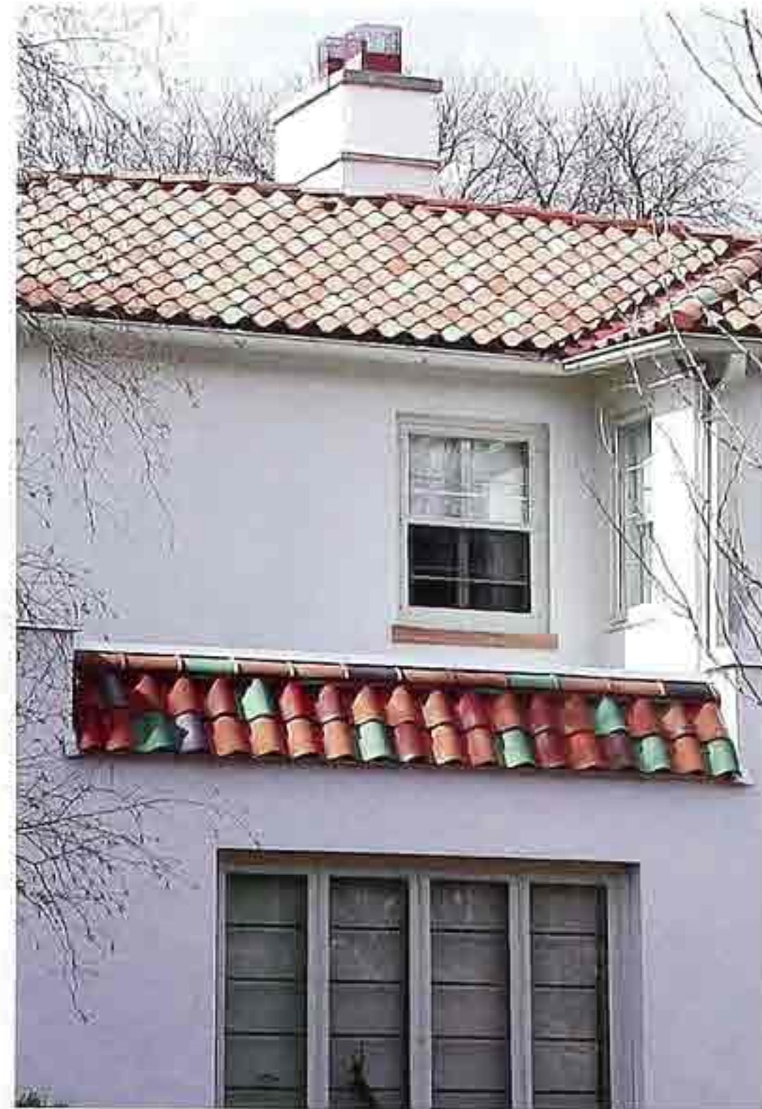
CR-55 Multicolored mission tiles on hipped roof with shed roof over window, 20th-c. American house
