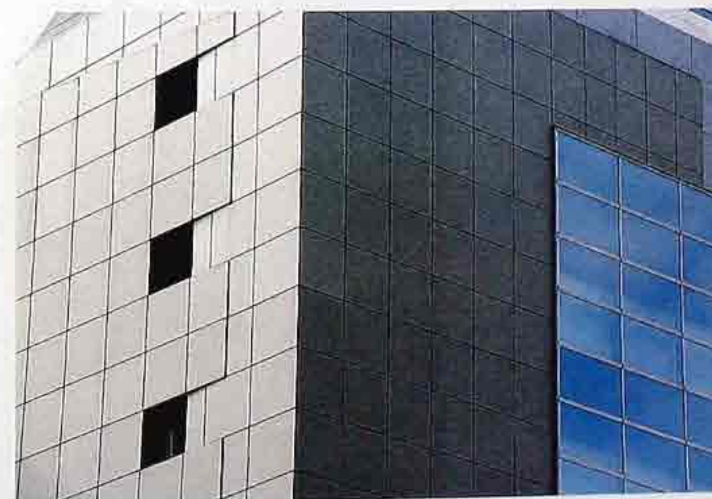
WA-137 Honed-granite veneer in stack bond with raised pattern around windows, modern commercial building
