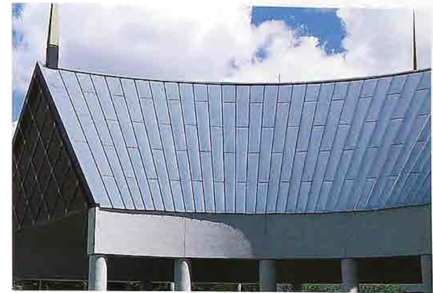
CR-27 Anodized aluminum or coated sheet steel with standing seams, curved gable roof, modern commercial building
