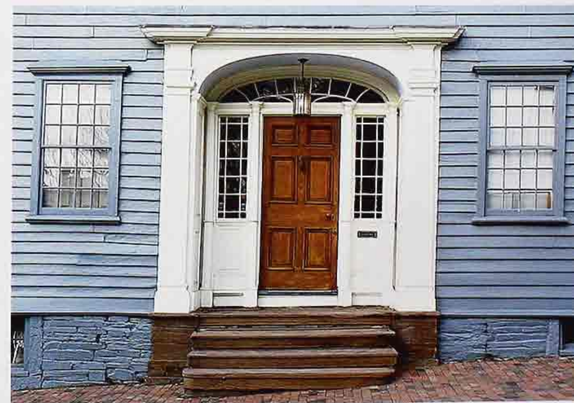
DW-86 Arched entry with crown molding and pilasters around paneled door, side lights, and fanlight, 18th-c. American house
