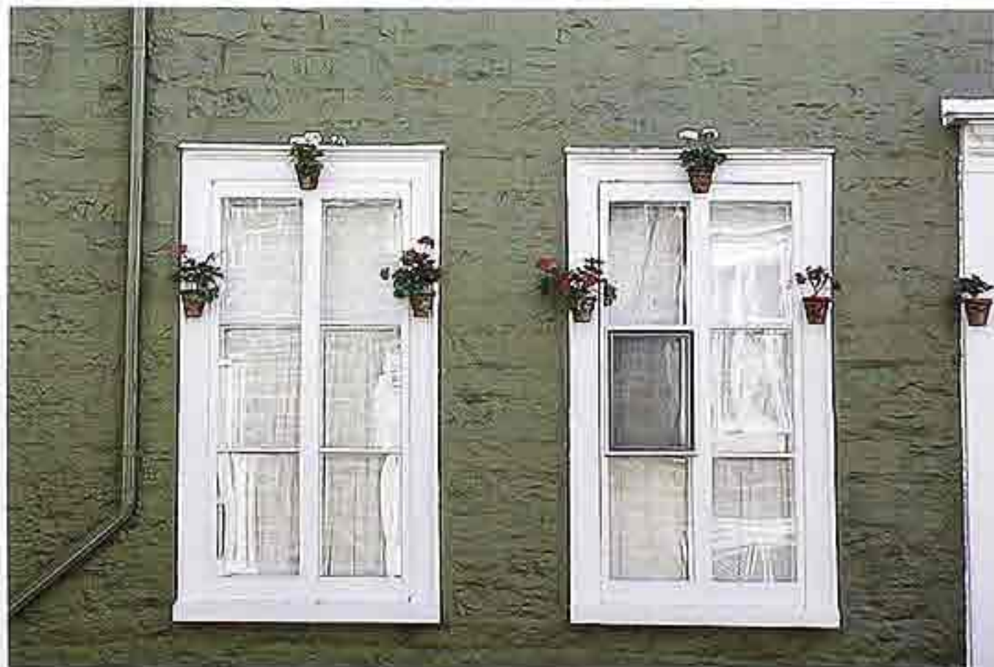
WI-106 Flat wood casing around double-casement windows
