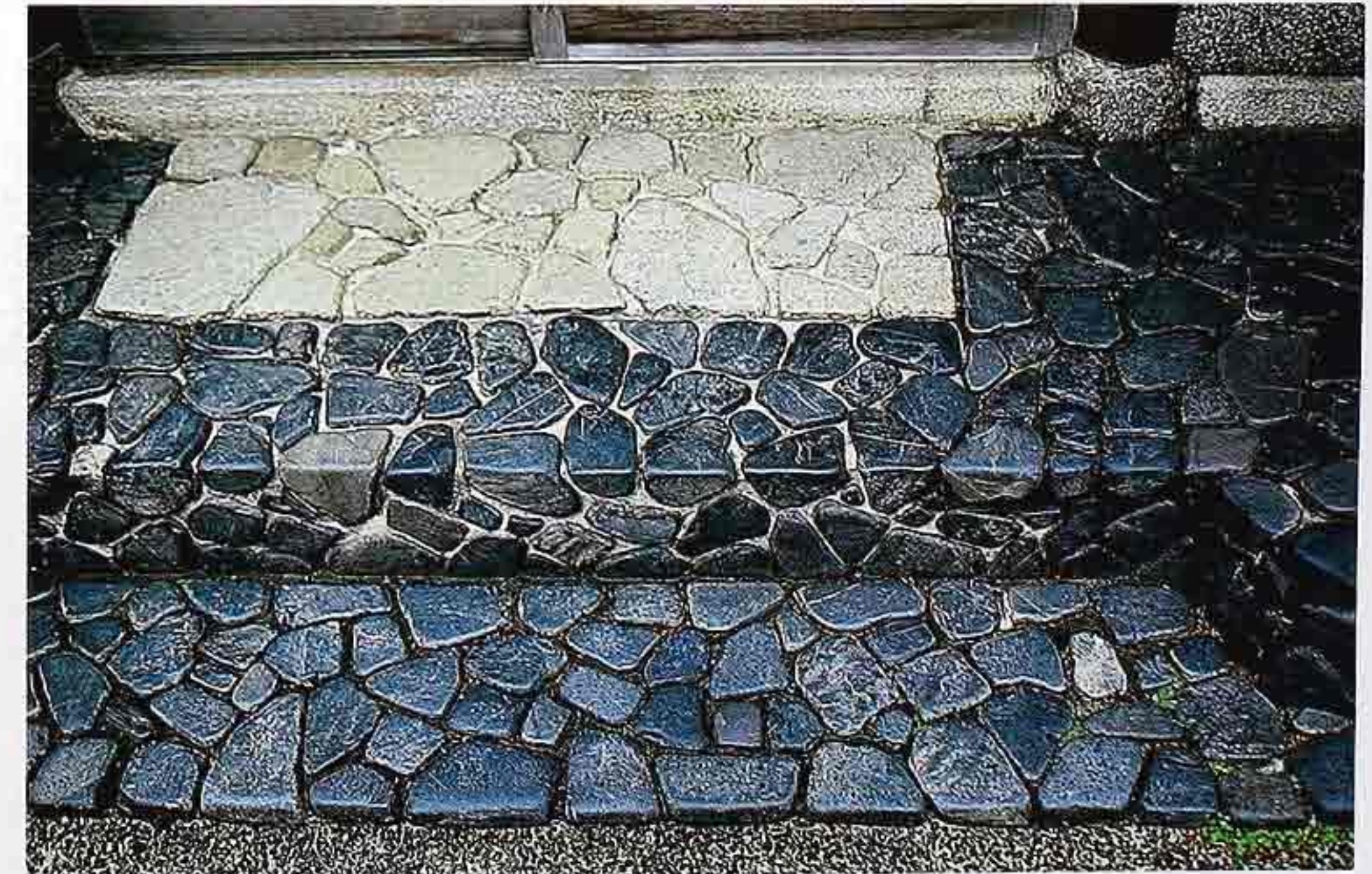
FP-42 Small, split, polished fieldstones set in concrete and bordering light-colored flagstone, forming steps
