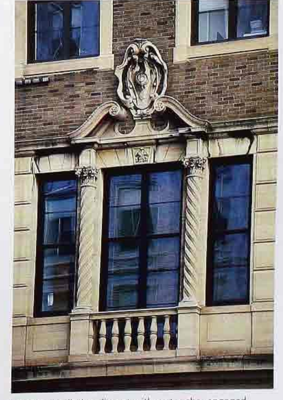
WI-139 Scrolled pediment with cartouche, engaged columns, and balustrade below window with side lights, apartment house
