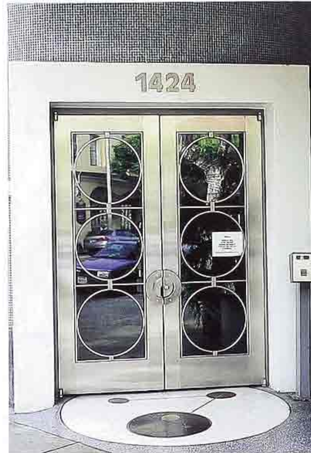
DW-46 Stainless steel double doors with full glass in circular muntins or grille
