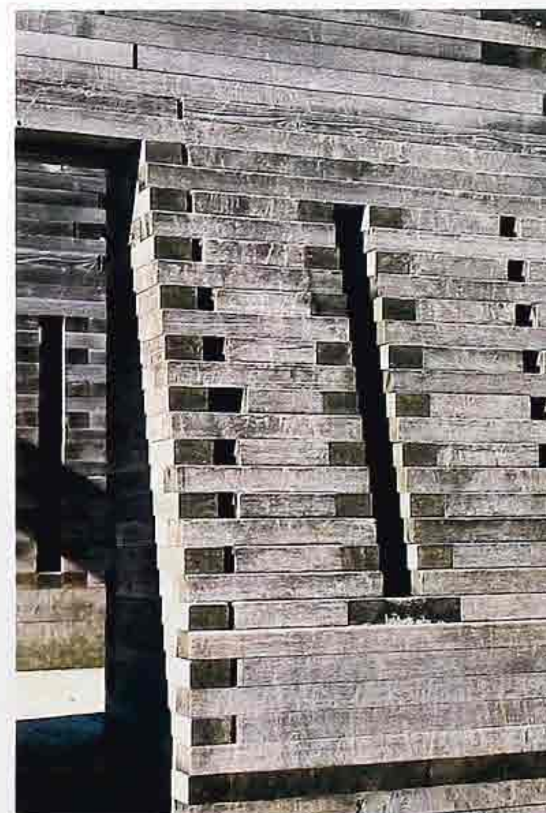
WA-49 Fortification-style battered wall with lapped-joint corners
