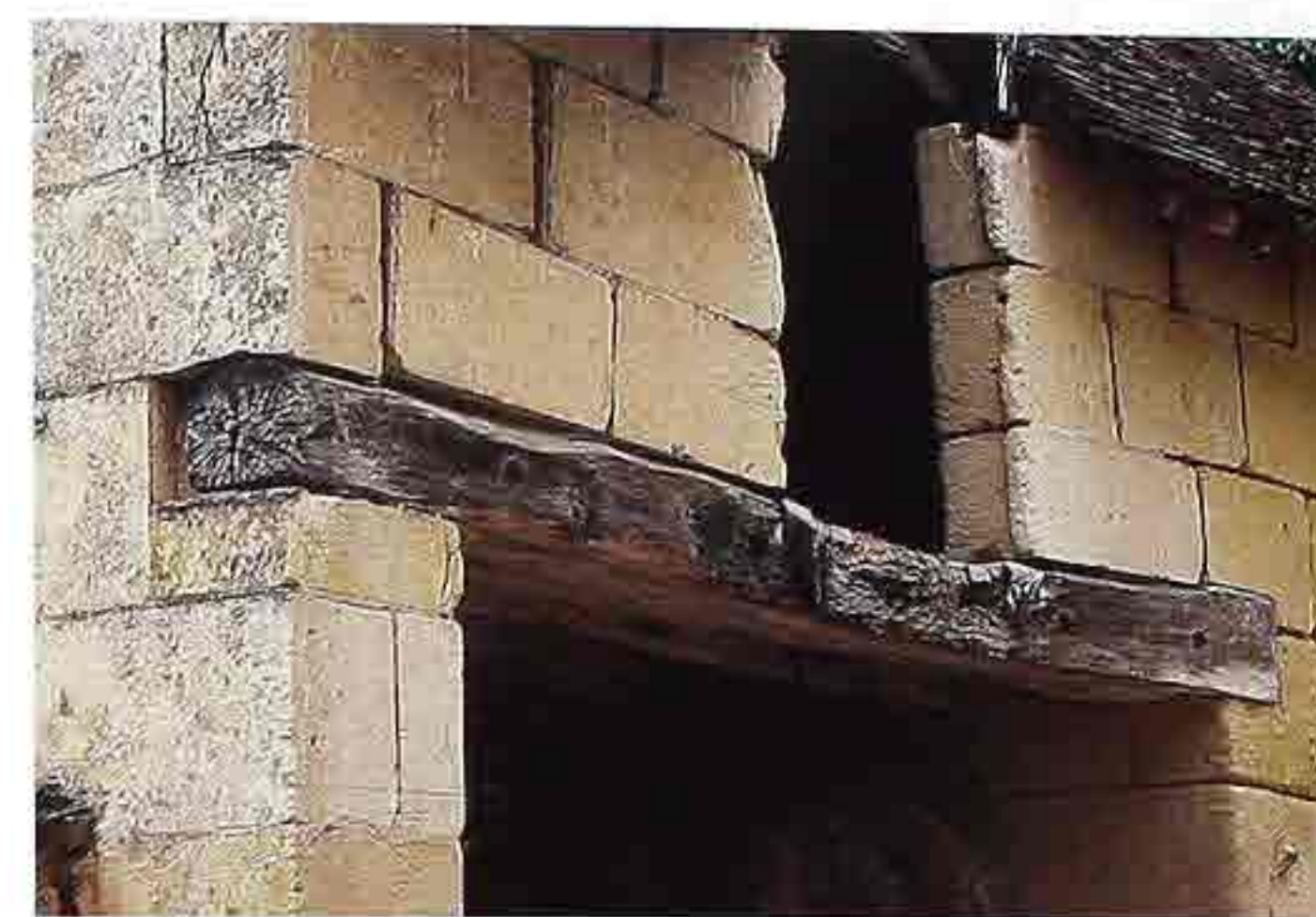
CP-109 Timber lintel in stone wall
