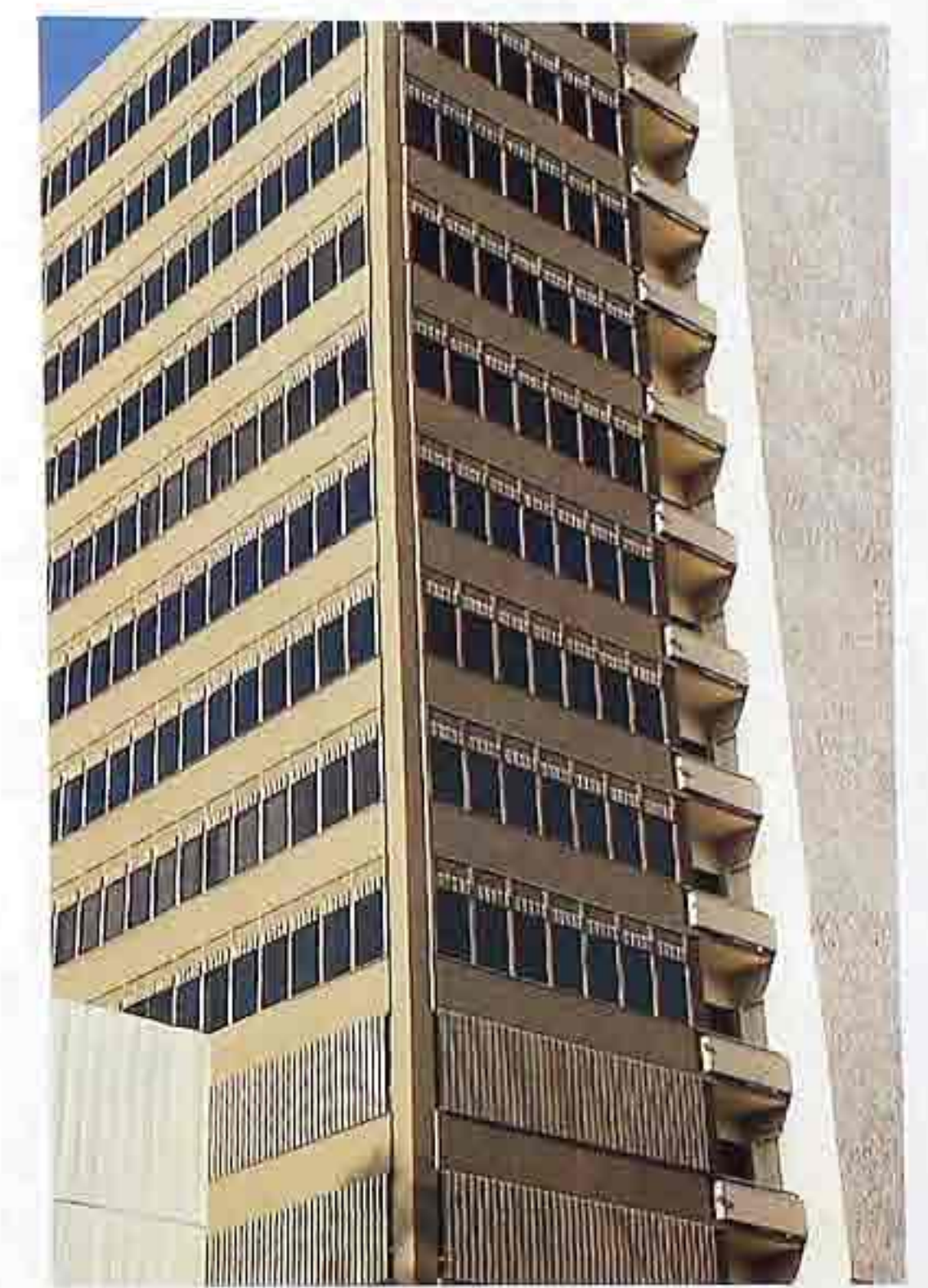
WA-303 Concrete building with metal trim
