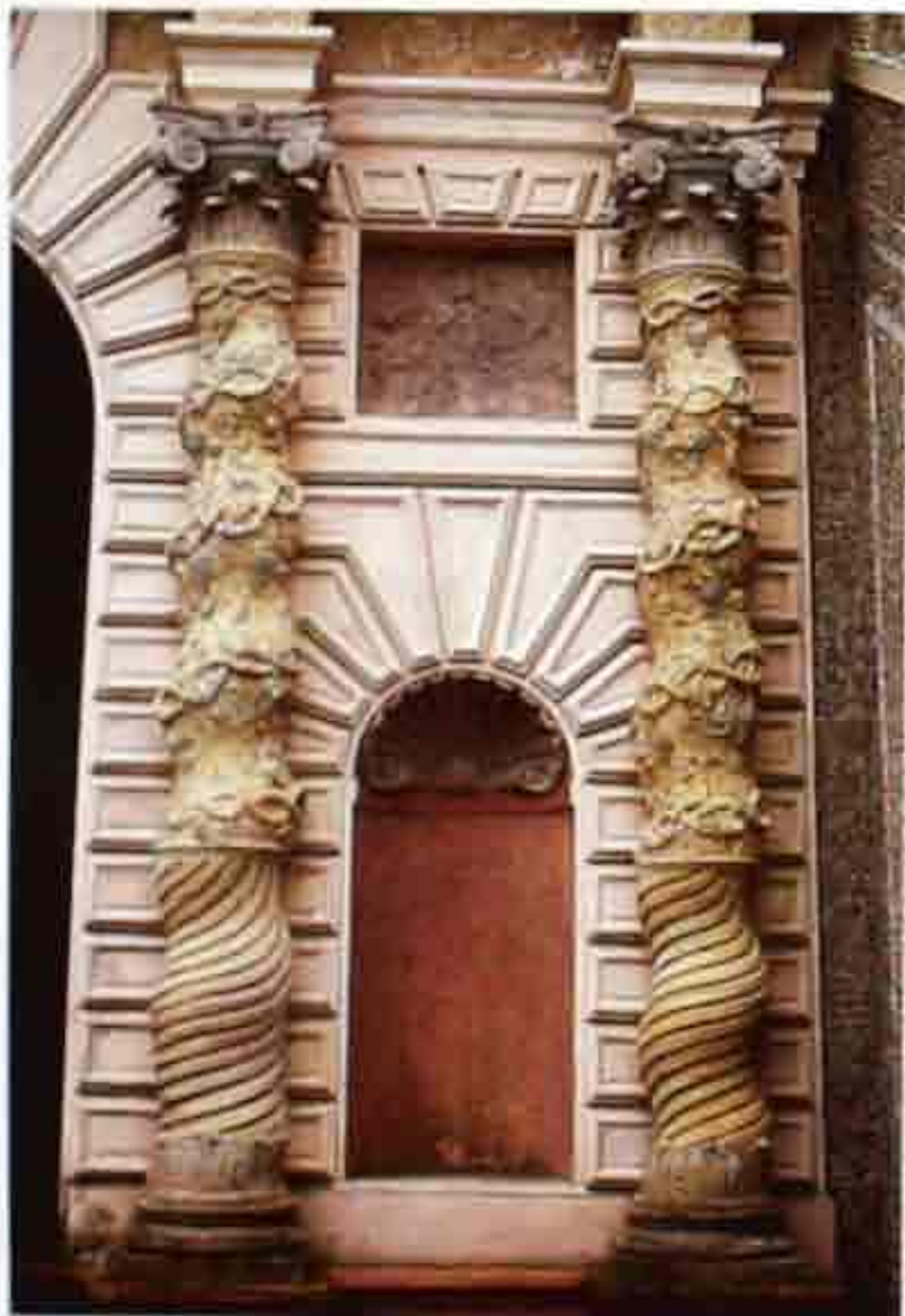
CP-67 Stone entryway with partially fluted Salomonic columns, garland ornament, and Composite capitals
