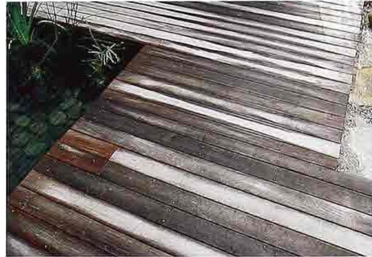
FP-11 Wood deck around reflecting pool (at left)
