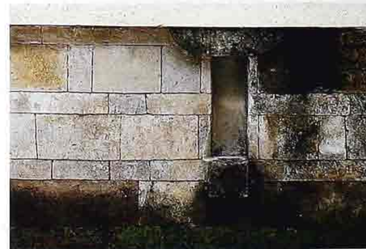
WA-80 Stone in coursed ashlar with bracket, niche, and perpendicular under niche, Bali
