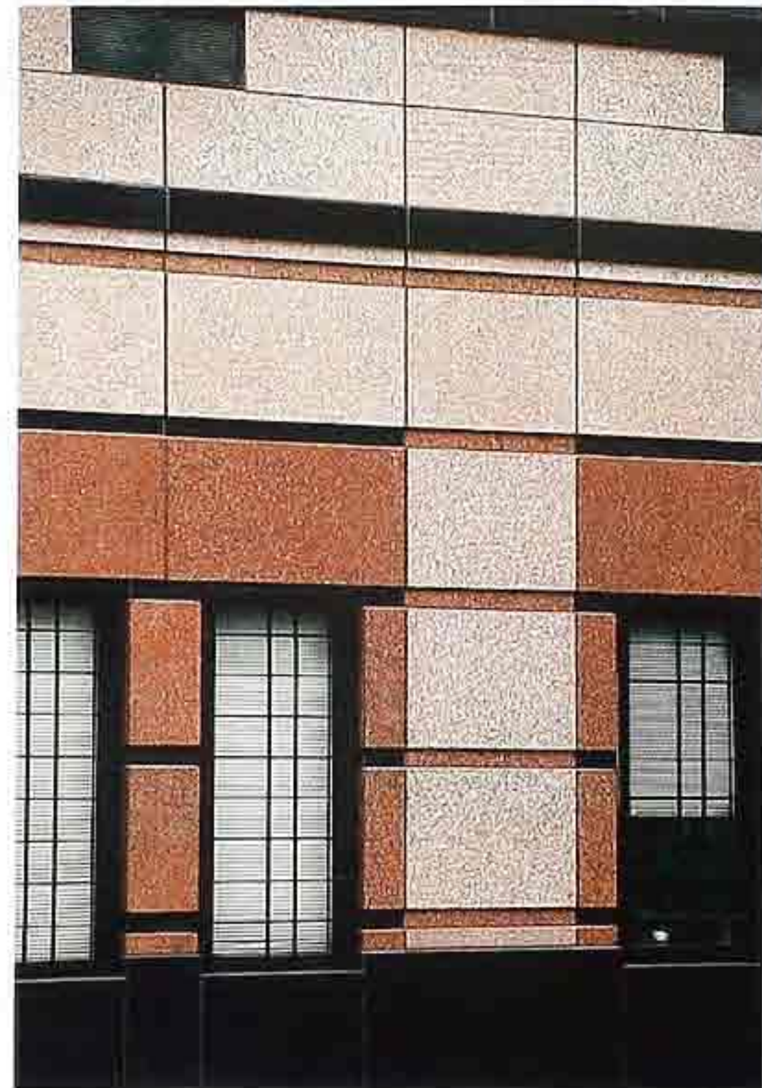
WA-146 Honed granite in stack bond with polychrome bands, modern apartment house
