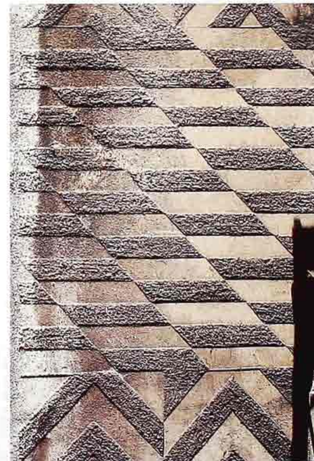
WA-219 Pre-cast textured concrete with chevron and diaper patterns
