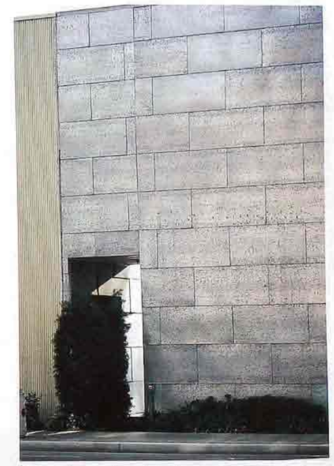
FA-16 Galvanized metal cladding in running-bond pattern
