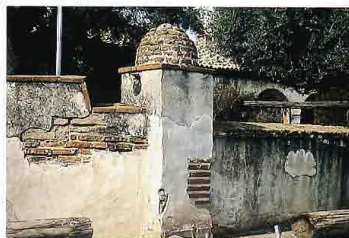
WA-259 Weathered whitewashed mud-stucco over exposed adobe brick courtyard wall, American Southwestern mission
