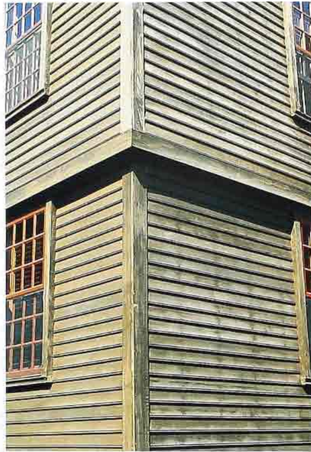
WA-37 Painted colonial clapboard house with wide corner board and a jetty between the first and second stories
