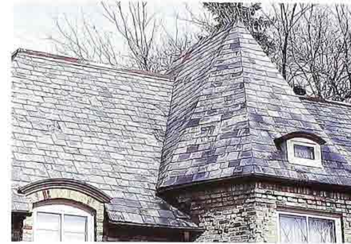
CR-58 Variegated slate roofing on hipped roof with pyramidal wall dormer, American house
