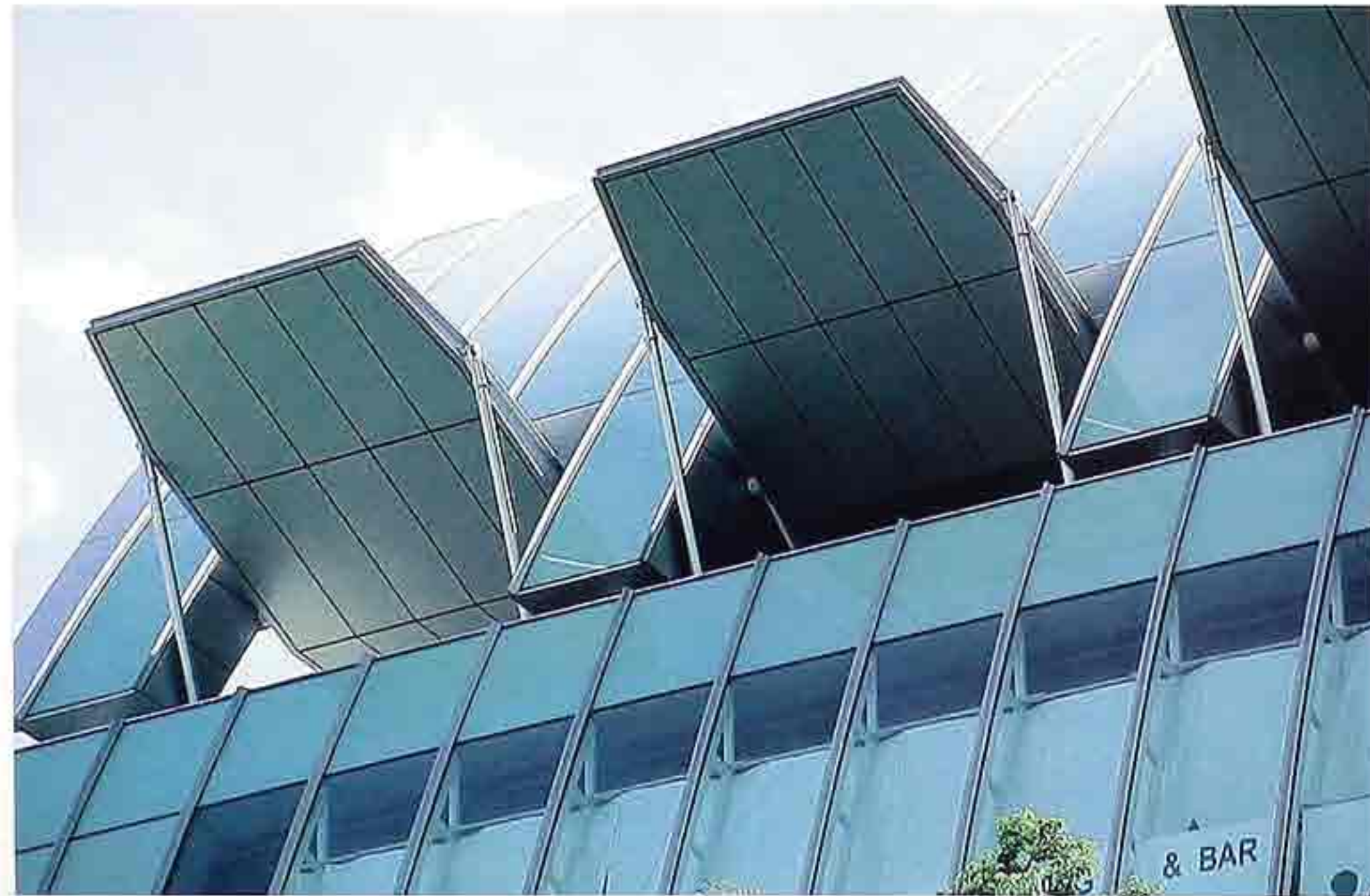
WI-204 Skylight shutters, modern commercial building
