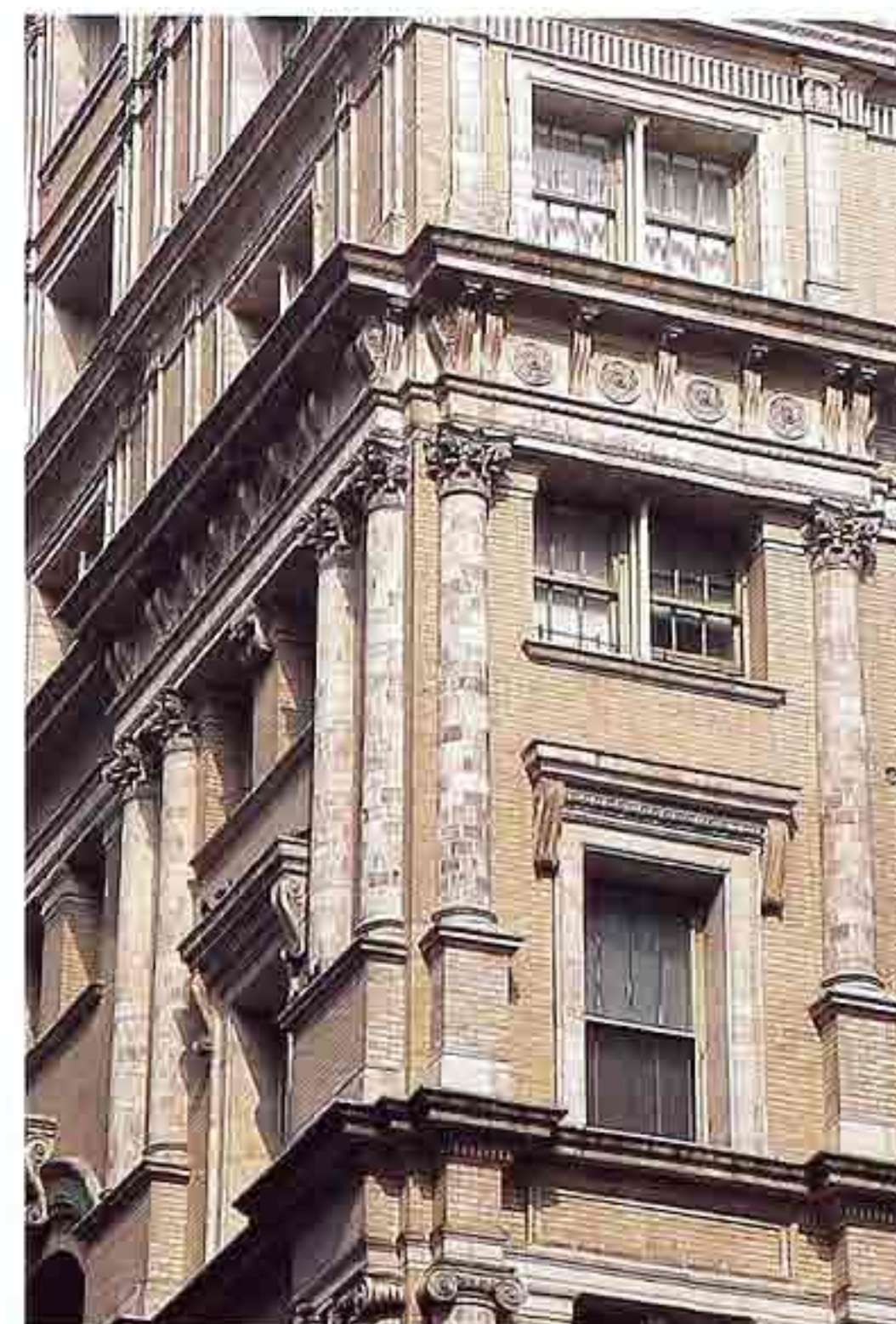
CP-92 Corinthian engaged columns
