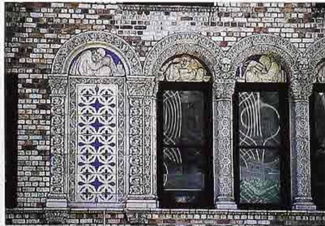
WI-144 Framed bas-relief tympanums and ornamented pilasters around windows; blind-arch window with glazed tile
