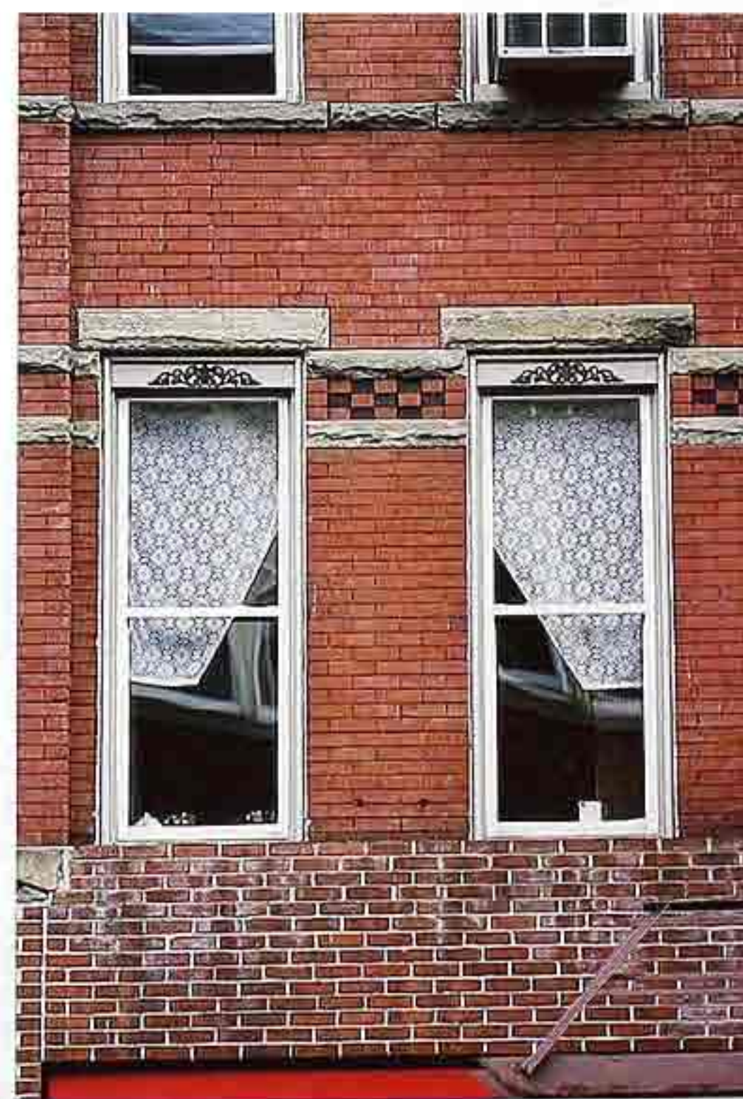
WI-124 Stone lintels and carved casing tops with stone and brickwork band around double-hung windows in brick wall
