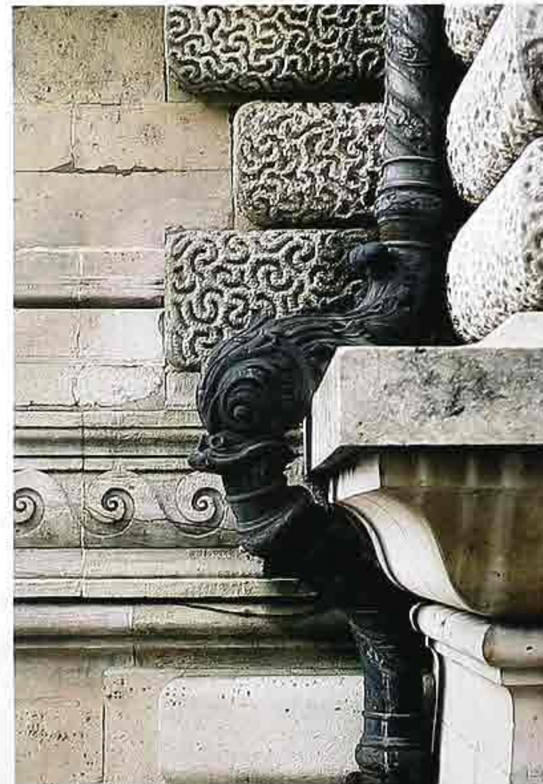
CR-158 Copper drainpipe and rainwater head
