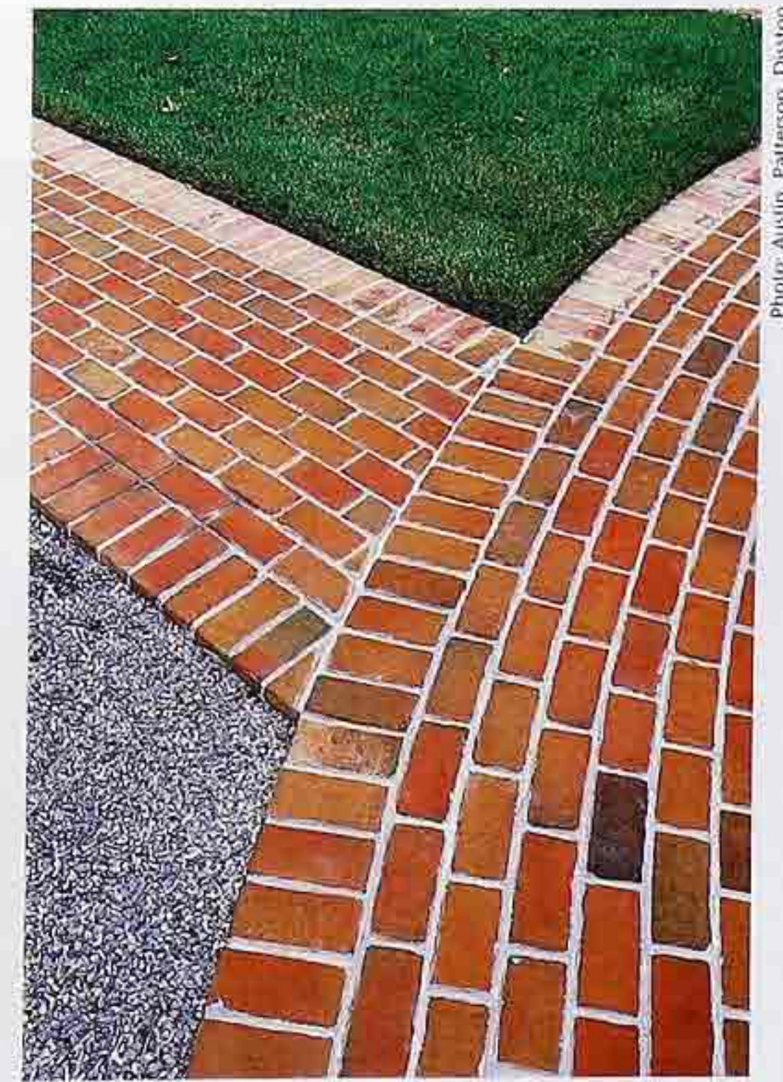
FP-64 Mortared brick in running bond, bordered by soldier courses in straight and curved paths intersecting with pebble path and grass, garden walk
