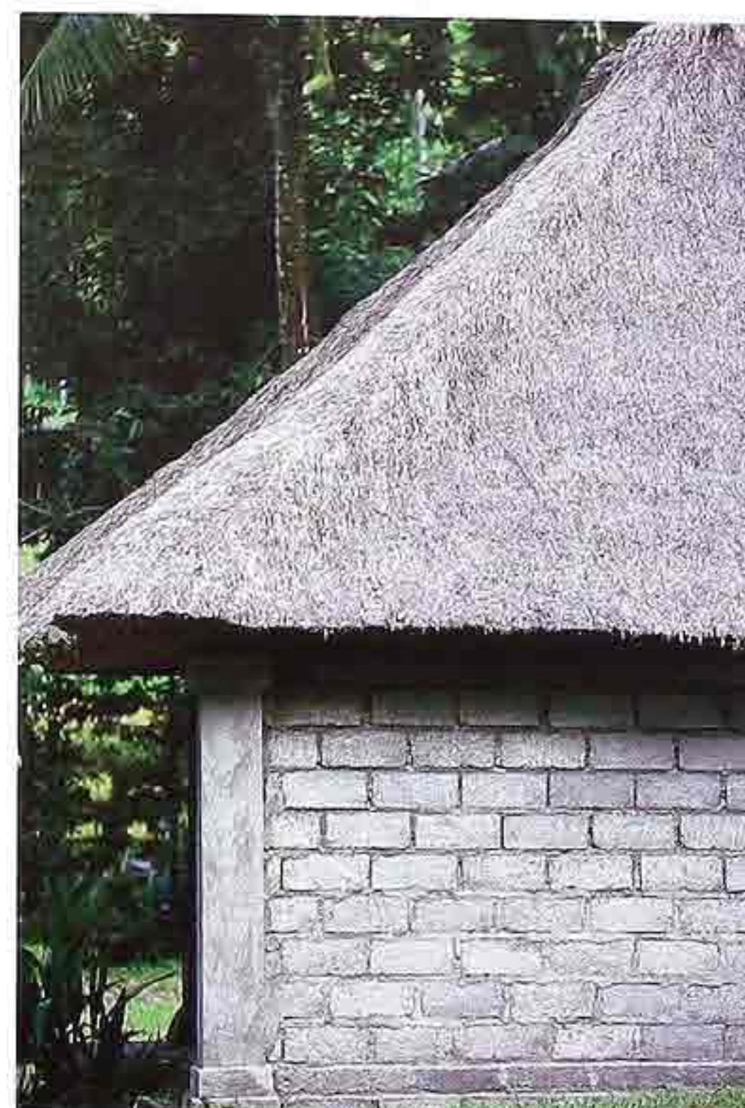
CR-70 Trimmed thatch on concrete-block building, Bali
