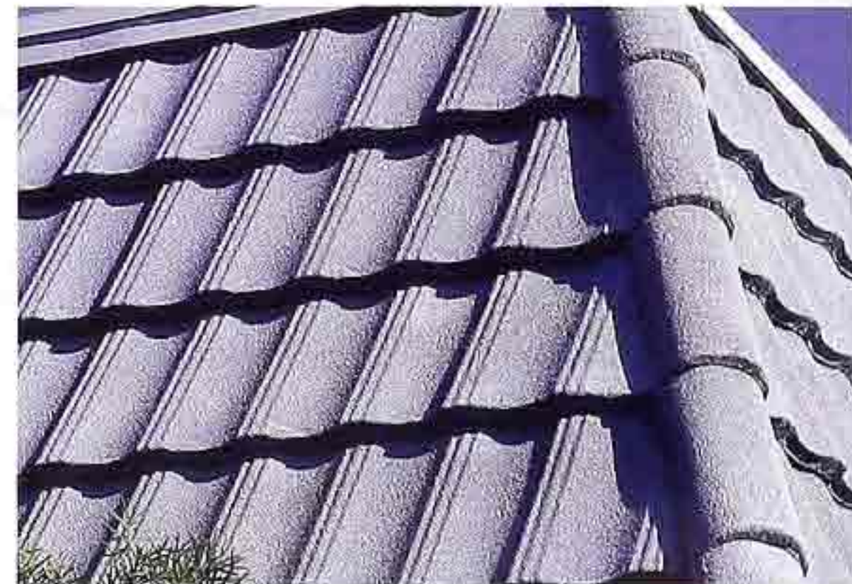
CR-47 Cast concrete pantiles on hipped roof with concrete ridge tiles on hip.
