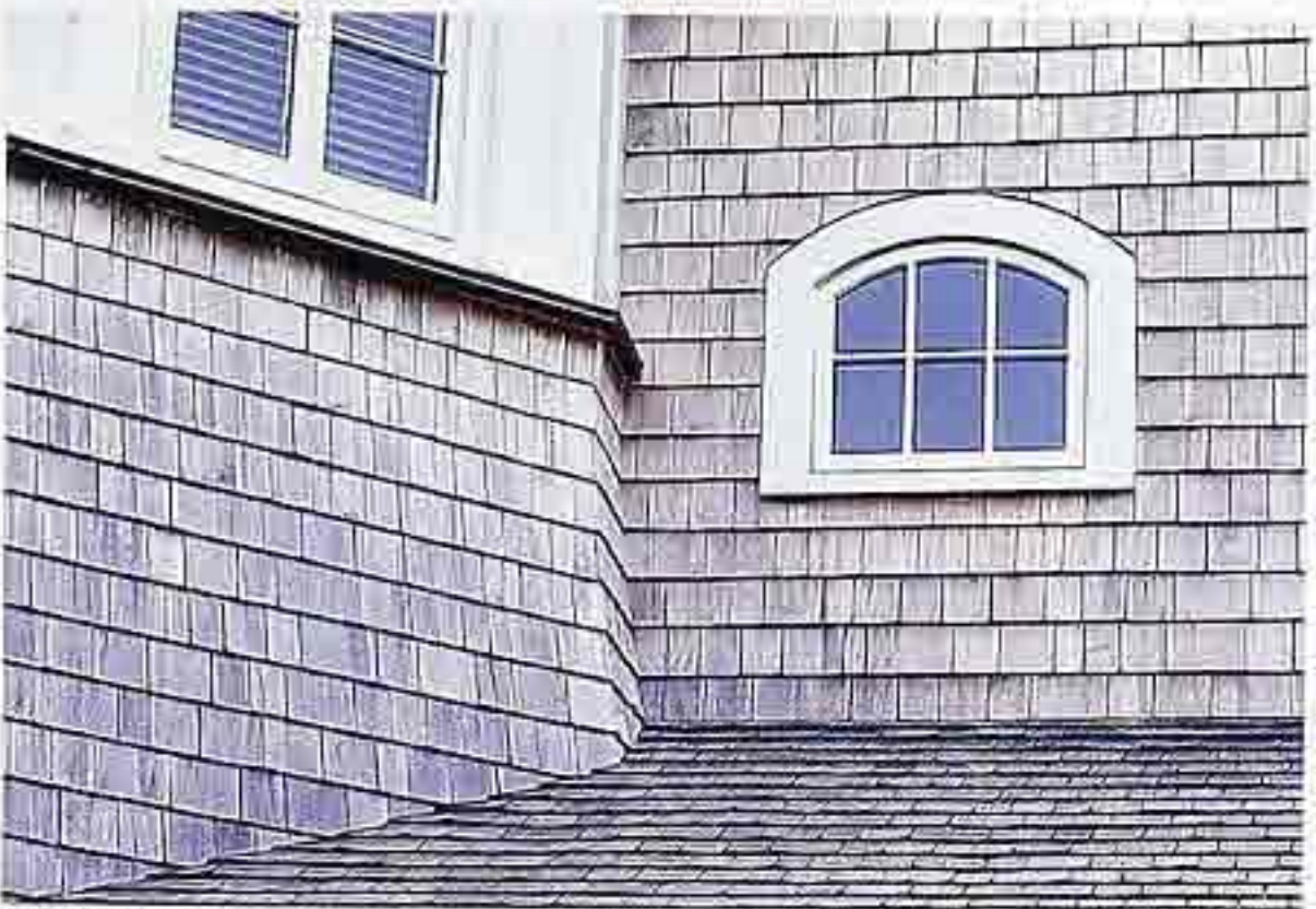
FA-49 Weathered Alaskan yellow cedar shakes in common coursing and segmental arch window, corner and roof detail
