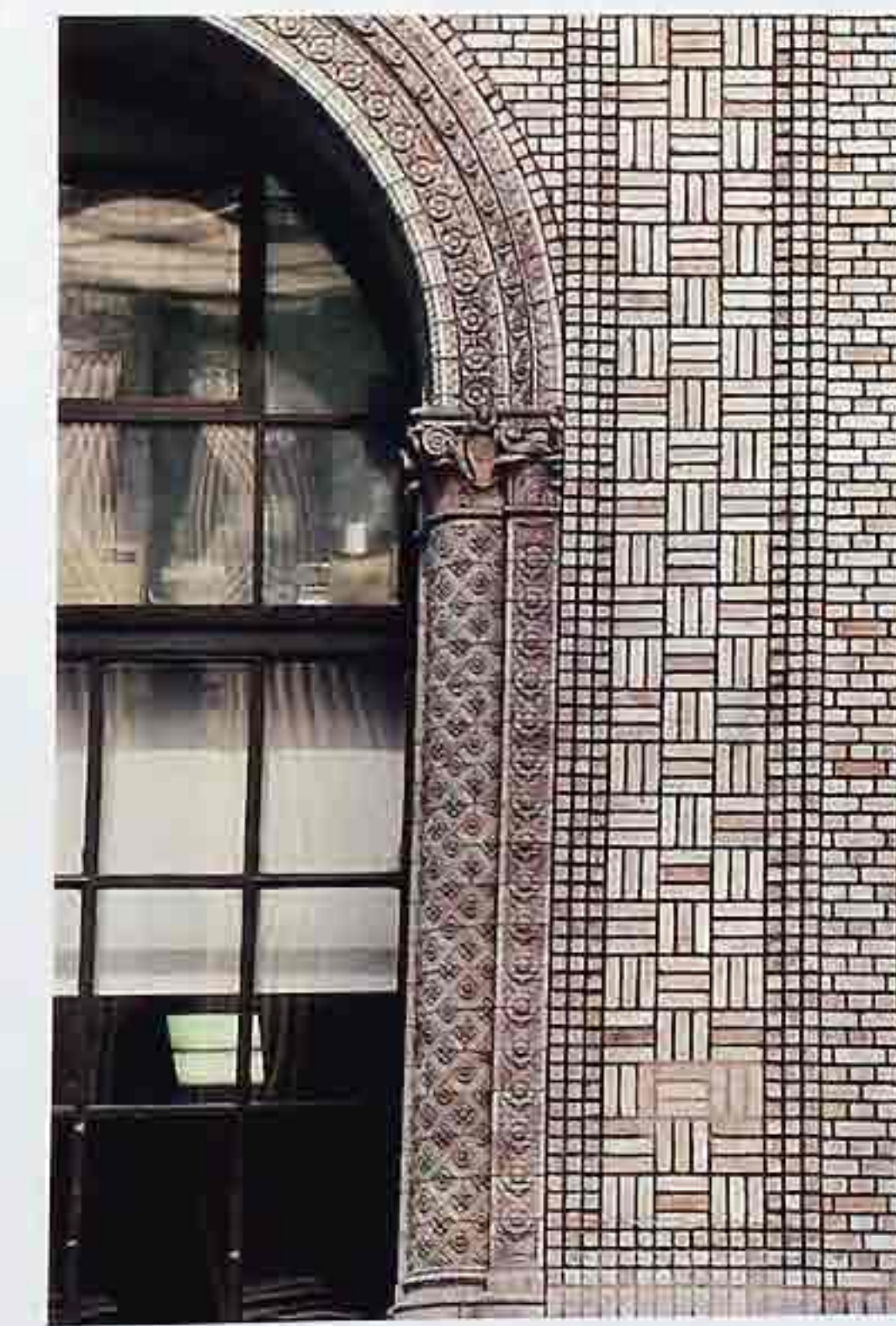
WA-204 Bands of decorative brickwork. Left to right: terracotta arch, stacked header rows, basket-weave, stacked header rows, English bond
