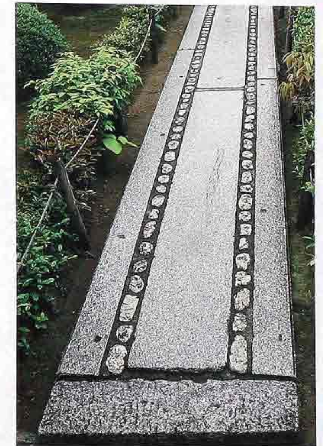
FP-48 Squared granite blocks with split-stone inset on garden path
