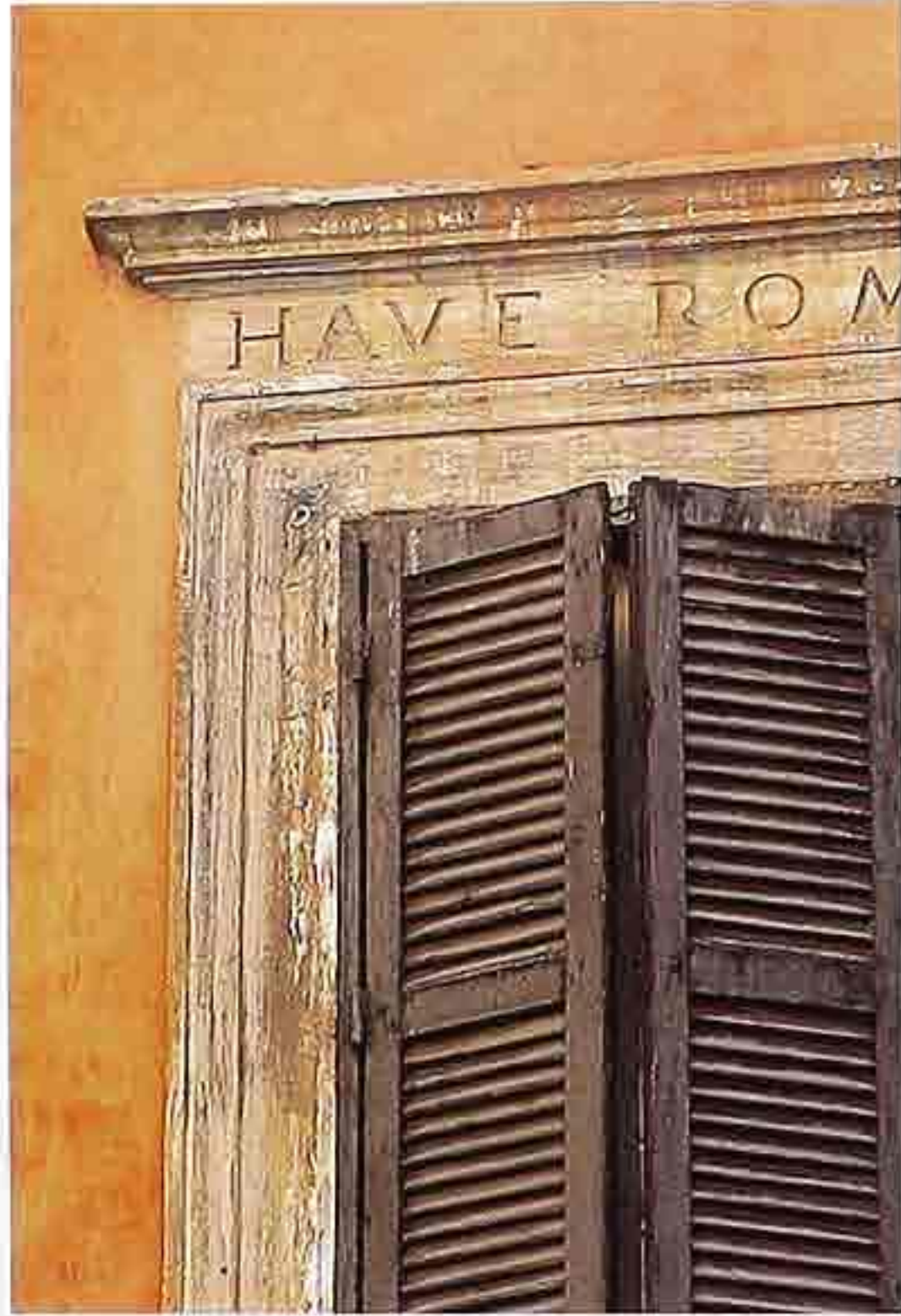
WI-132 Stone classical casing around shuttered window, old Roman building
