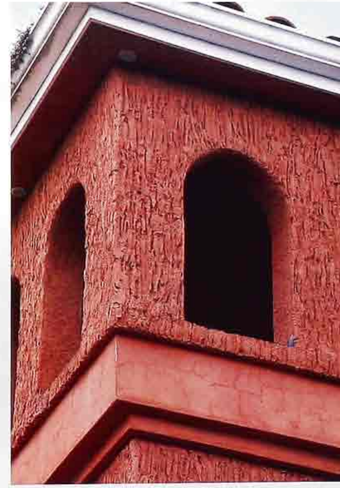
WA-236 Colored rough-troweled finish on stucco with smooth stucco band forming jetty, Italian-villa-style modern commercial building
