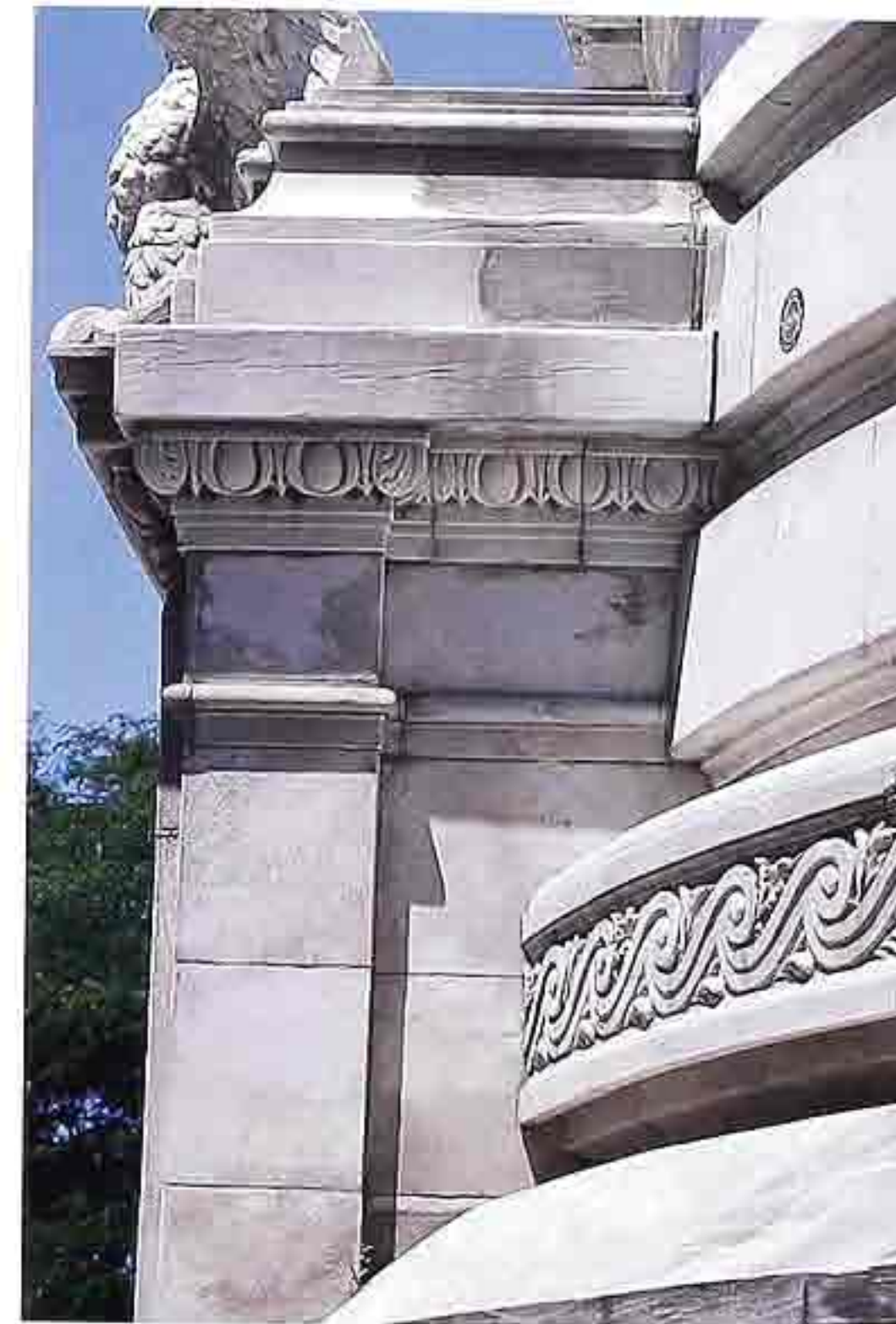
OM-63 Bottom right: Vitruvian scroll; upper left: egg-and-dart molding. Fascia above and below ornated molding
