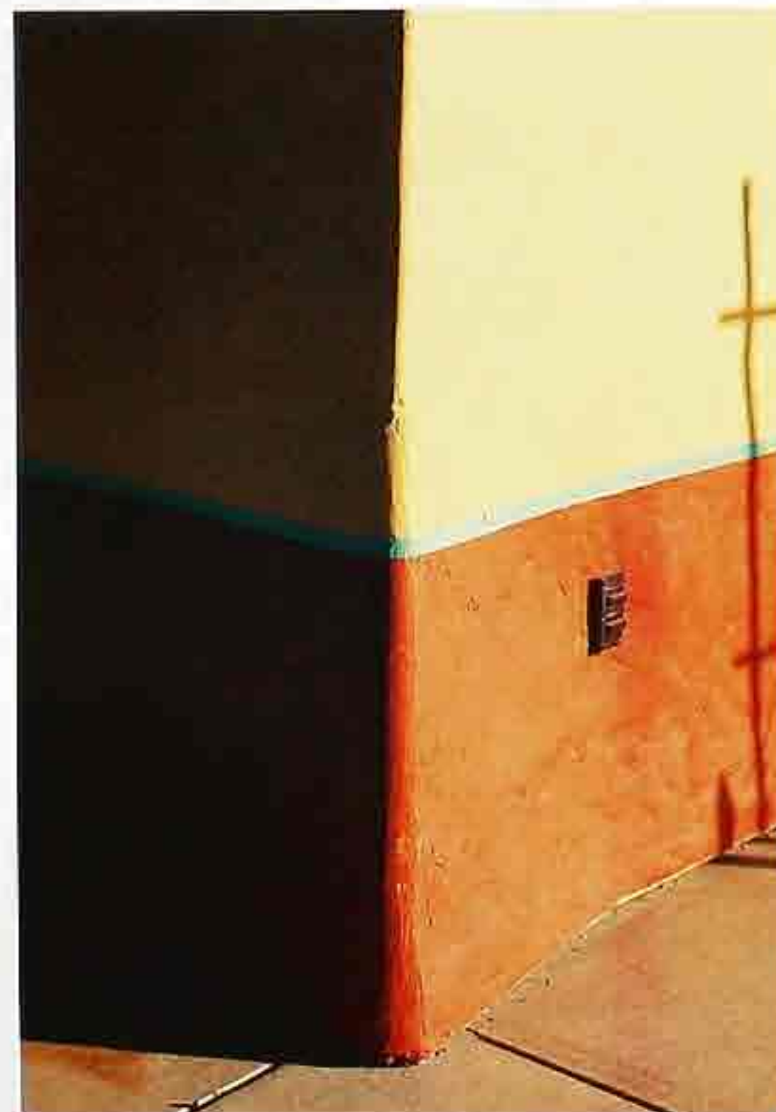
WA-232 Flared, rounded corner of smoothed painted stucco imitating a detail of traditional American Southwestern adobe house
