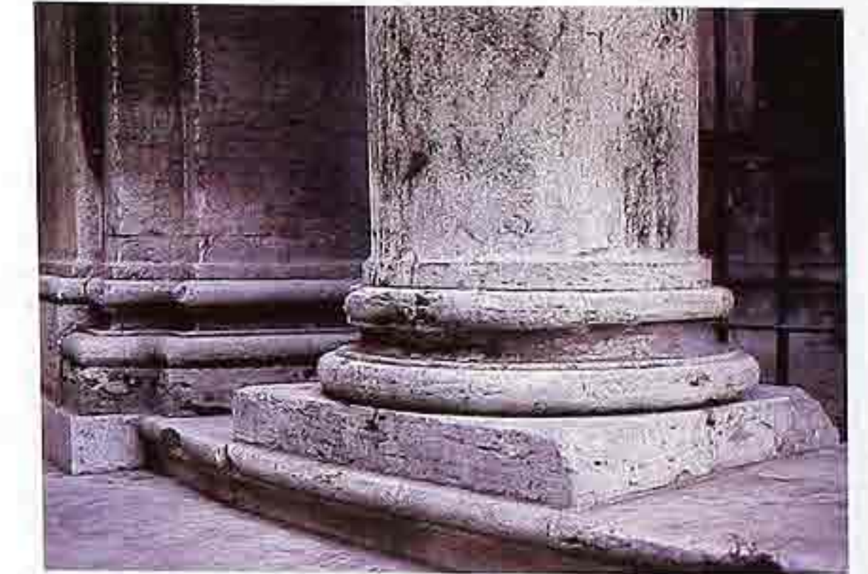
CP-36 Attic base of weathered travertine column on square plinth
