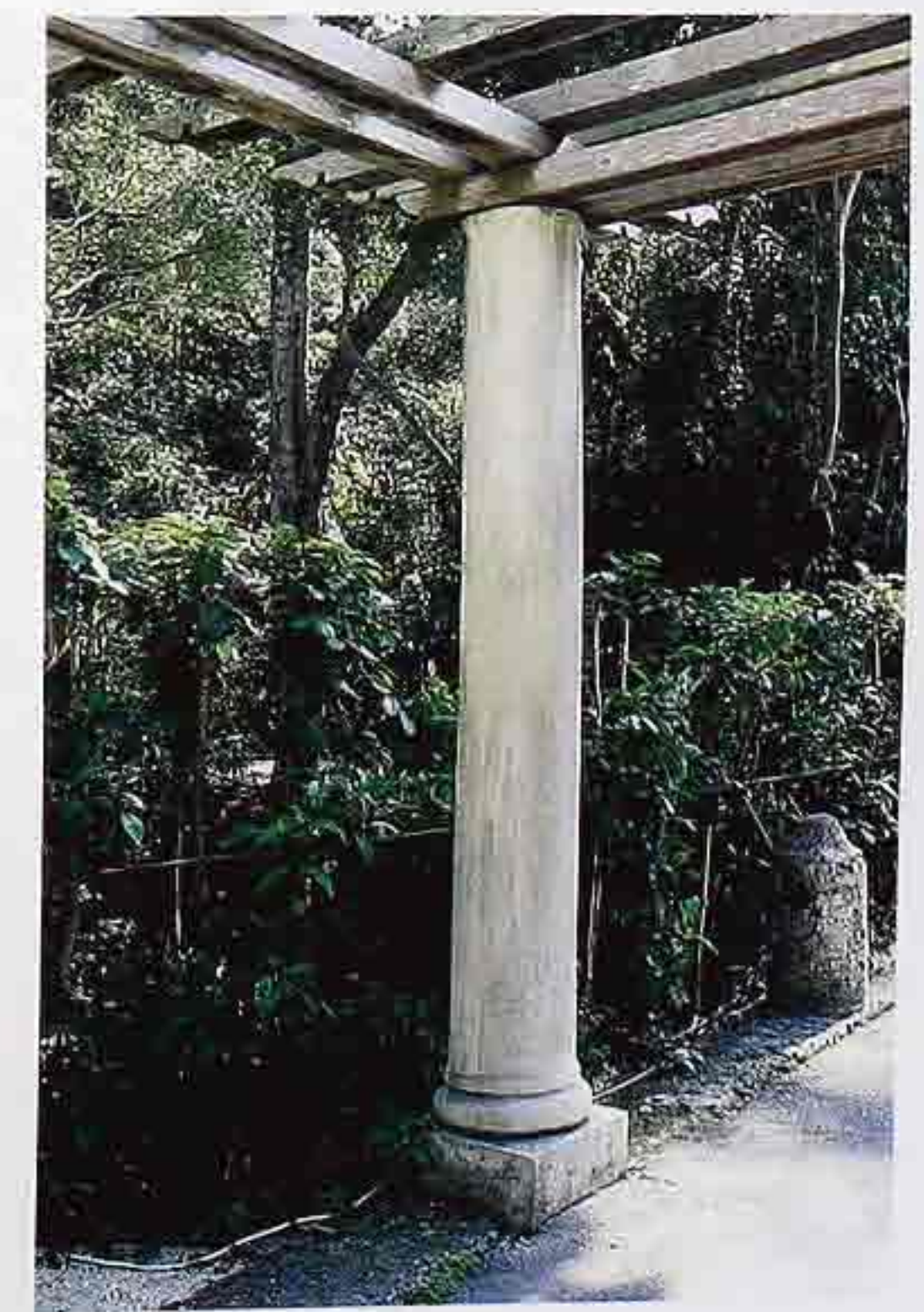
CP-137 Stone post with Attic base supporting wooden garden trellis
