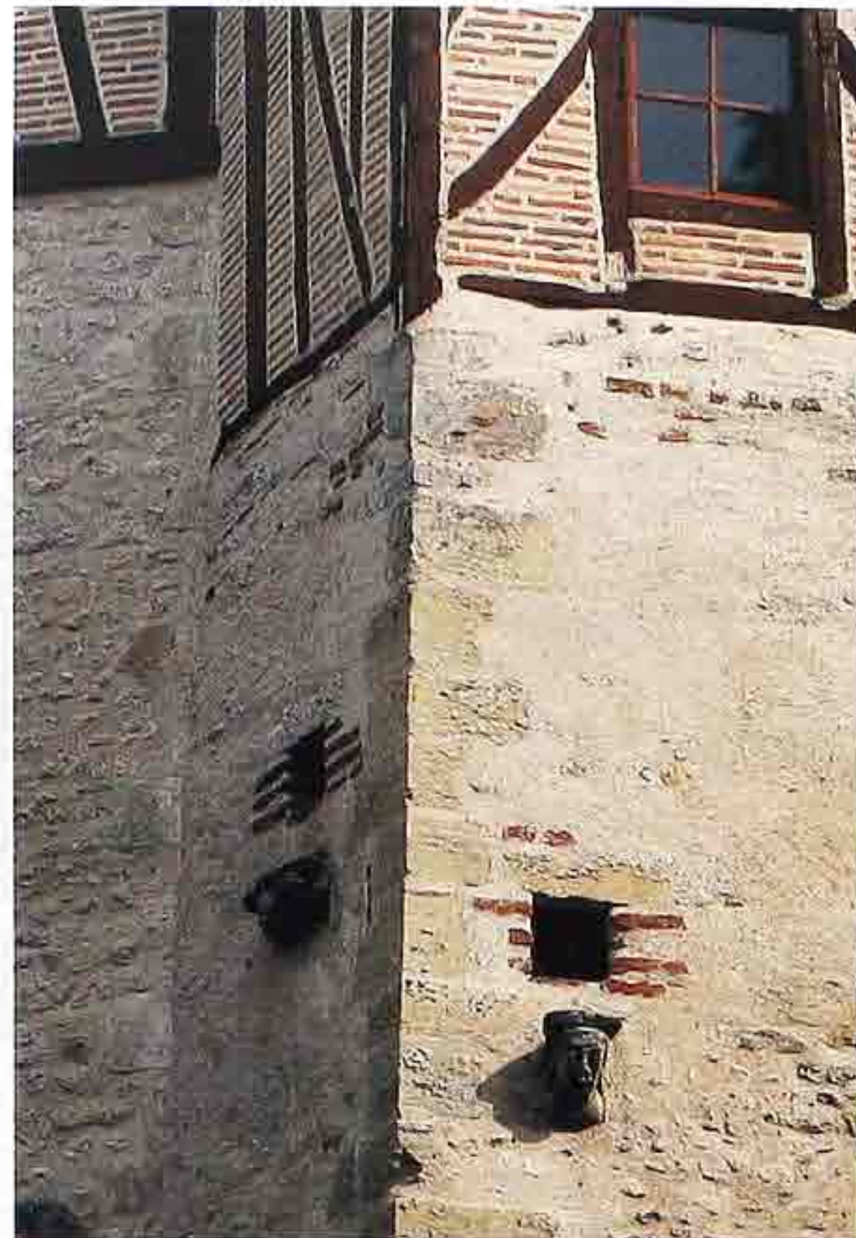
WA-291 Half-timber upper story with brick infill and stucco lower story with stone quoins
