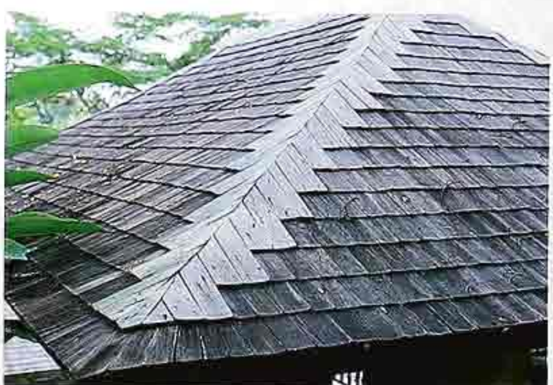
CR-69 Wood shingles on hipped roof with contrasting shingles along hip
