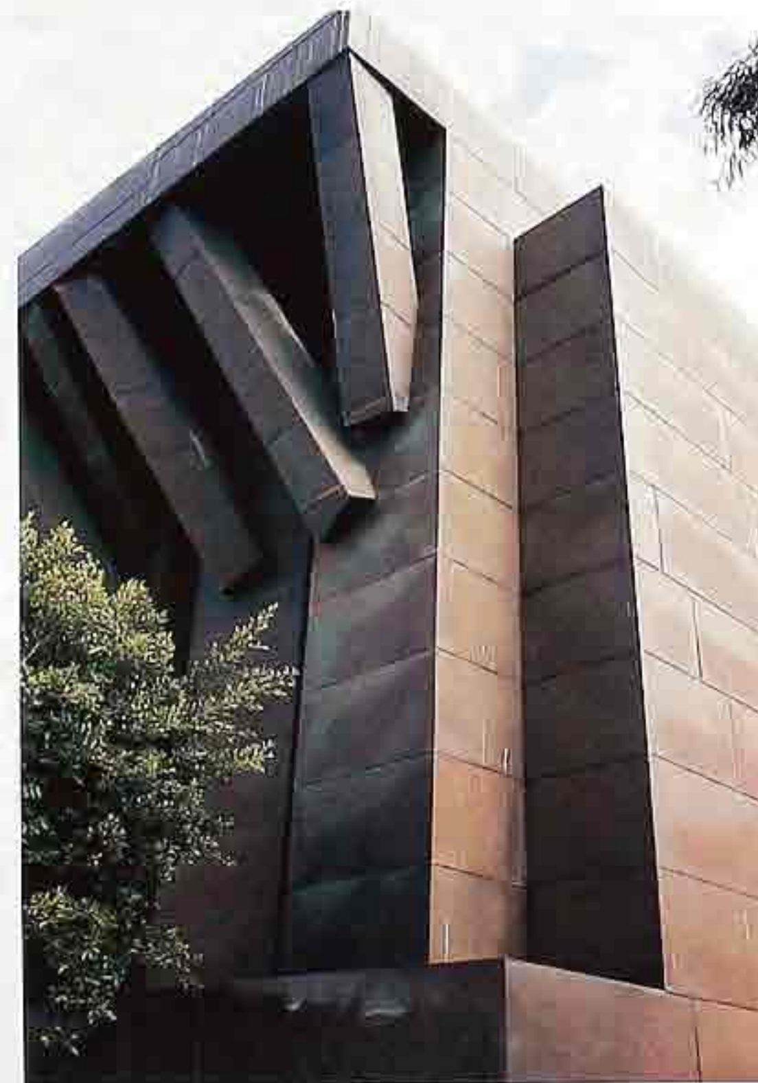
FA-13 Copper cladding, modern commercial building
