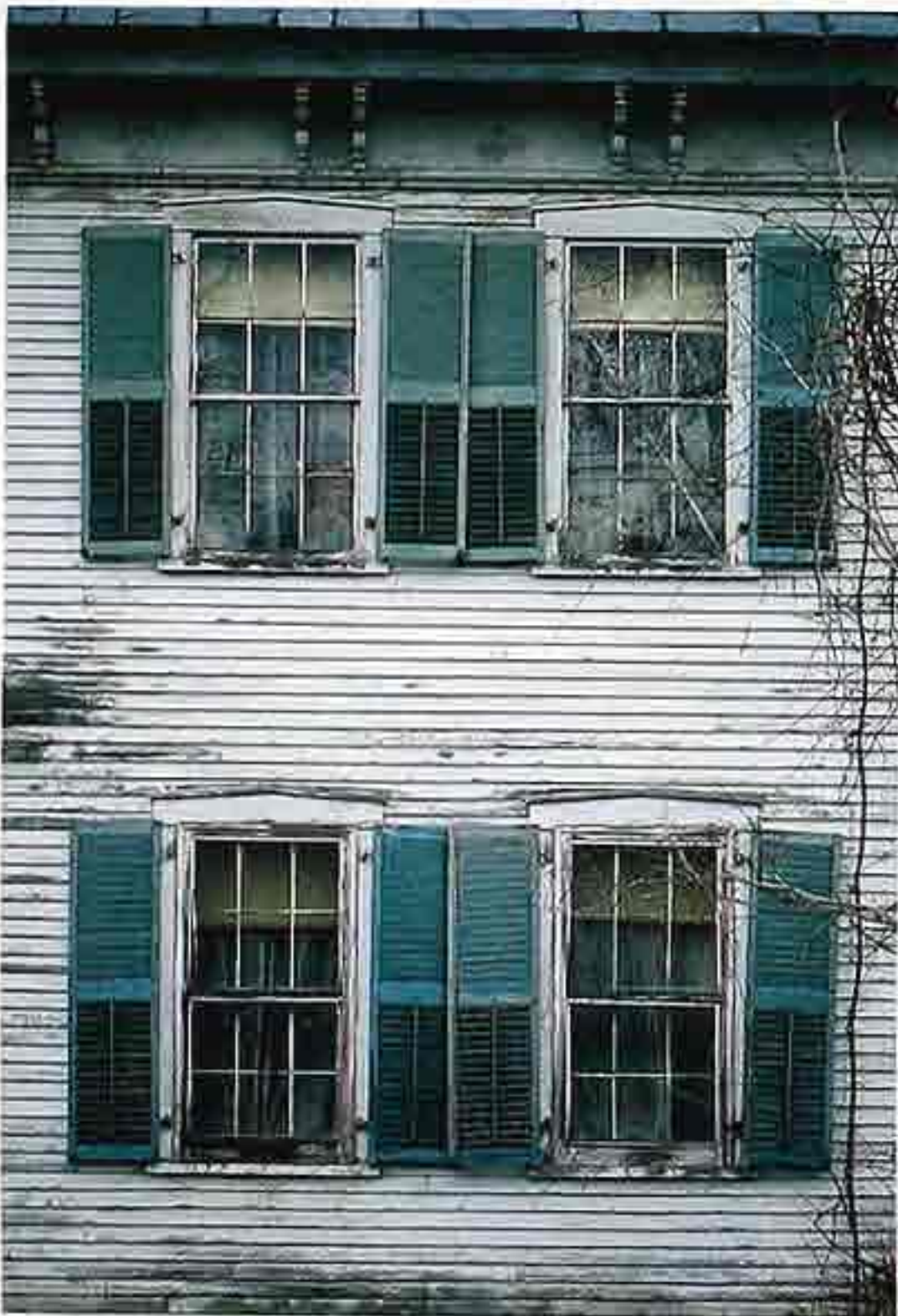
FA-94 Weathered painted clapboard facade
