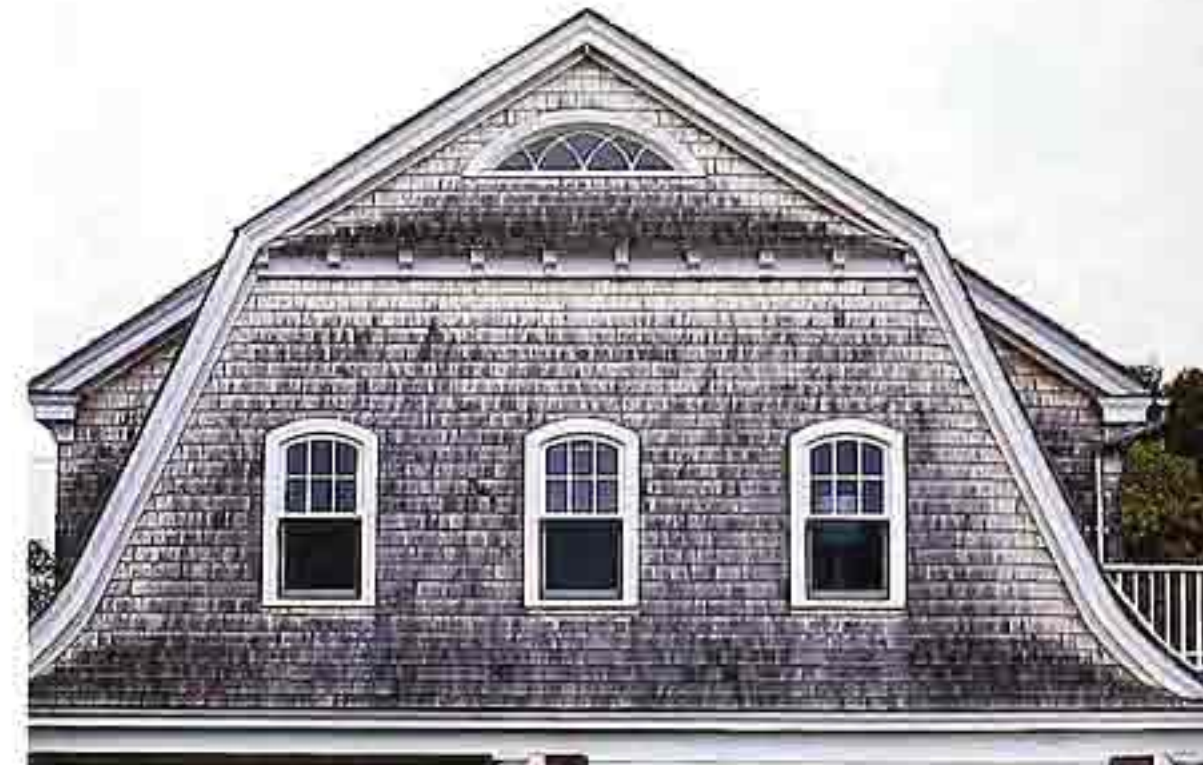
CR-96 Gable-end wall of flared gambrel roof with white cedar shingles; corbelled tie spanning gable
