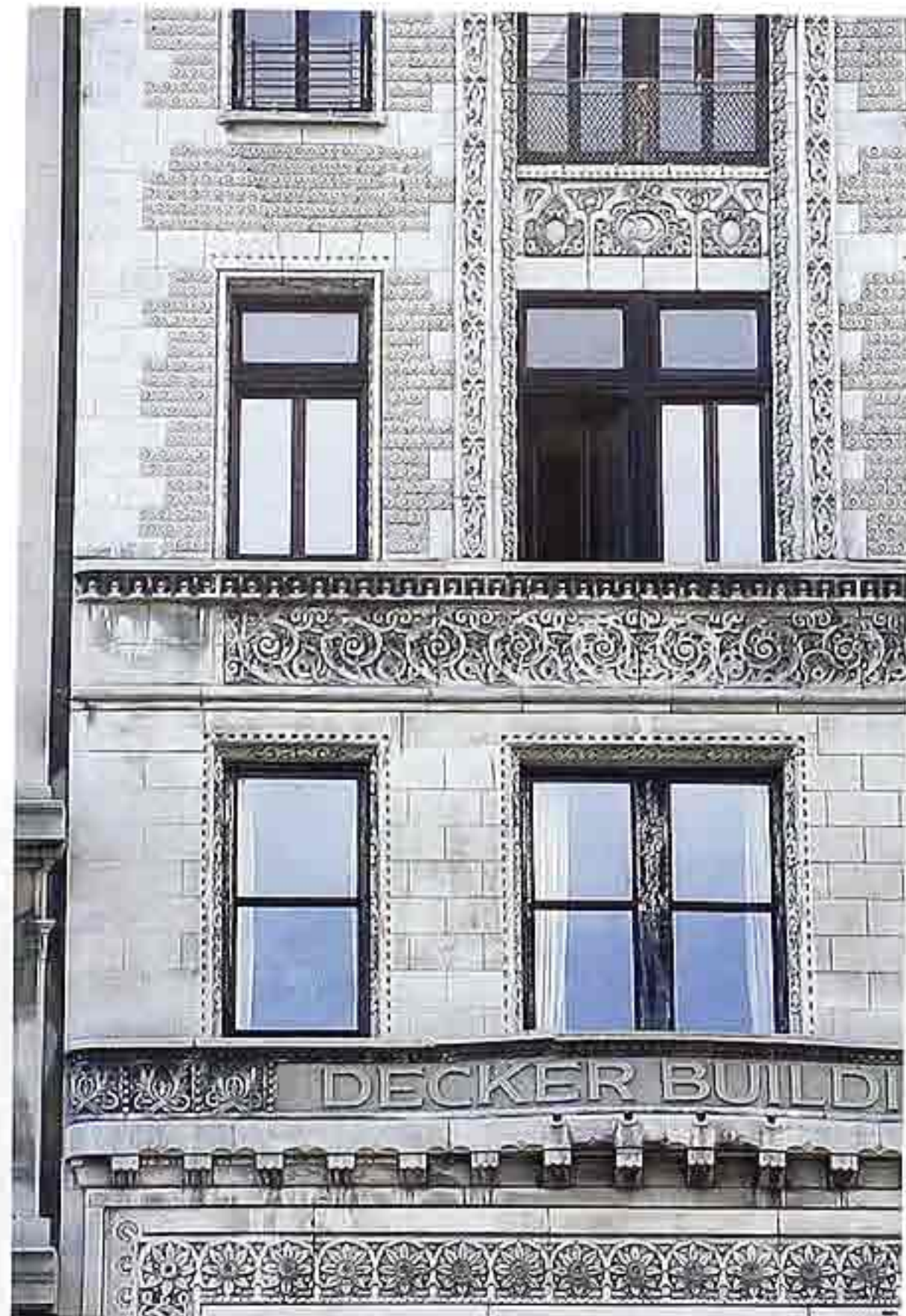
FA-112 Molded cornices and window surrounds with running ornament on multistory masonry facade
