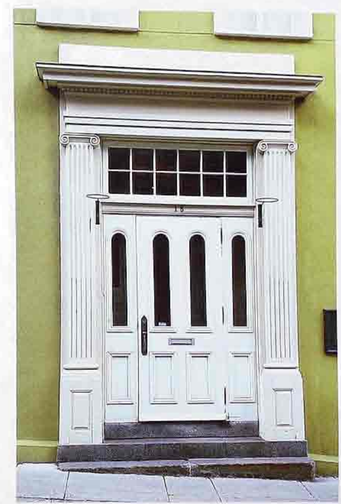
DW-70 Paneled double doors and side lights with lancet-shaped lights and twelve-light transom; letter slot; ionic-style pilasters and entablature
