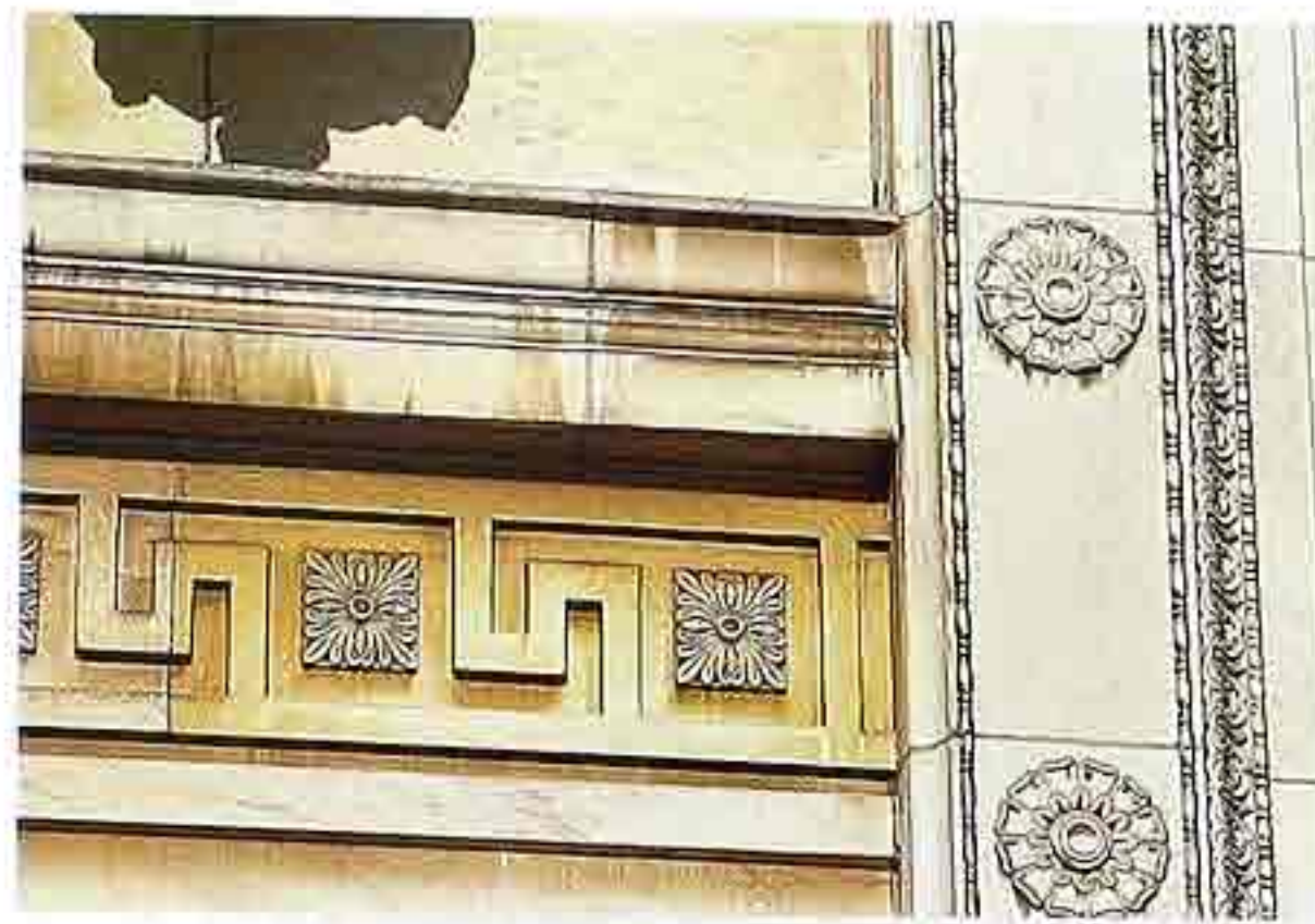
OM-57 Greek-key band with square floral element; jamb molding with rosettes framed by ornated ovolo molding
