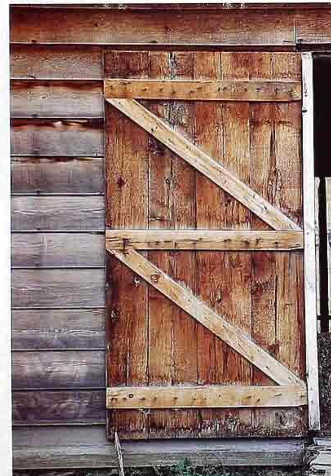
DW-25 Plain-sawn planks with double Z-brace, farm shed
