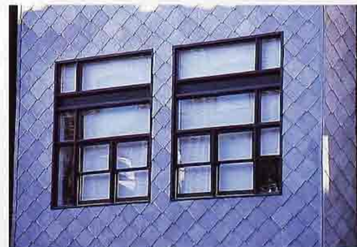
WI-102 Top to bottom: rectangular transom lights; fixed lights; pairs of one-over-one double-hung windows and fixed side lights, modern apartment house
