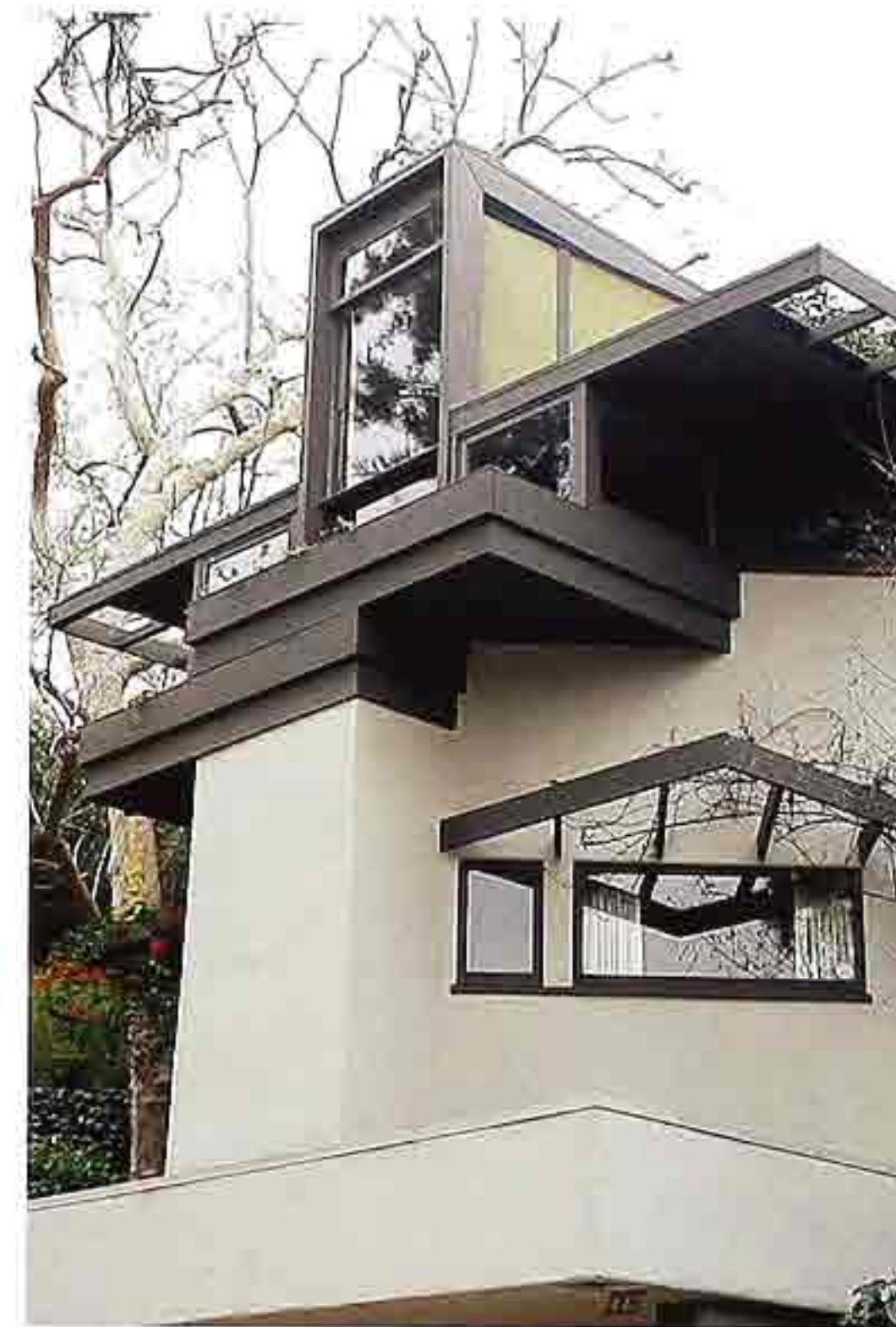
CR-109 Overhangs of multileveled flat roofs, modern house
