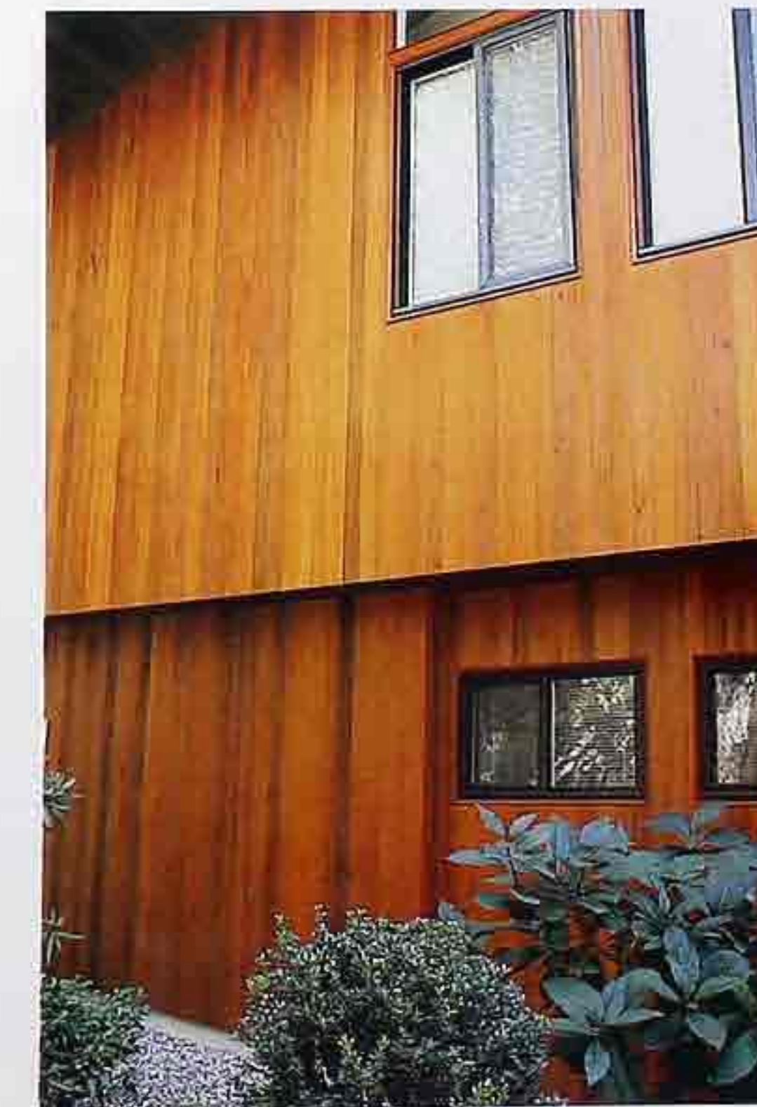
WA-50 Stained and sealed vertical siding with second-floor jetty and sliding metal-framed windows, modern house
