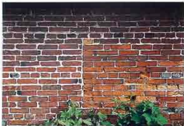
WA-153 Common bond, seventh-course header, in garden wall with repair
