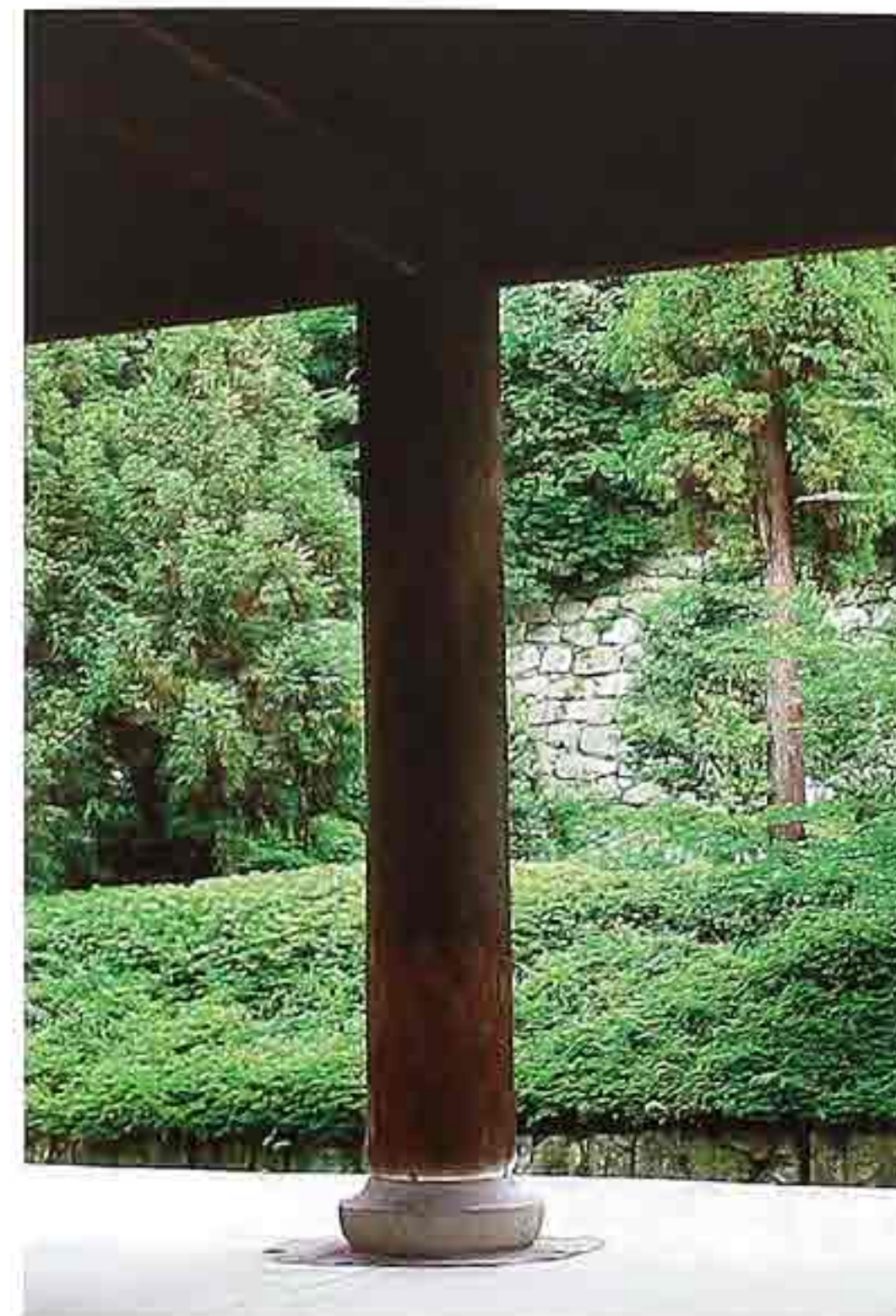
CP-134 Timber post on turned stone base supporting roof of veranda
