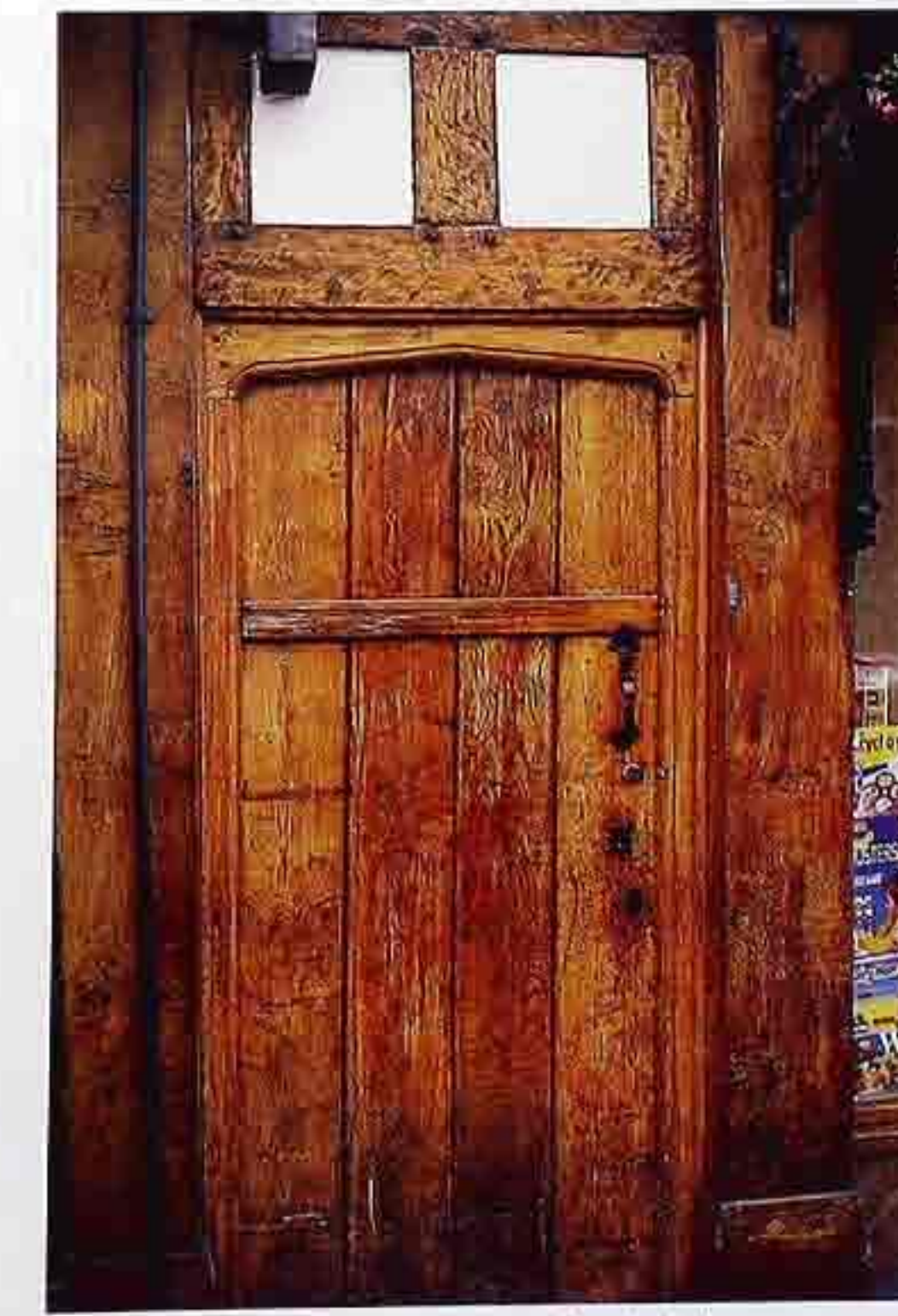
DW-36 Rustic wood-plank door with single brace, wrought-iron hardware, and two-paneled transom window; cambered arch; 16th- or 17th-c. England
