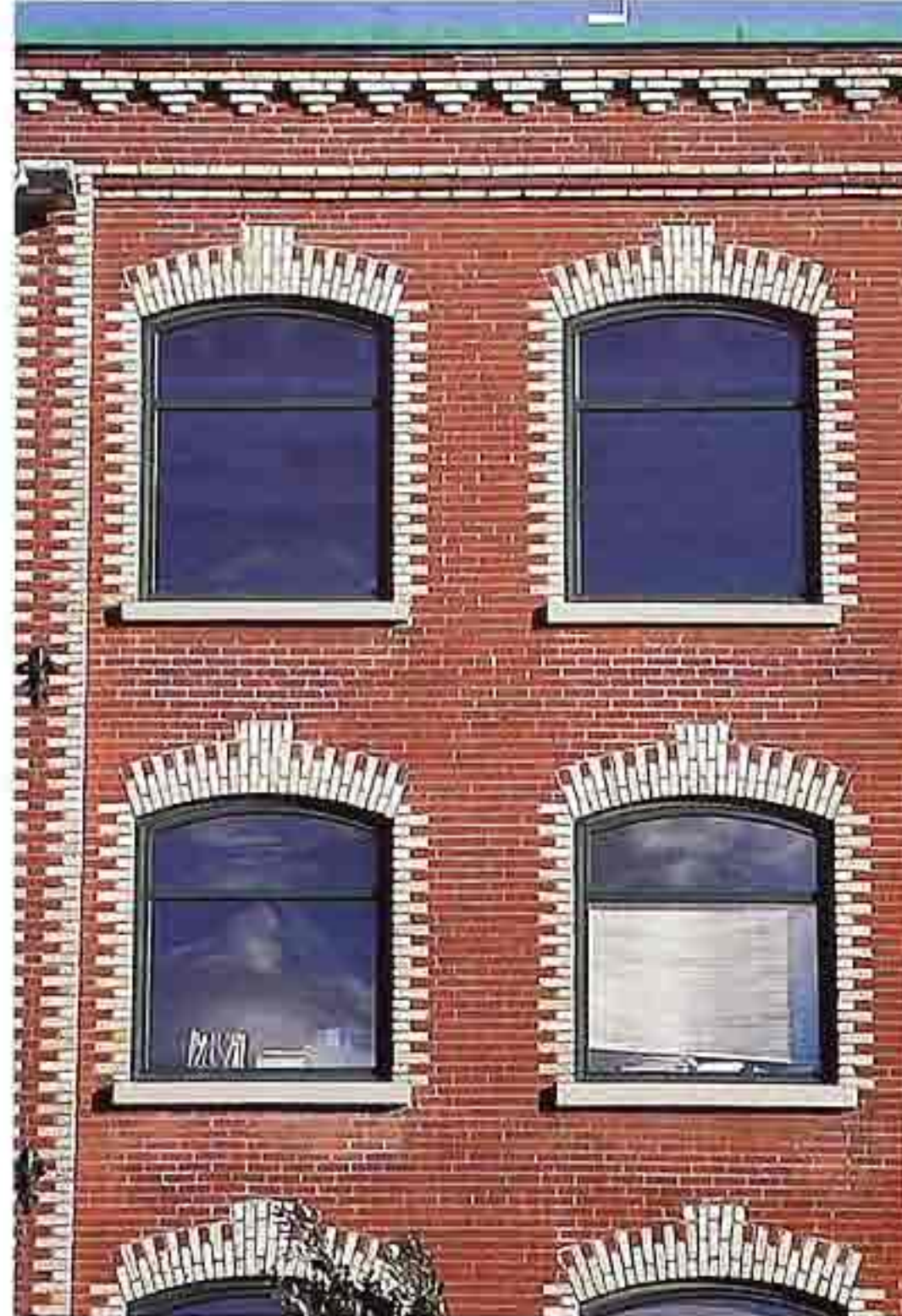
WI-119 Gauged-brick segmental-arch windows with brick quoins and "keystones" in contrasting color
