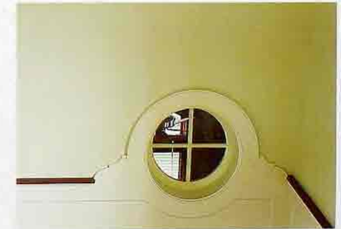
WI-62 Circular clerestory window divided by muntins, with a flat wood profiled frame, modern house
