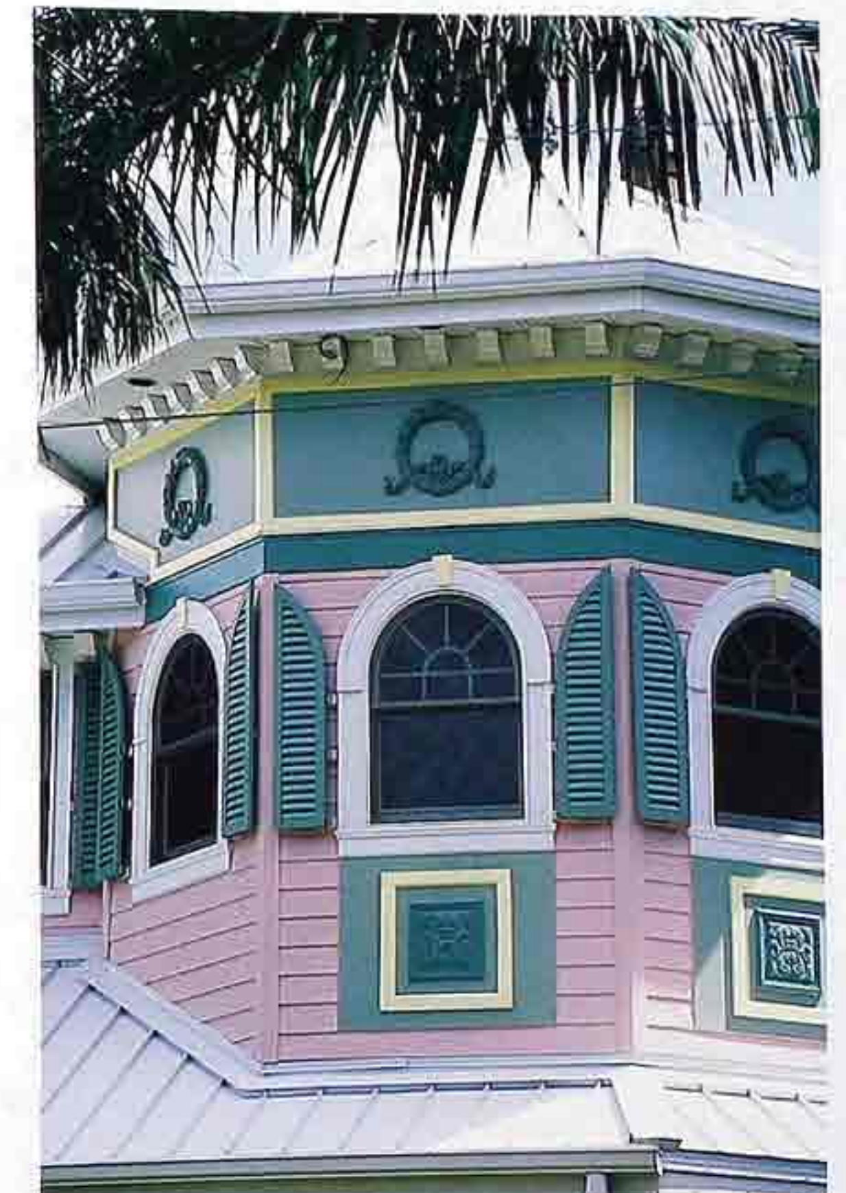
FA-80 Octagonal turret on contemporary polychrome house, modillion cornice, repeated ornament, and ornamental shutters around windows
