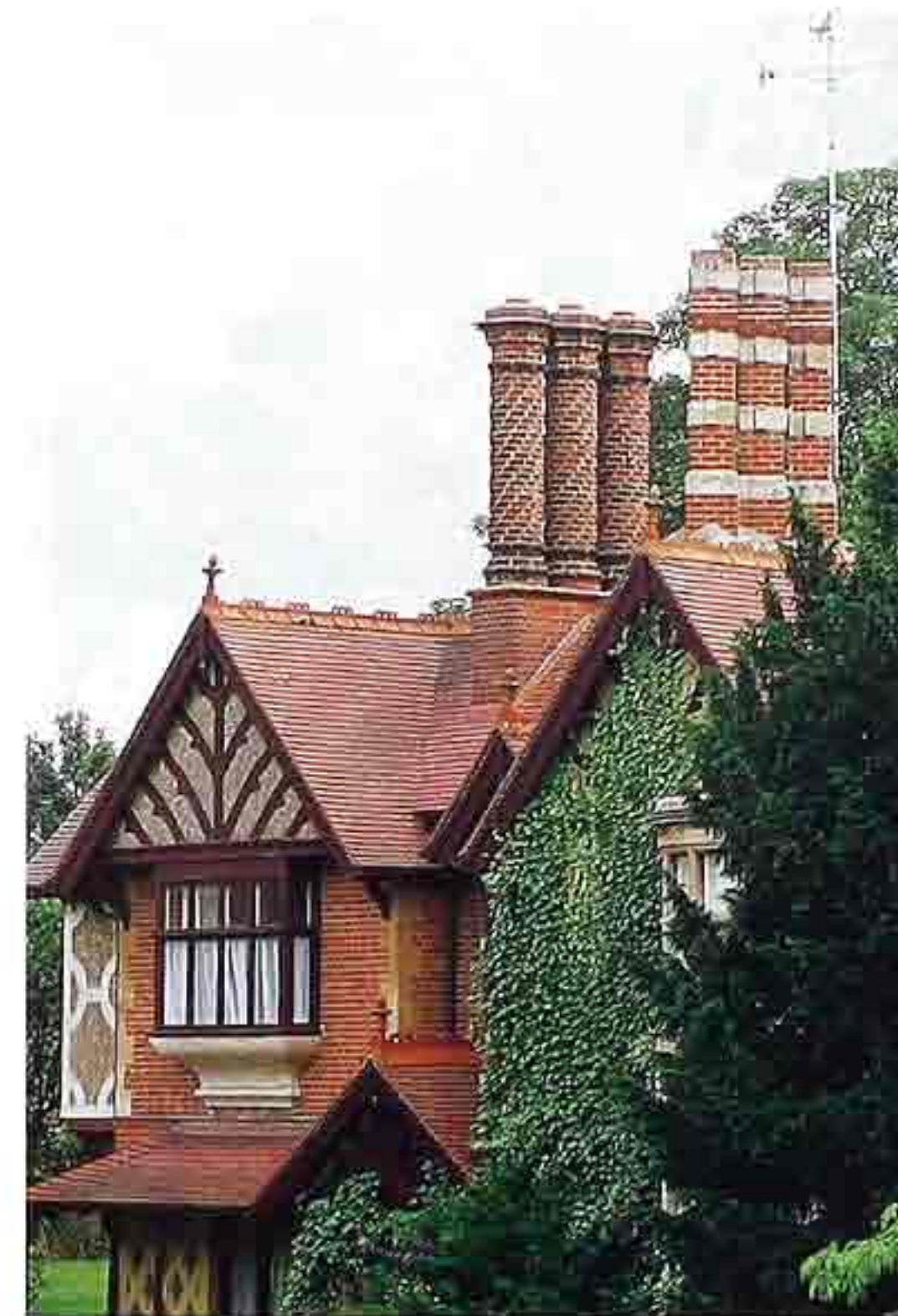
CR-143 Brick-pilaster chimneys: spiral (left); banded (right)
