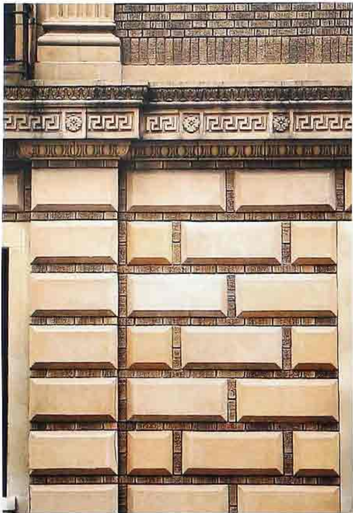
WA-290 Rusticated stone blocks in running bond, surrounded by brick; egg-and-dart pilaster cap and molding, with relief ornament band between stories
