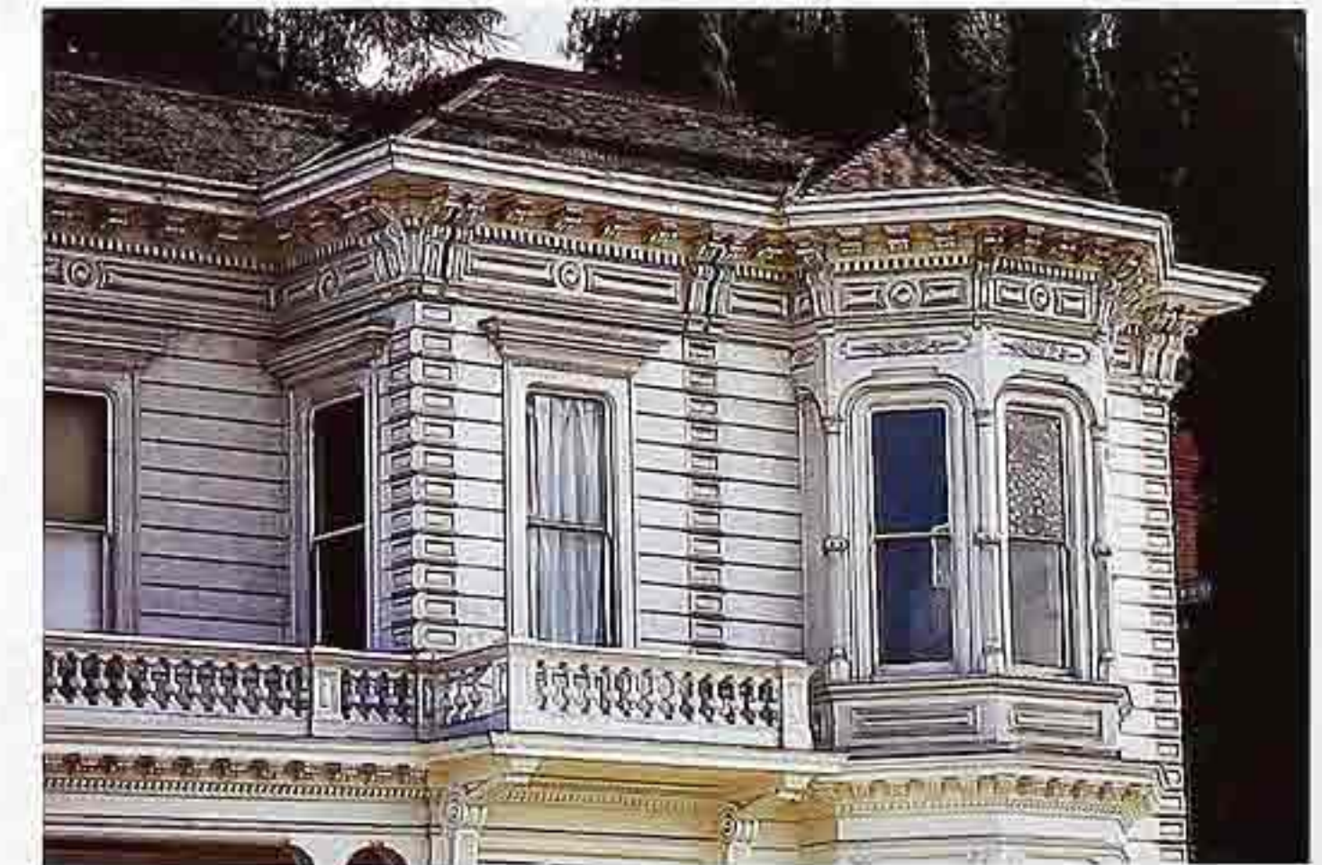
WI-116 Ornament, molding, and balustrade around double-hung windows in cant-bay and wall windows; 19th-c. American clapboard house
