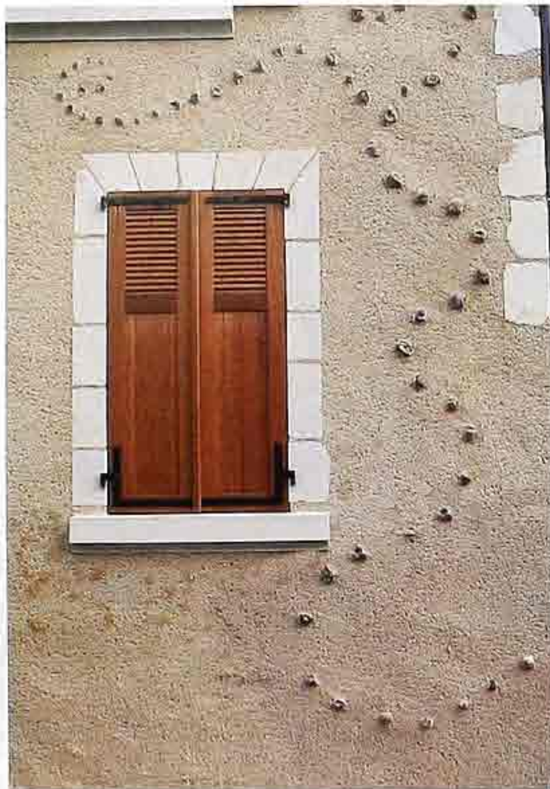
WA-230 Stucco with dimension-stone window and corner quoins and natural stone insets in serpentine design; louvered shutters, house
