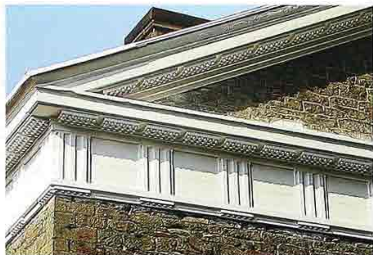
OM-86 Triglyphs with guttae alternating with plain metopes; mutules with guttae in the soffit
